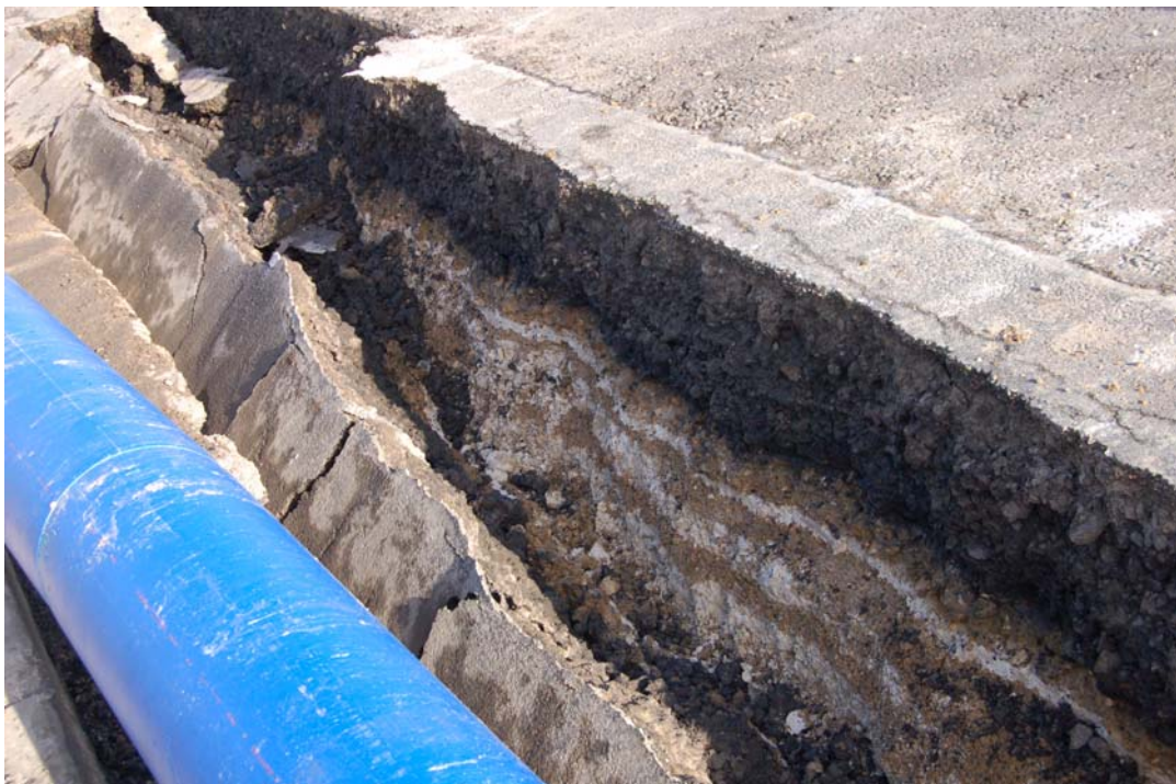
Plate 2. Detail of Causeway construction deposits
