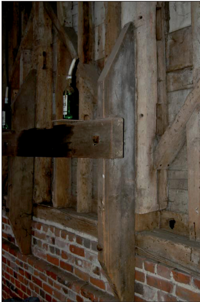
Plate 10 Bearing box bracket for former milling machinery
