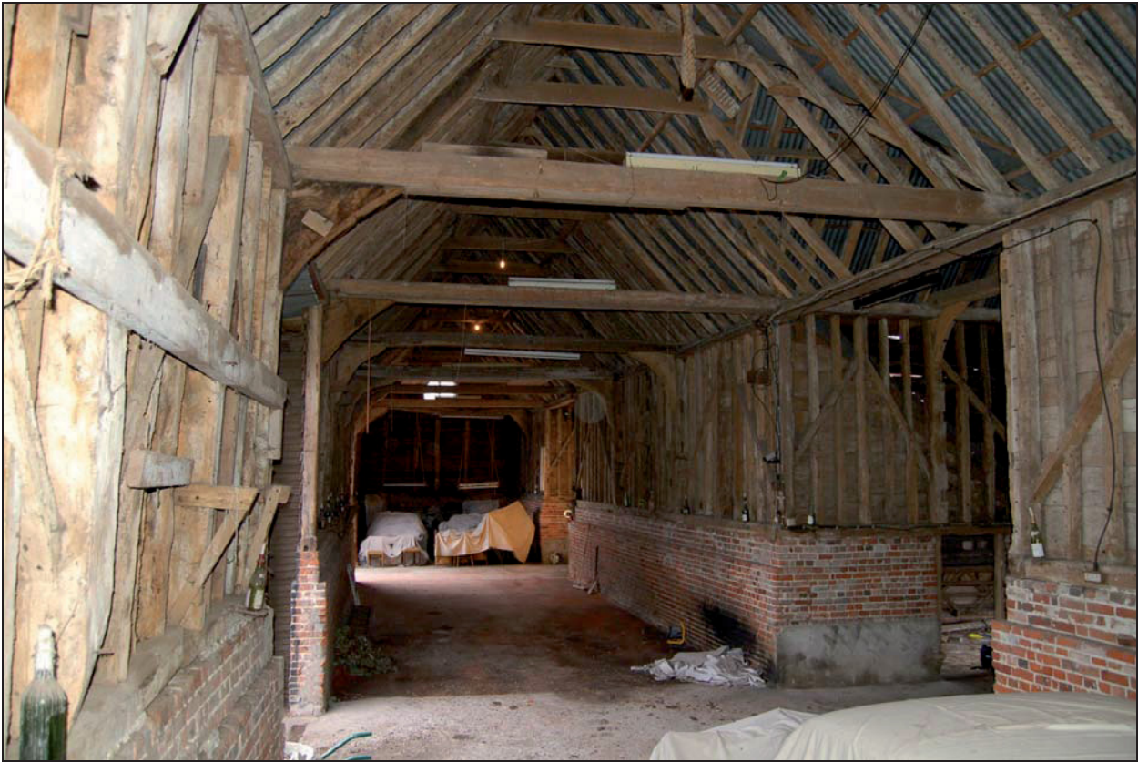
Plate 7 Interior of barn viewed to south
