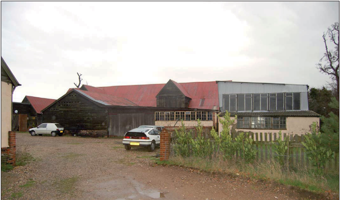
Plate 4 Modern additions to barn
