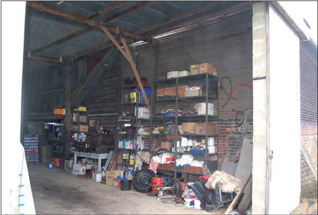
Plate 5 Rebuilt south wall of barn inside garage
