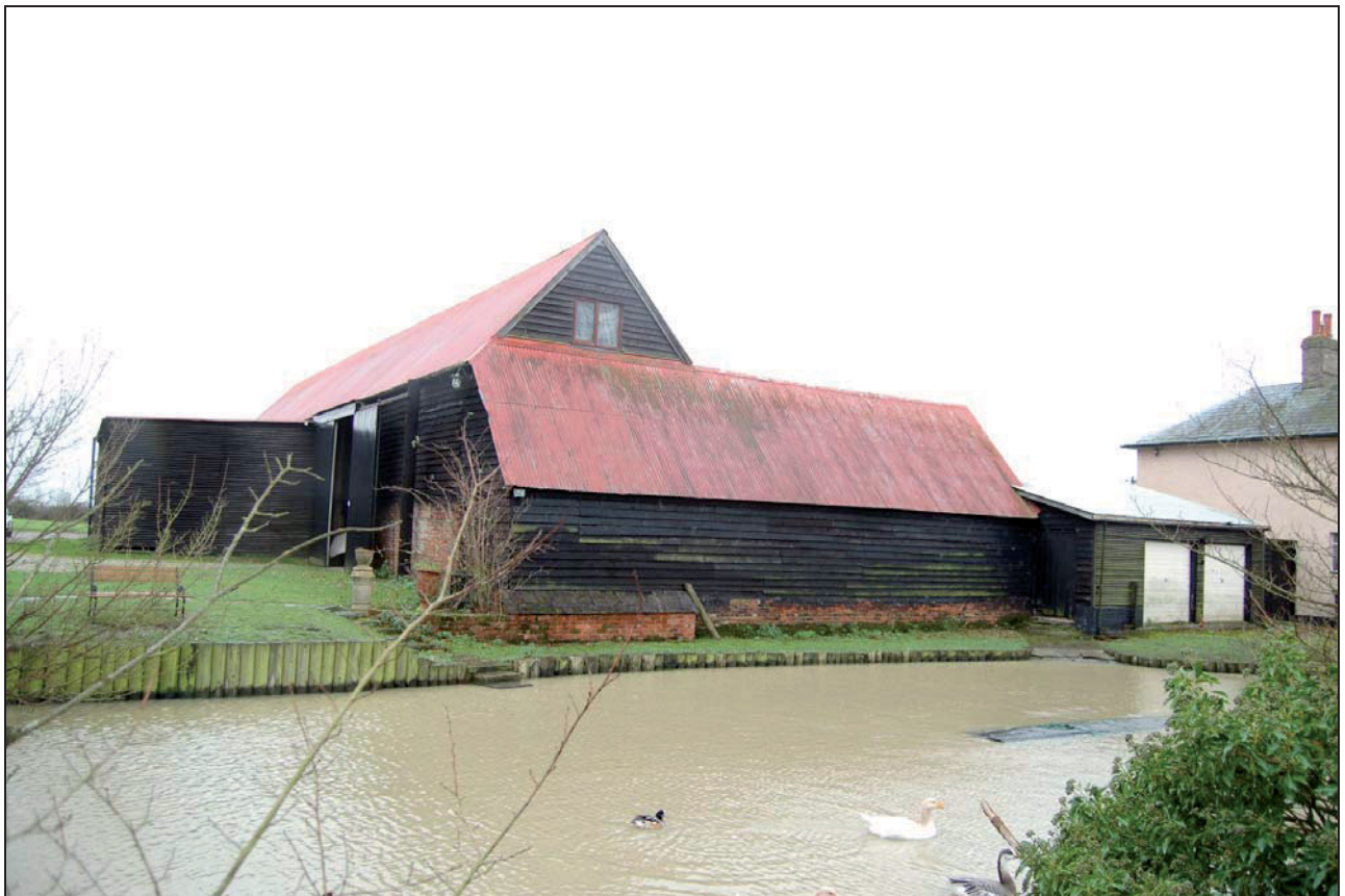
Plate 2 Barn, cowhouse and shed 7 viewed towards south
