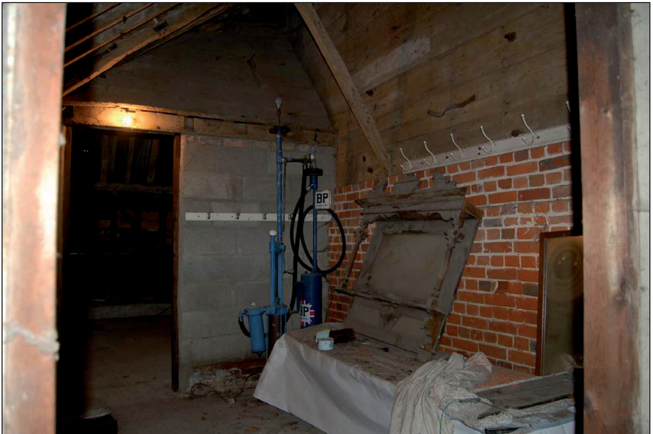
Plate 14 Interior of loose box 3a
