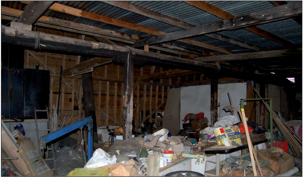
Plate 19 Southern side of shelter shed 4 from inside pole barn
