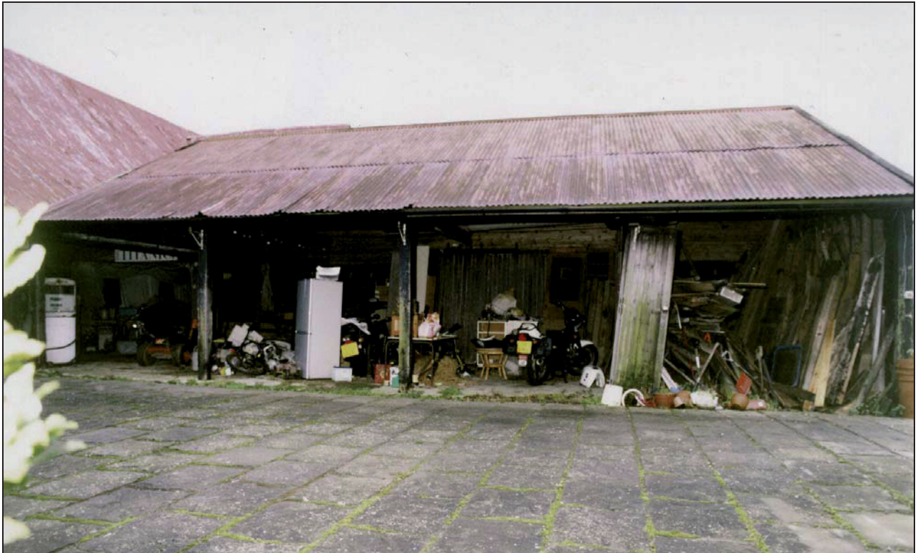
Plate 18 Shelter shed 4 viewed to south
