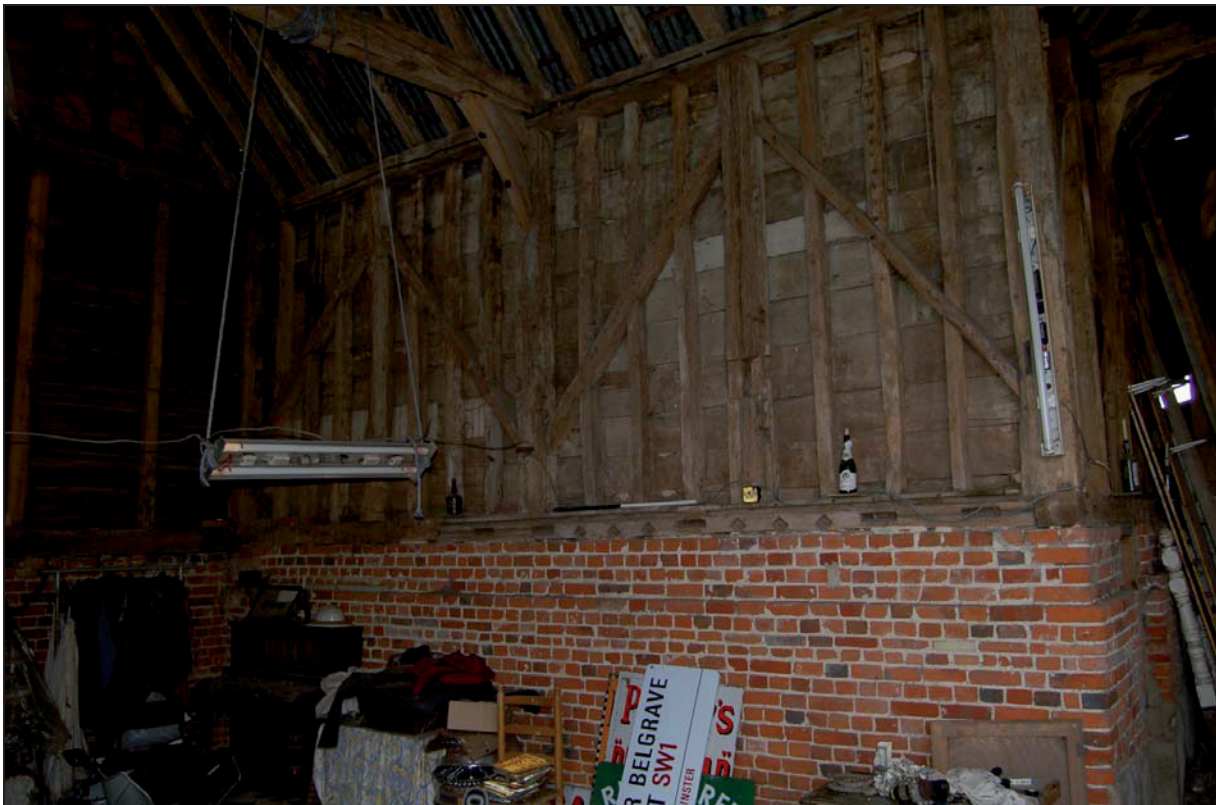
Plate 8 Reused wall plate used as sill
