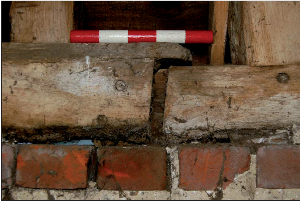
Plate 9 Bridle joint with over-lipped face in sill
