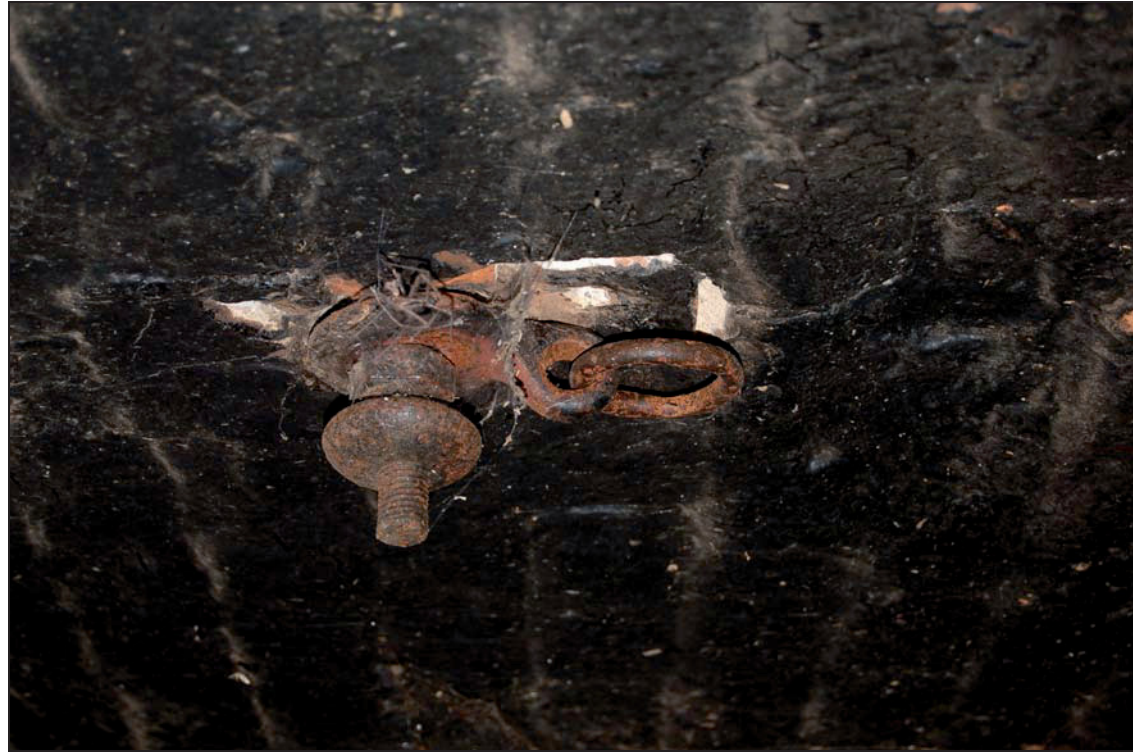
Plate 17 Tethering point
