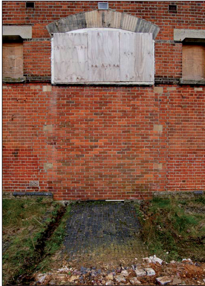
Plate 7 Blocked rear stable doorway and fittings for litter sheds
