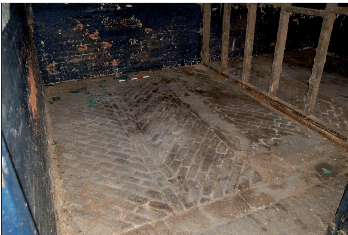
Plate 29 Stall flooring in officer's stable
