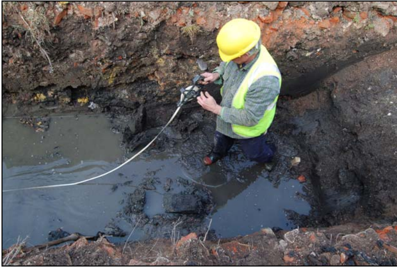
Plate 4 North end of trench 2, looking west
