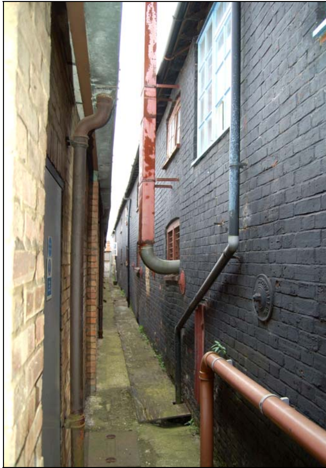
Plate 13 Sequence of gridded germinating floor windows including one in covered-up light well
