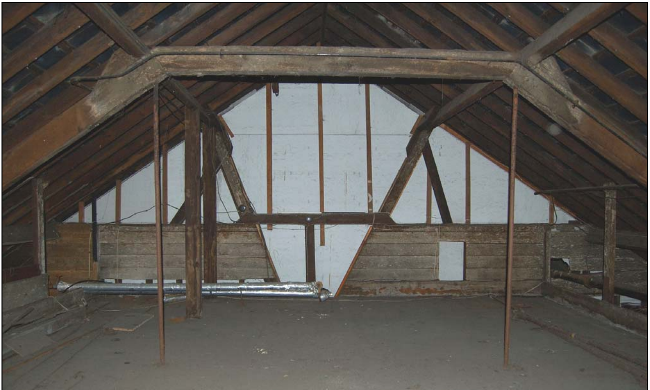
Plate 20 Rebuilt kiln wall and inspection hatch
