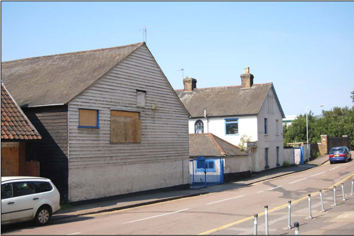
Plate 1 Malting viewed from Station Road to north-west
