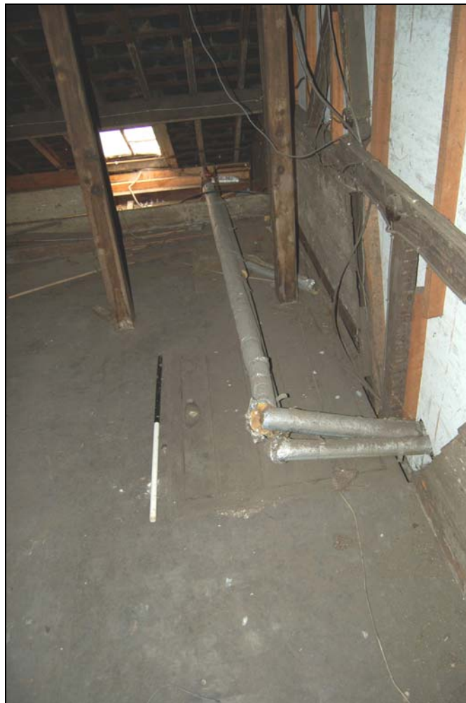
Plate 22 Trapdoor for hoist with shovelling hatch in background (1m scale)
