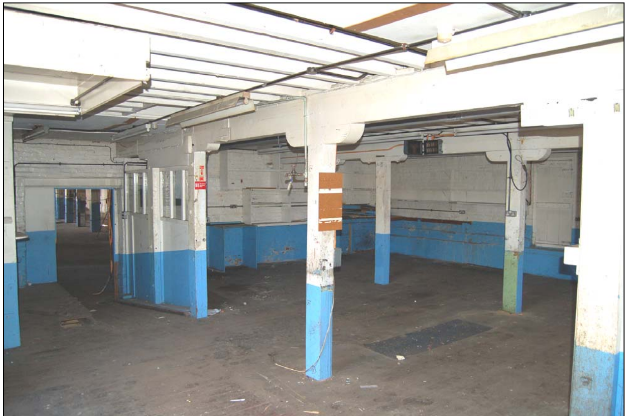
Plate 26 Ground floor of maltstore
