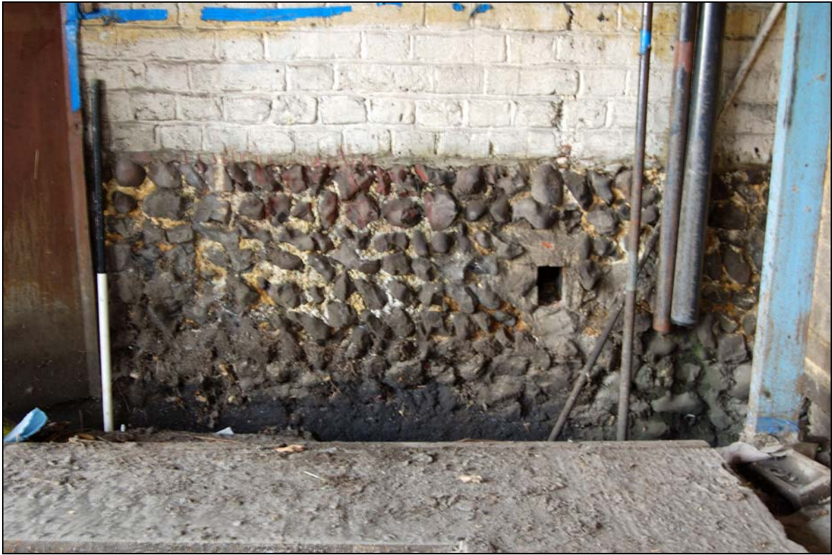
Plate 15 Flint wall to earlier construction, part of west wall of germinating floors
