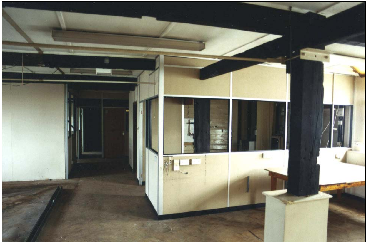
Plate 12 Remaining southern wall of barley store inside office partition (right)
