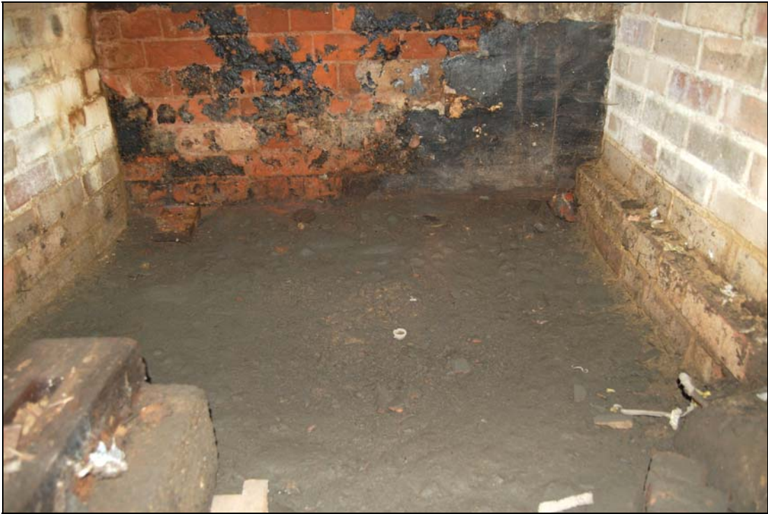
Plate 27 Cobbled yard surface below maltstore floor
