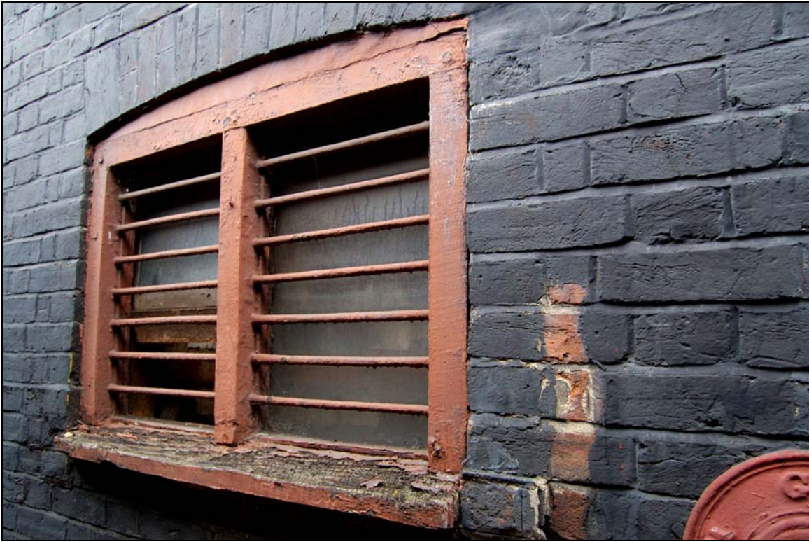
Plate 7 Original window to germinating floors
