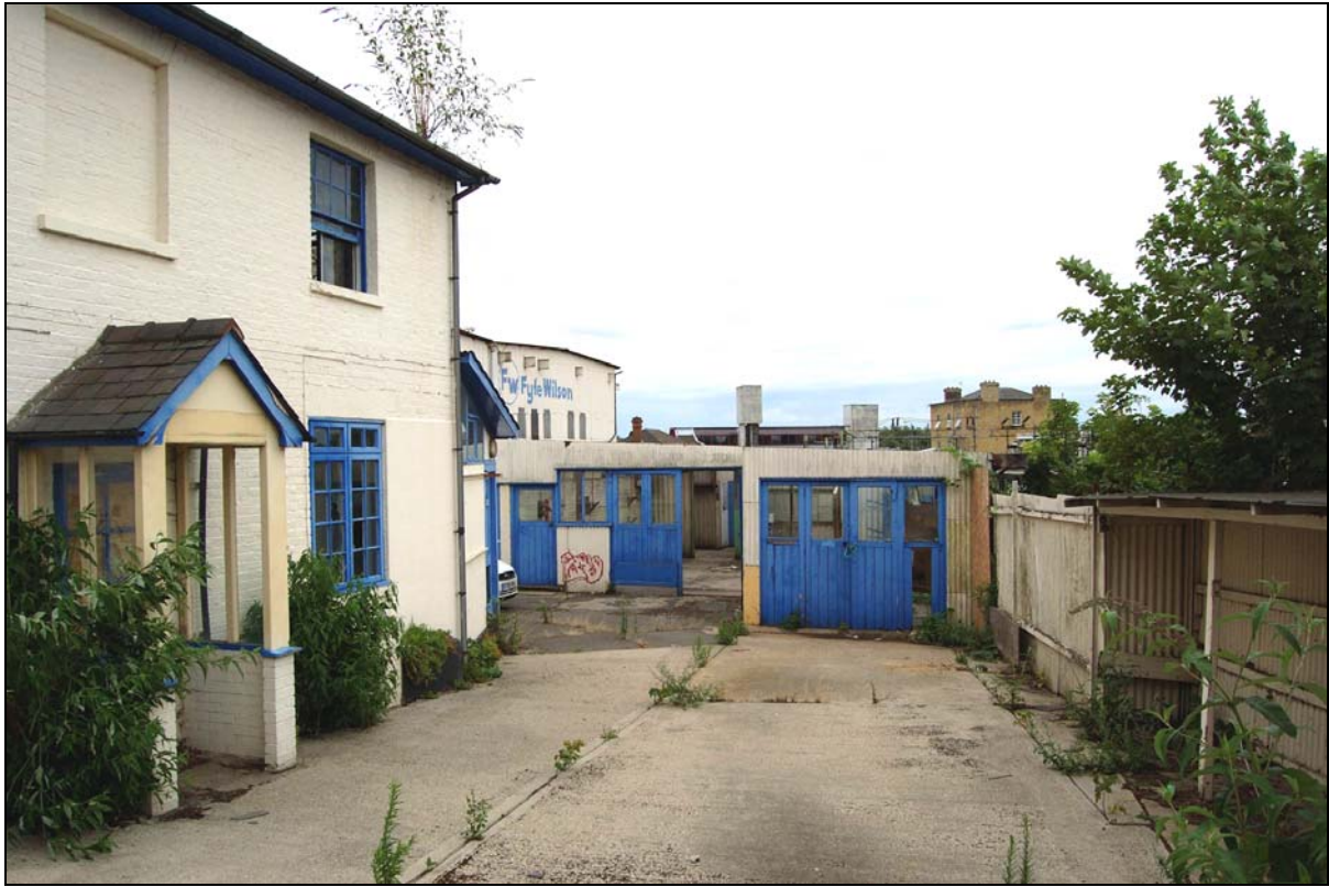
Plate 31 View toward 20th-century welding shop and loading bay
