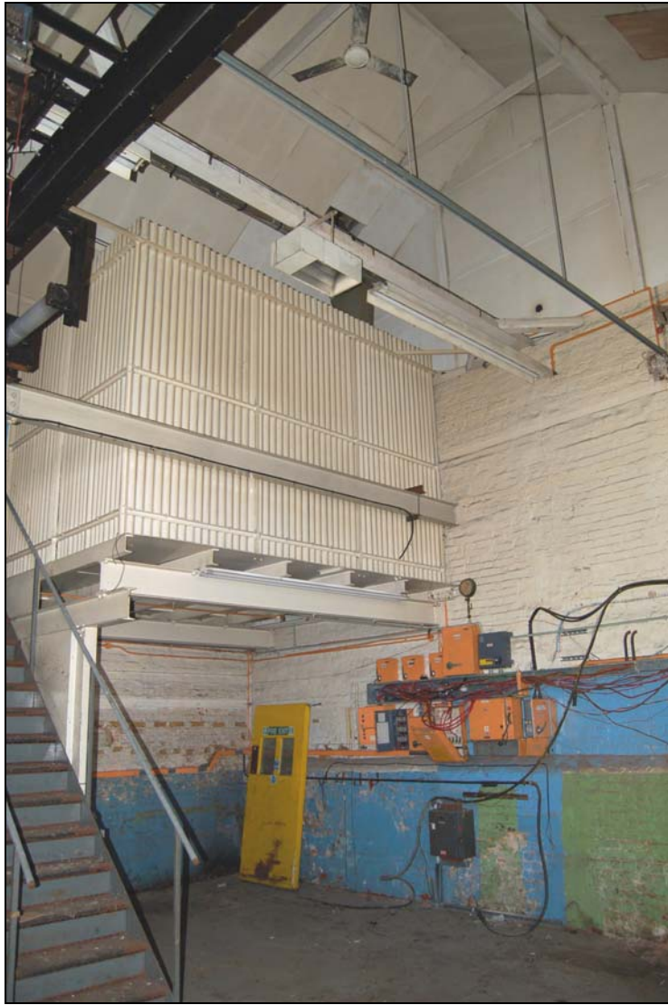
Plate 23 Stripped-out kiln interior
