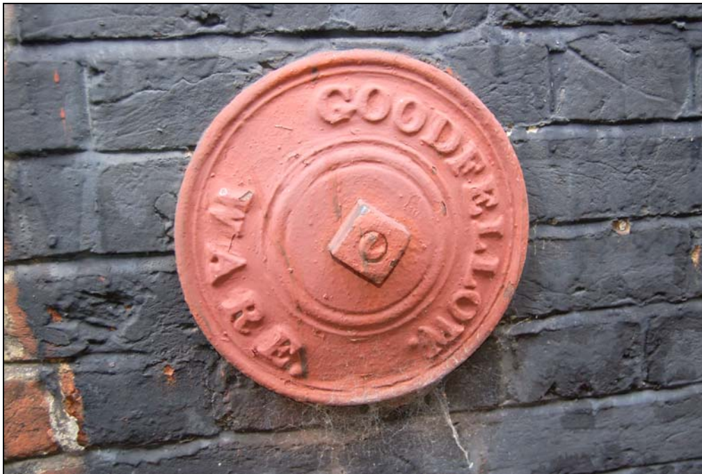
Plate 14 Cast tie rod plate with maker's name
