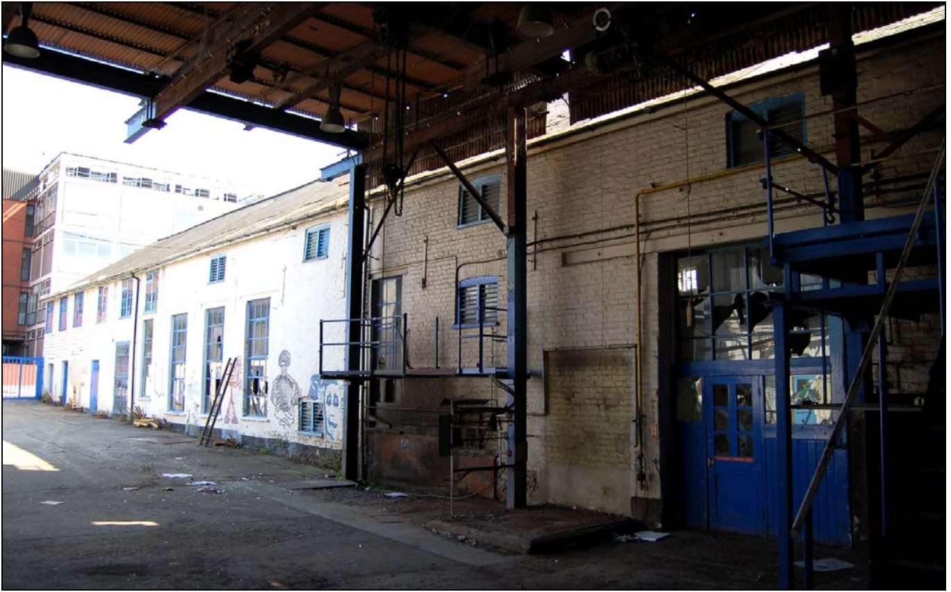
Plate 3 South end of barley store and germinating floors viewed from south-west
