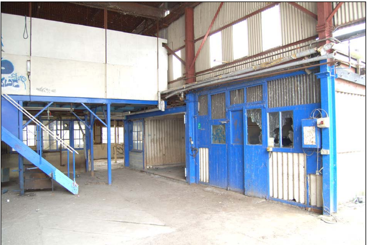
Plate 32 View inside loading bay
