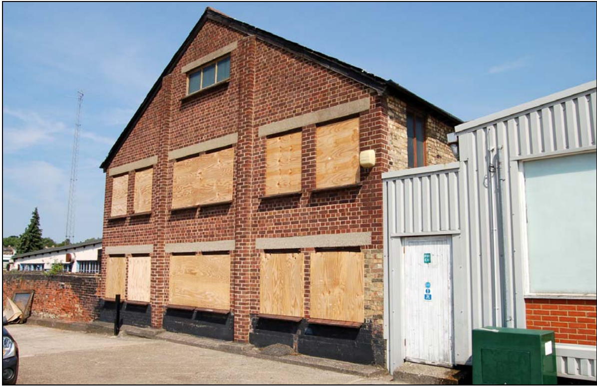
Plate 25 Maltstore viewed from south-east
