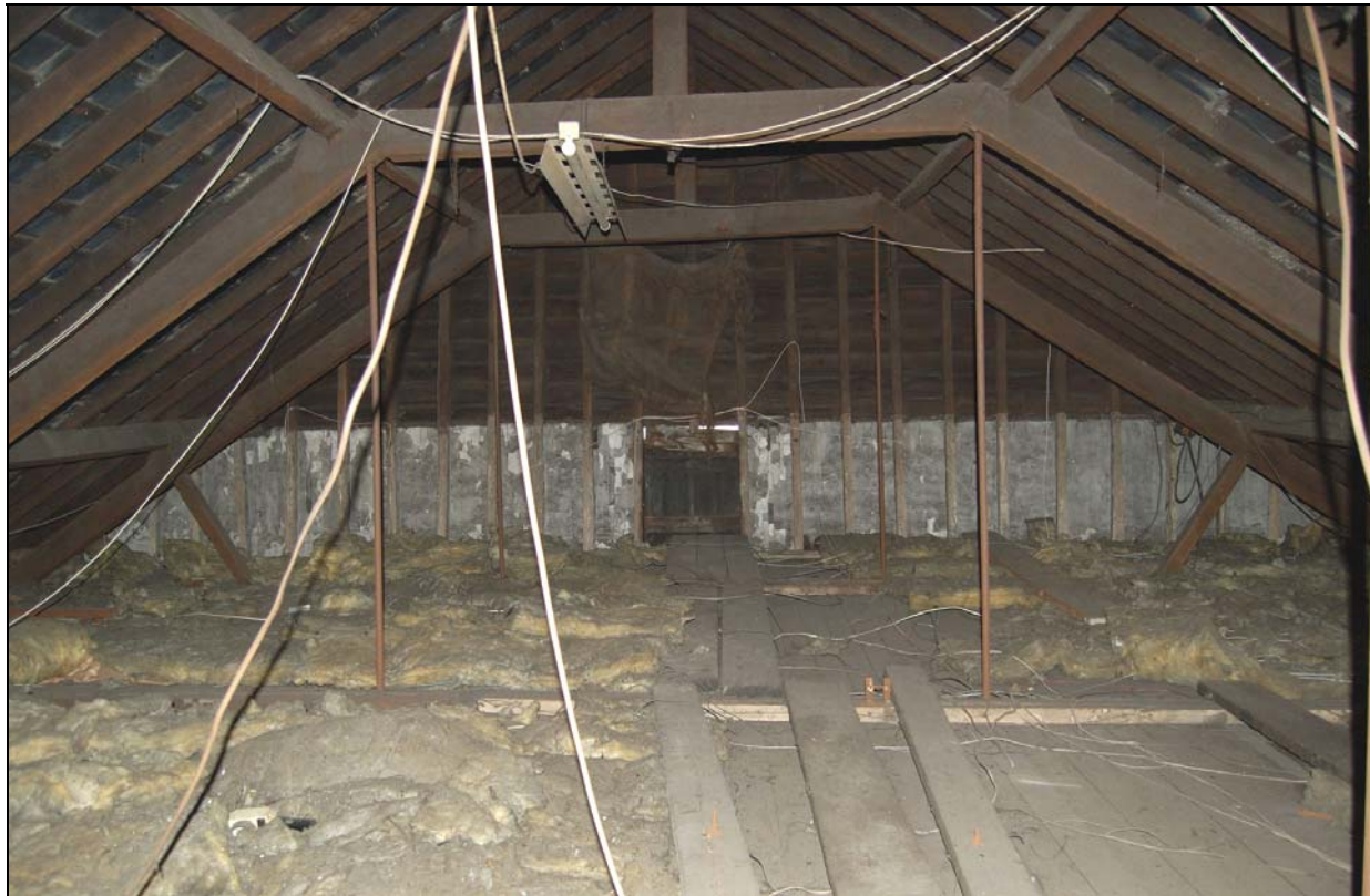
Plate 10 Small taking-in door at north end of barley store loft
