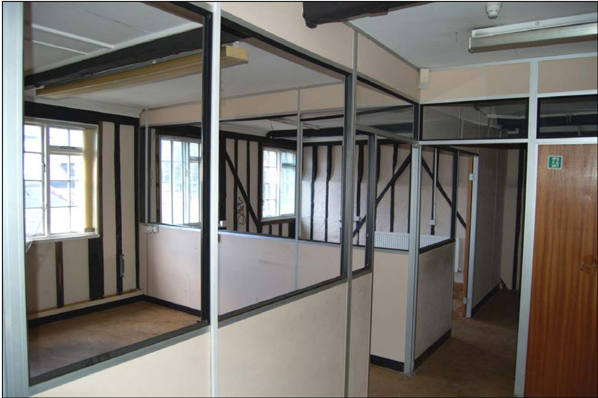
Plate 9 Timber framing and inserted partitions on first floor of barley store
