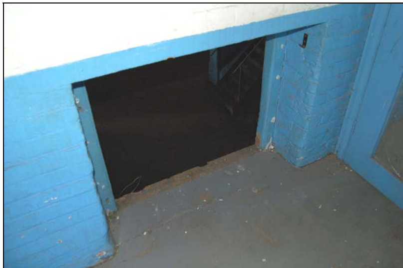
Plate 24 Shovelling hatch from kiln to maltstore
