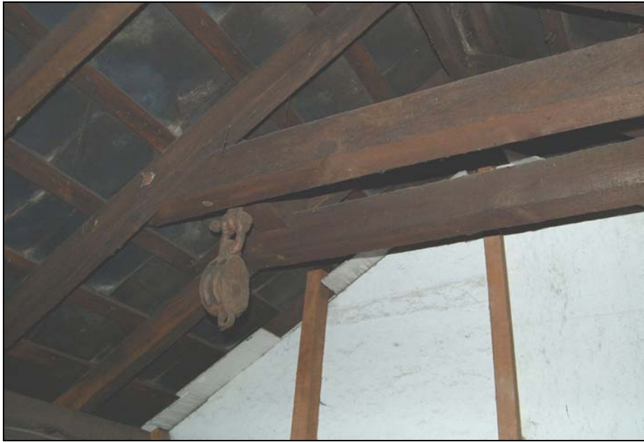
Plate 21 In situ hoist at kiln end of germinating floors
