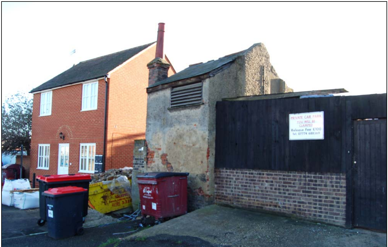
Plate 2 Shed viewed from west
