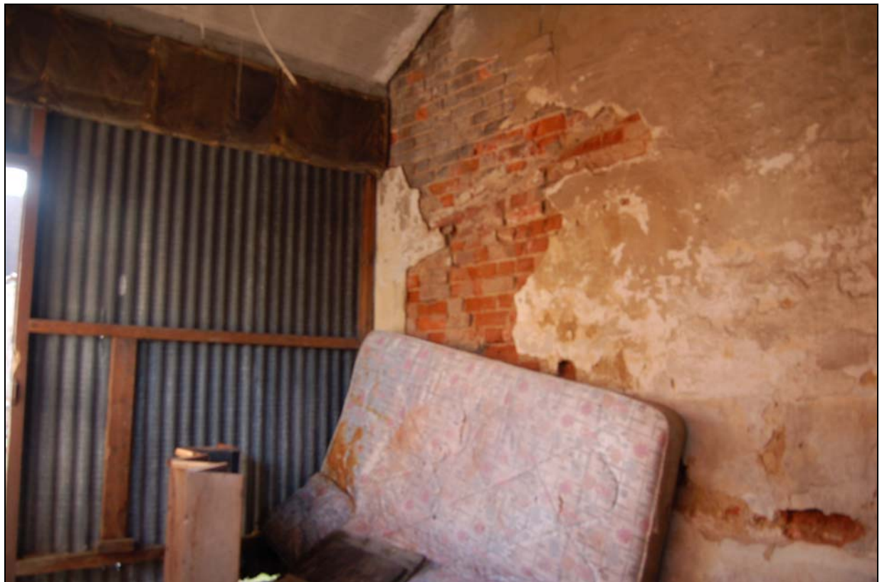
Plate 6 Interior viewed from north
