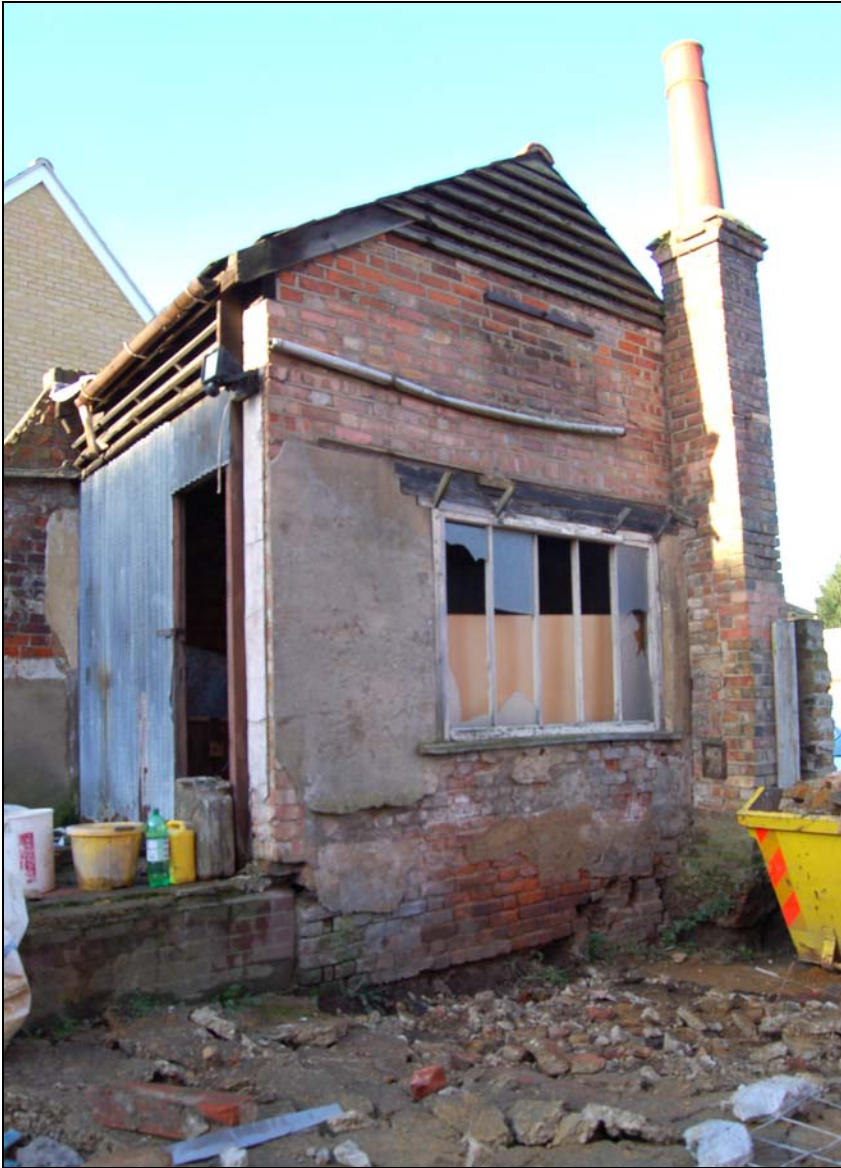
Plate 3 Shed viewed from east
