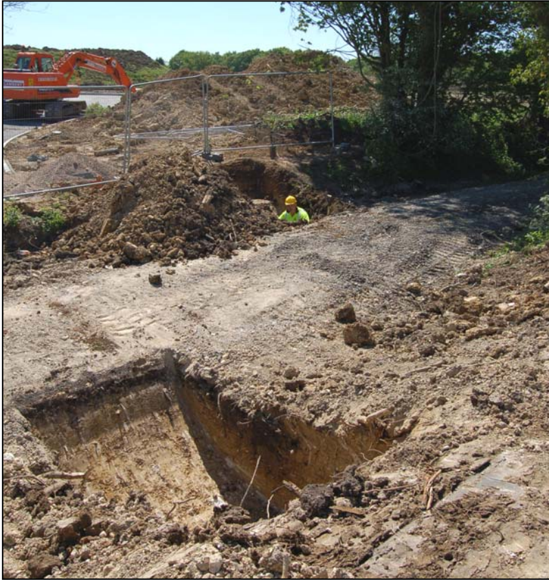
Plate 1 – Trenches under excavation, facing south
