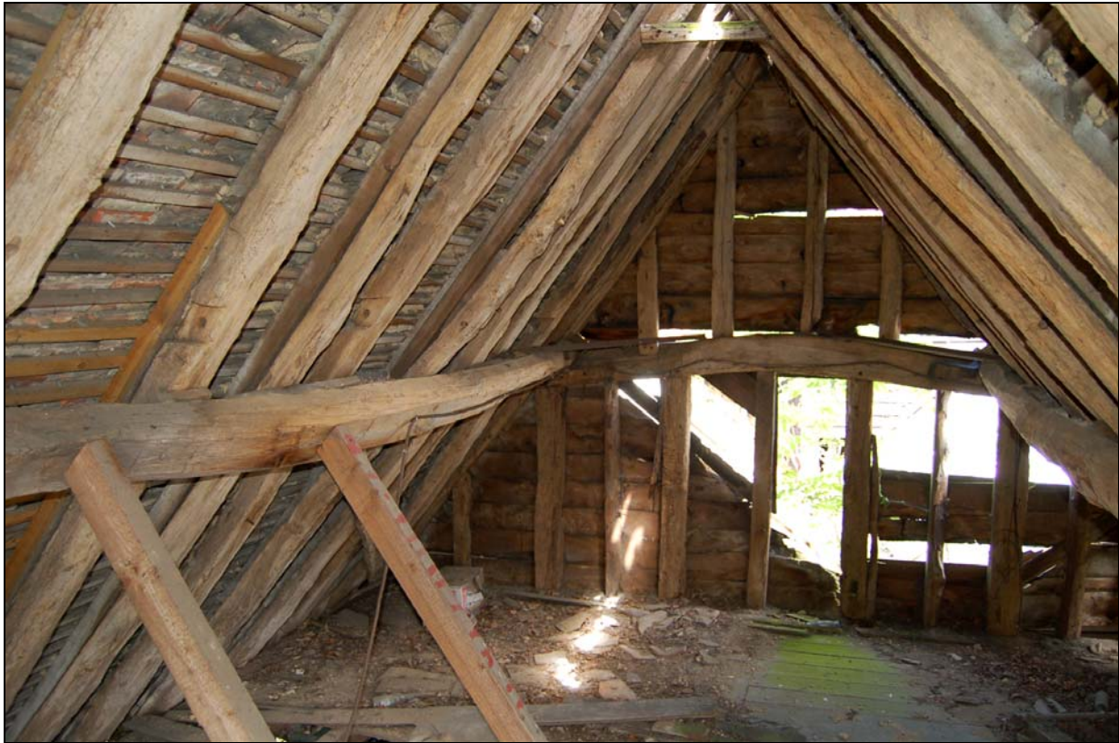
Plate 23 Propped purlin and original north wall of byre
