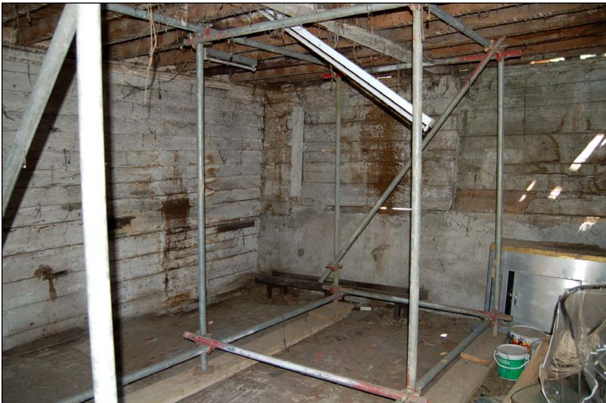
Plate 18 Tackroom interior viewed from south-west
