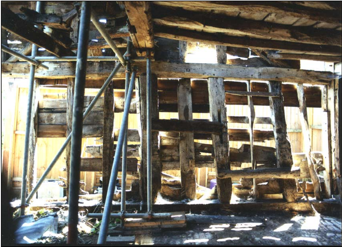
Plate 21 Original studwork in south wall of byre
