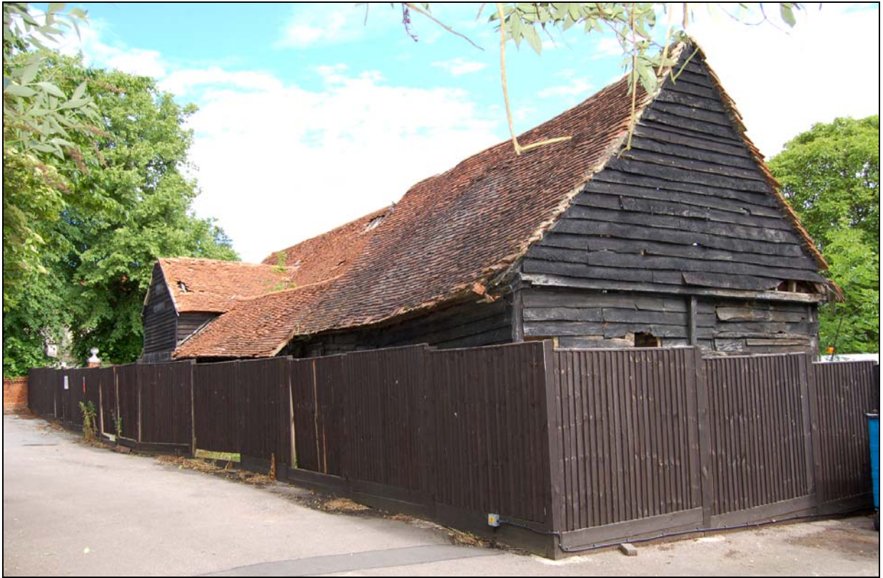
Plate 13 Byre and other buildings viewed from south
