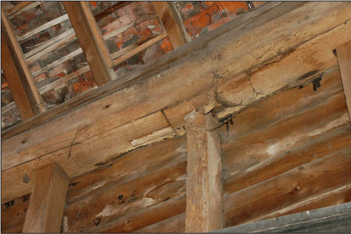
Plate 9 Partly-observed bridge scarf joint with squinted abutments
