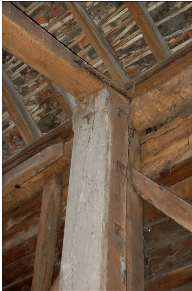
Plate 8 Reused bridging joist to support tie beam by west door
