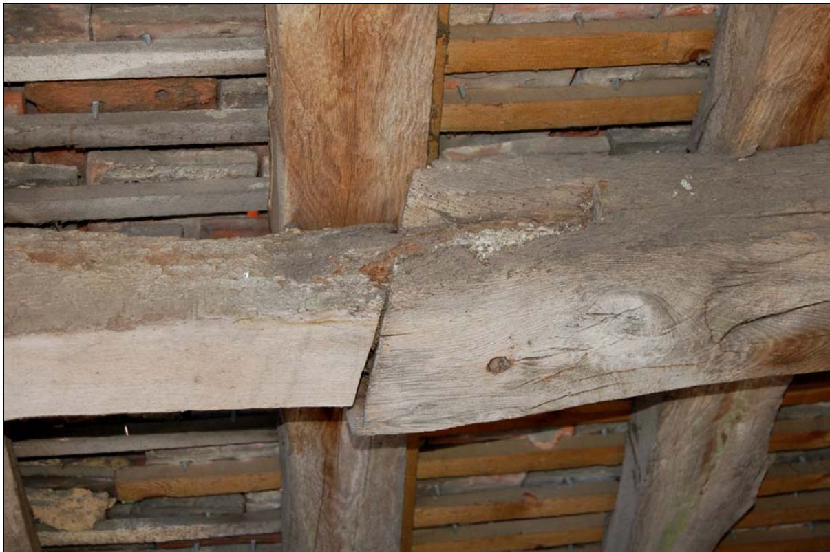
Plate 24 Purlin with bridle scarf with squinted abutments in roof of byre
