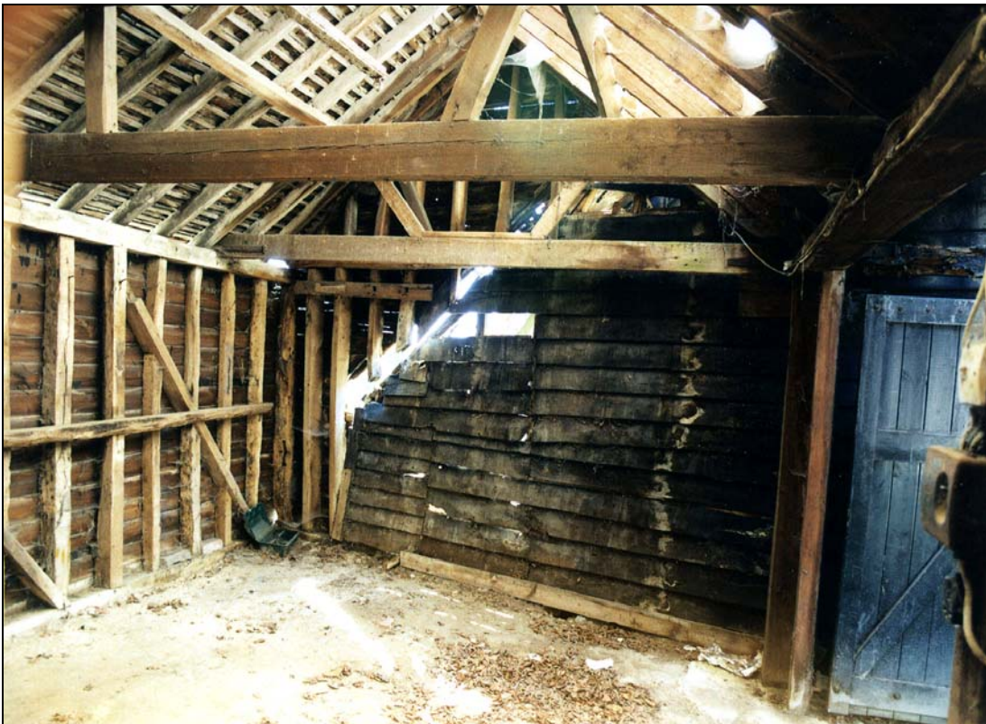
Plate 12 Inside rear part of cart shed, including stabling
