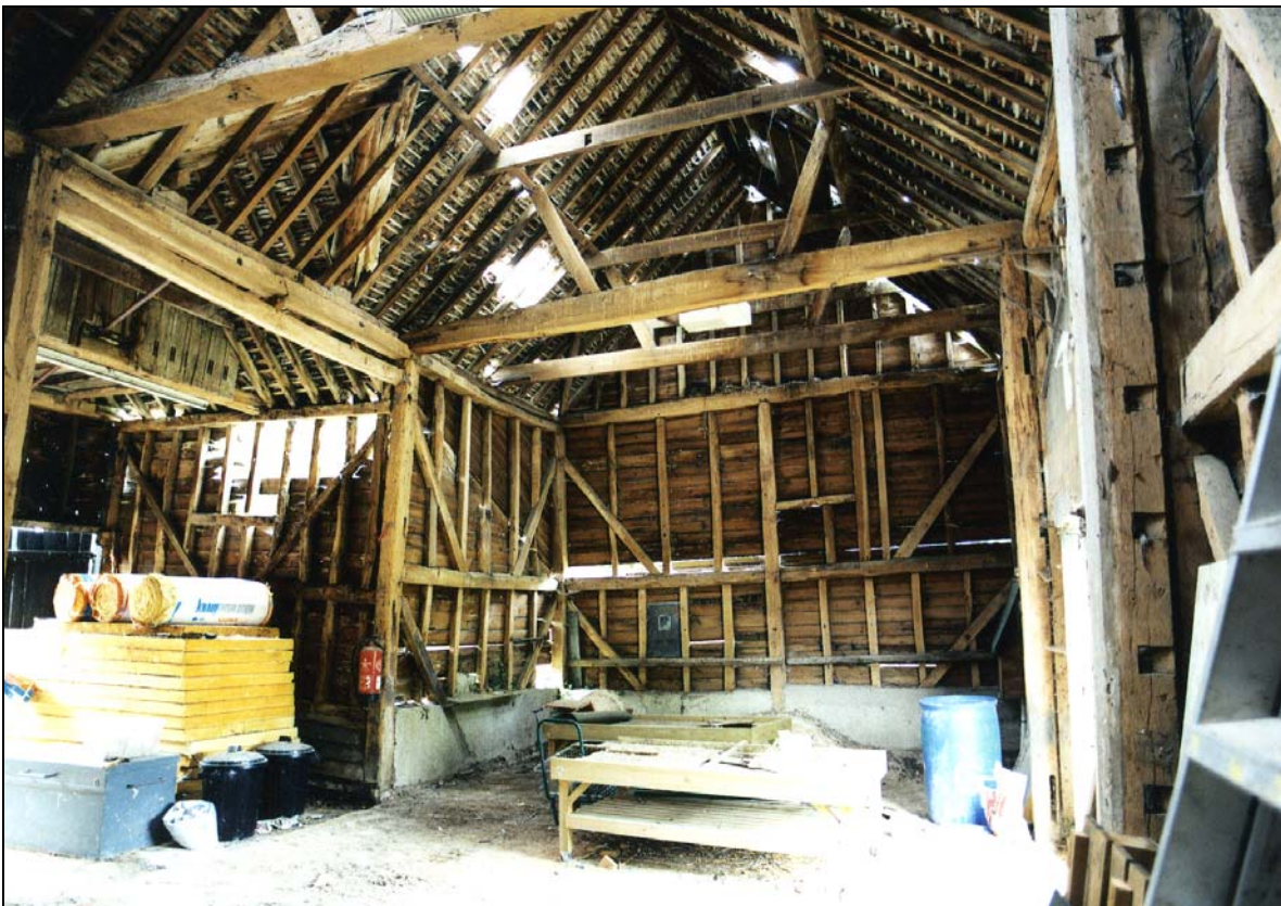
Plate 6 Interior of barn viewed toward porch (north-west)
