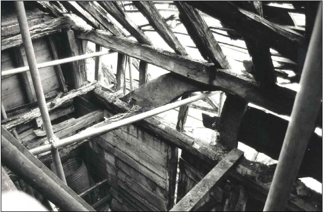
Plate 25 Heavy bracing member on east wall of byre
