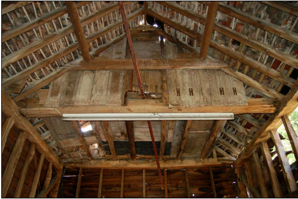
Plate 7 Dovecote inside porch
