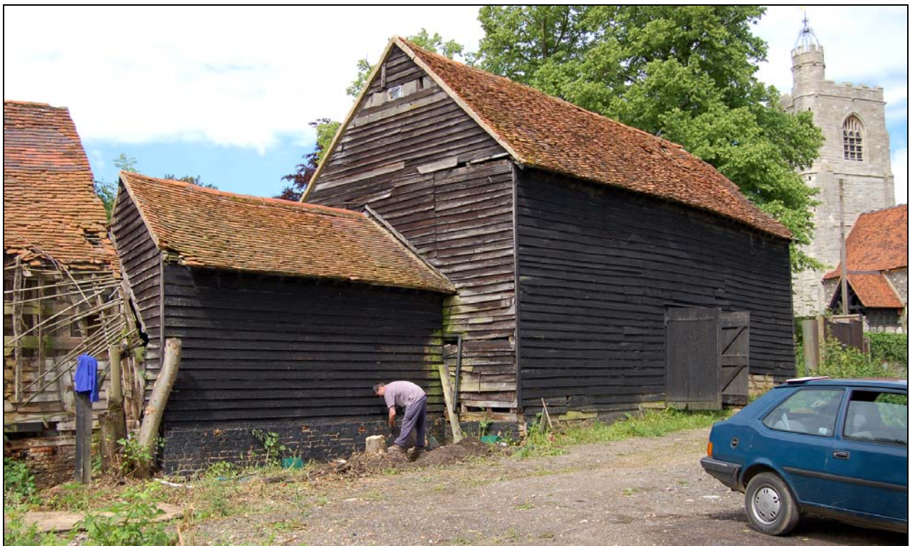
Plate 4 Barn and cart shed viewed from east
