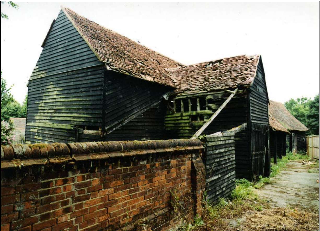
Plate 2 Barn viewed from north-west
