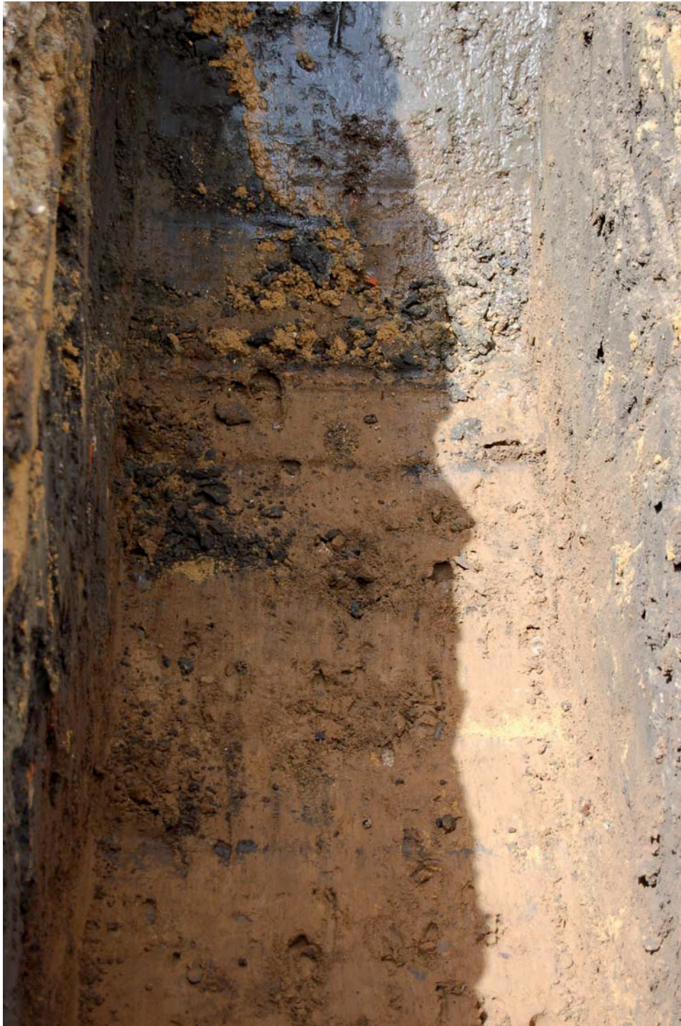
Plate 2. Southern foundation trench, looking north-west.
