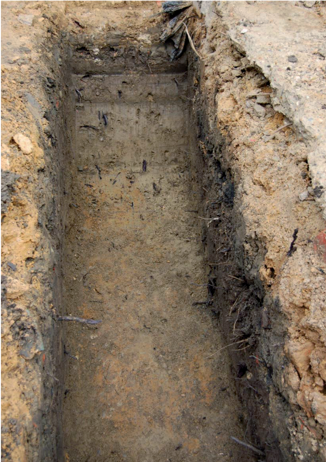
Plate 1. Northern foundation trench, looking north-west.
