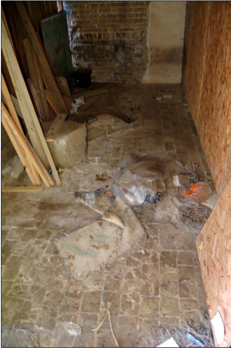
Plate 32 Gault brick floor in former stall
