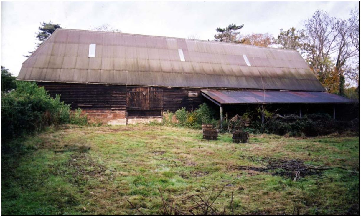
Plate 14 South-east elevation of barn 2
