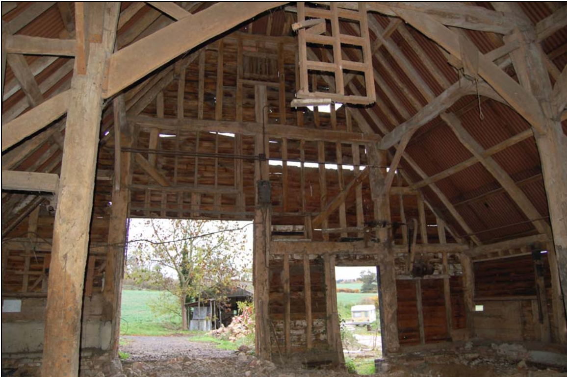
Plate 10 Partly rebuilt north wall in barn 1a
