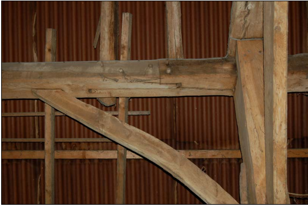
Plate 20 Edge-halved and bladed scarf joint connecting two builds in barn 2
