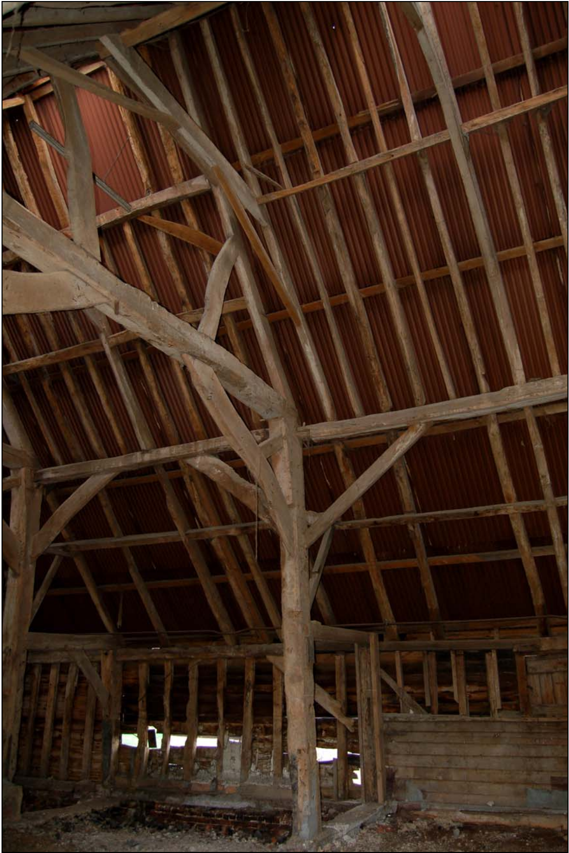
Plate 13 Comparison of two builds at southern end of barn 1a
