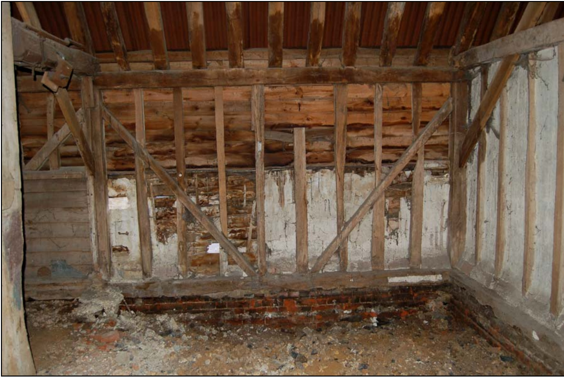
Plate 9 Primary bracing and plastered panels in barn 1b
