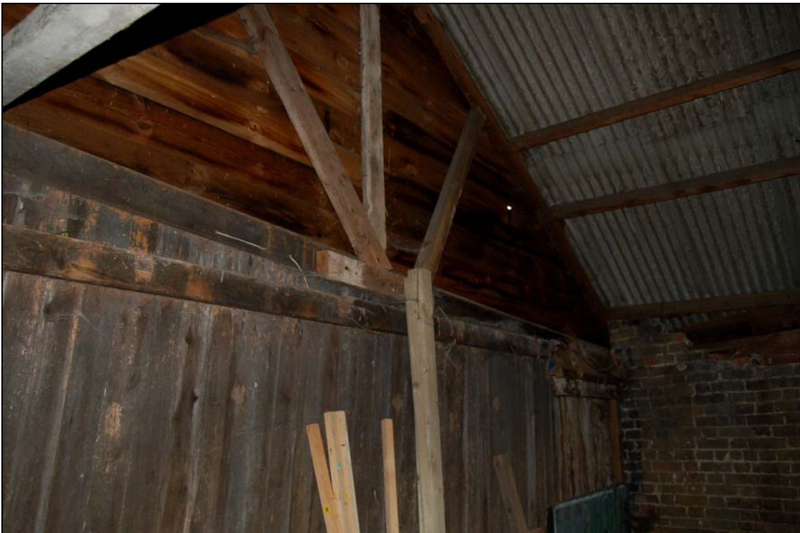
Plate 31 Original king post roof truss
