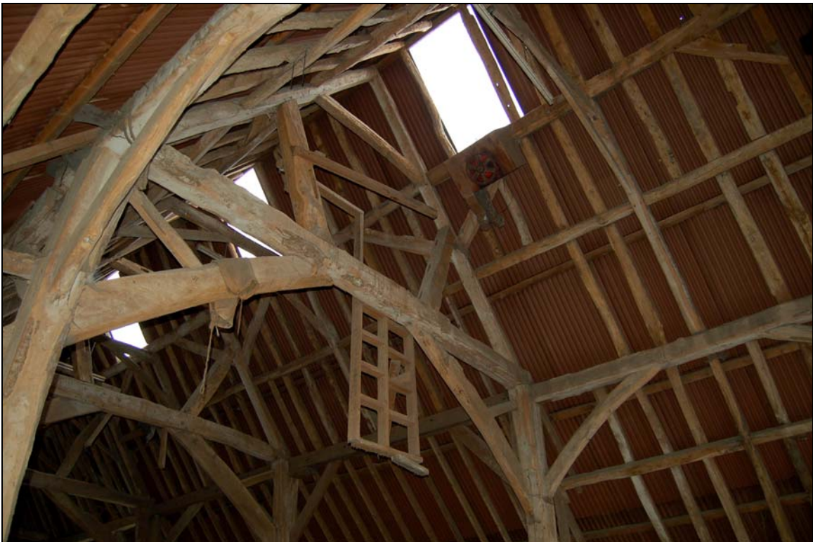
Plate 12 Belt rack and motor in butt-purlin roof in barn 1a
