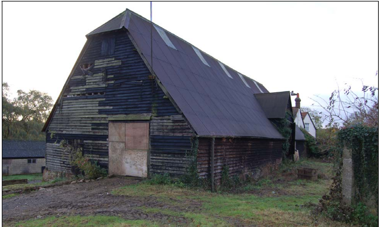
Plate 2 Barn 1 viewed from north-west
