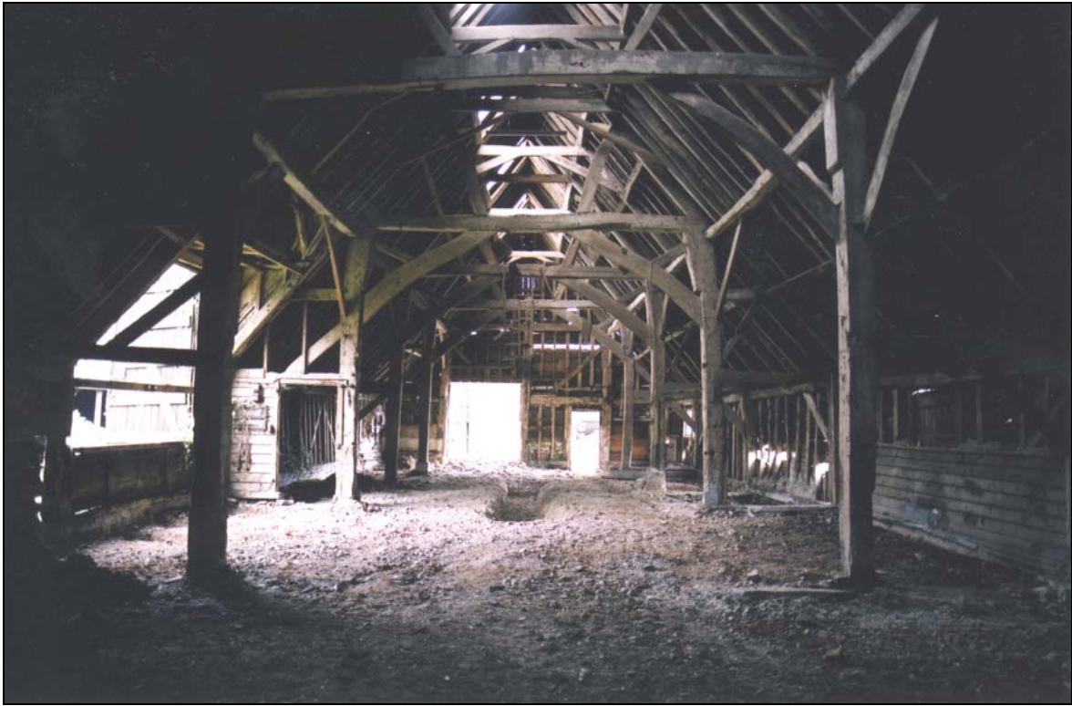
Plate 7 Interior of barn 1 from 1b to north gable wall
