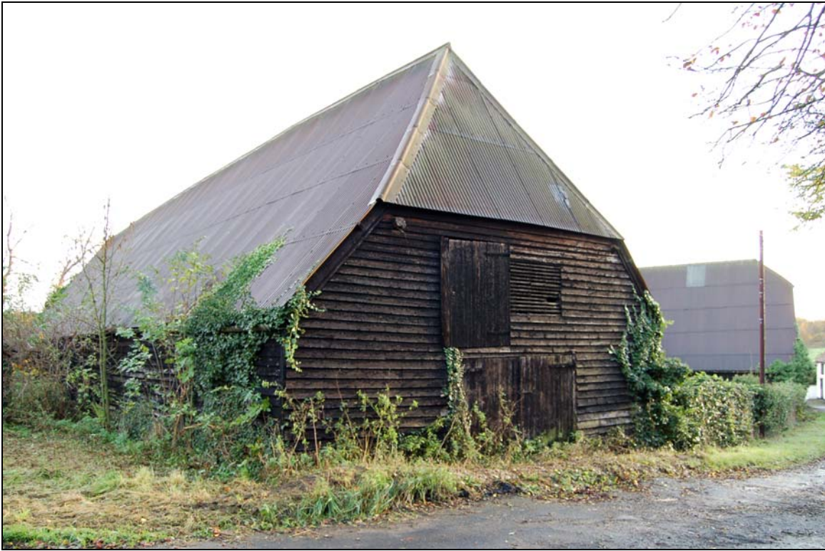
Plate 16 south-west elevation of barn 2
