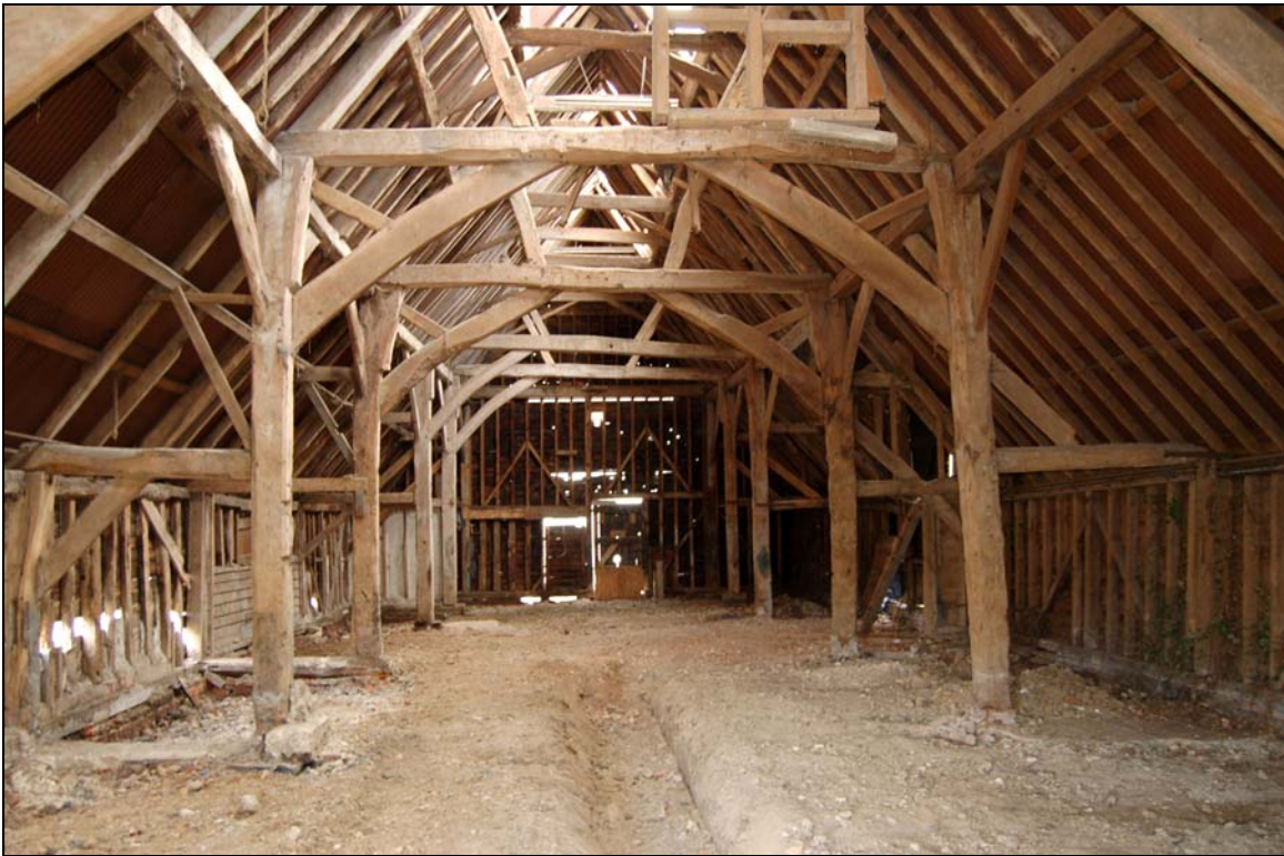
Plate 6 Interior of barn 1 from 1a to south gable wall
