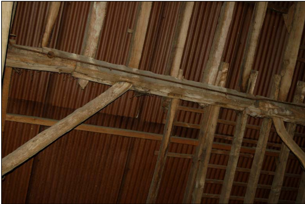
Plate 19 Reused wall plate connecting aisle plates in barn 2
