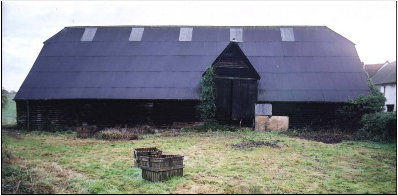
Plate 3 West elevation of barn 1
