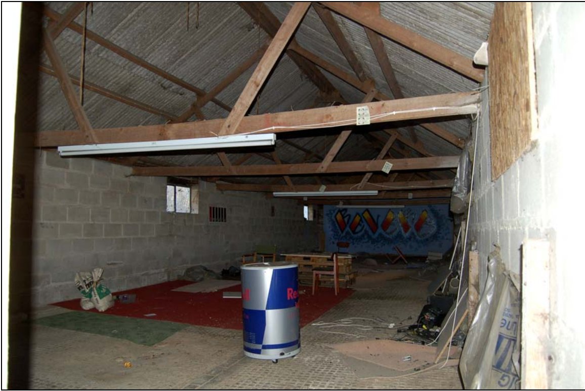
Plate 30 Interior of building 4 viewed to south
