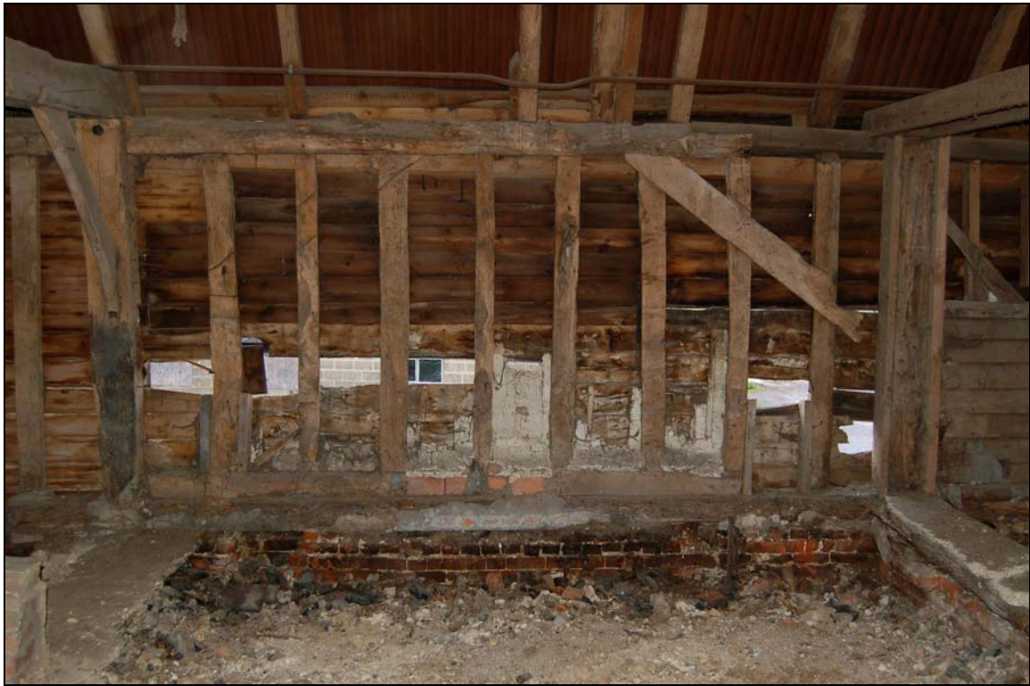
Plate 8 internal bracing in barn 1a
