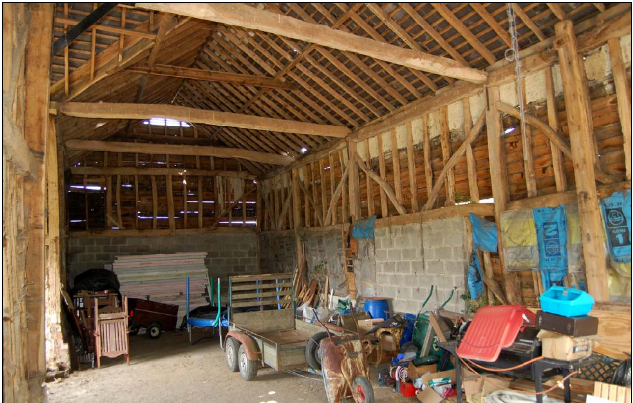
Plate 8 Interior of barn viewed to west
