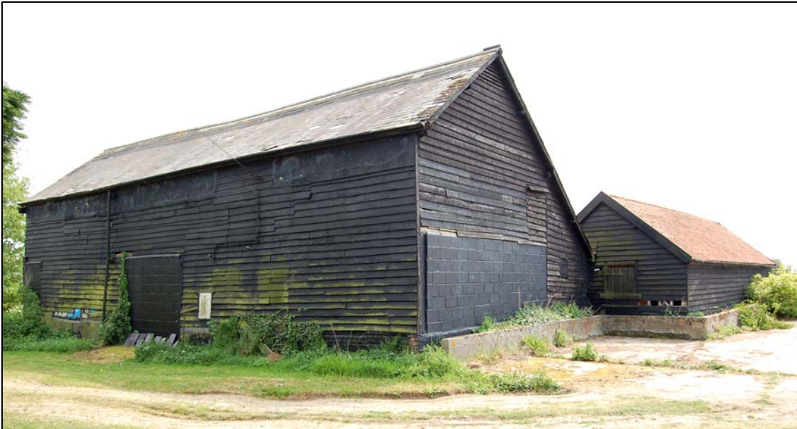
Plate 6 Rear of barn & cowshed viewed to south-east
