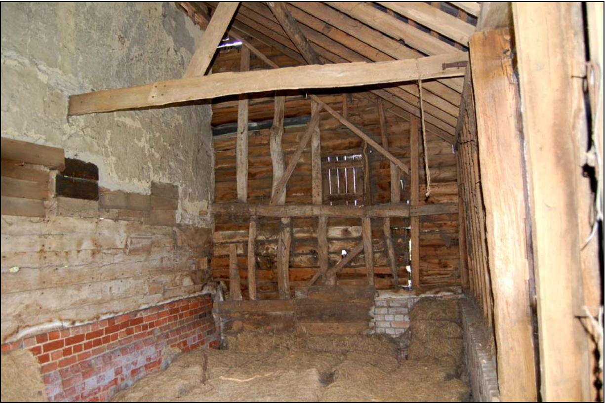
Plate 13 Extension & roof raise to shed 1b on eastern wall
