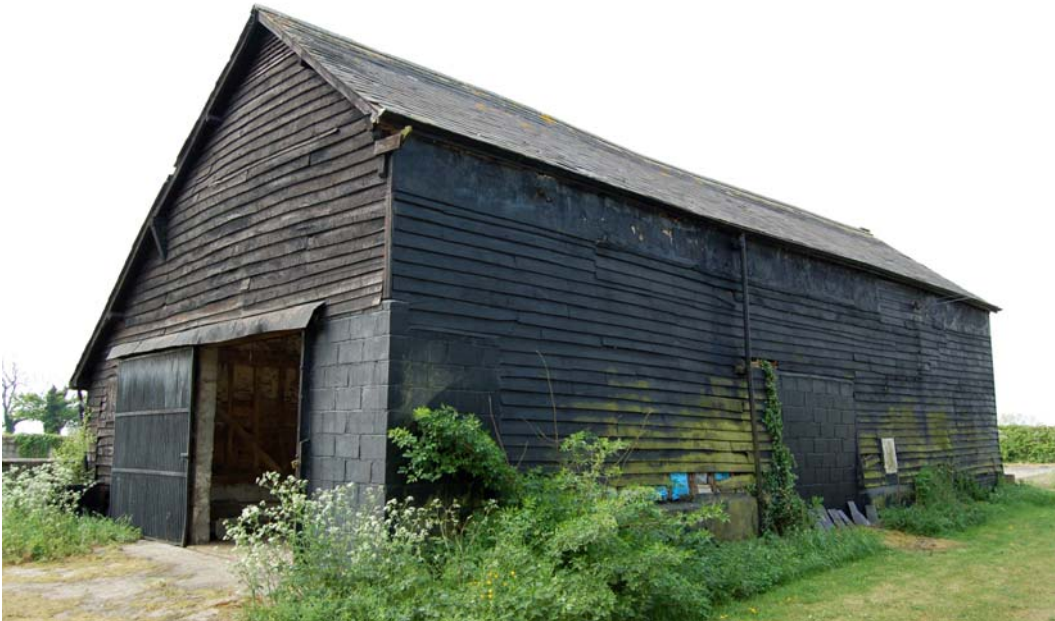
Plate 4 Barn viewed to south-west
