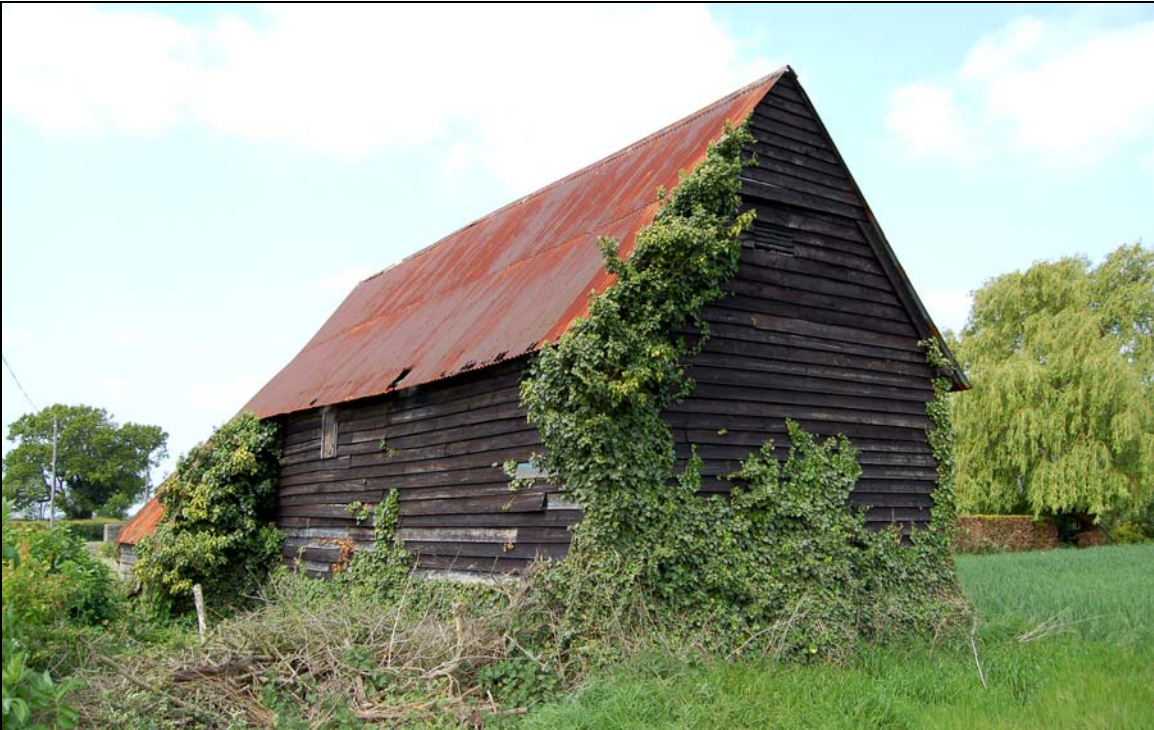
Barn viewed from south-east
