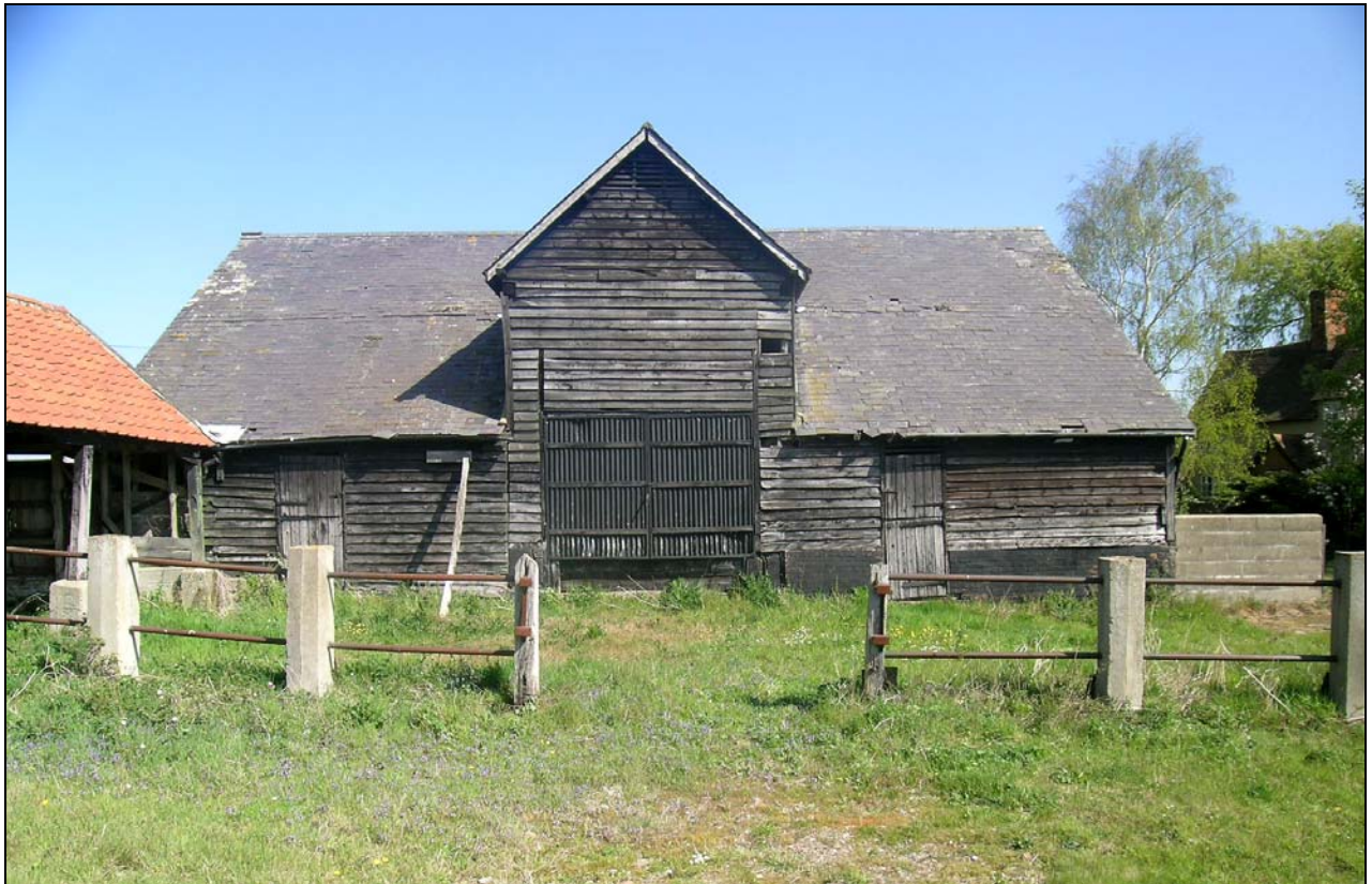
Plate 2 South elevation of barn
