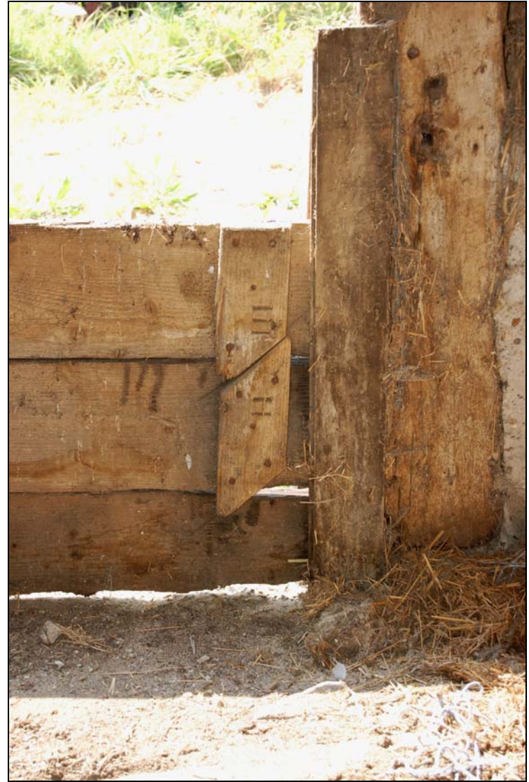
Plate 10 Detail of construction and markings to threshold leap
