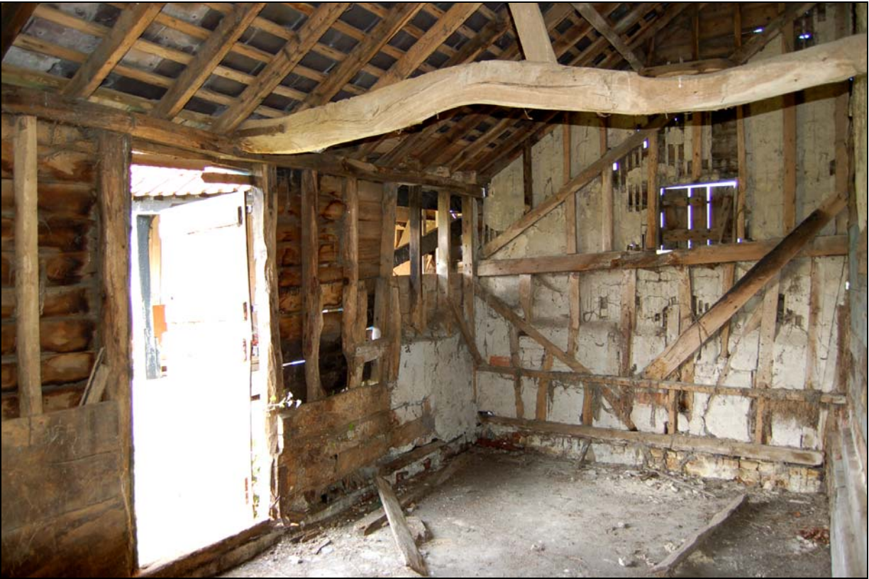
Plate 11 Interior of loose box 1a viewed to south-west
