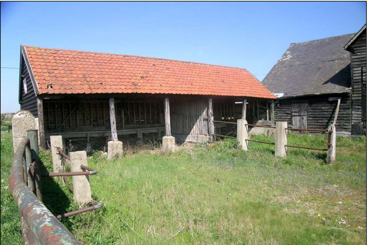
Plate 14 Eastern elevation of cowshed viewed across yard
