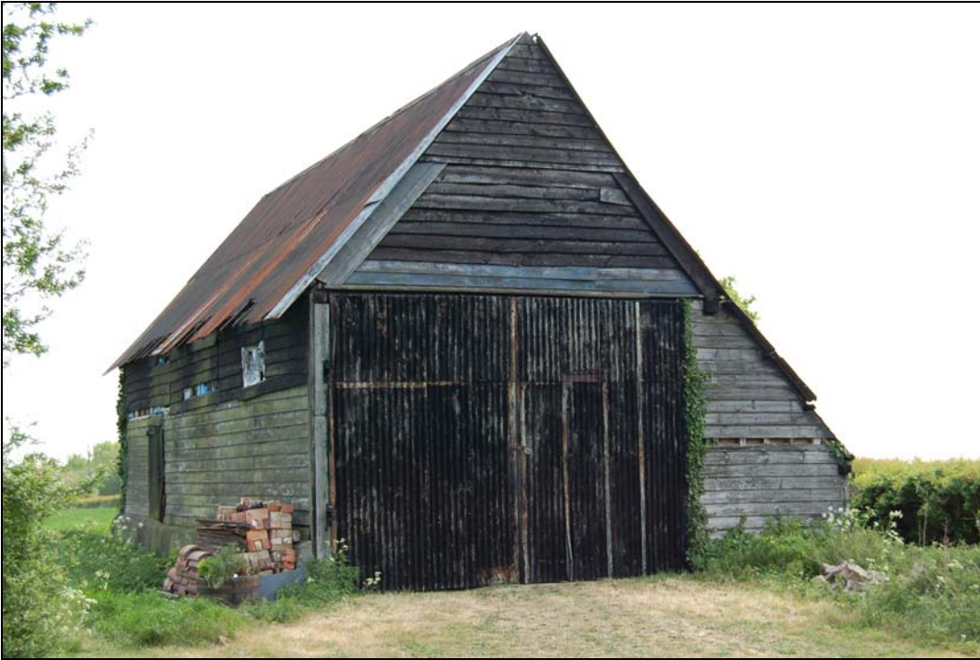
Barn viewed from north-west
