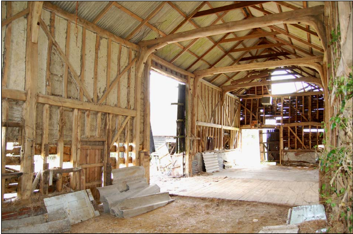
Plate 11 Interior of barn viewed to south
