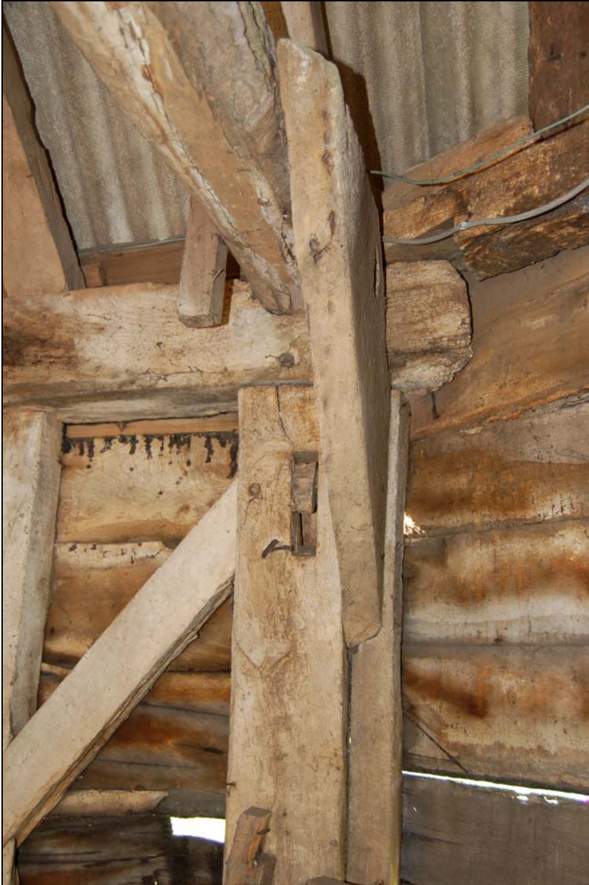
Plate 23 Construction detail of byre extension
