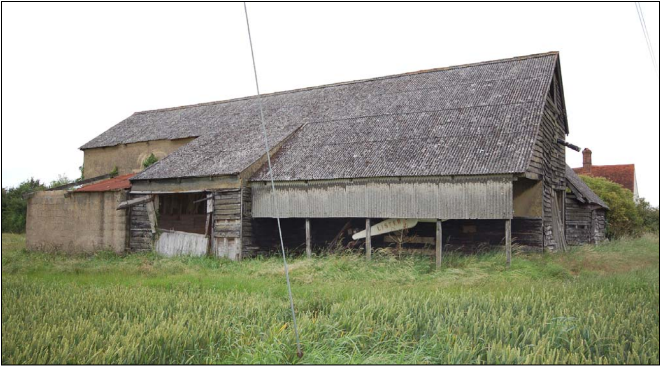
Plate 7 West elevation of barn
