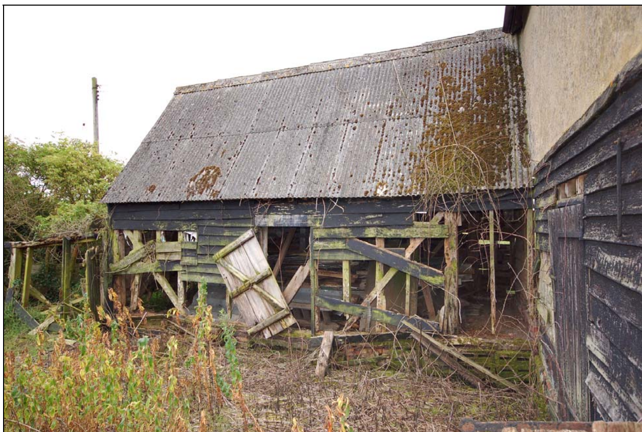
Plate 19 North elevation of byre
