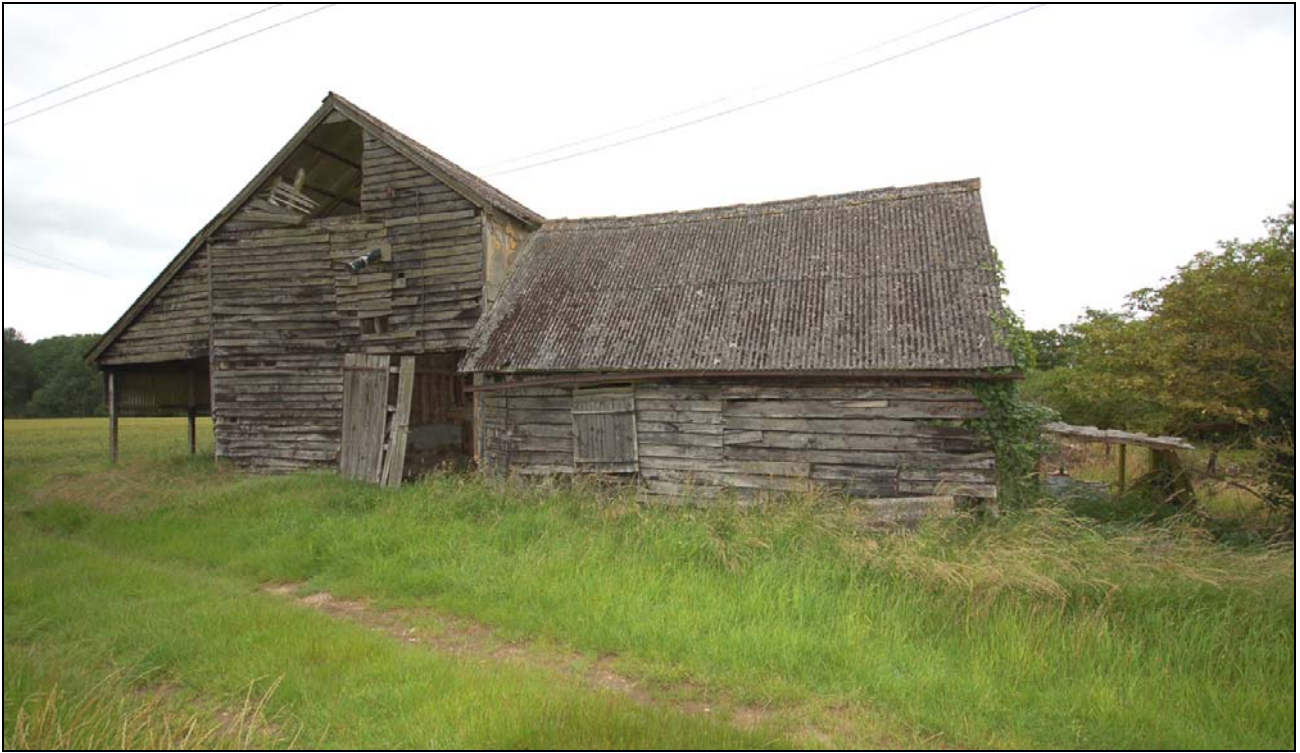
Plate 1 South elevation of barn and byre
