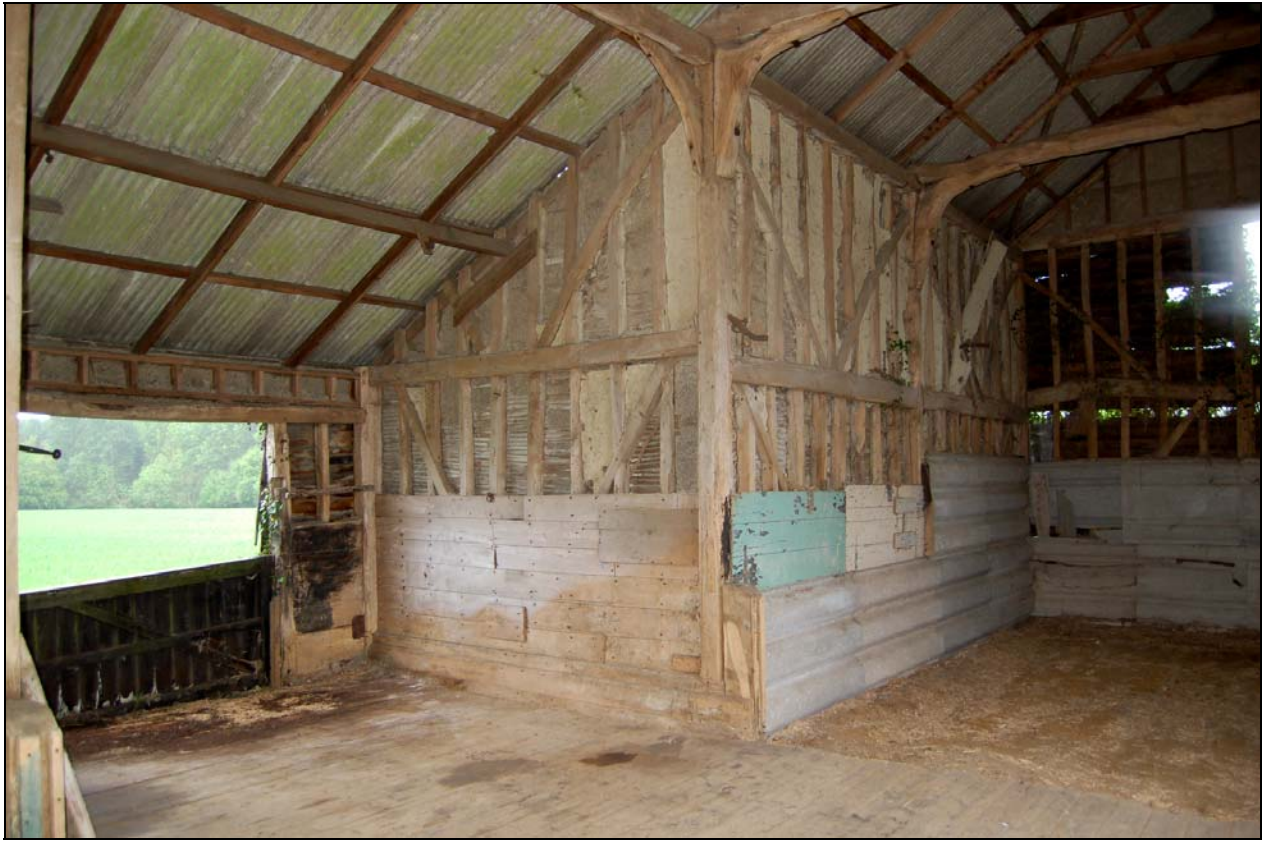
Plate 17 Detail of porch construction
