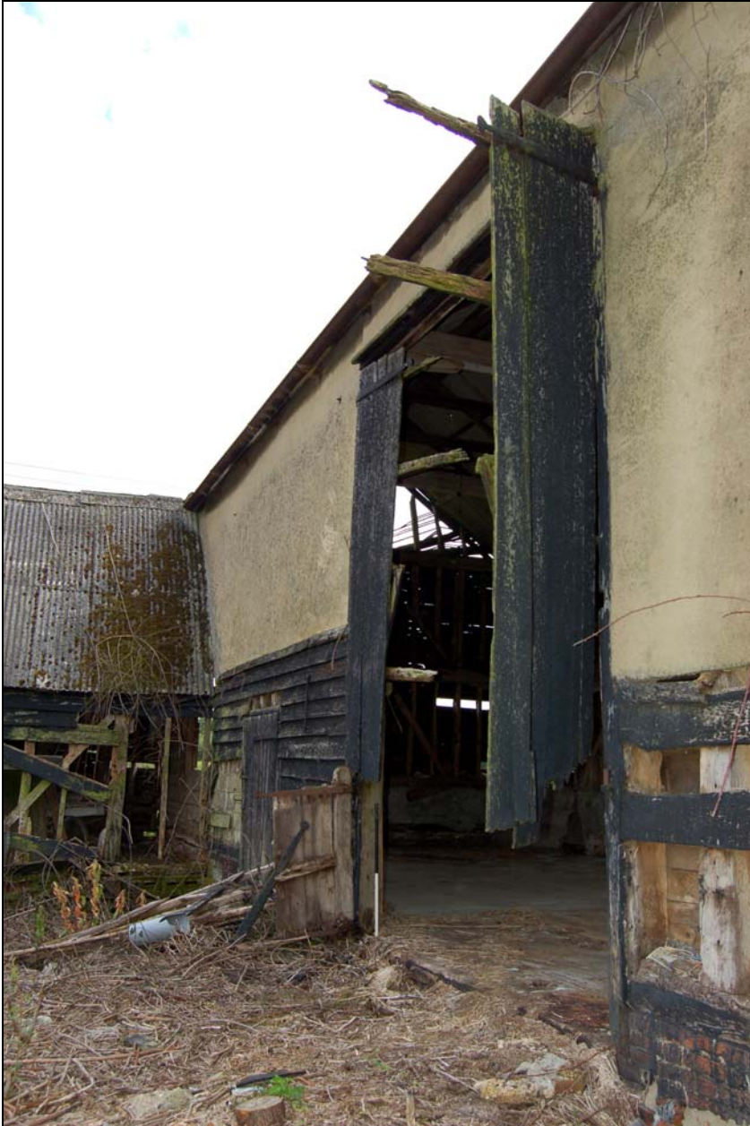
Plate 3 Barn doors on east side
