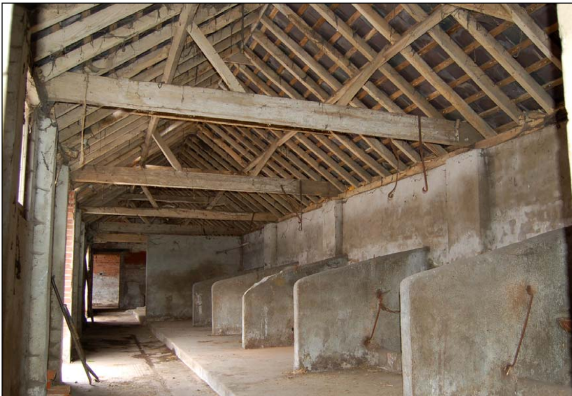
Plate 22 Interior of shelter shed 5 viewed to west
