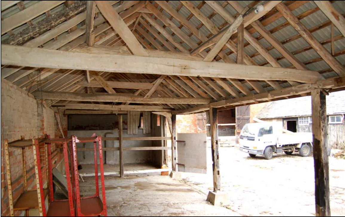
Plate 6 Interior of shelter shed 1 viewed to east
