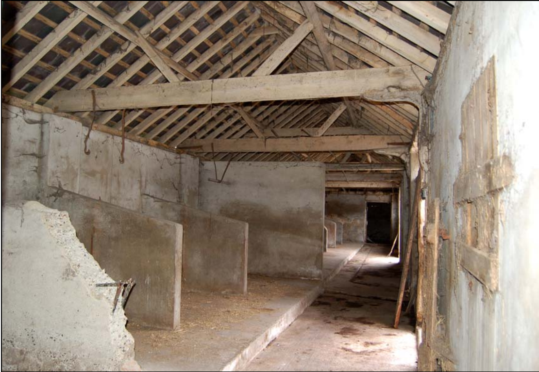
Plate 21 Interior of shelter shed 5 viewed to east
