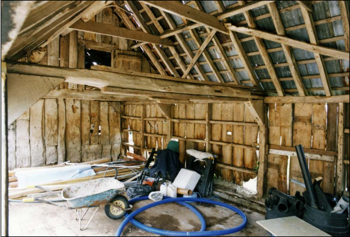
Plate 29 Interior of wagon lodge, east side
