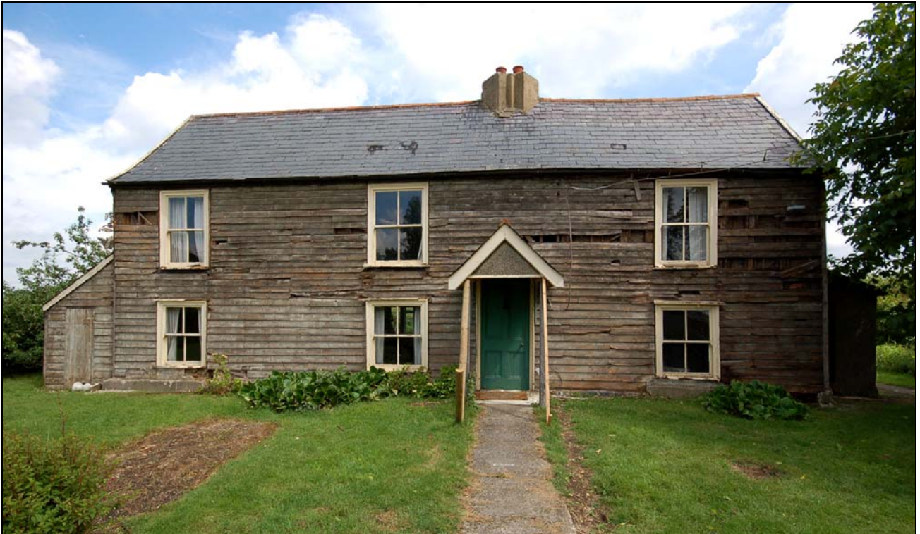
Plate 32 Front elevation of farmhouse
