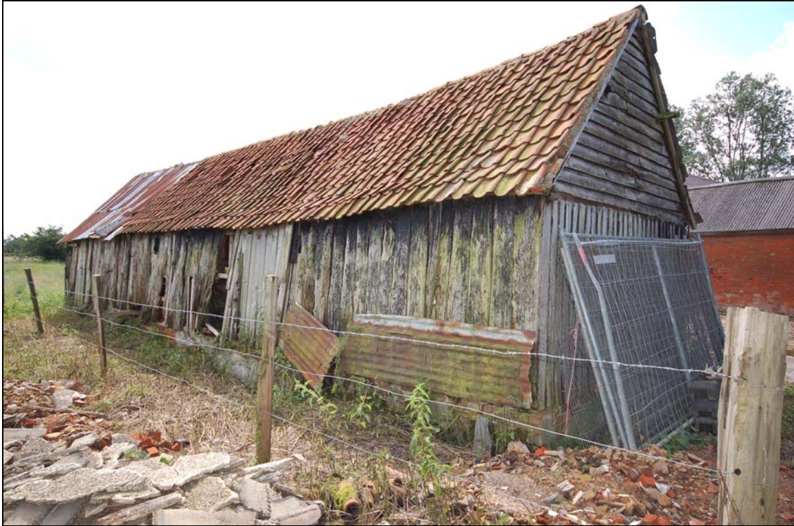
Plate 27 Rear wall of wagon lodge 8 viewed from north-west
