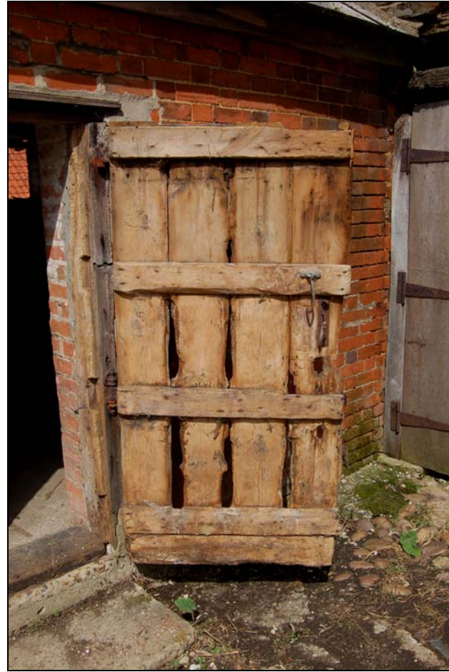
Plate 8 Original door into loose box 2
