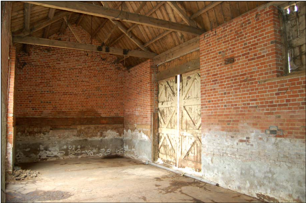
Plate 18 Interior of barn viewed to south
