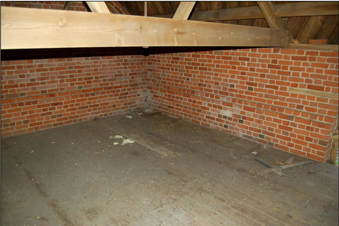
Plate 16 Hay hatch in north-east corner
