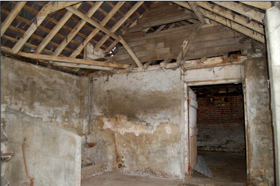
Plate 24 Cistern platform in shelter shed 5
