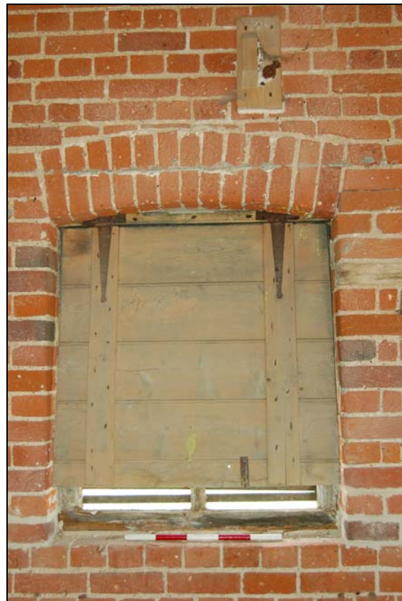
Plate 10 Shuttered malthouse window vent
