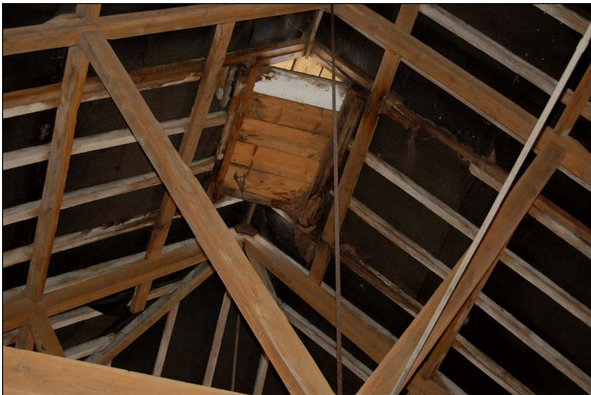
Plate 11 Roof truss and louver viewed from interior of malthouse
