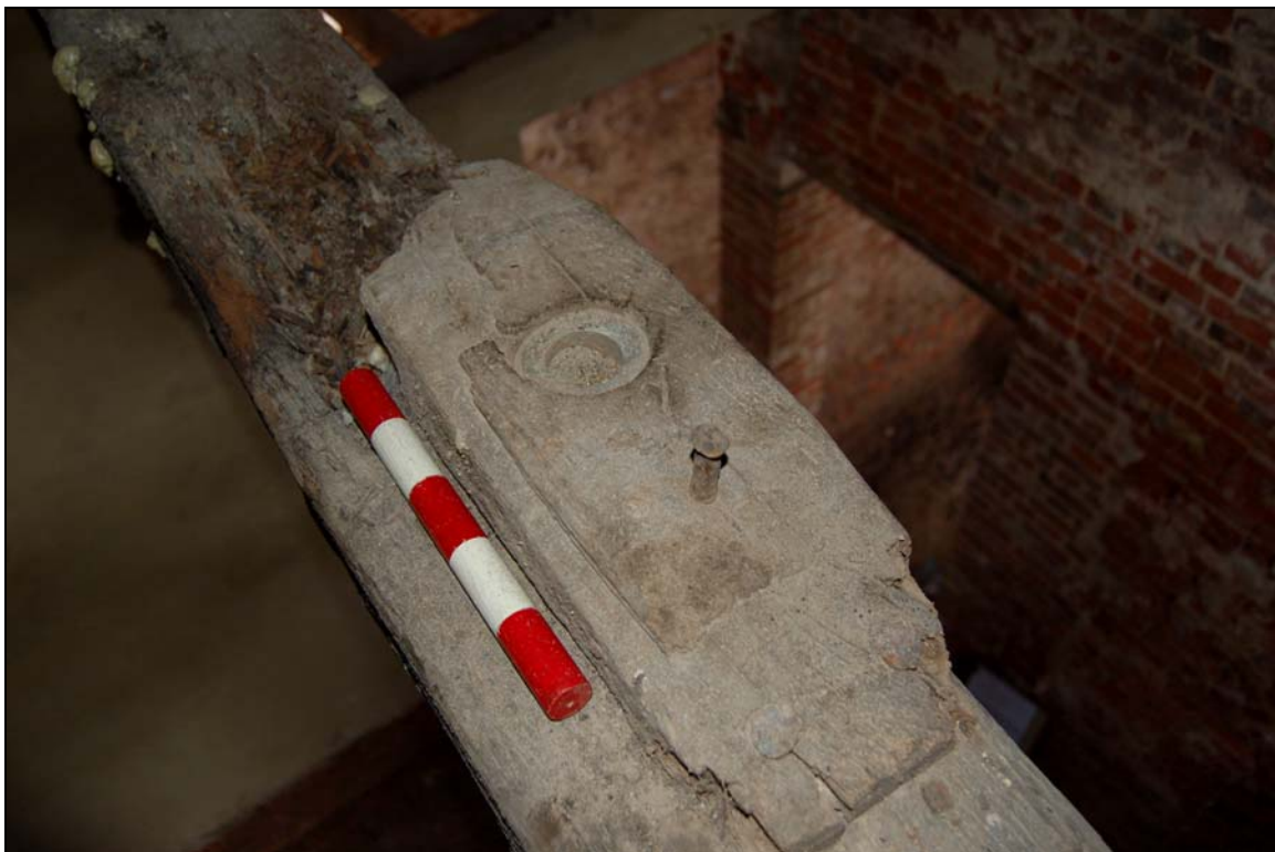
Plate 15 Detail of cowl shaft base
