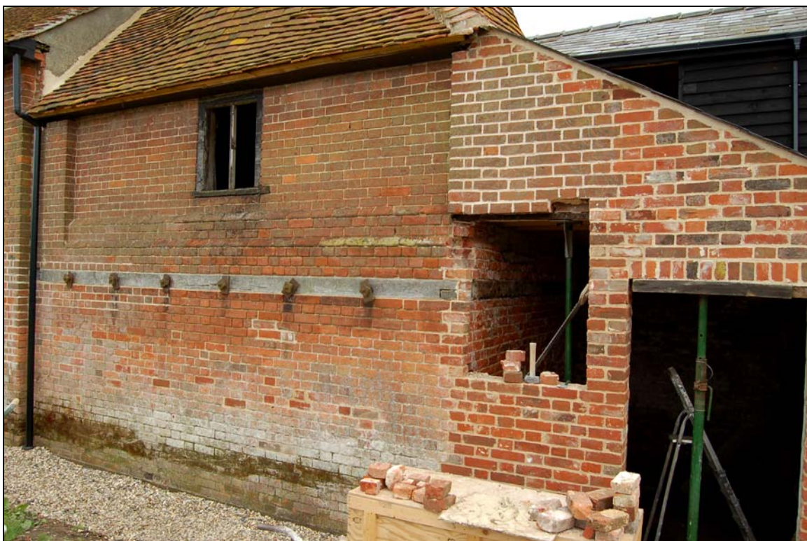
Plate 12 Tension bolts for wire mesh kiln floor and fuel store
