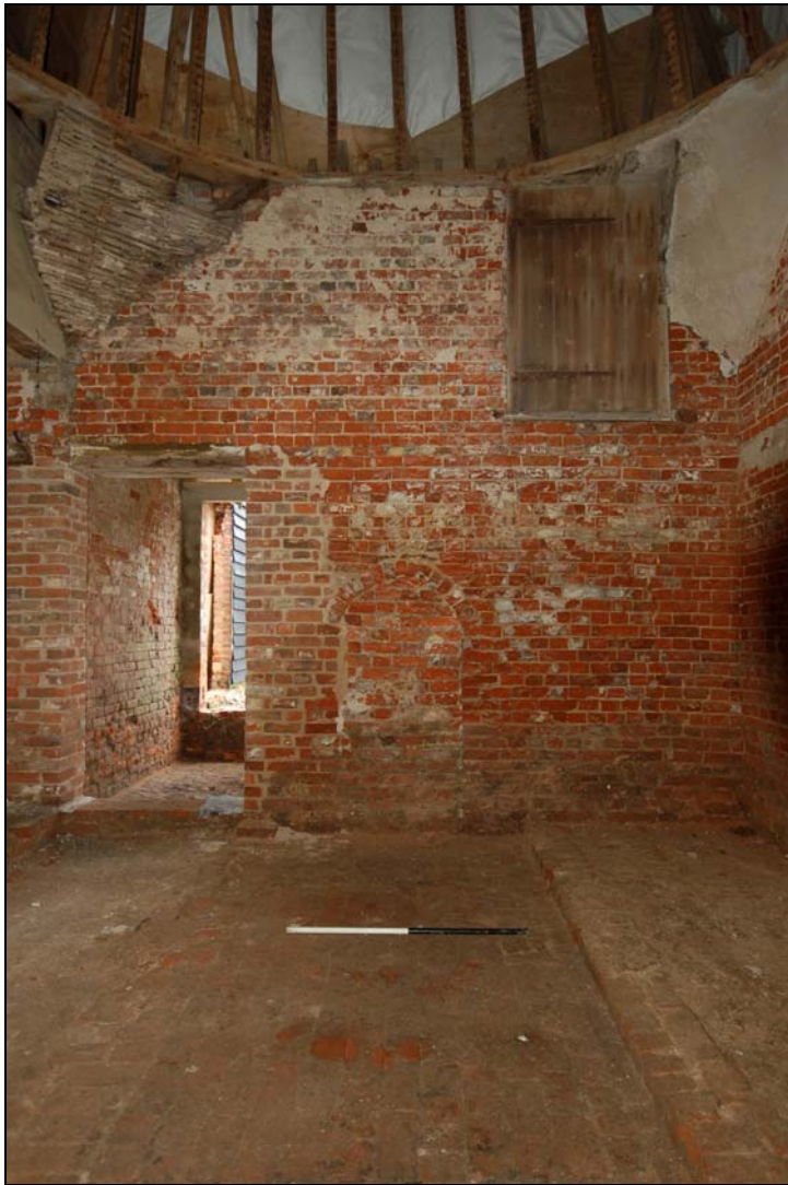
Plate 13 Remains of kiln furnace and blocked stoke hole
