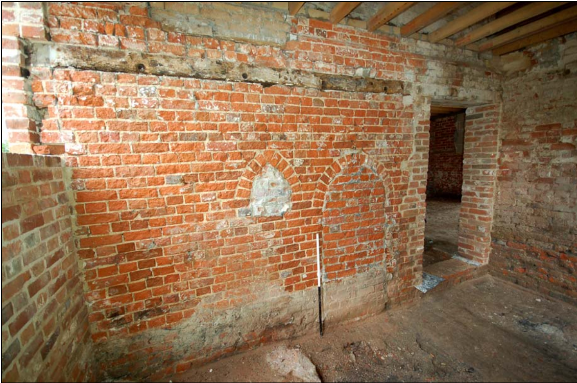
Plate 19 Blocked stoke hole and wall recess inside fuel store
