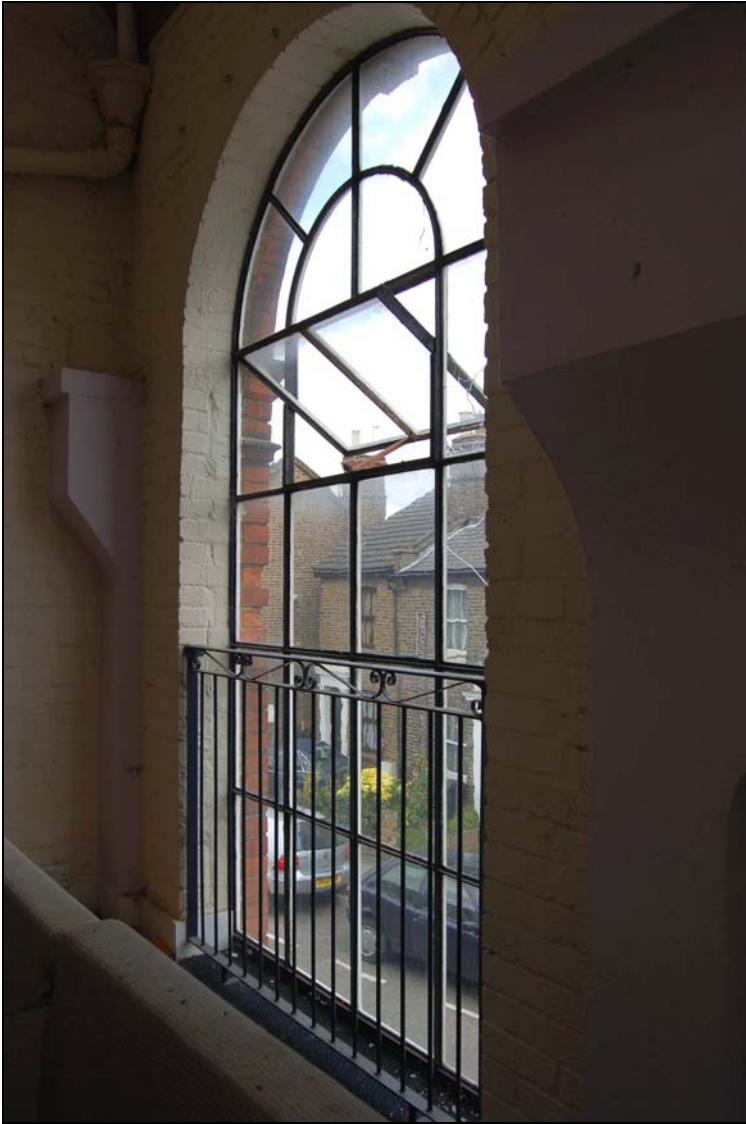
Plate 15 Detail of iron-framed window on north wall
