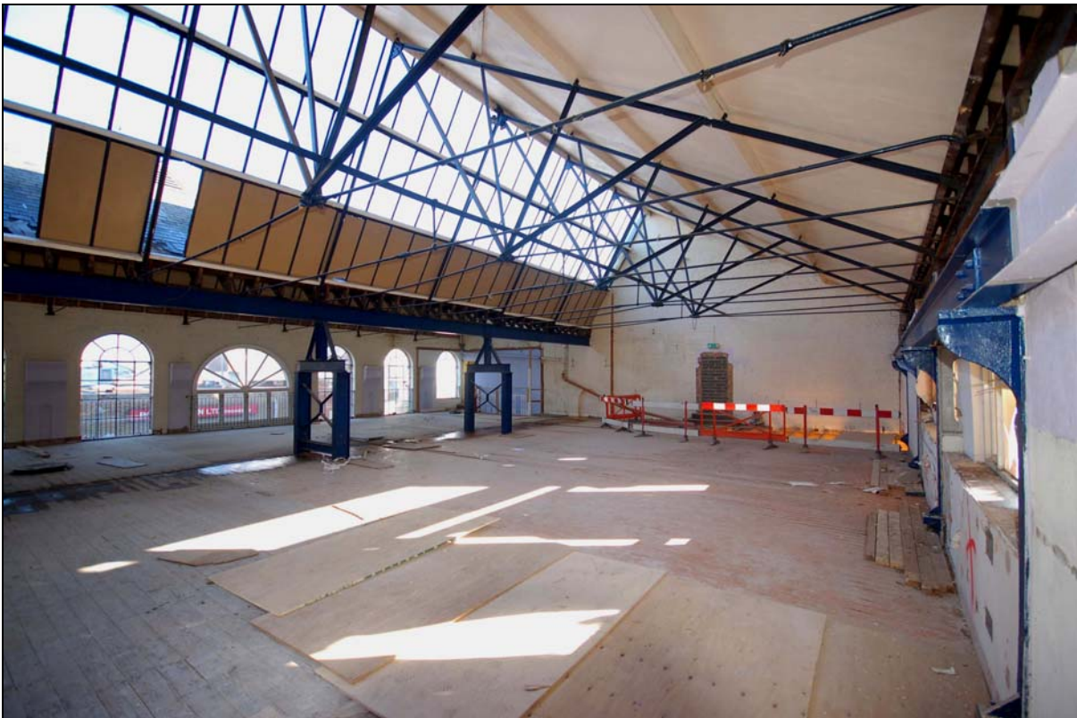
Plate 12 Top floor of gym after strip, viewed from south-west
