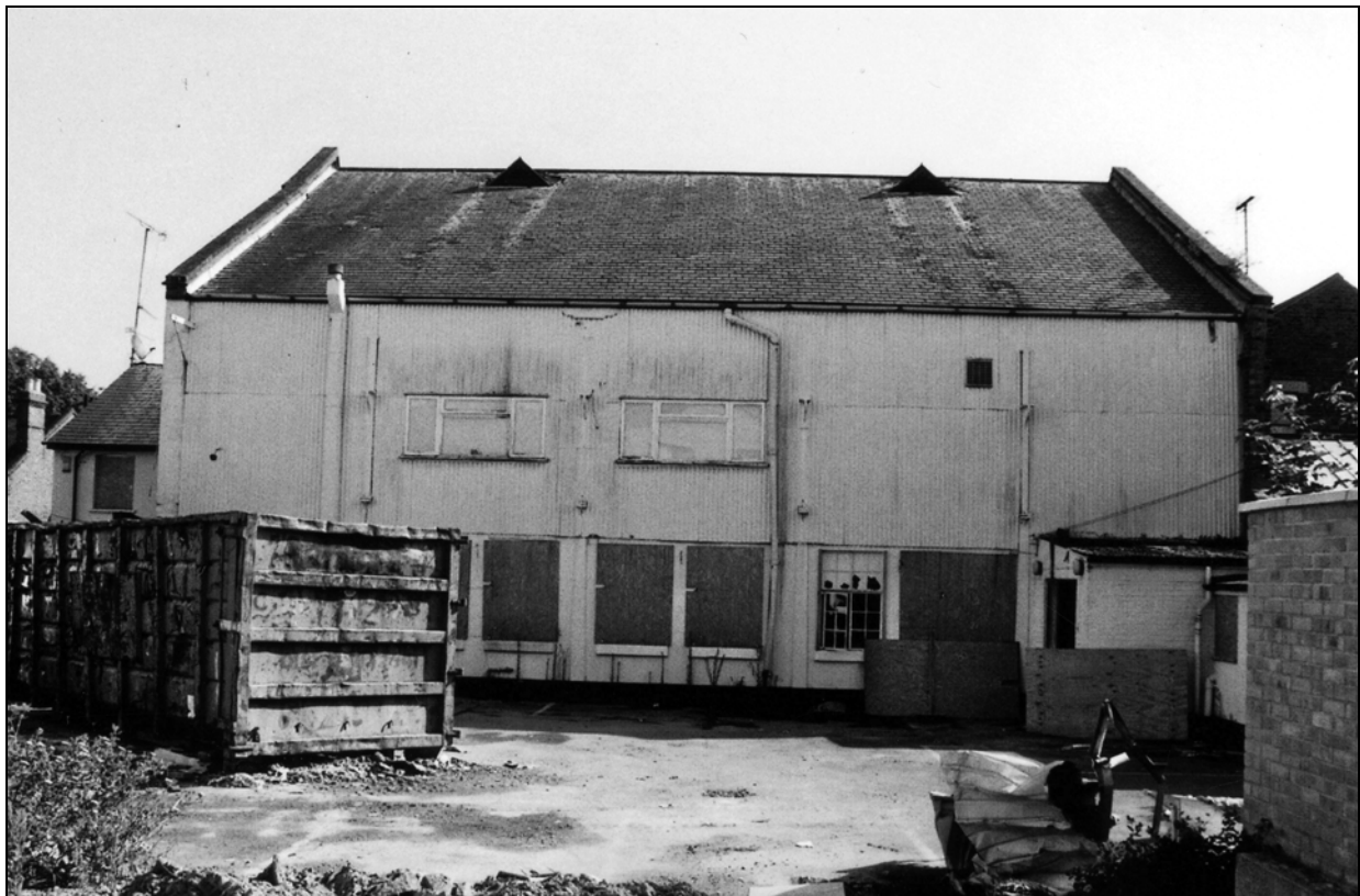
Plate 4 Re-built rear (south) elevation of engine house
