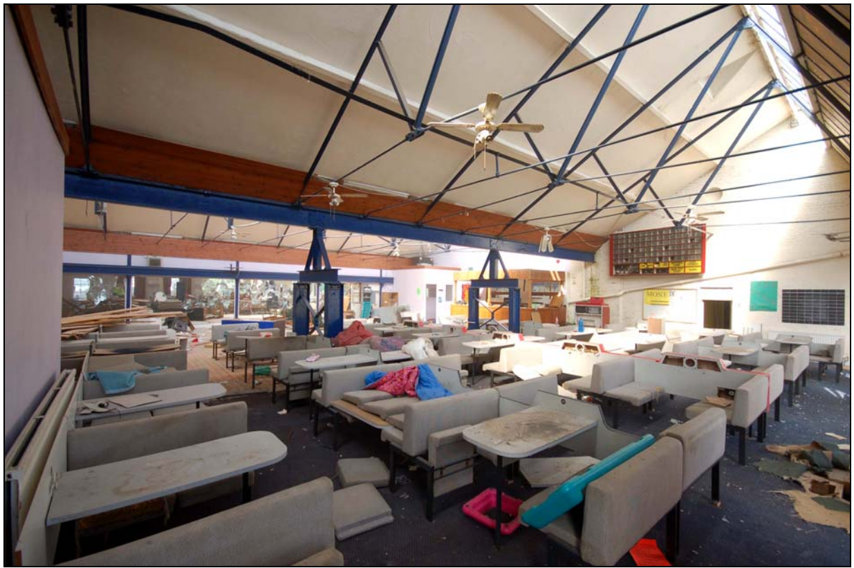
Plate 10 Top floor of gym before strip, viewed from north-east
