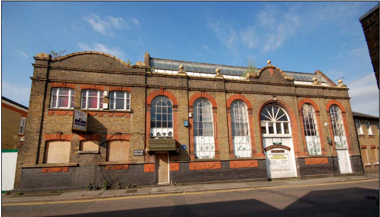
Plate 1 Listed Anchor Street frontage
