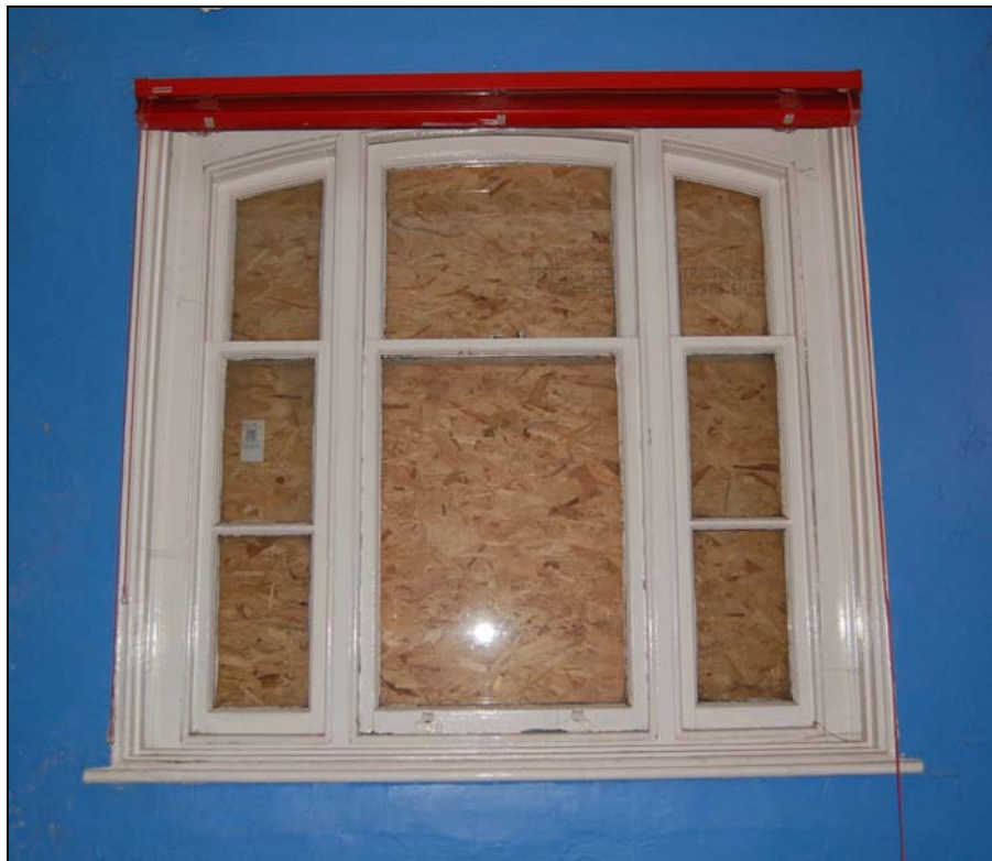
Plate 18 Detail of front office window
