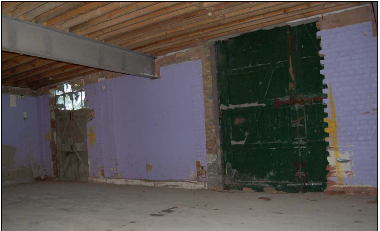
Plate 8 Original doors into engine house from Anchor Street
