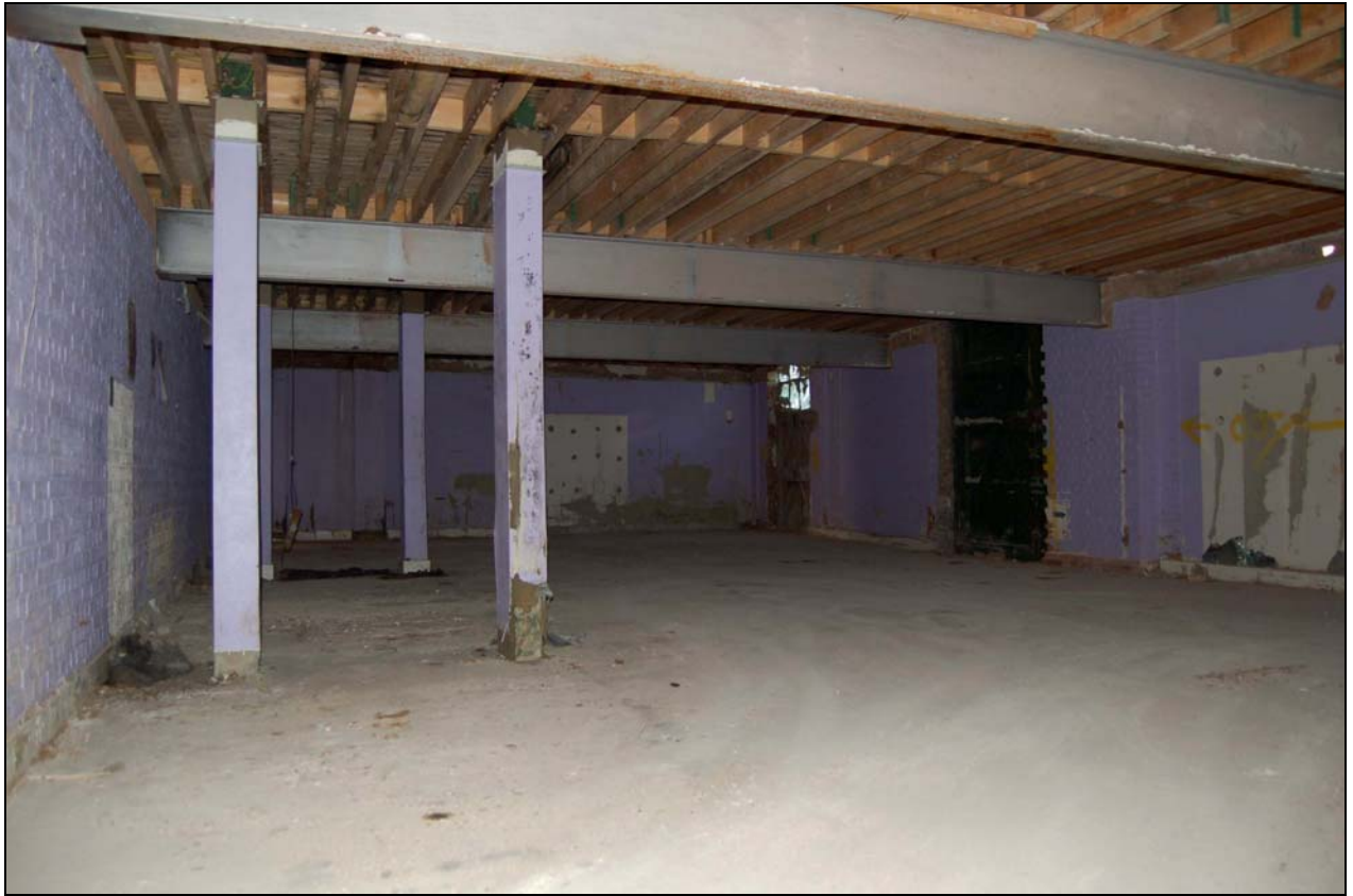
Plate 7 Ground floor (north) of engine house viewed to west
