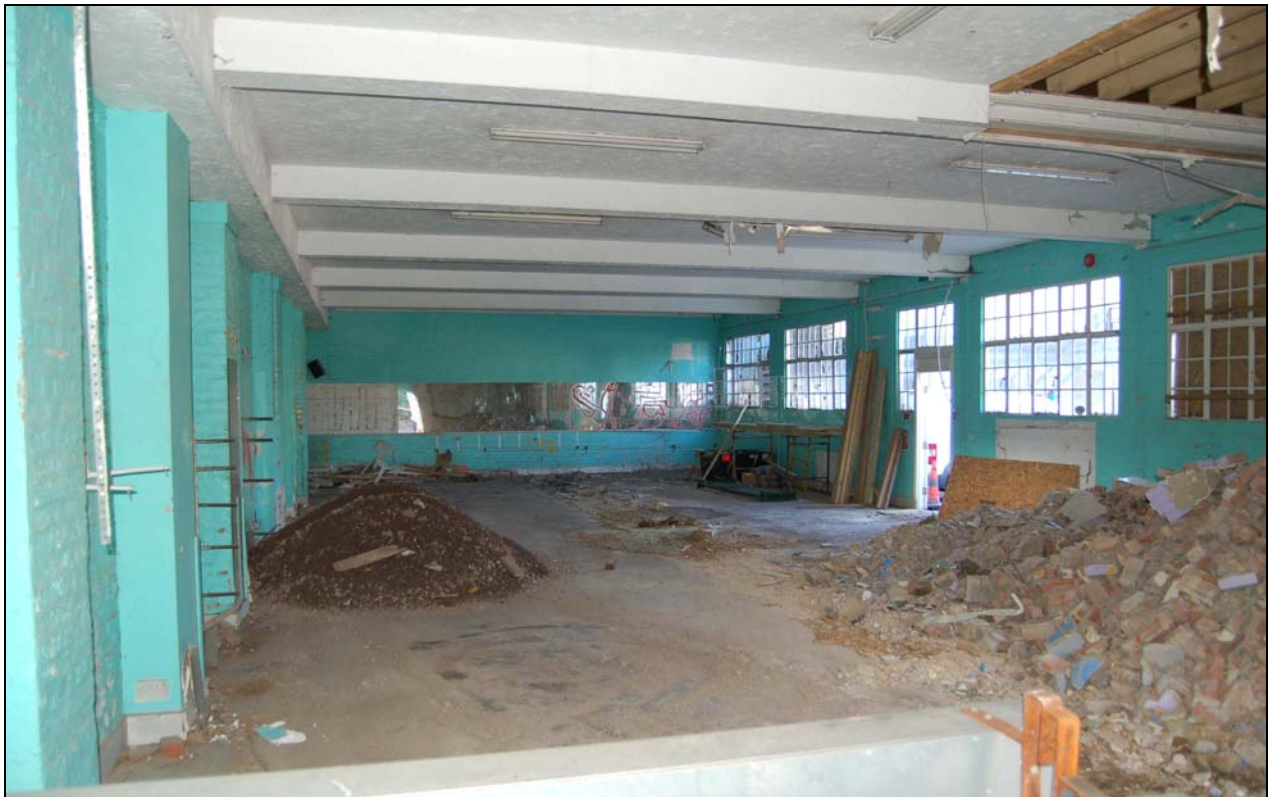
Plate 26 Interior of warehouse 5/boiler house viewed to west
