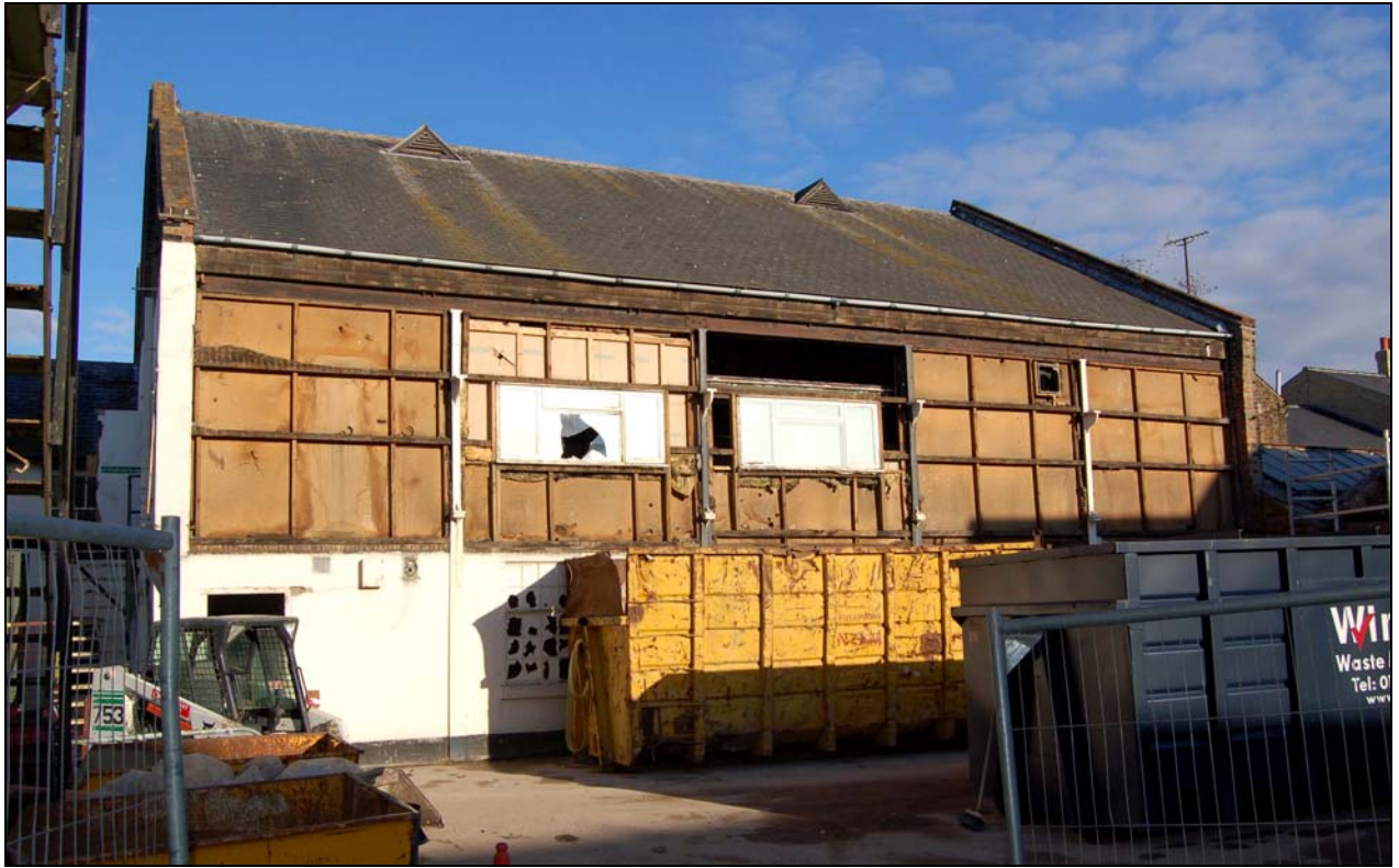
Plate 5 Rear elevation of engine house after cladding removed
