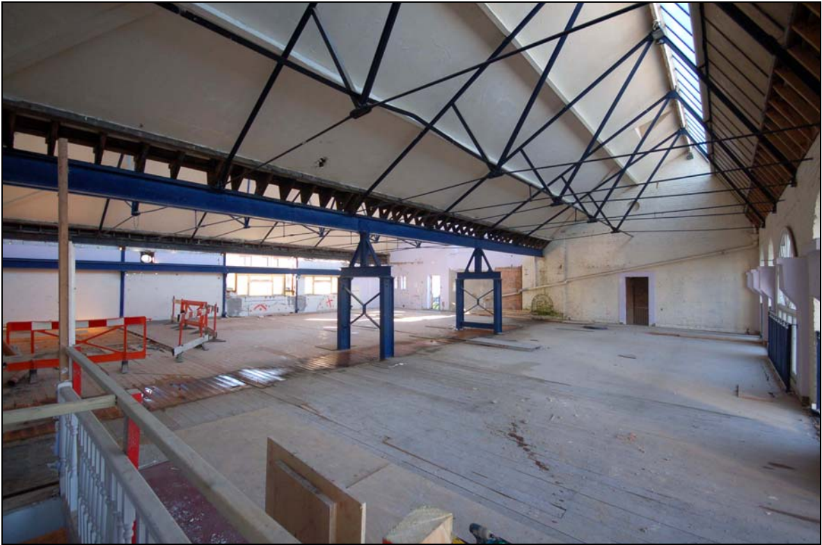
Plate 11 Top floor of gym after strip, viewed from north-east
