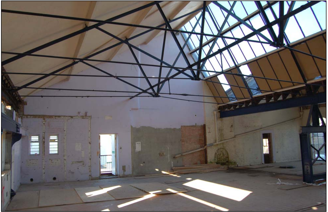
Plate 13 Removed chimney scar on west wall of engine house
