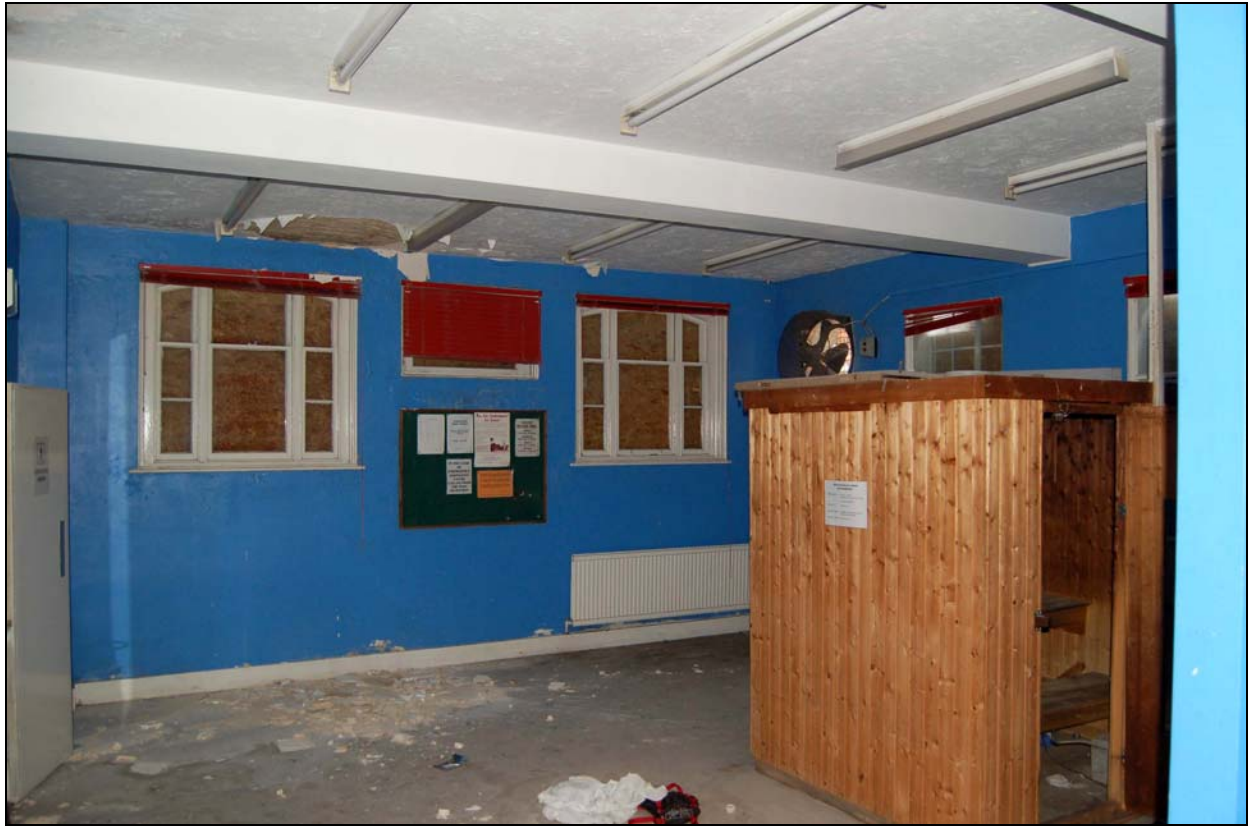
Plate 17 Ground floor office interior north wall before strip
