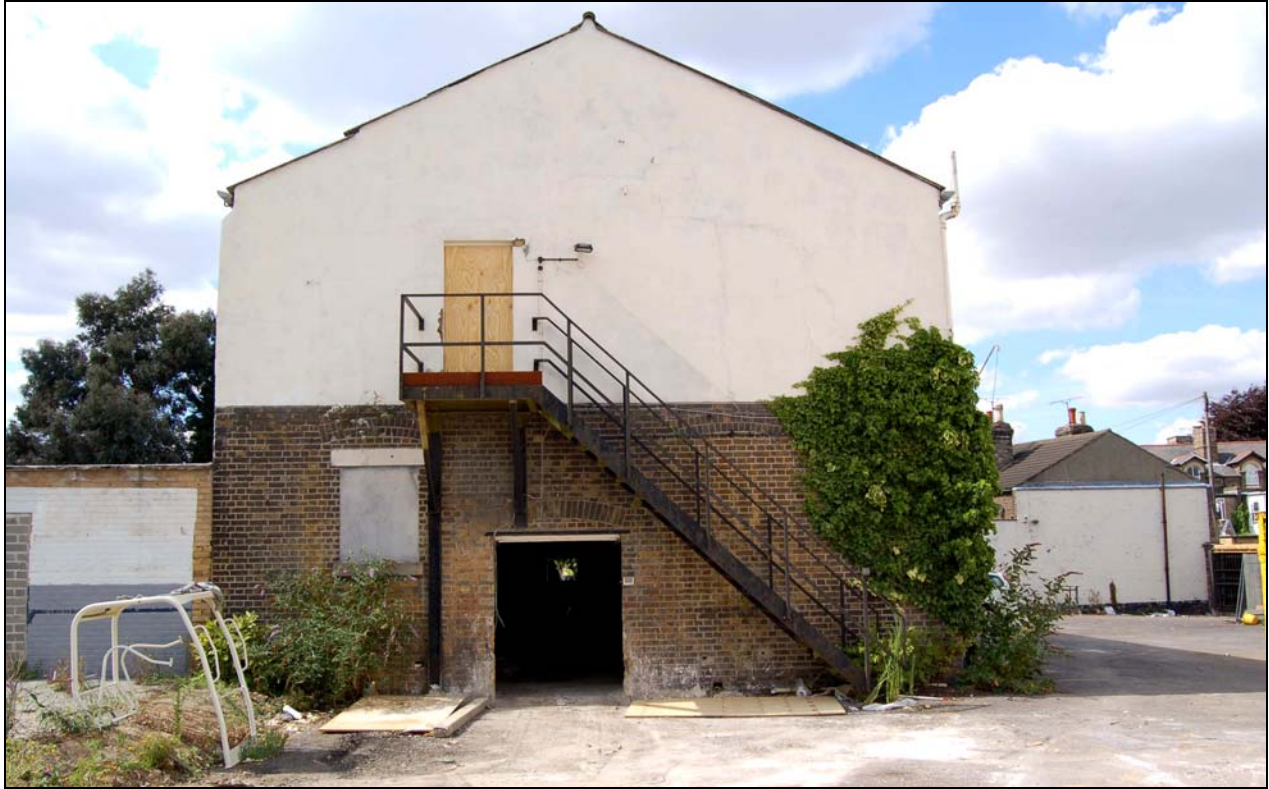
Plate 25 East wall of boiler house incorporated into warehouse 5 wall
