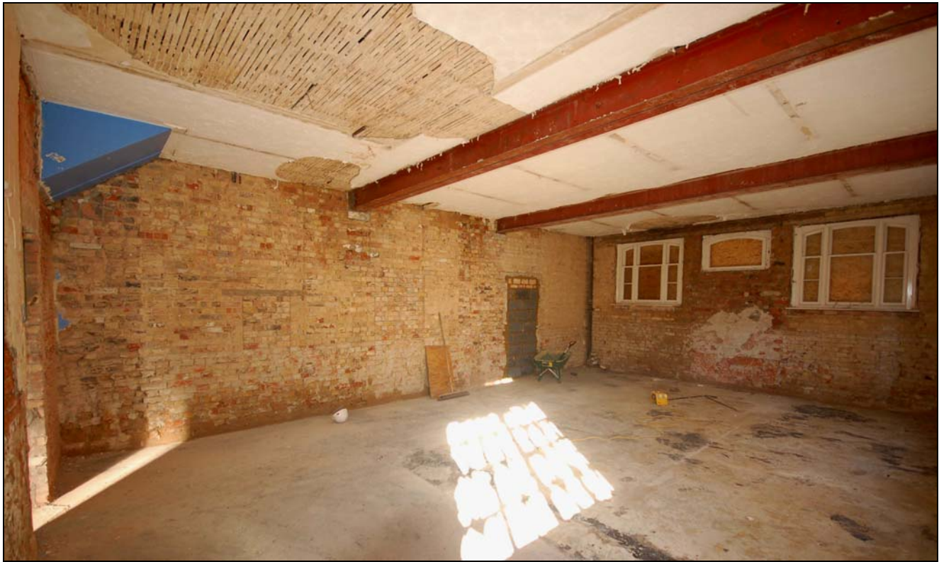
Plate 20 Blocked areas in front (north) part of office after strip
