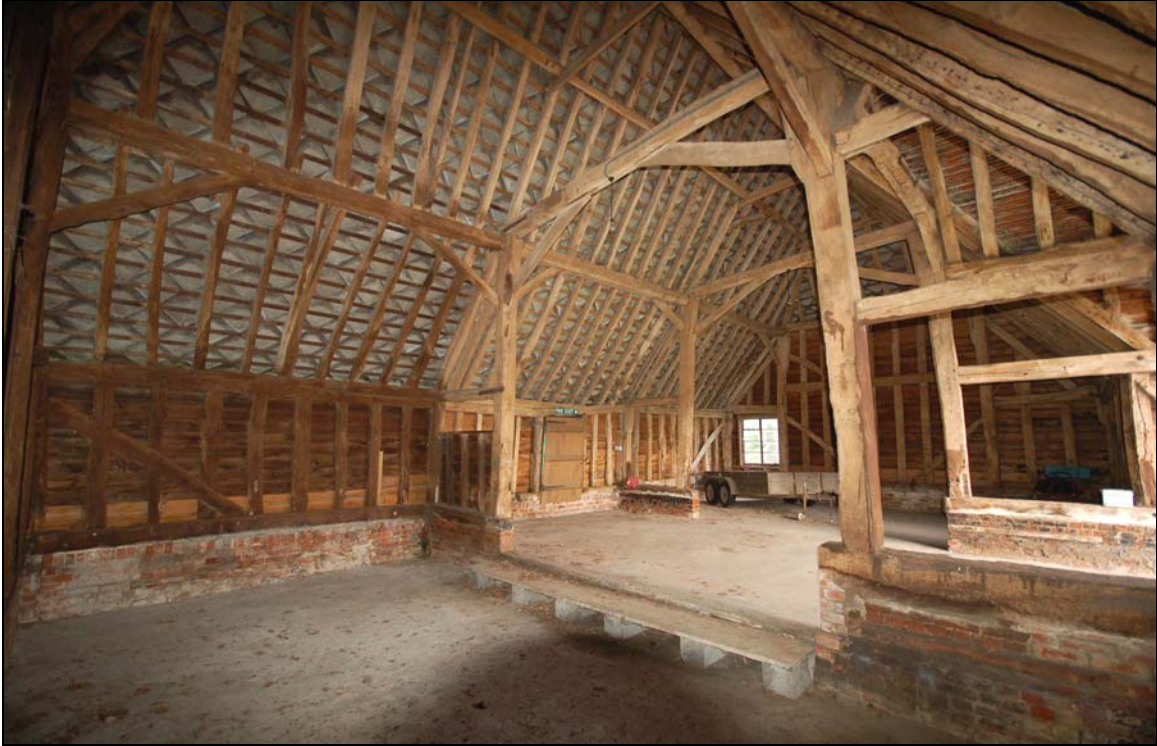
Plate 7 Interior of barn 1 viewed from south-west
