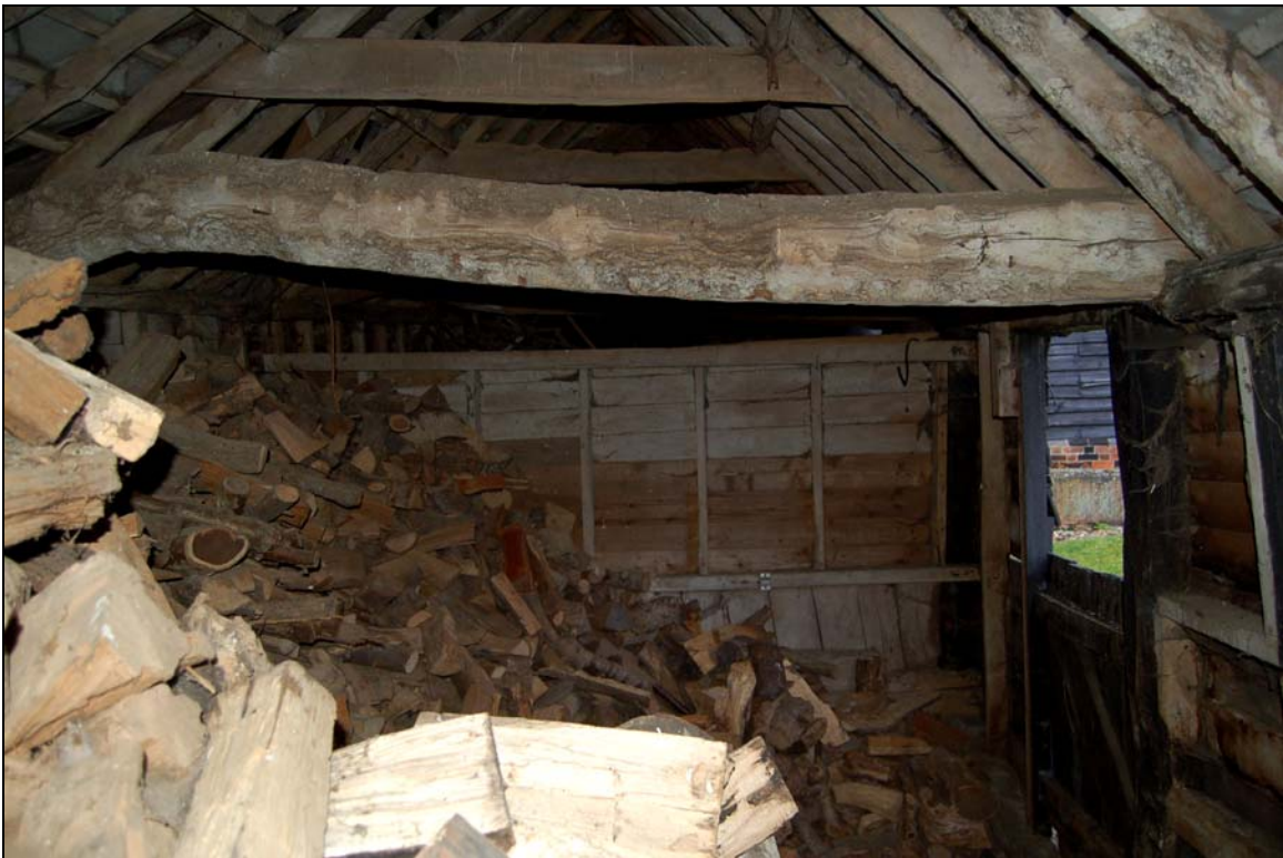
Plate 18 Interior of shelter shed 3
