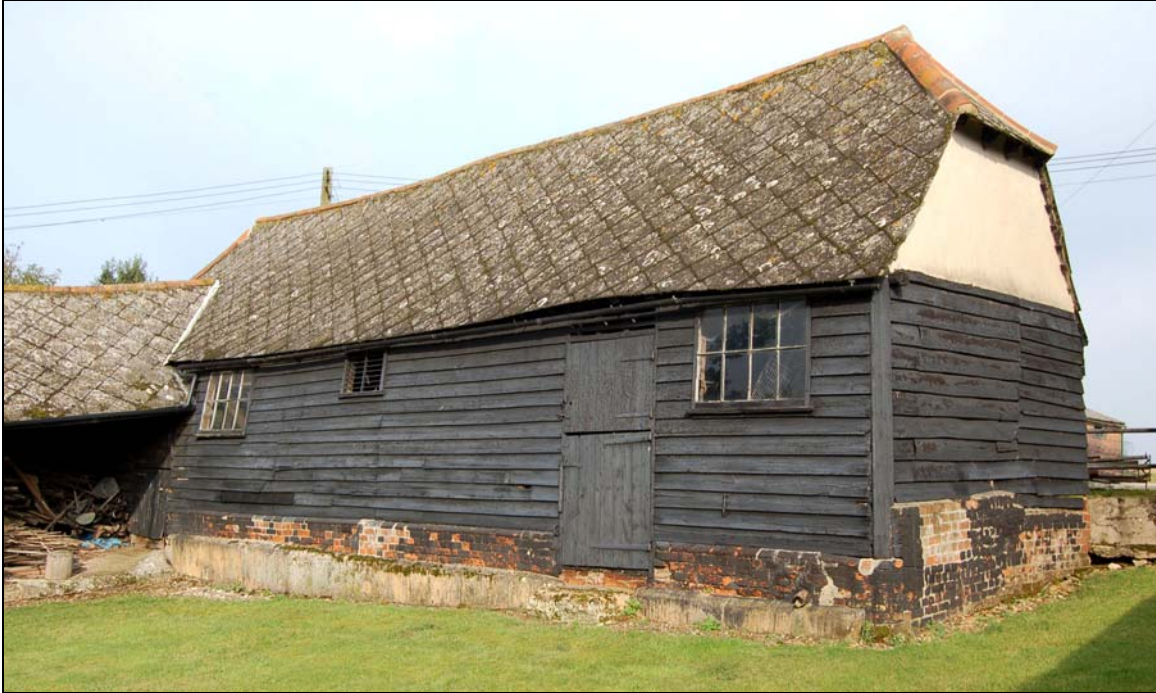
Plate 19 East elevation of byre 4
