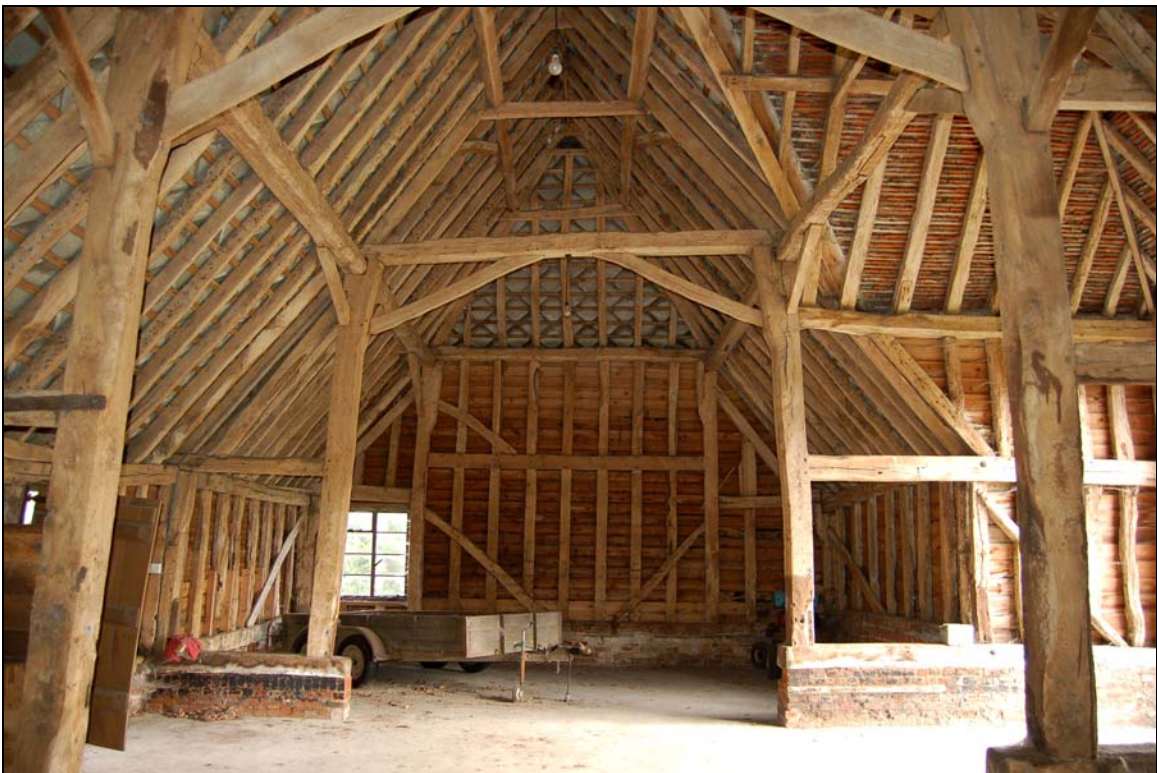
Plate 8 Interior of barn 1 viewed to east end
