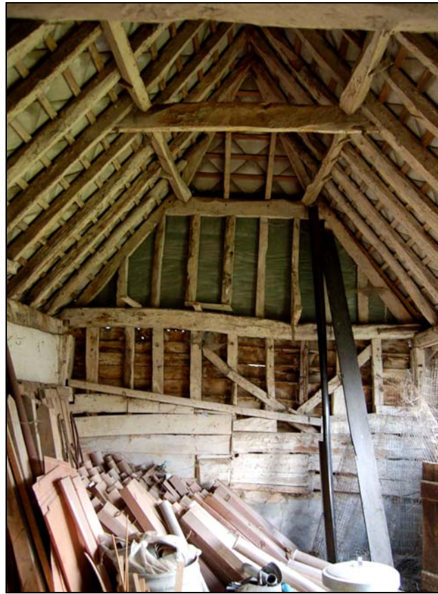
Plate 24 Secondary south wall of byre
