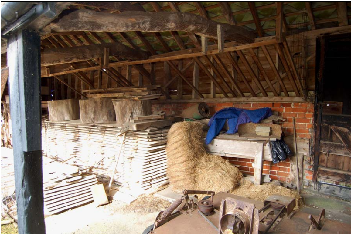
Plate 28 Interior of shelter shed 6 showing original fixtures
