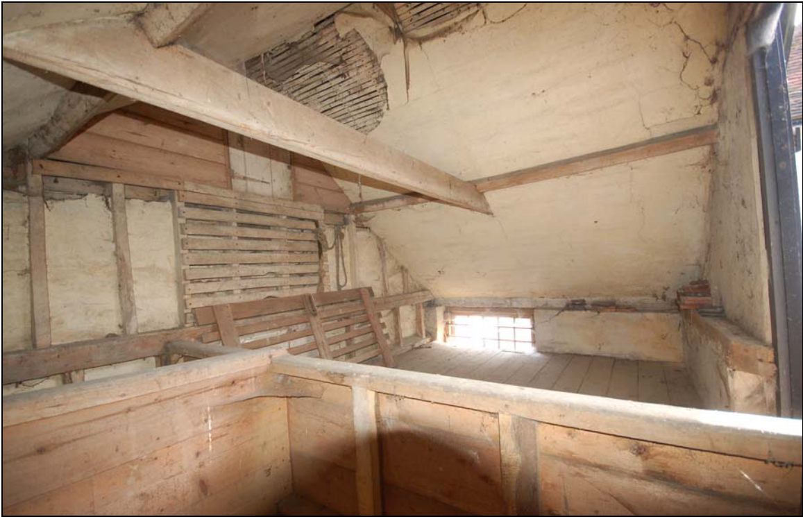
Plate 45 Loft interior viewed from bins on north side
