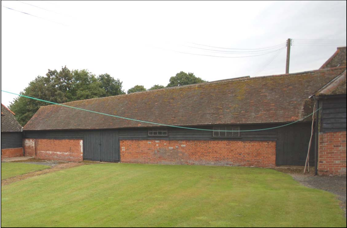
Plate 13 Rear elevation of shelter shed 2 viewed from west
