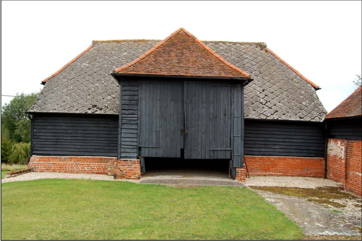
Plate 5 Front view of barn 1
