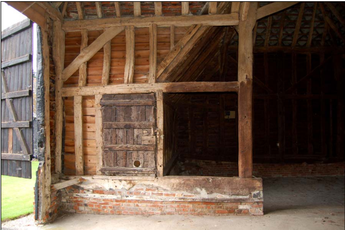
Plate 12 Midstrey west wall in barn 1, showing door
