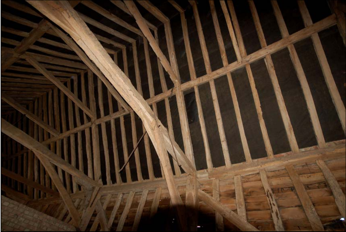
Plate 33 Detail of butt-purlin roof in barn 7
