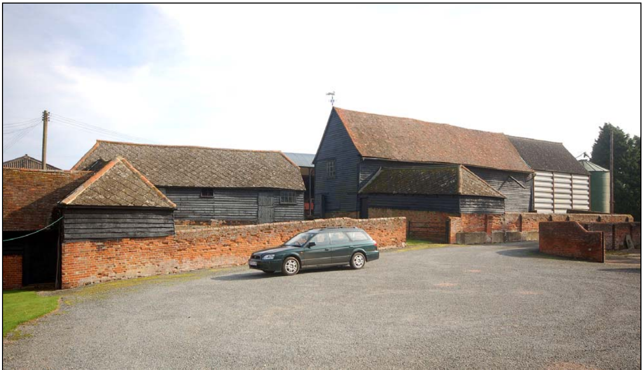
Plate 2 View across tarmac yard to yards B & C (east)
