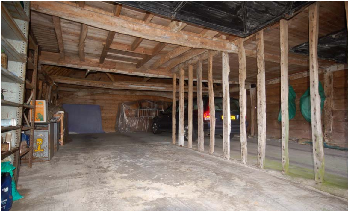
Plate 40 Interior of granary 10 viewed to south partition wall showing granary above
