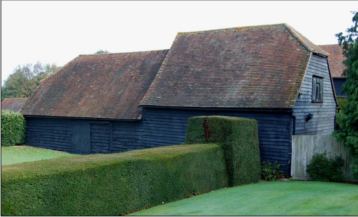
Plate 37 Exterior of machine store 9 & granary 10 from south-west
