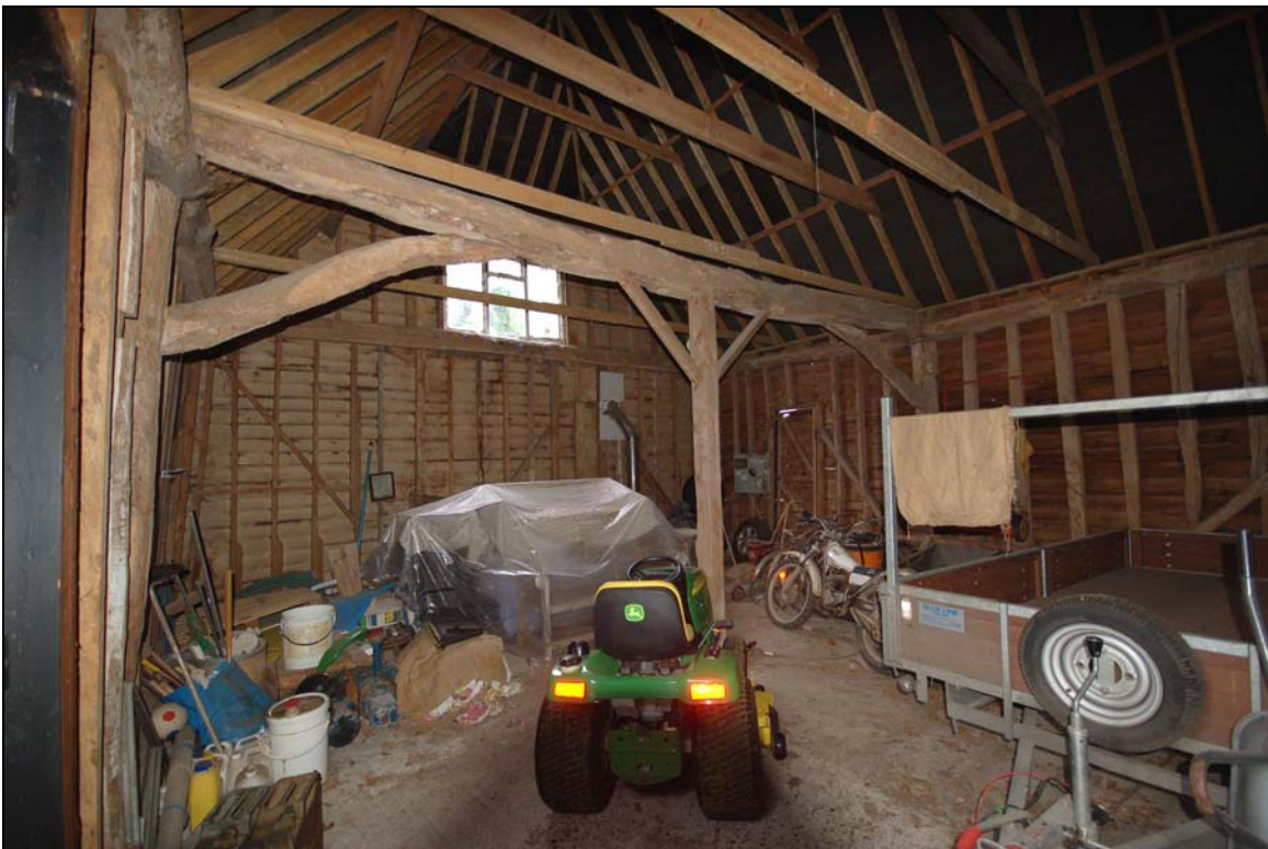
Plate 38 Interior of machine store 9 showing in-filled south wall
