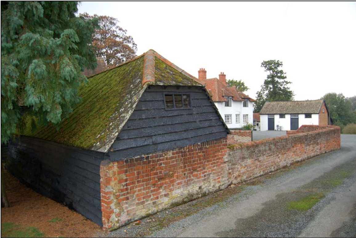
Plate 35 Under-built east wall of shelter shed 8 with stables 11 & farmhouse in background
