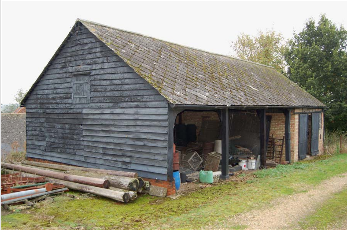
Plate 25 Bull pen/cart shed viewed from south-east
