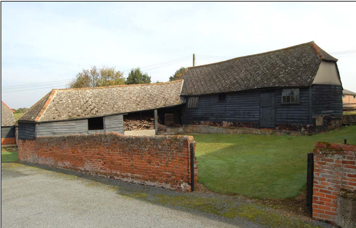
Plate 16 Yard B with shelter shed 3 & byre 4
