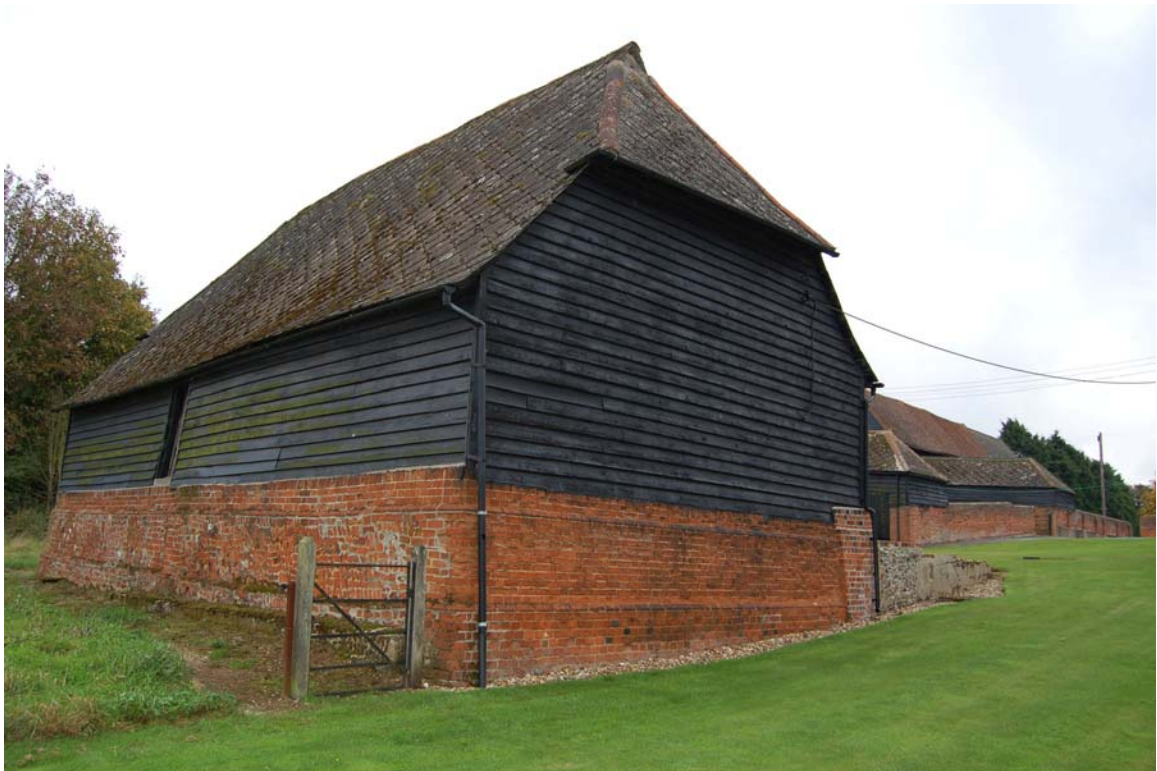
Plate 6 Barn 1 viewed from north-west up slope toward yard B
