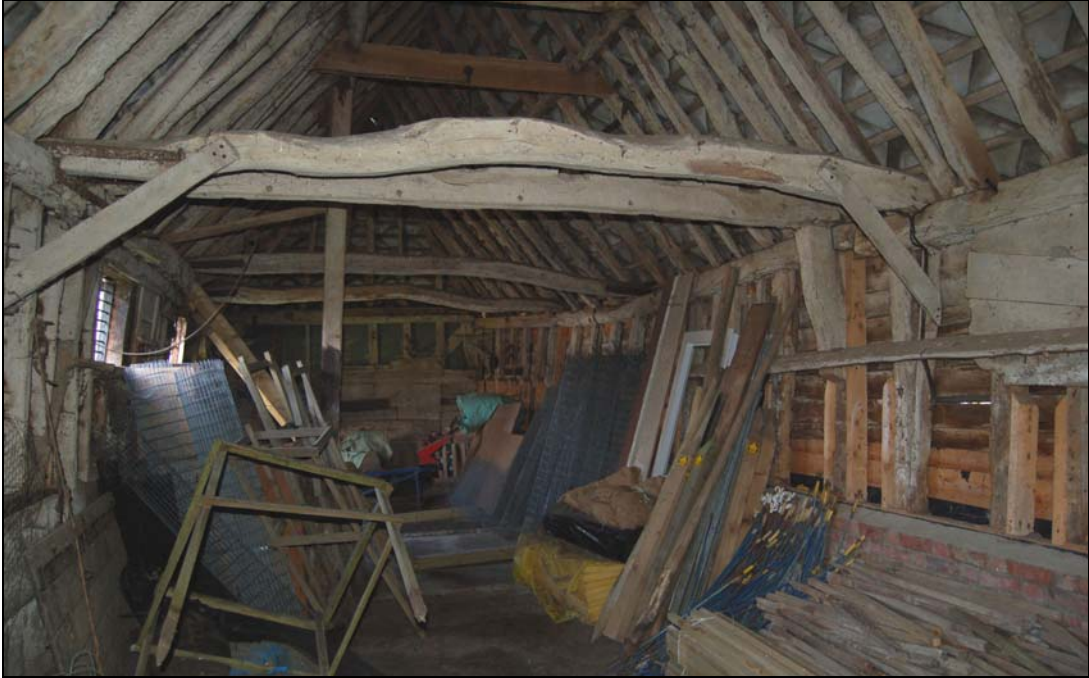
Plate 21 Interior of byre from south extension
