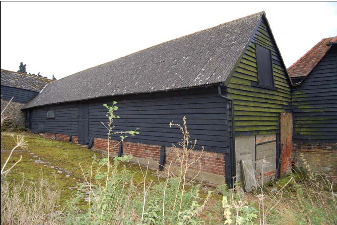
Plate 14 In-filled open front of shelter shed 2
