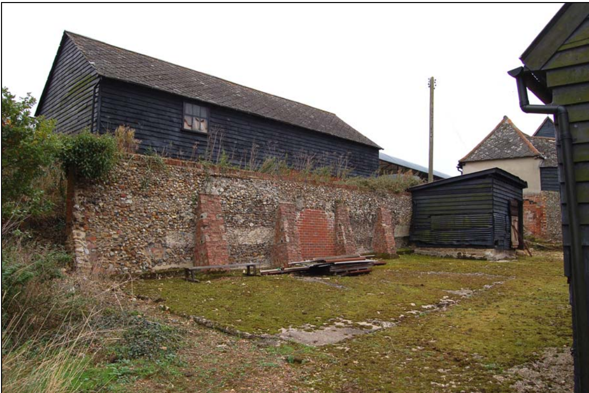
Plate 26 Rear of bull pen, flint retaining wall & modern shed in former stock yard
