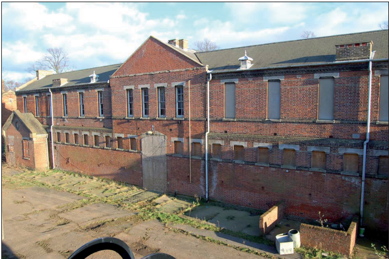
Plate 6 North-west elevation of stable block
