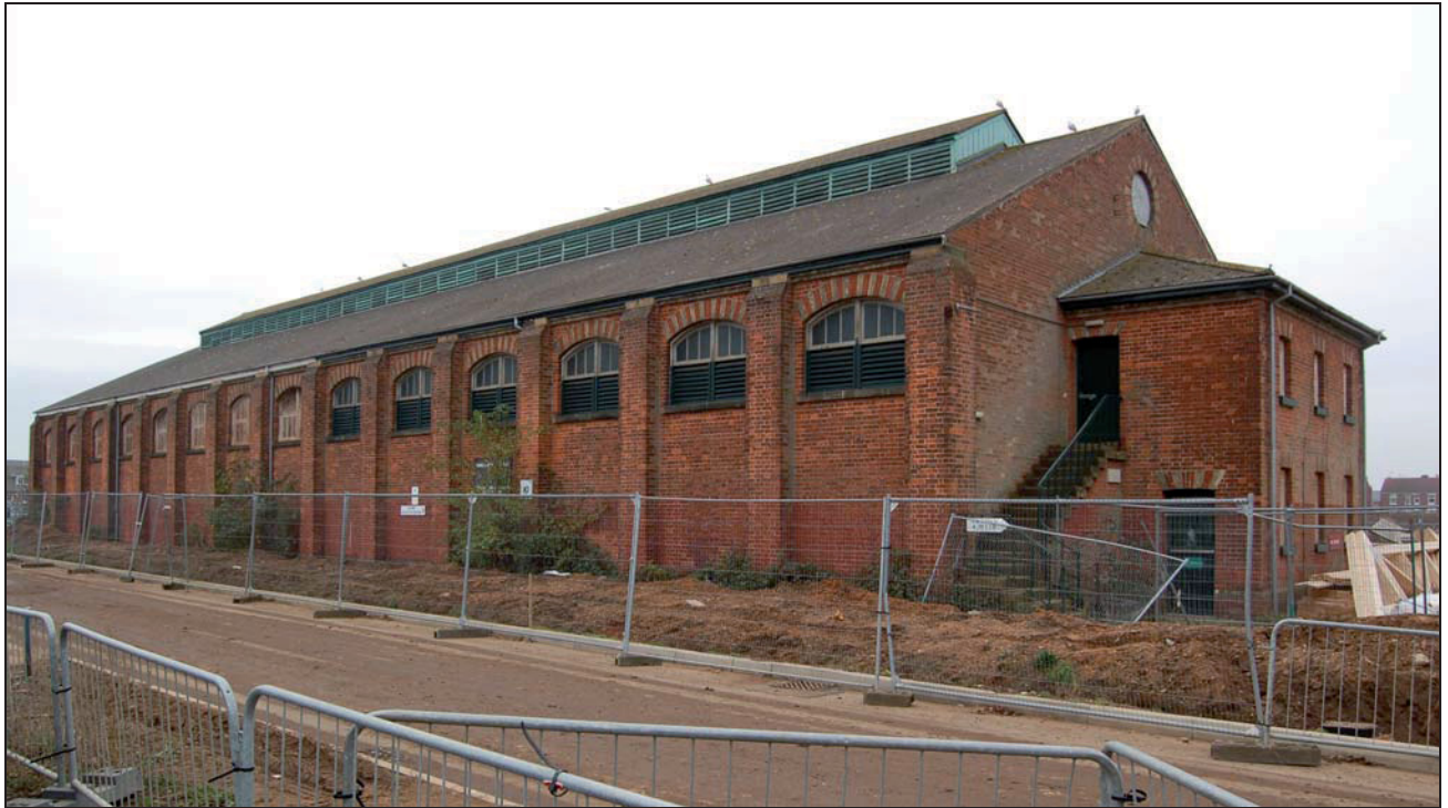
Plate 39 Main (south-east) elevation of riding school
