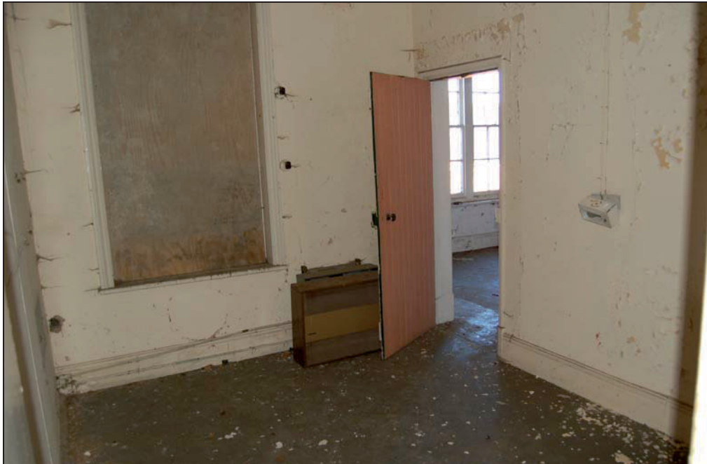
Plate 33 Interior of north-west training quarters in former recreation room
