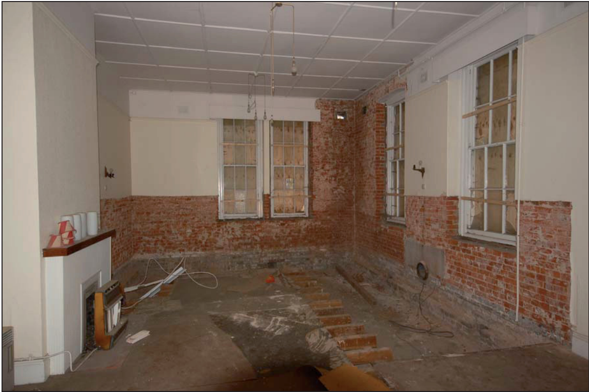
Plate 27 Tap room 4 partially stripped
