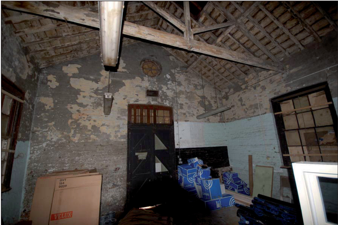
Plate 16 Interior of former forge
