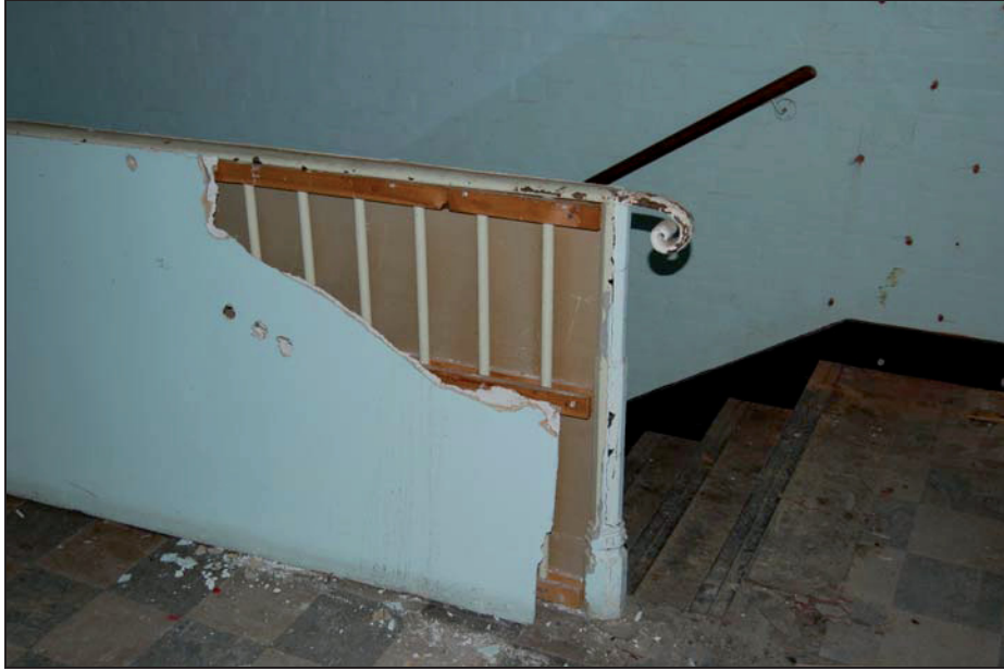
Plate 31 Balustrade on top landing
