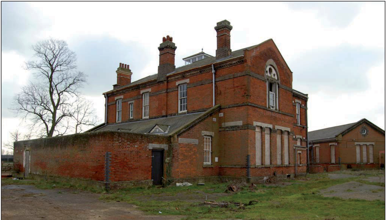
Plate 20 Canteen and sergeants mess viewed from north
