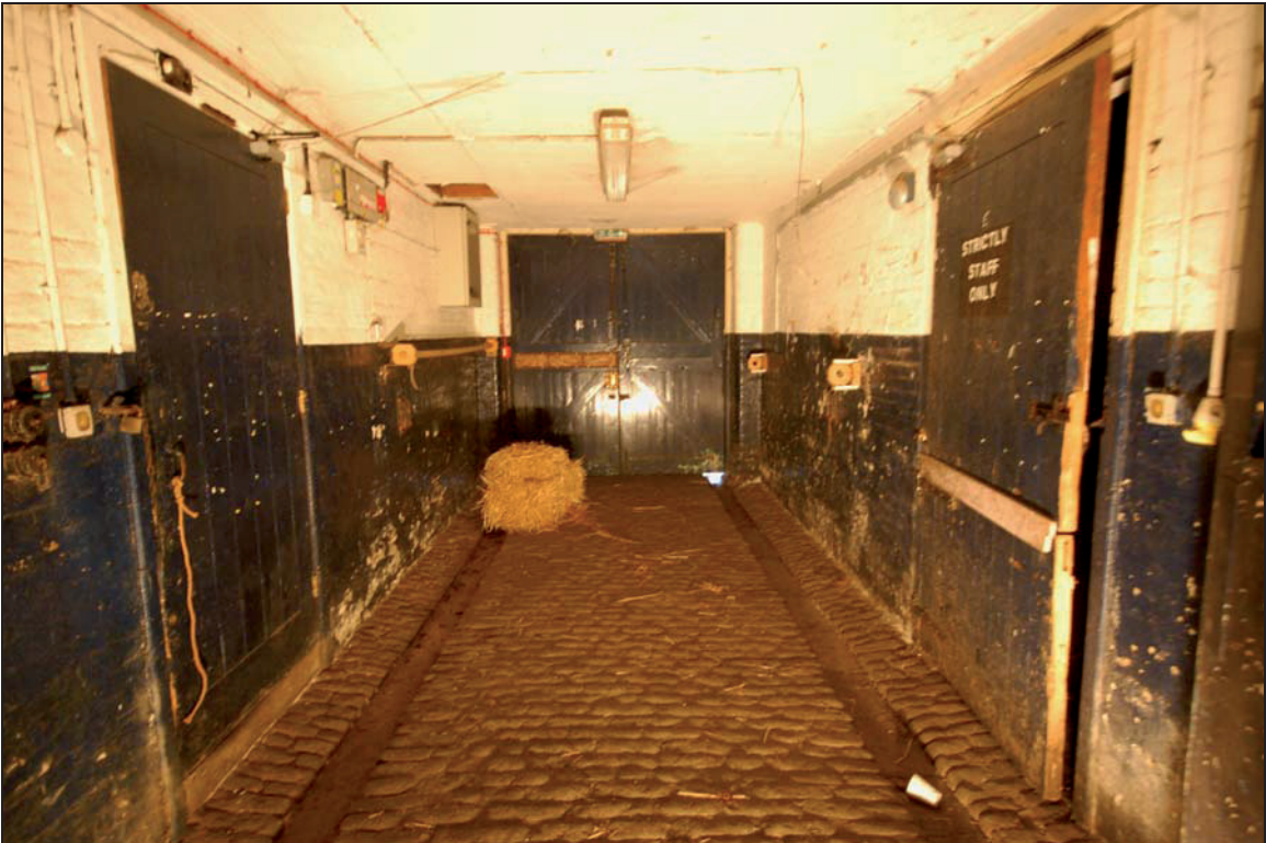
Plate 12 North-east stable door and drainage gully
