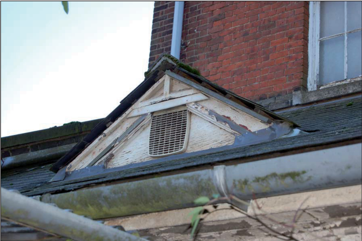
Plate 22 Roof vent above kitchen in sergeants mess
