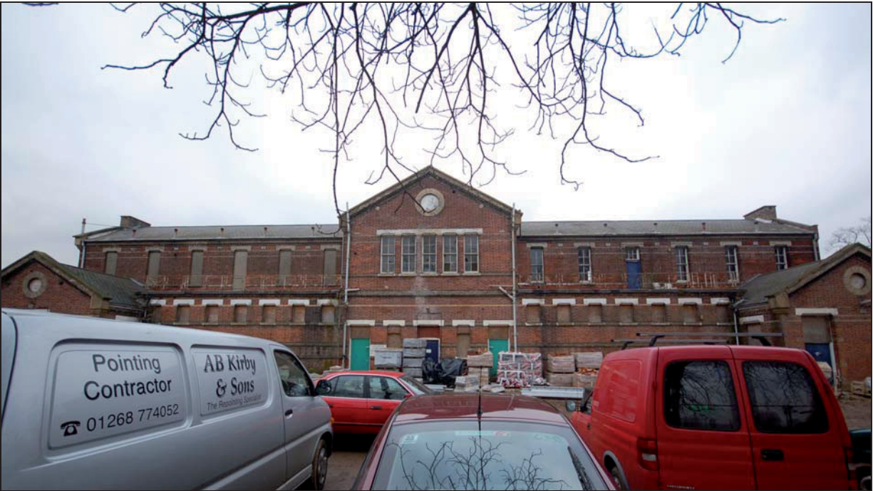
Plate 1 Main (north-east) façade to stable block A
