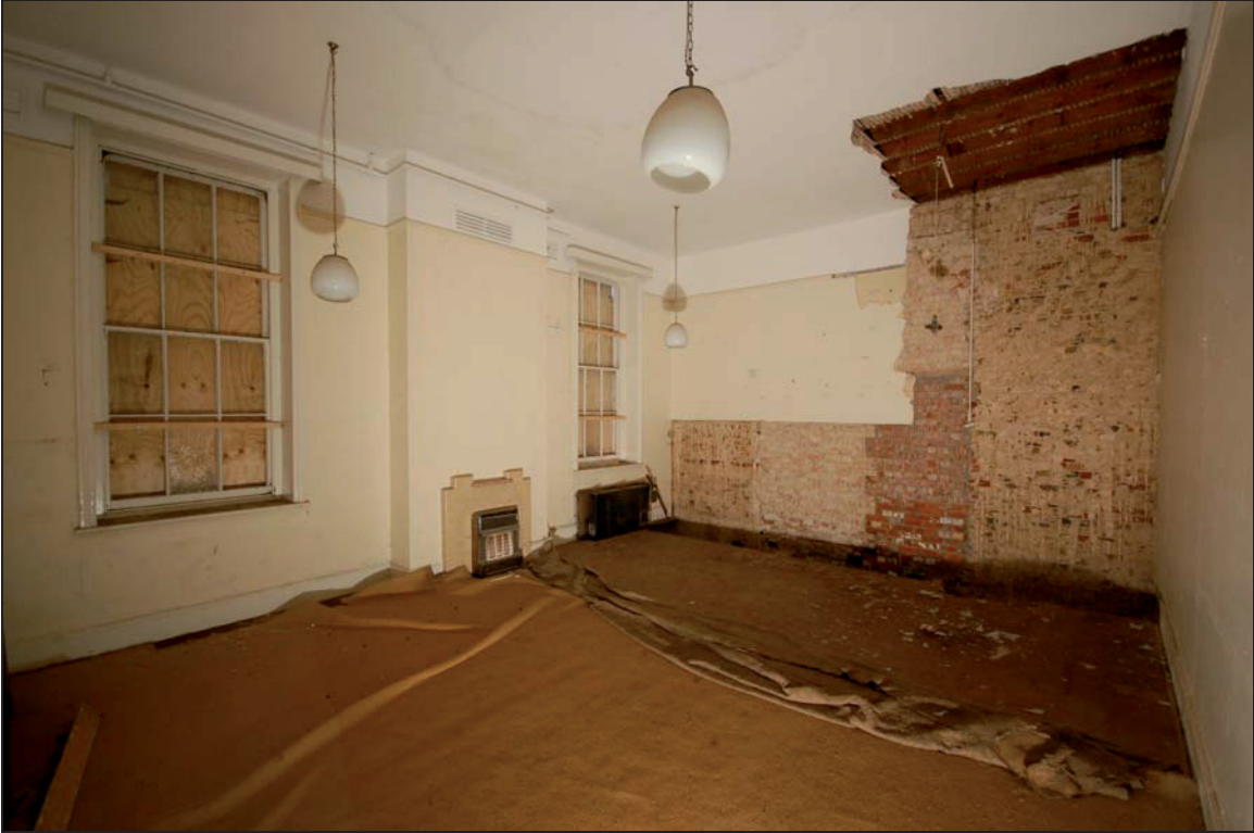
Plate 29 Billiard room 9 viewed to blocked former arch
