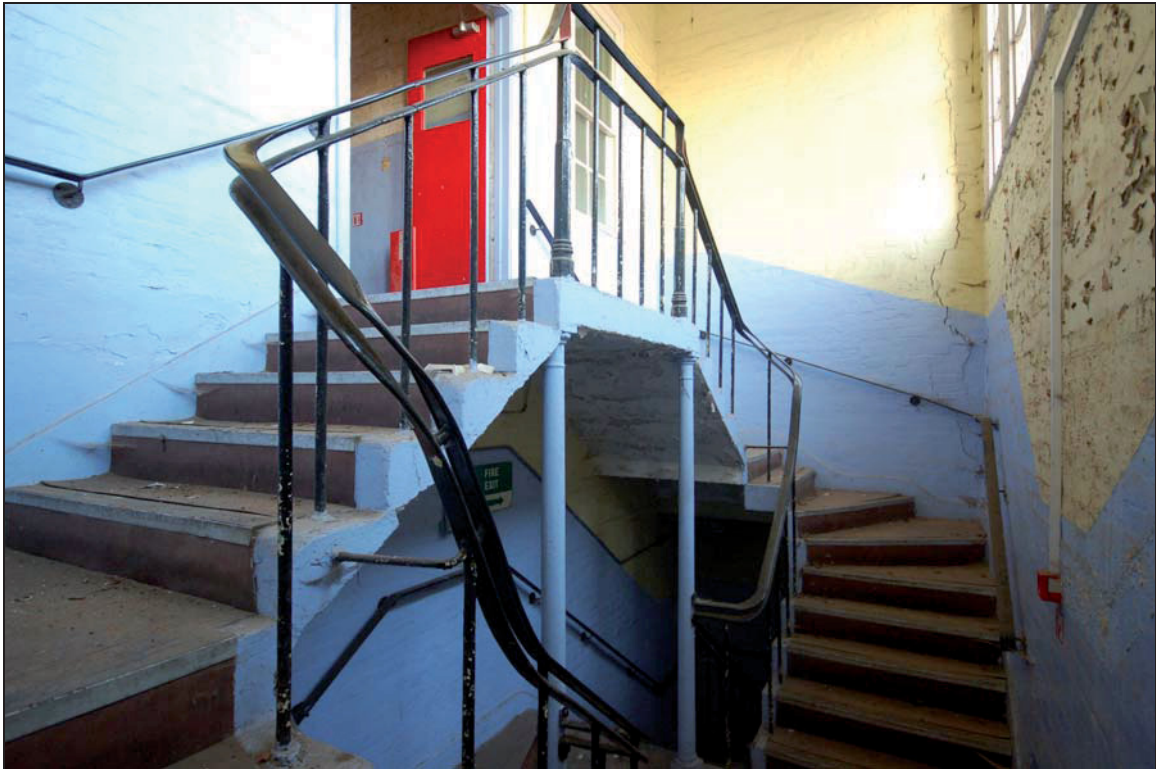
Plate 14 Stairs and barrack room landing
