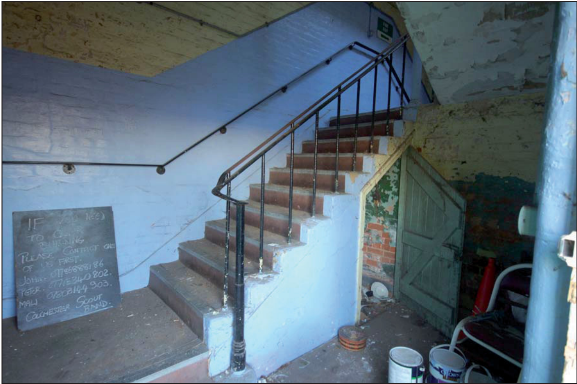
Plate 13 Stairs to barrack rooms
