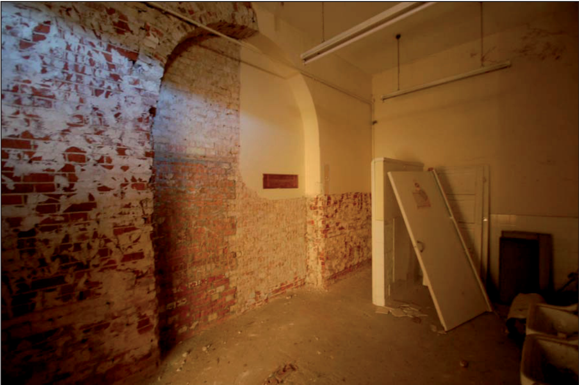
Plate 30 Blocked arch inside caterers room 10
