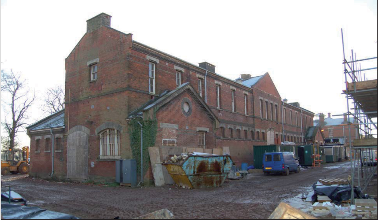
Plate 5 North-west and north-east elevations of stable block
