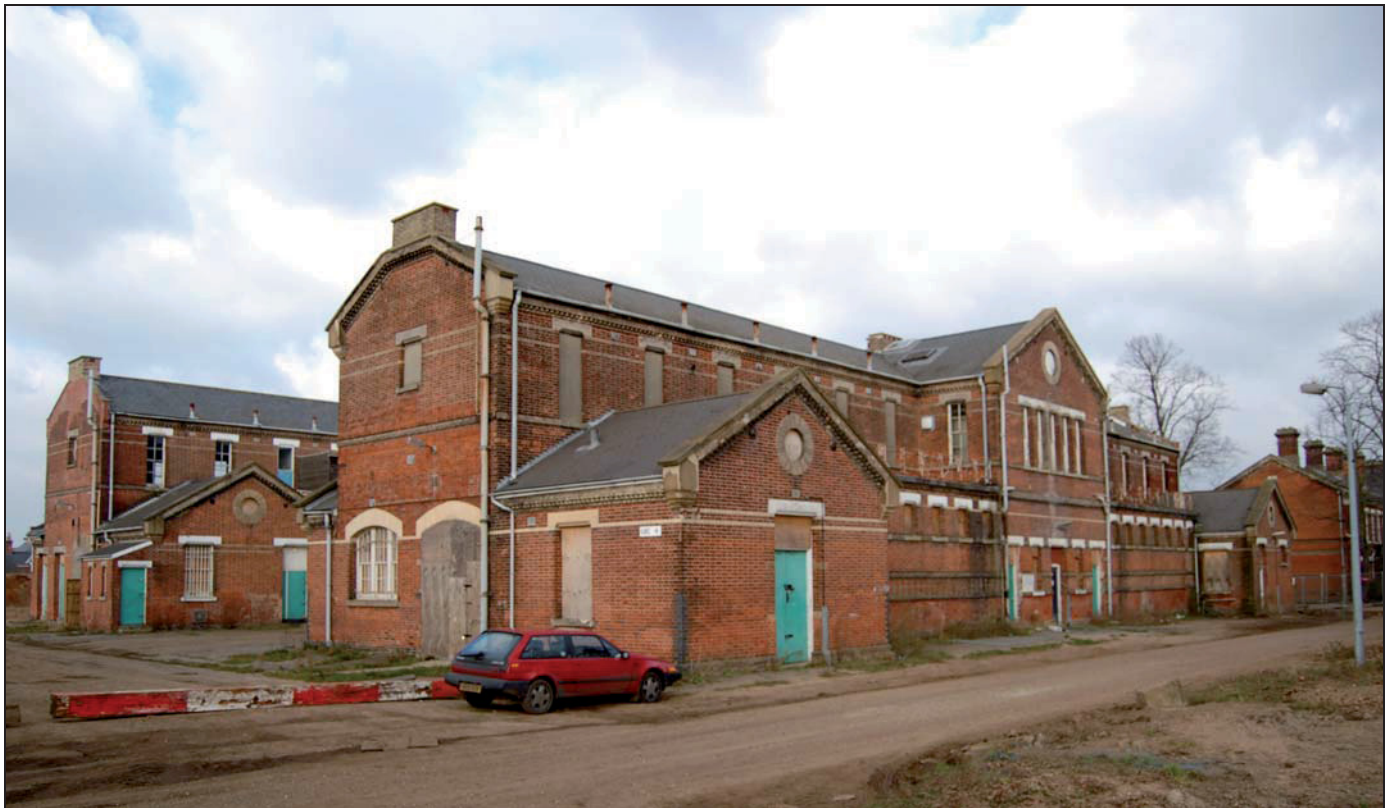
Plate 2 Stable blocks A & B viewed to north before conversion works started
