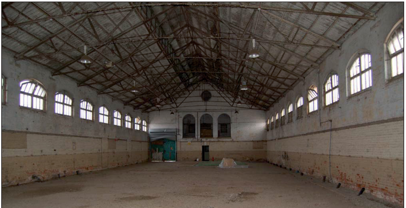
Plate 42 Interior of riding school viewed to gallery at north-east end
