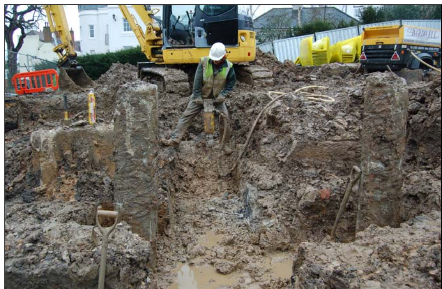
Plate 3 Removal of old concrete underpinning
