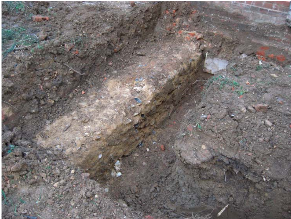
Plate 6. Trench 2 looking north-west, showing 16th-century flint wall 37 exposed during building works. As in Plate 5, the top of the wall had an even surface interpreted as supporting a timber-framed superstructure (the wall is 0.55m wide)
