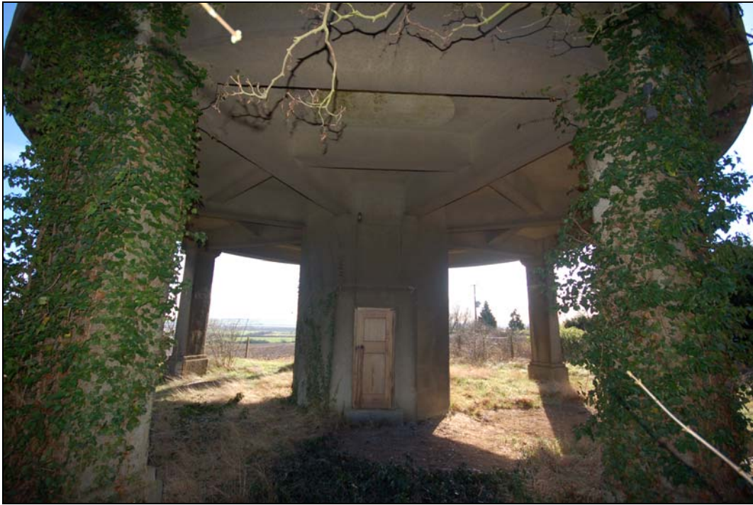
Plate 3 Entrance into tower and structural detailing to underside of tank
