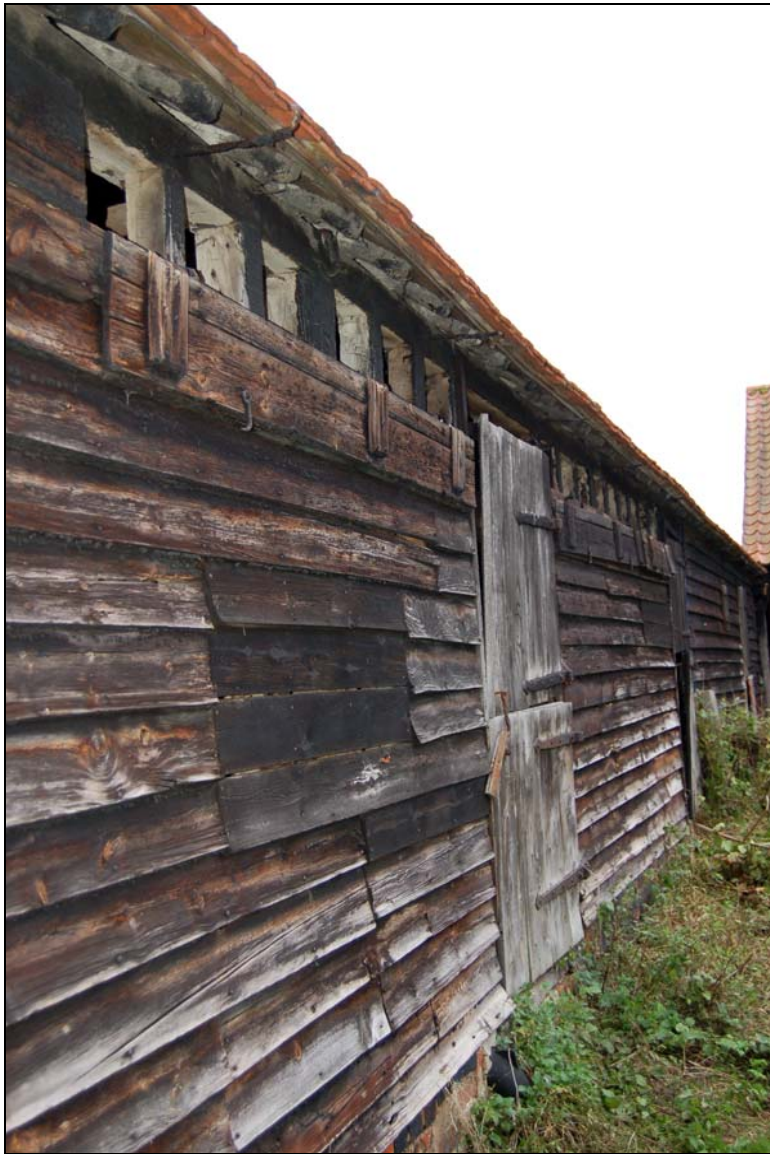
Plate 5 Detail of air vents on south elevation of stables
