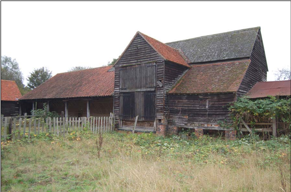
Plate 16 West elevations of cowshed and barn
