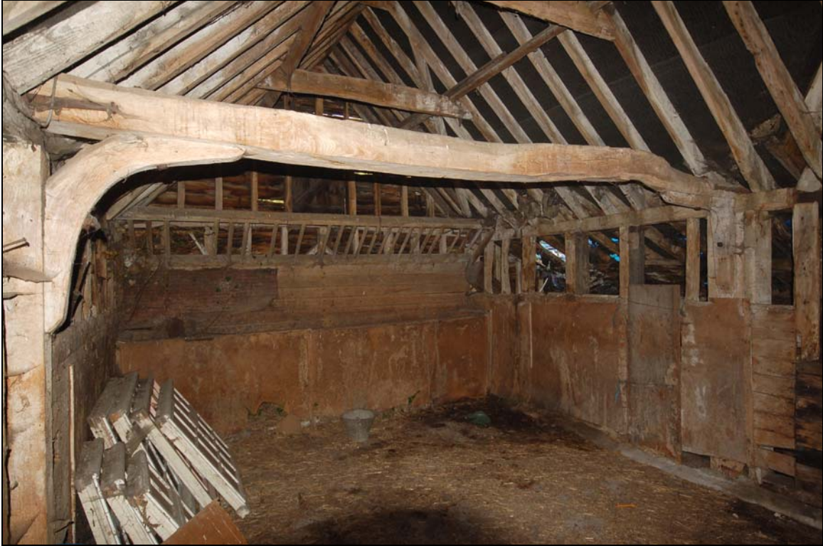
Plate 7 Interior of stall A viewed to west
