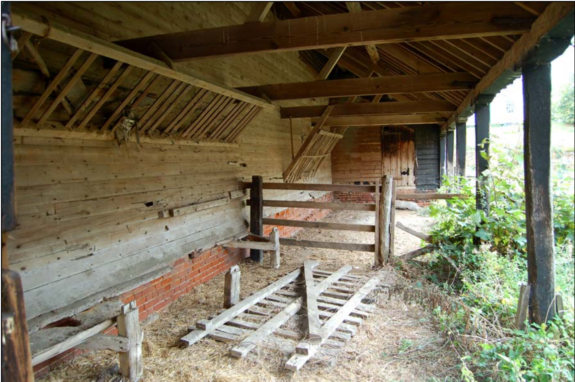
Plate 18 Interior of cowshed showing outline of former barn outshot
