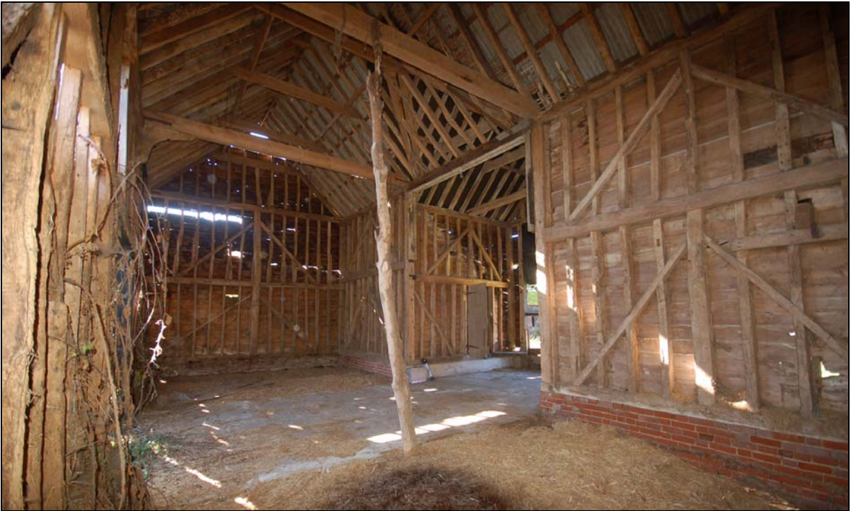
Plate 22 Interior of barn viewed to south-west
