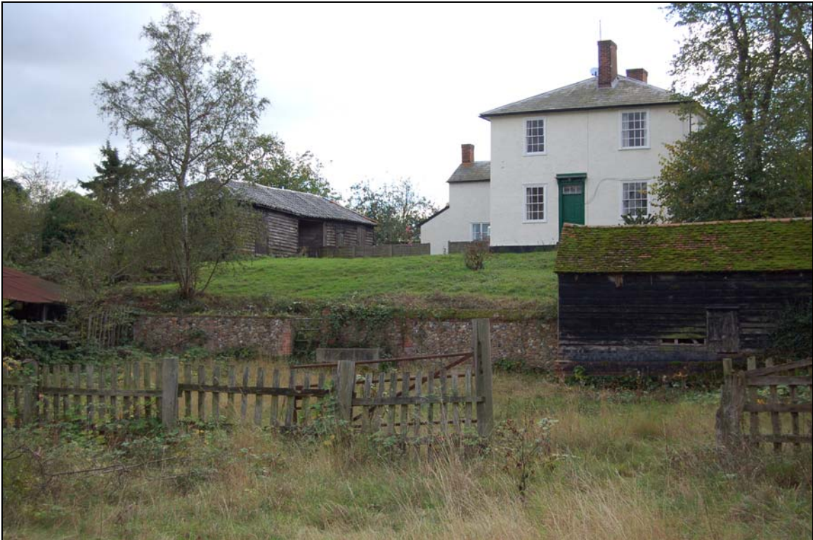
Plate 28 Farmhouse and hackney stables viewed from yard
