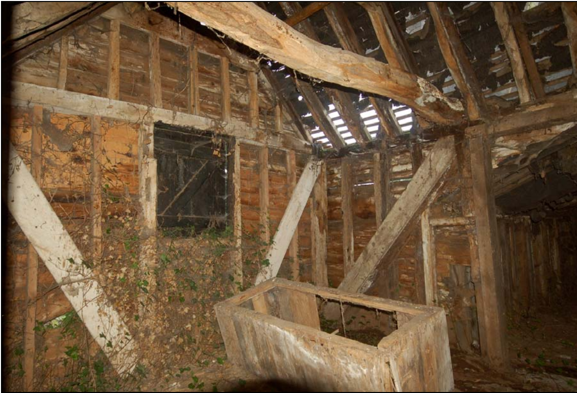
Plate 14 Interior of stable porch
