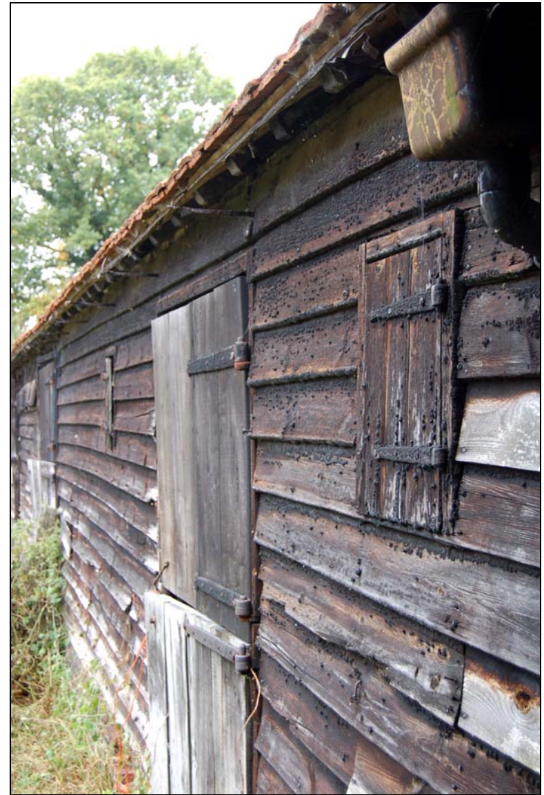
Plate 6 Detail of hatches and door fixtures on south elevation of stables
