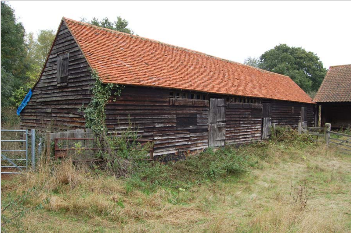
Plate 4 South and west elevations of stables
