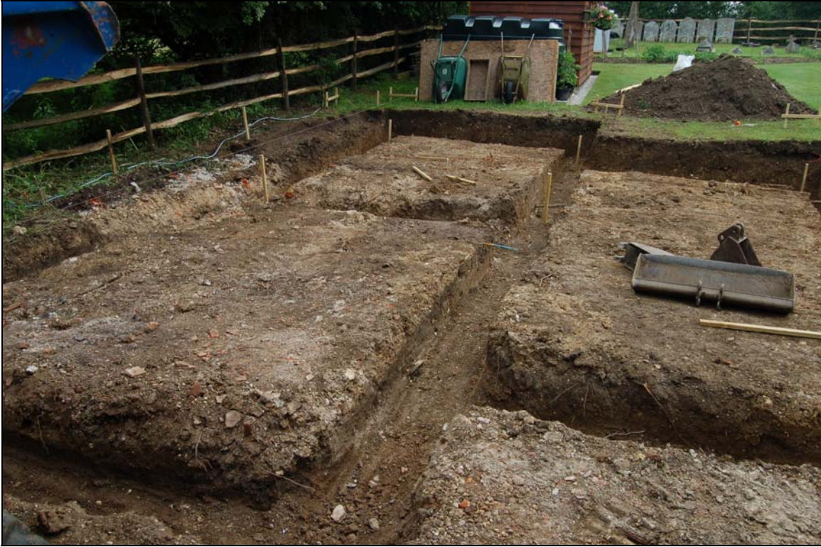
Plate 1. Footprint of the new garage
