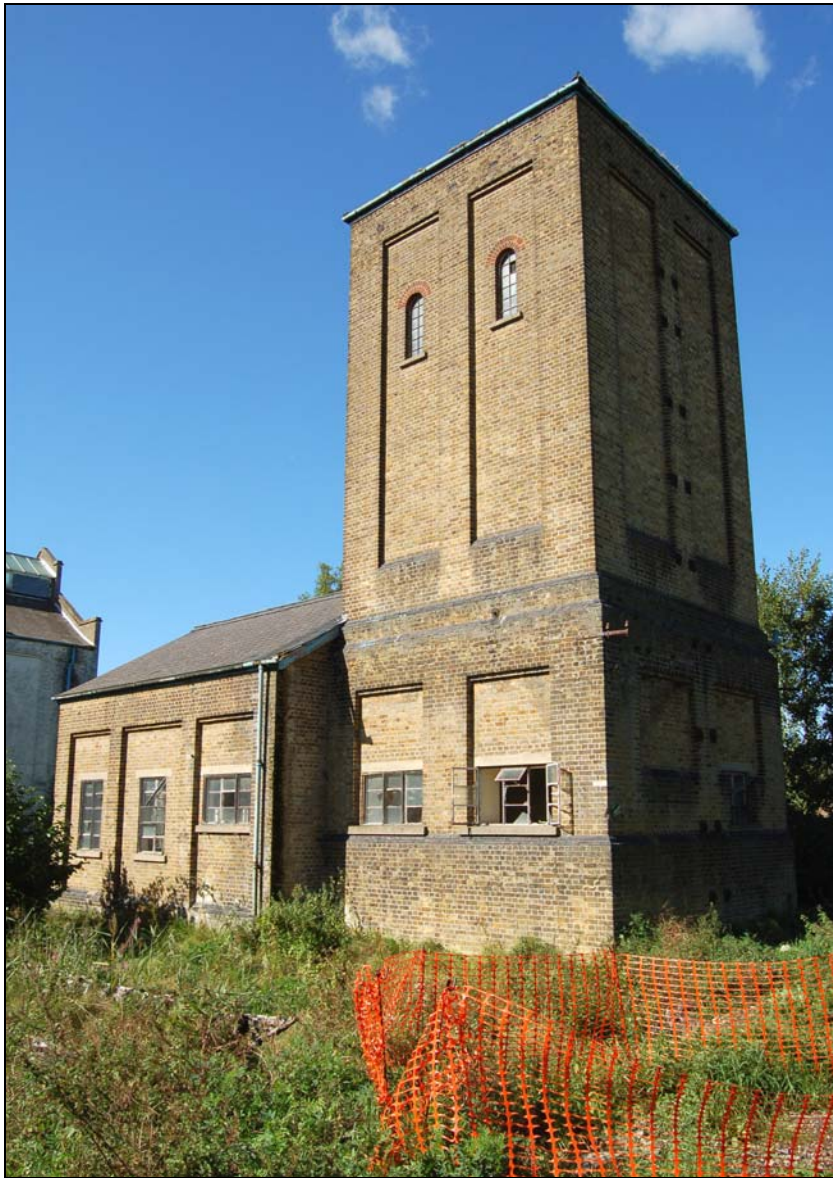
Plate 15 Accumulator viewed toward pump house (north-west)
