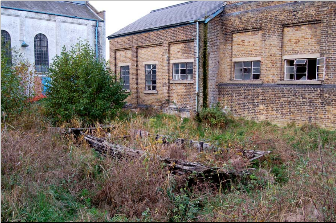
Plate 17 South-east accumulator elevation with explosives barge in foreground
