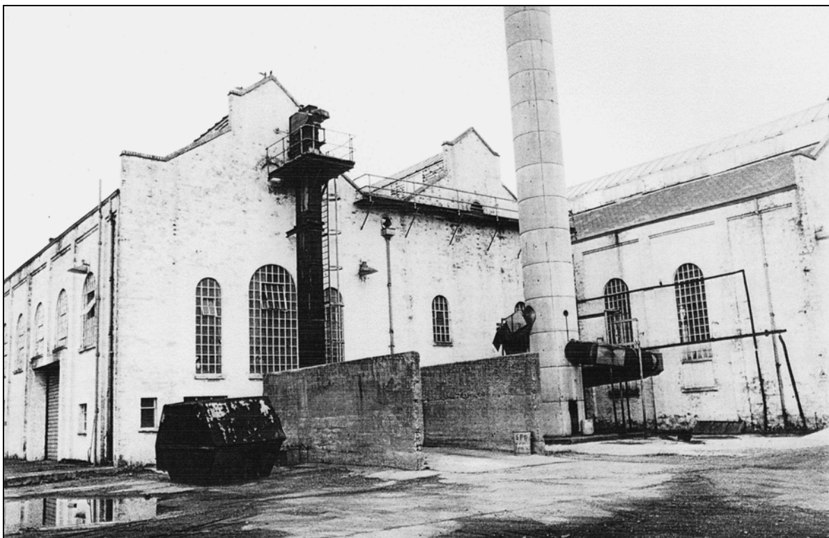
Plate 4 Power house viewed from south after closure
