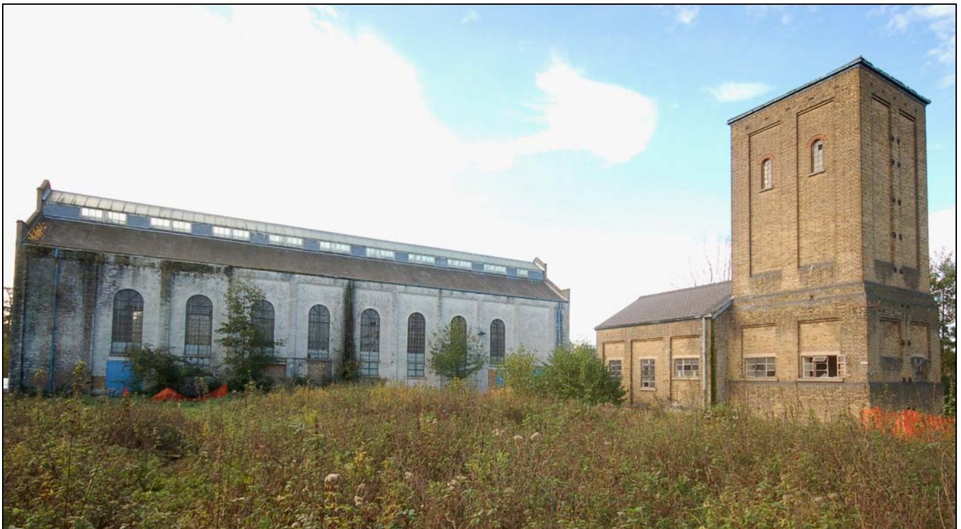
Plate 2 Power house and accumulator viewed from east
