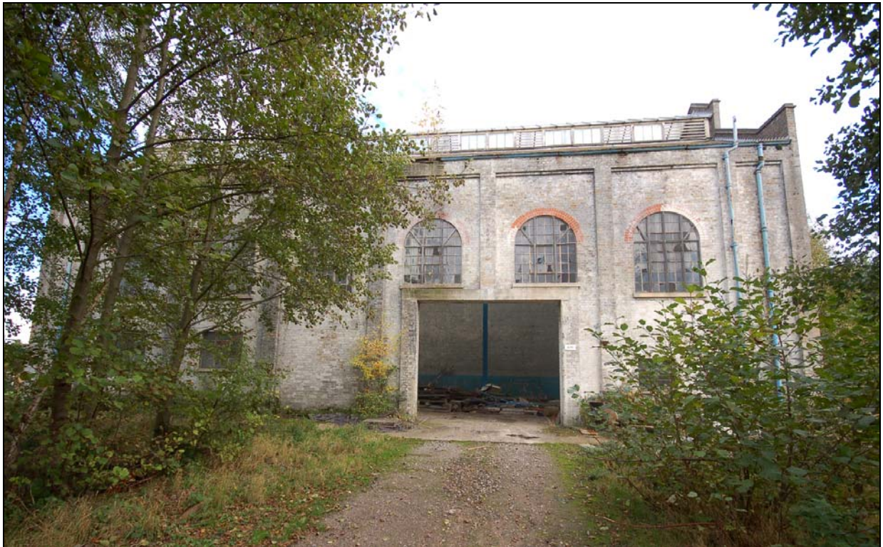
Plate 6 South-west boiler house elevation
