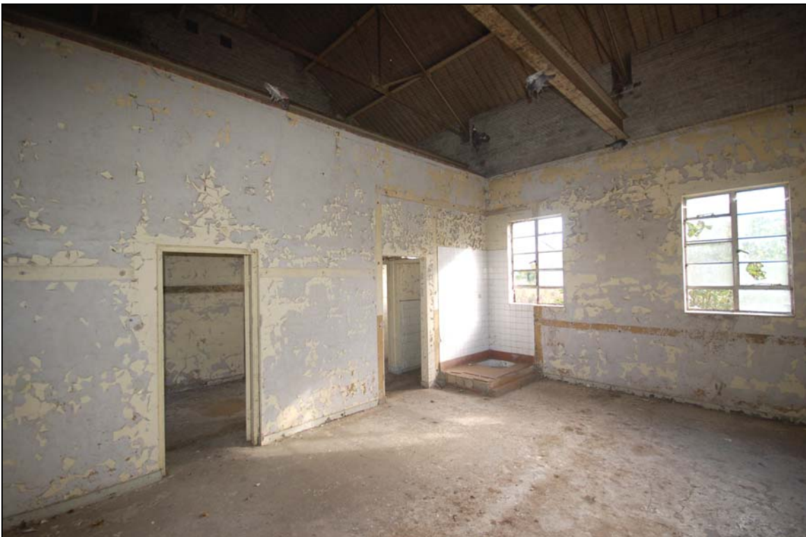
Plate 18 Interior of pump house viewed toward east
