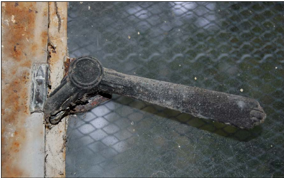
Plate 10 Detail of decorous steel window handle on south-west elevation
