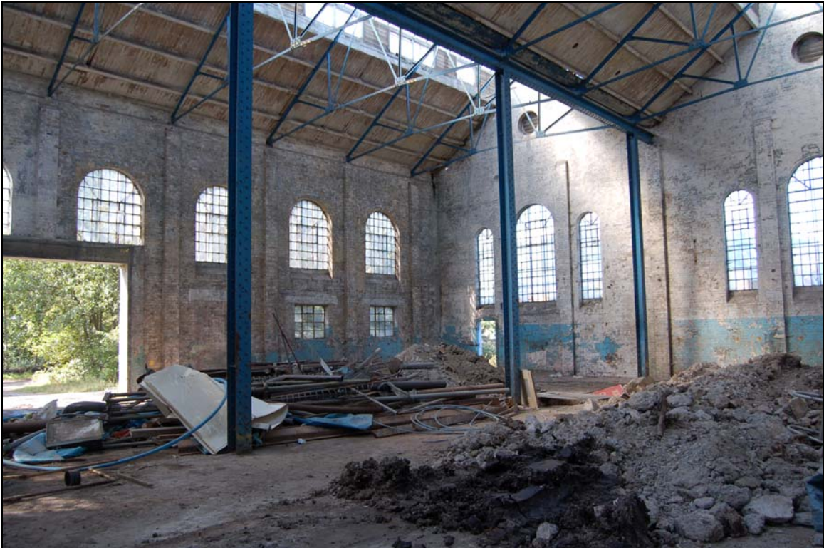
Plate 8 Interior of boiler house viewed to west
