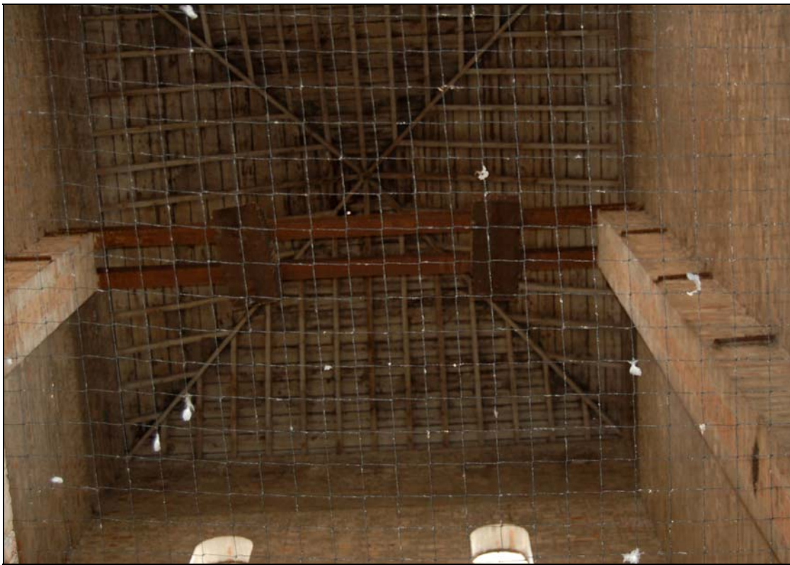
Plate 20 Weight bin buffers at top of tower
