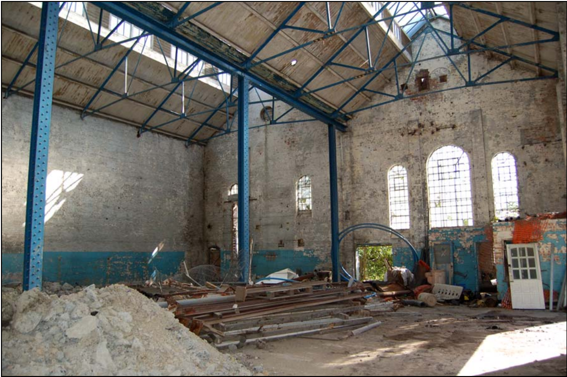
Plate 7 Interior of boiler house viewed to east
