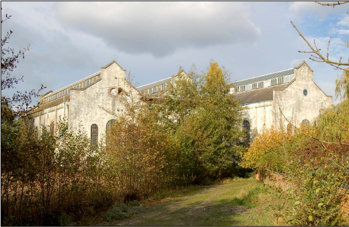
Plate 3 Power house viewed from south
