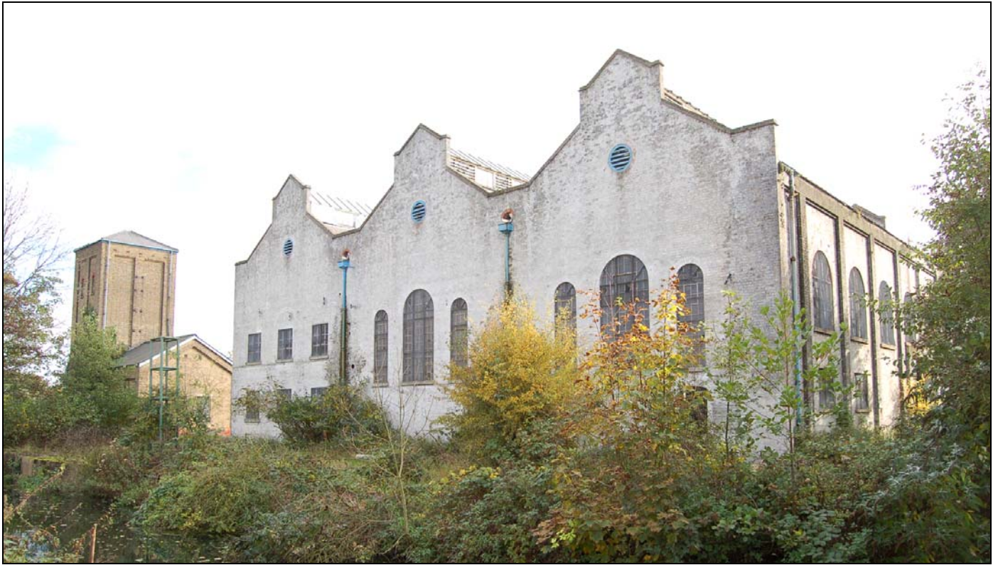
Plate 1 Power house and accumulator viewed from west
