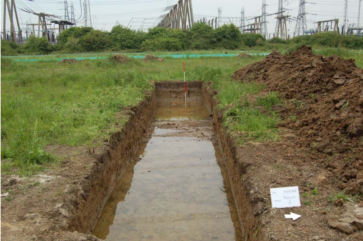
Plate 3. Trench 2, general view looking west
