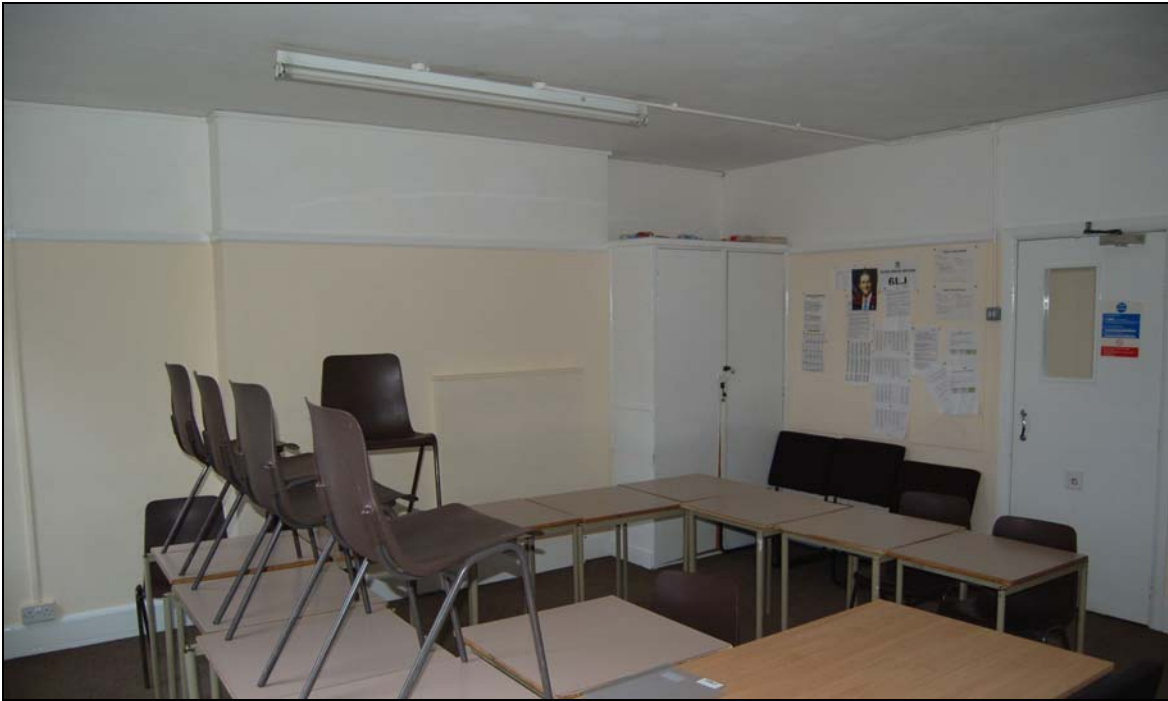
Plate 27 Typical first floor classroom inside the extension
