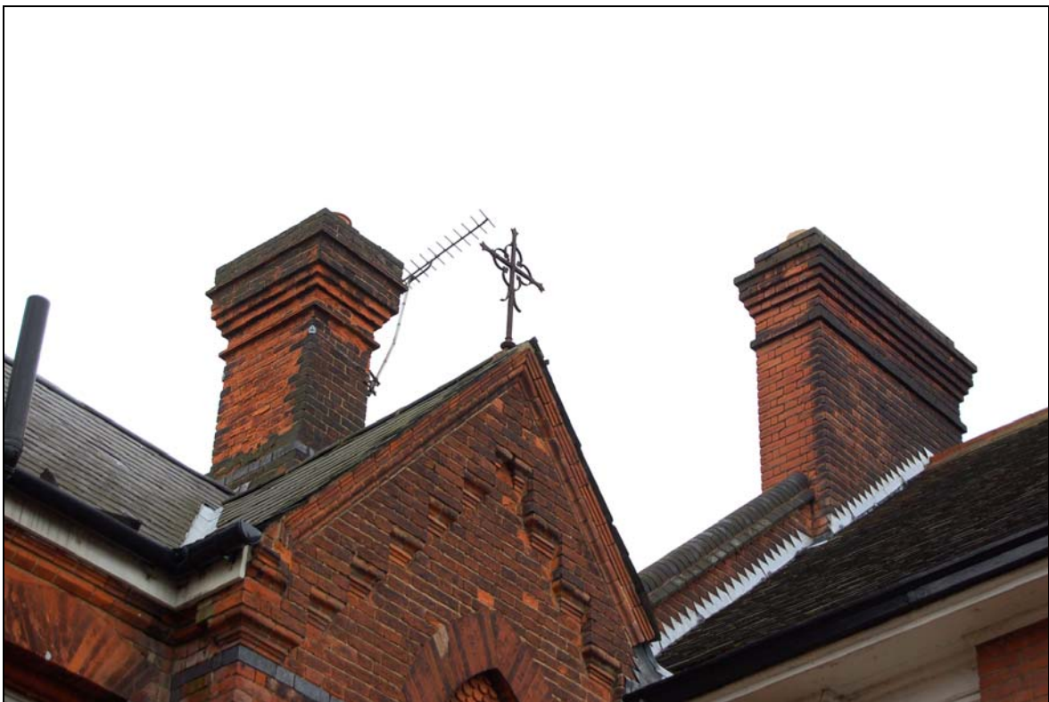
Plate 2 Iron cross over main entrance to Otway House
