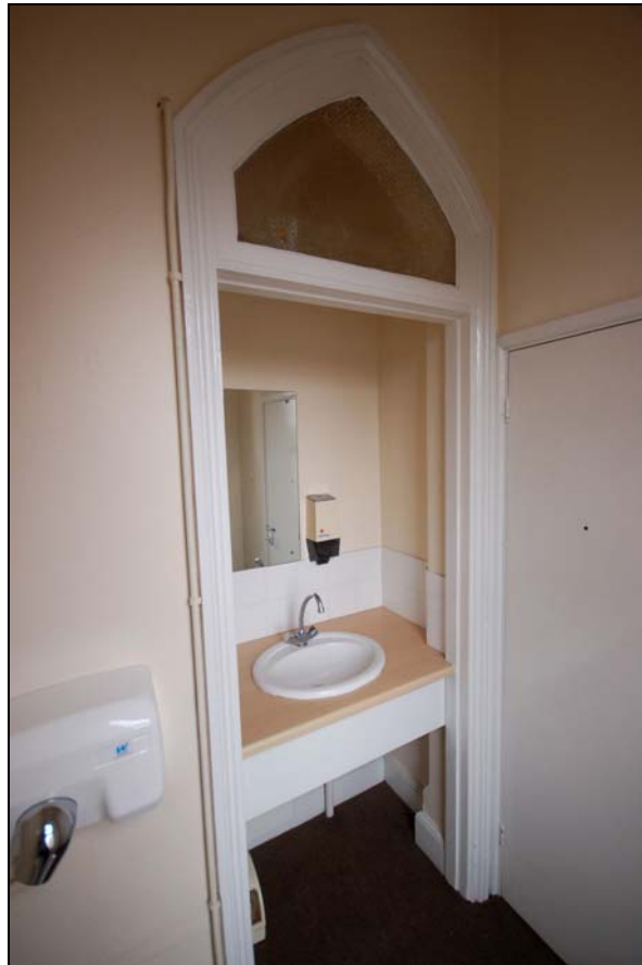
Plate 20 Wash basin in altered doorway now part of room 12
