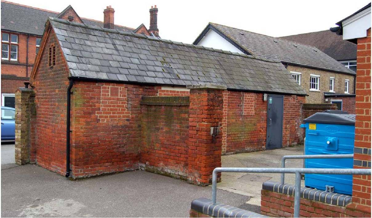
Plate 31 The armoury, former Otway House outbuilding range and yard
