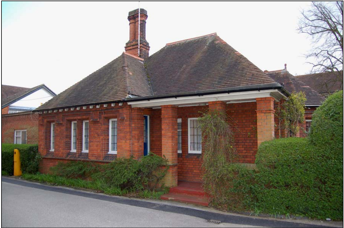
Plate 37 Marshall's Lodge viewed from west
