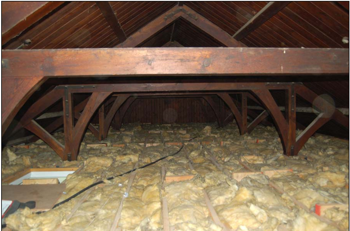
Plate 36 Roof trusses inside CCF headquarters
