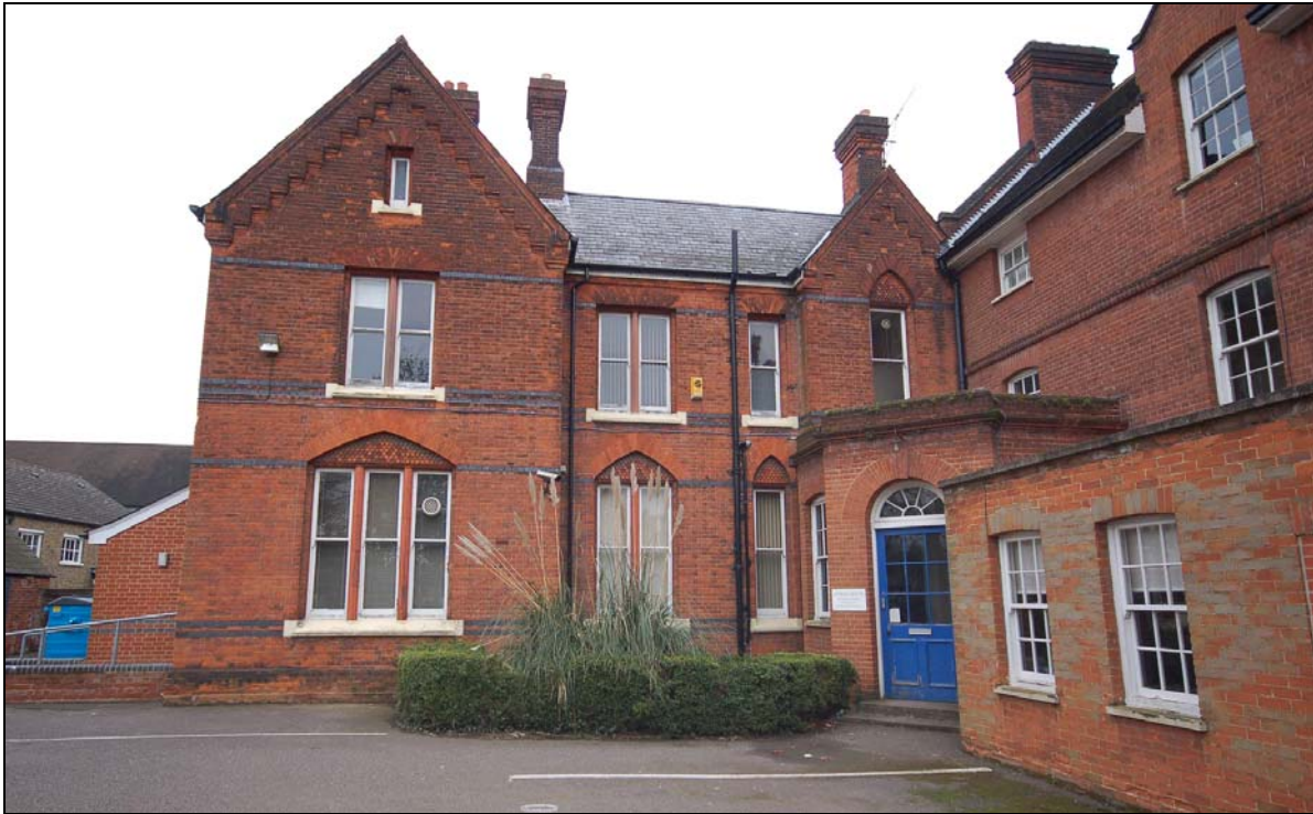
Plate 1 Former Otway House façade, with 1928 extension
