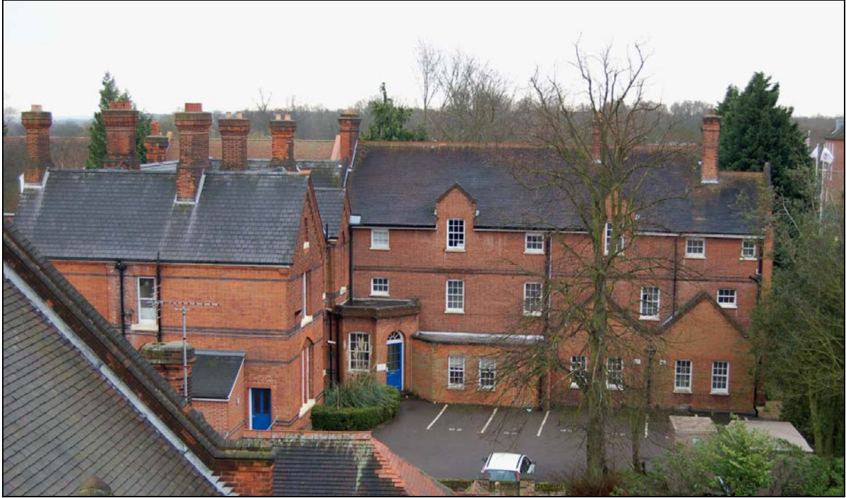
Plate 21 Otway House and extension viewed from clock tower to north-west
