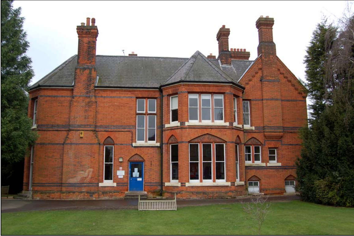
Plate 5 North-east elevation of Otway House
