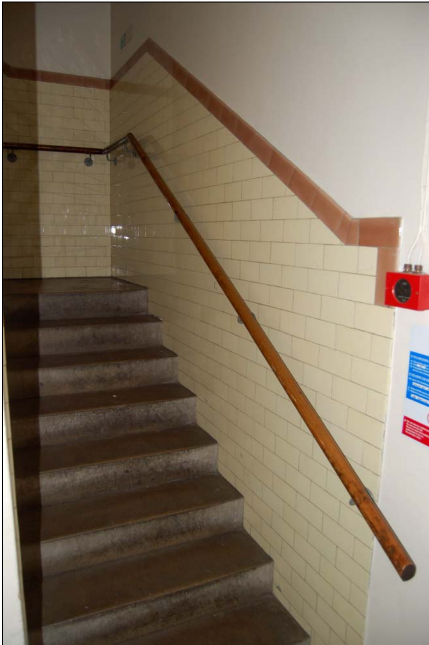
Plate 25 Stairs E9 to first floor
