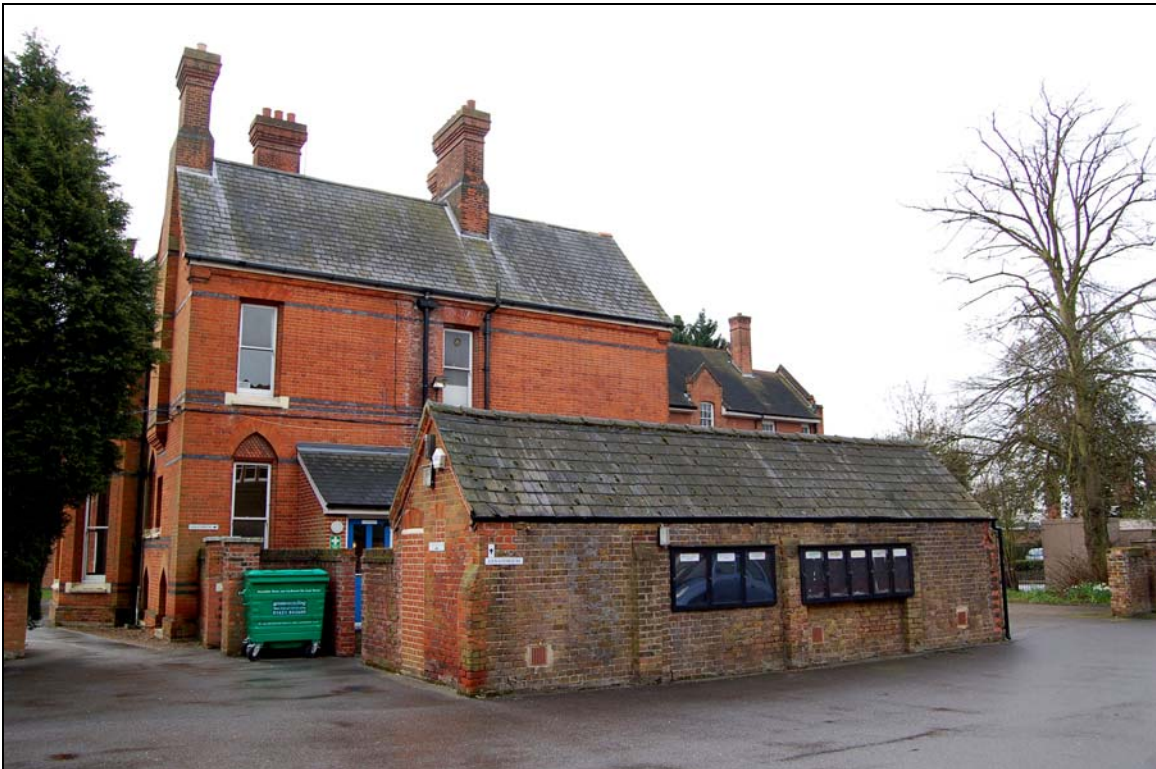
Plate 6 North-west elevation of Otway House with CCF armoury in foreground
