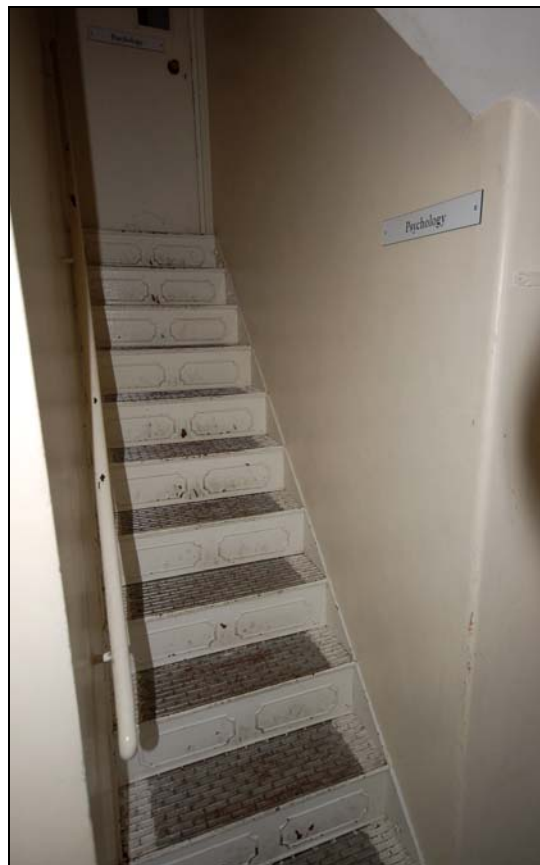
Plate 28 Iron stair to second floor
