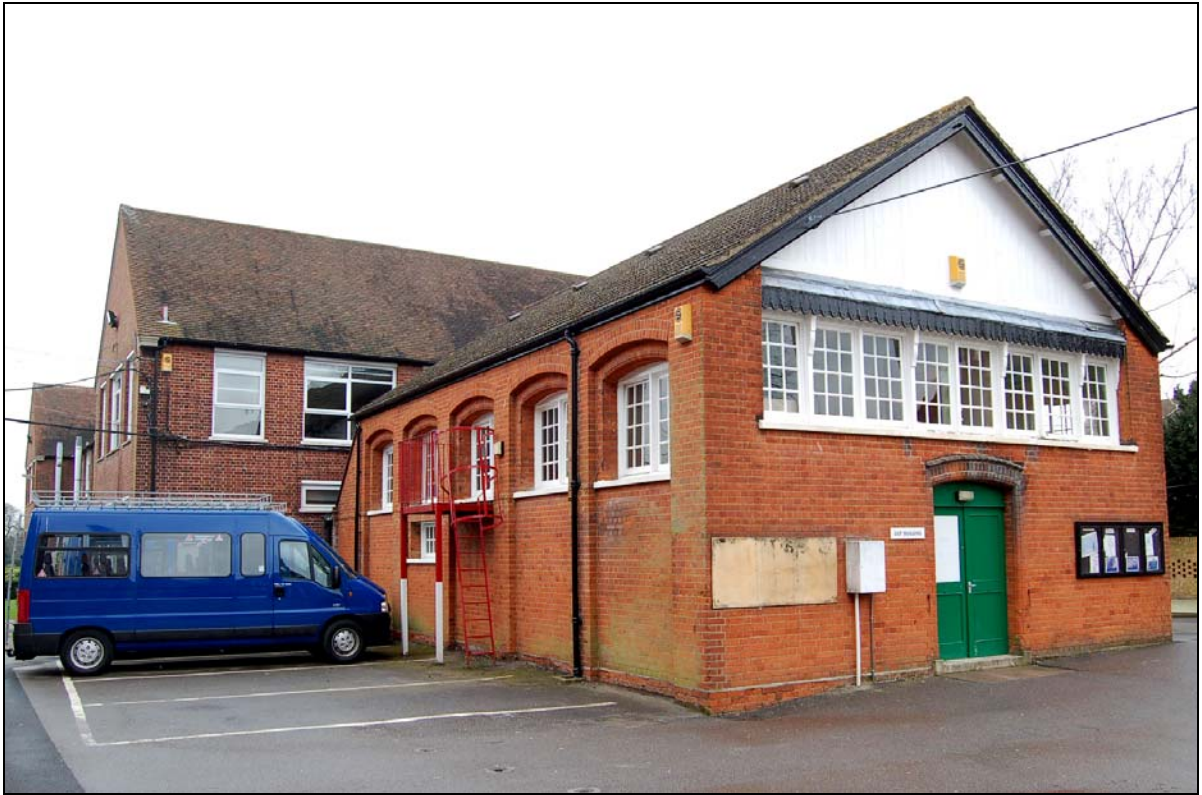
Plate 33 CCF Headquarters viewed from west
