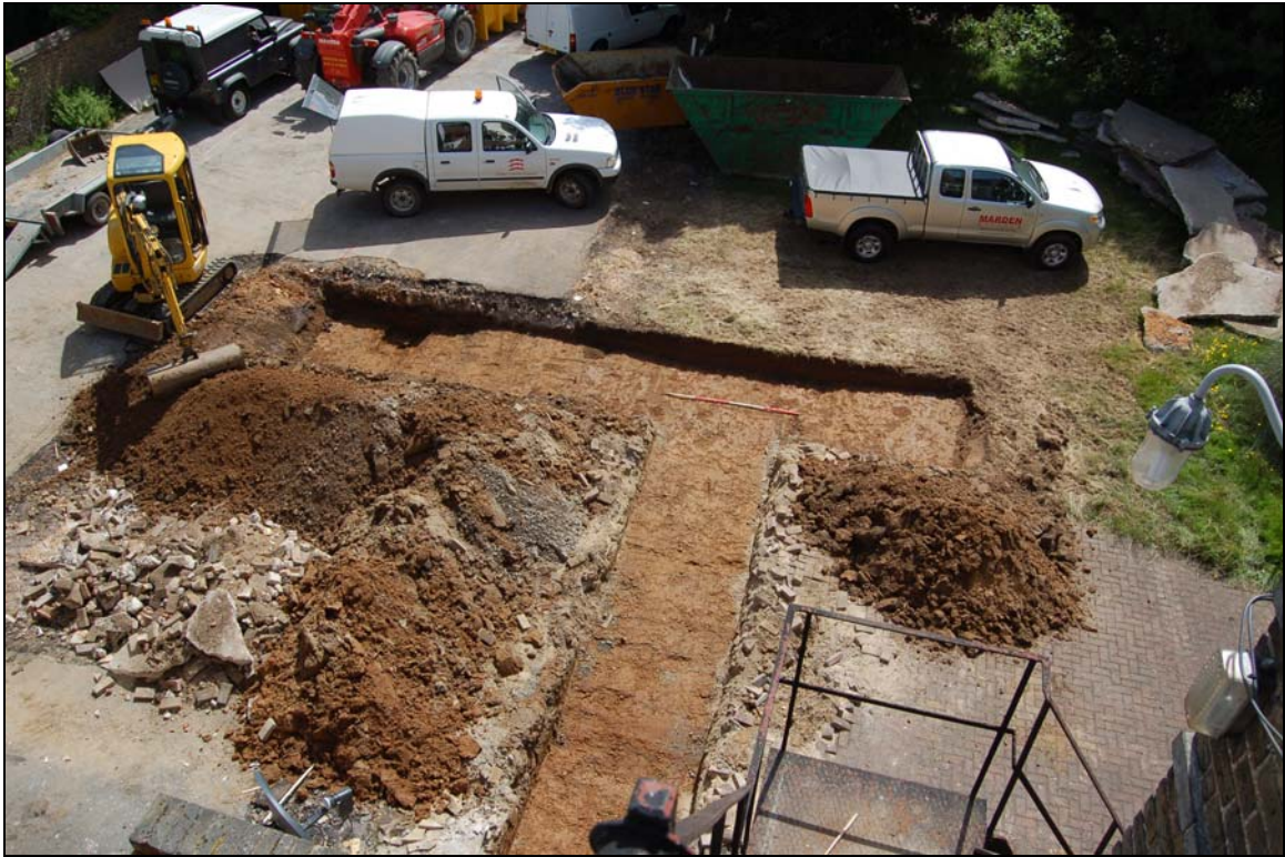
Plate 2: trenches A and B
