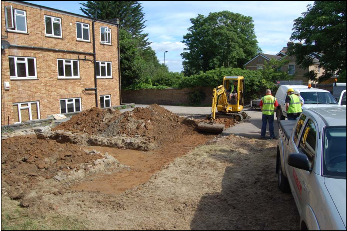
Plate 1: trenches A and B
