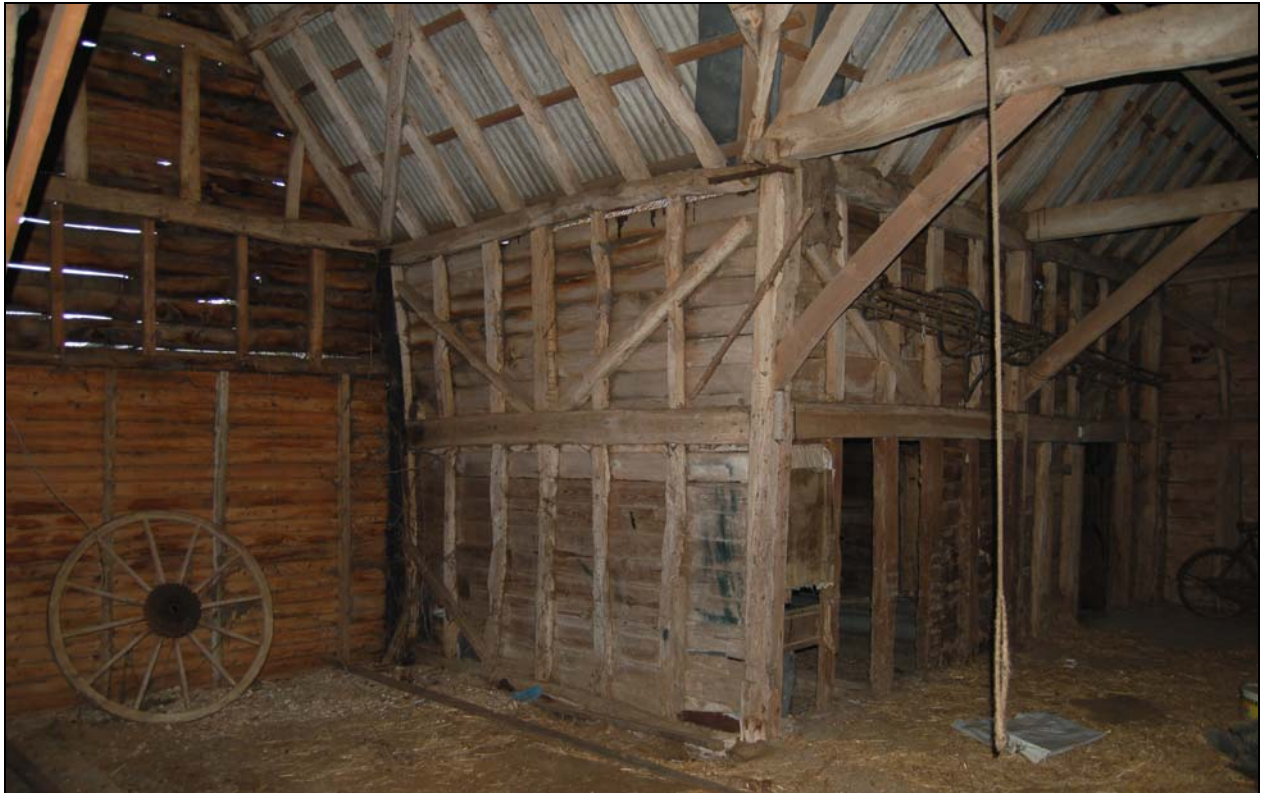
Plate 17 In-filled former cart doorway to barn 2 porch
