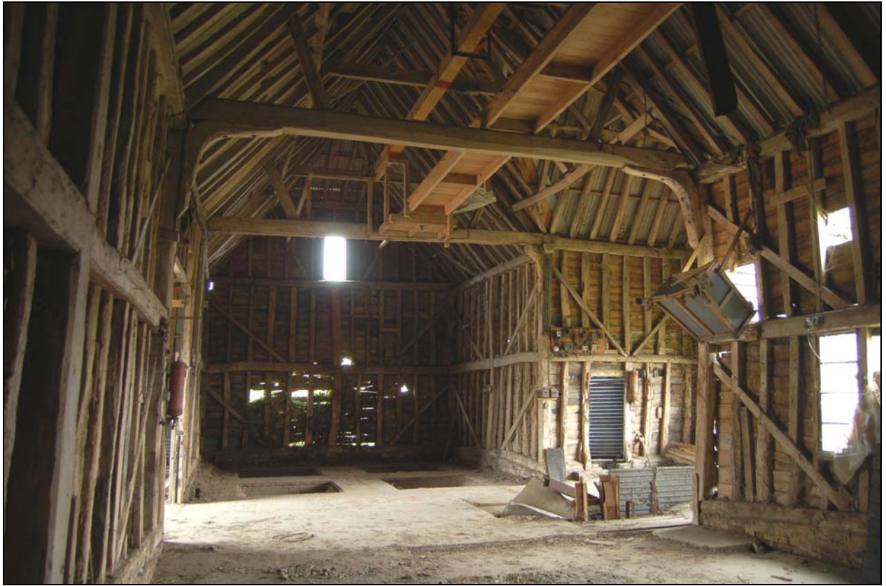
Plate 9 Interior of barn 1 viewed to west (former silos)
