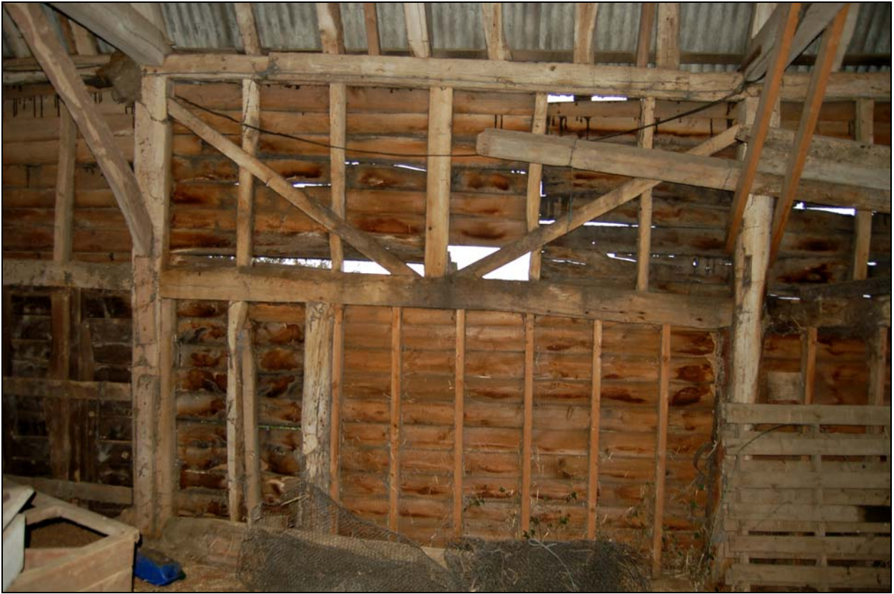
Plate 19 In-filled former door opening in barn 2
