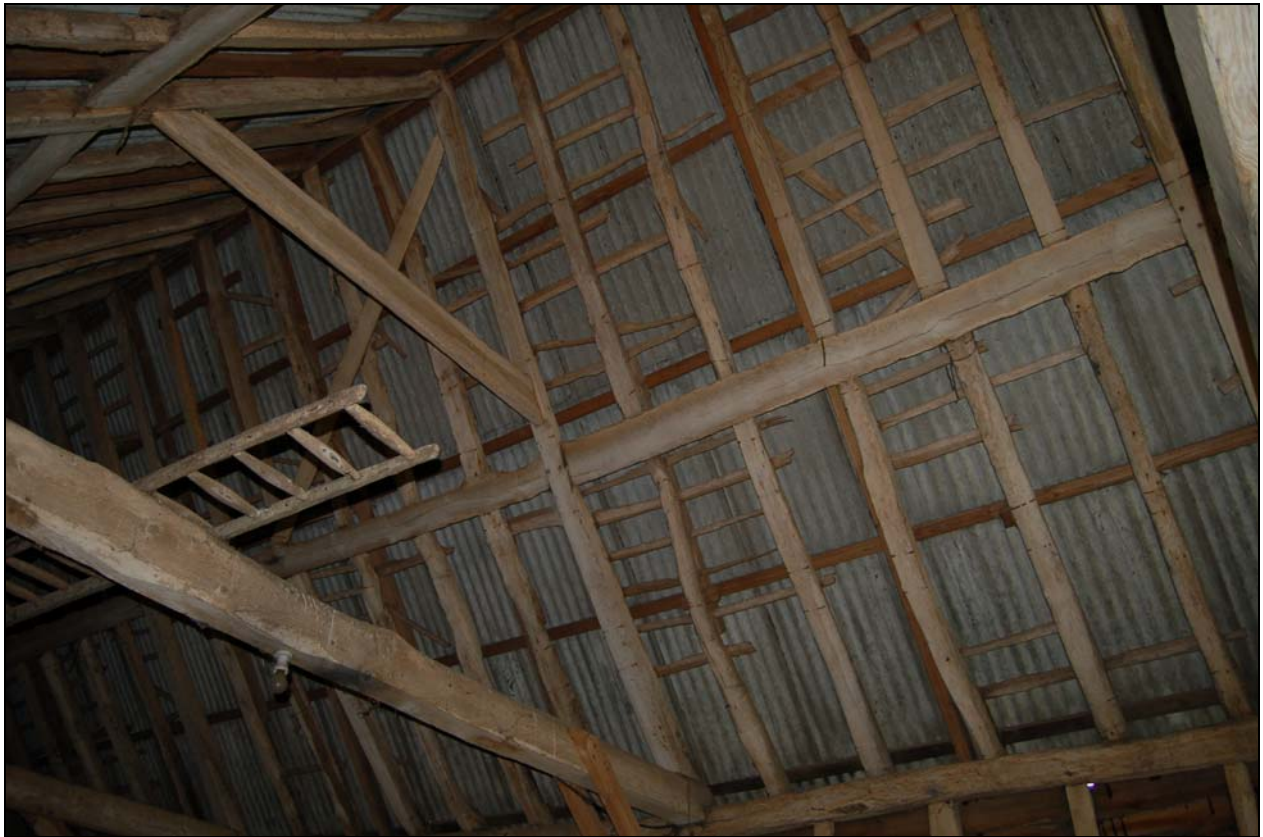
Plate 20 Detail of butt-purlin roof in barn 2
