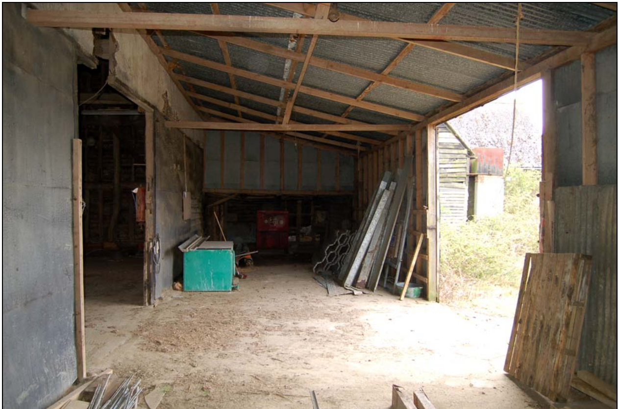
Plate 6 Enclosed south elevation of barn 1 viewed from west
