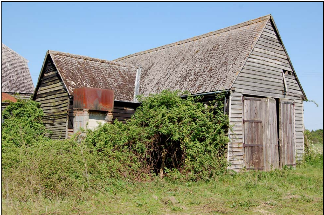
Plate 12 Barn 2 viewed from south-west
