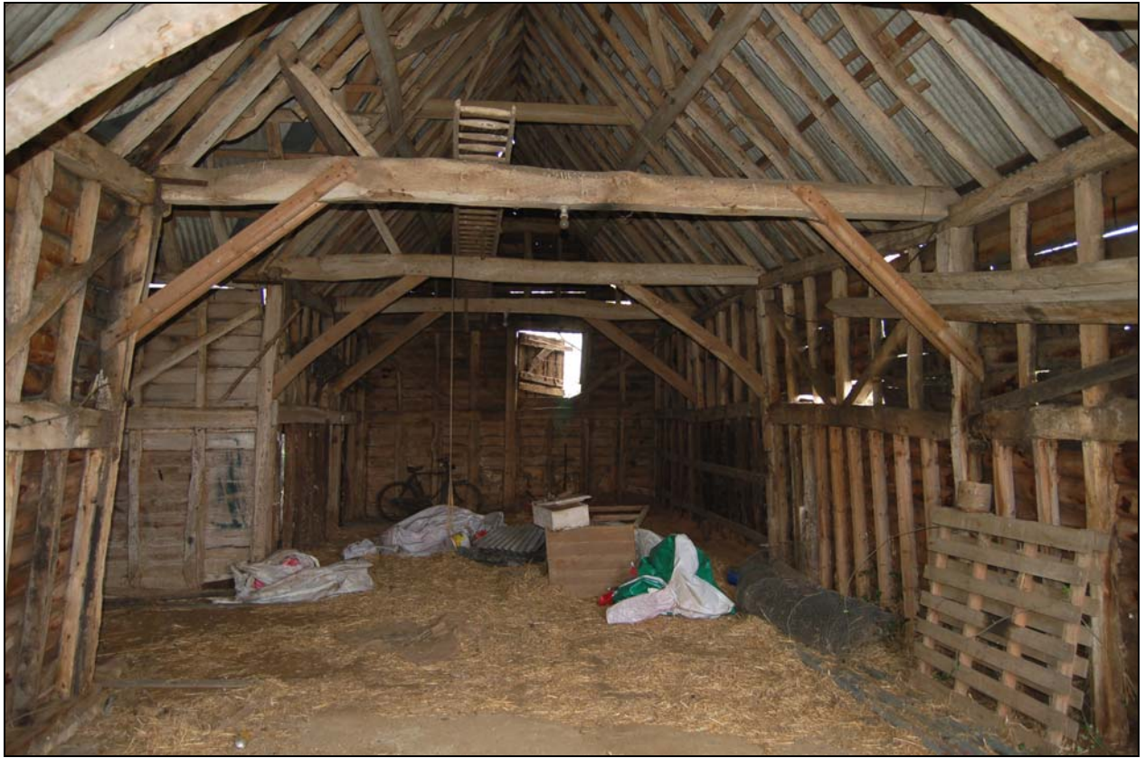
Plate 15 Interior of barn 2 viewed from south
