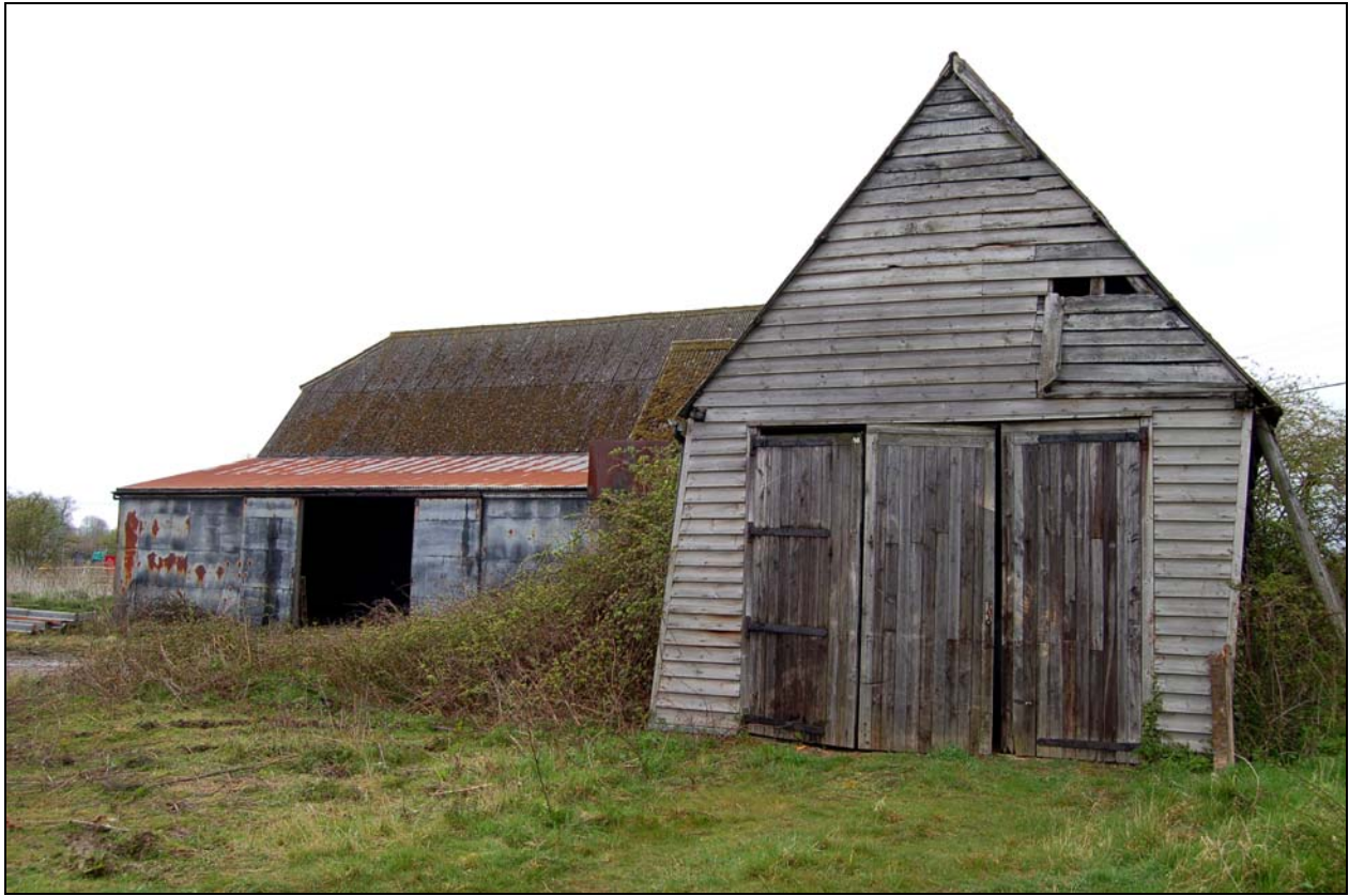
Plate 13 Rebuilt western gable of barn 2 with shed 3 in background
