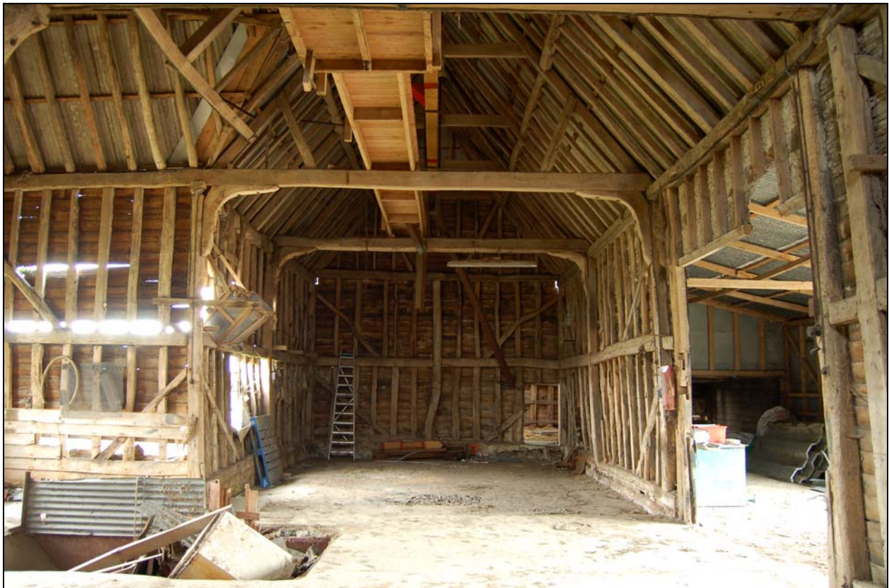
Plate 8 Interior of barn 1 viewed to east
