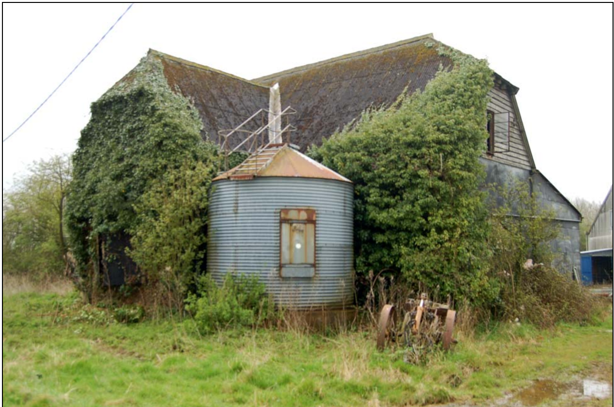
Plate 4 Barn 1 viewed from north-west
