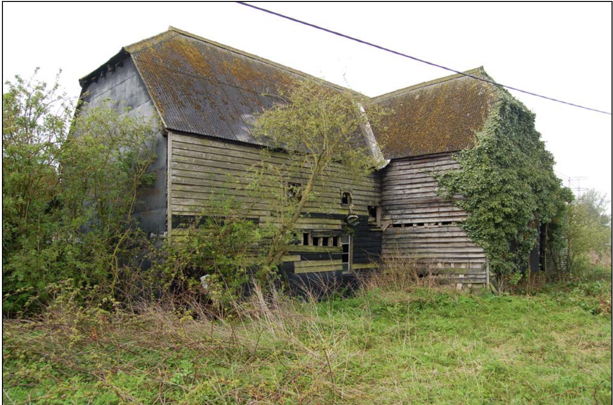
Plate 5 Barn 1 viewed from north-east
