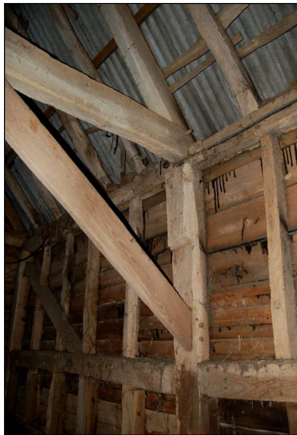
Plate 18 Detail of typical gunstock jowl and bracing in barn 2
