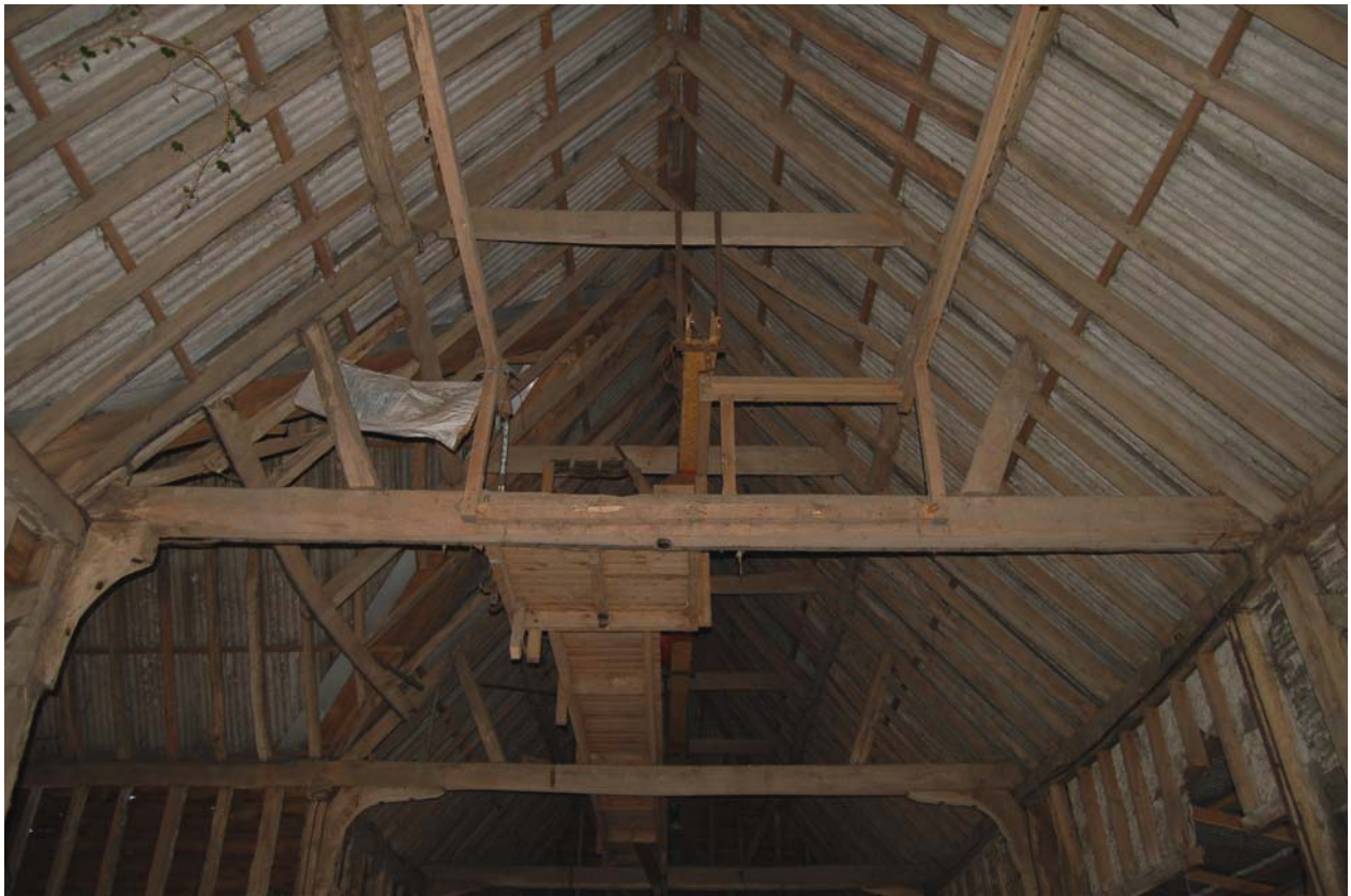
Plate 11 Butt-purlin roof detail and grain conveyer inside barn 1
