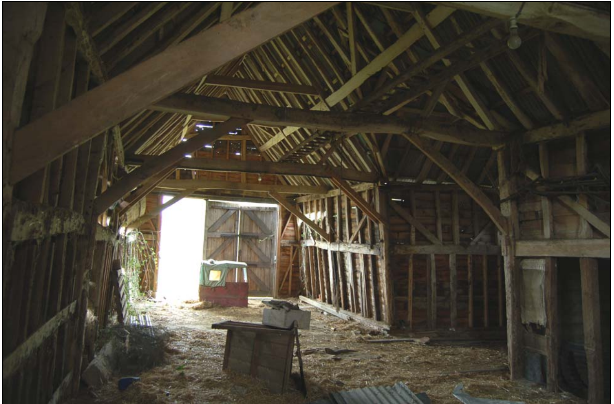
Plate 16 Interior of barn 2 viewed from north
