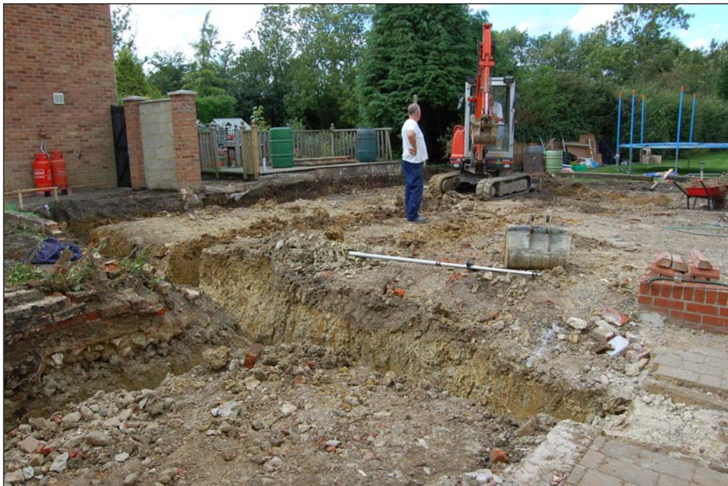
Plate 2 : General view of site after cutting foundation trenches, looking north-west.
