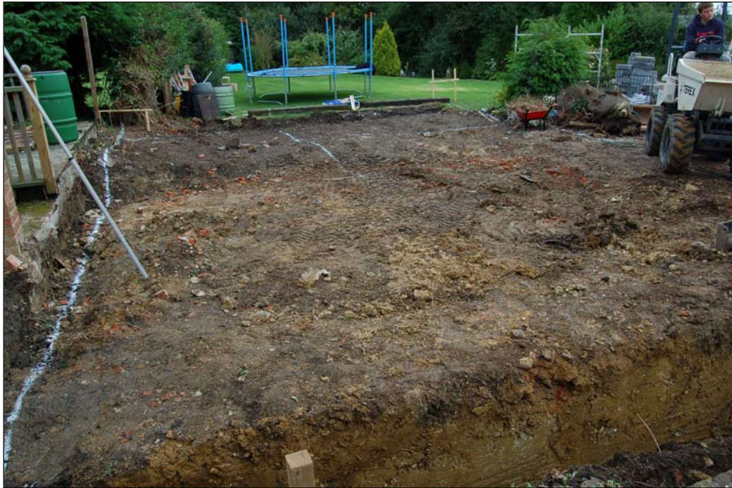
Plate 1 : General view of site after demolition of outbuildings, looking north.
