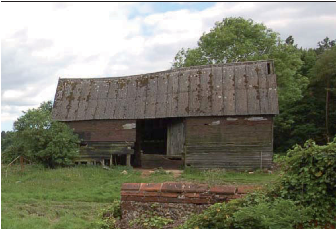
Plate 12 North elevation of barn 3
