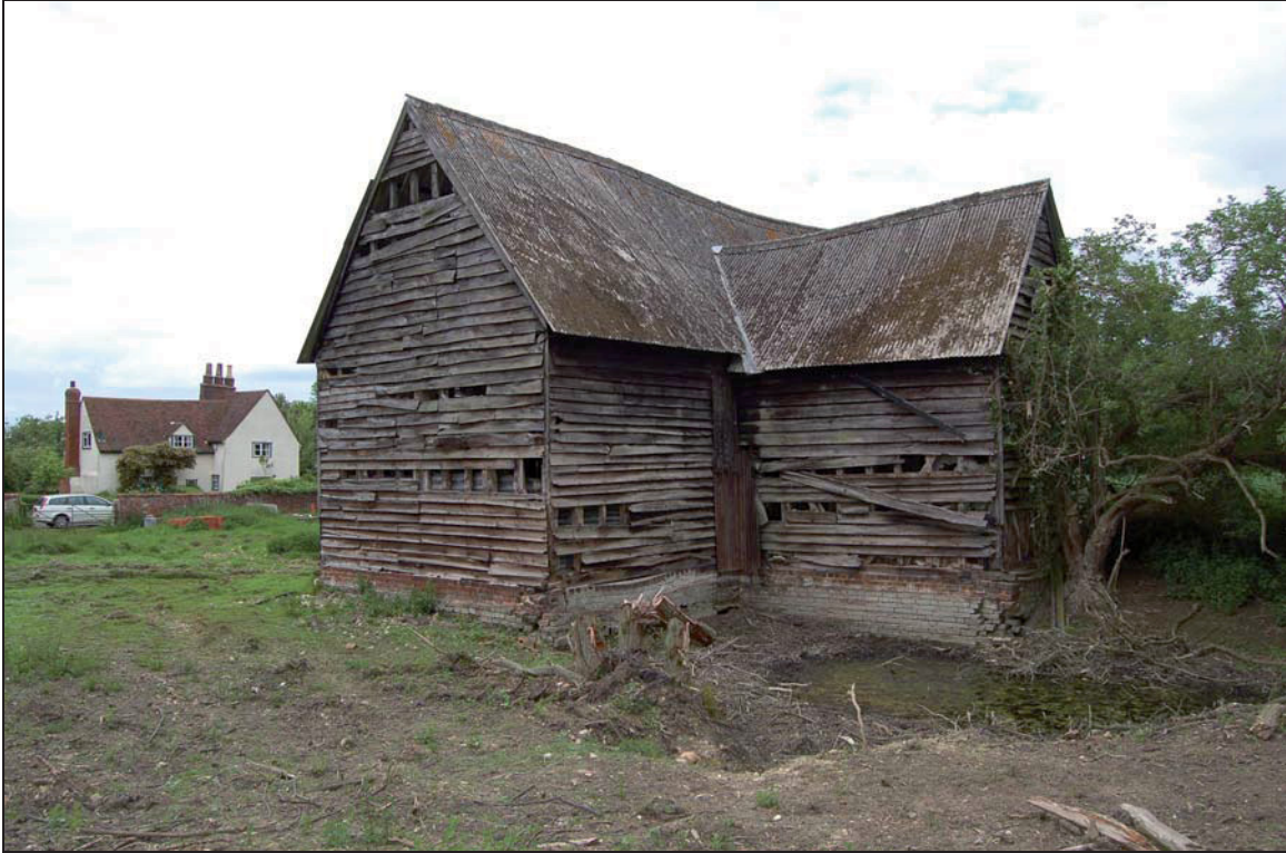
Plate 15 Barn 3 viewed from south-west with farmhouse in background
