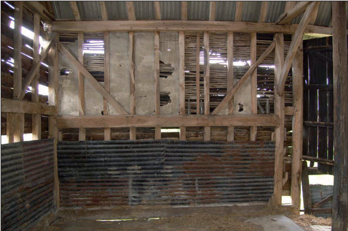
Plate 18 Lime-plastered wall-framing to west end of barn 3
