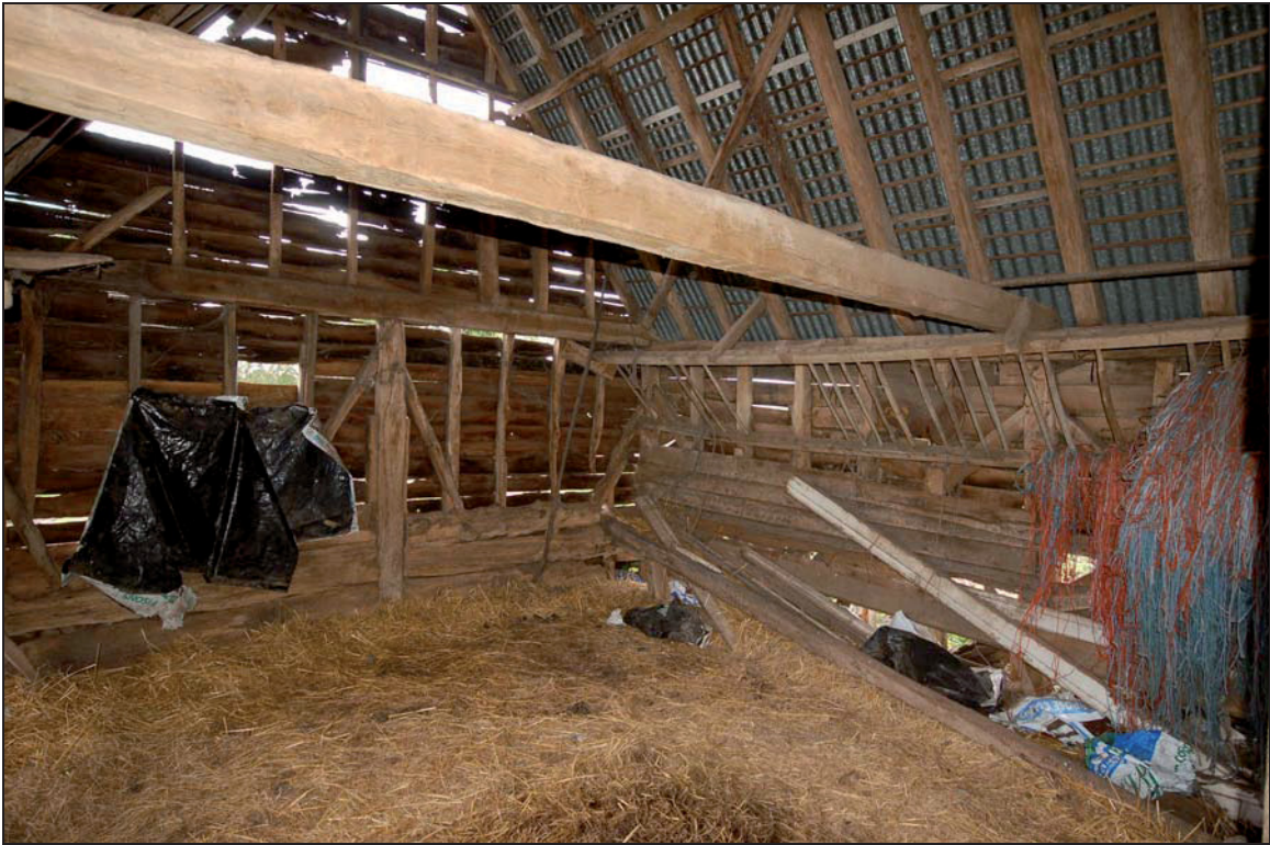
Plate 23 Interior of stables viewed to south-west
