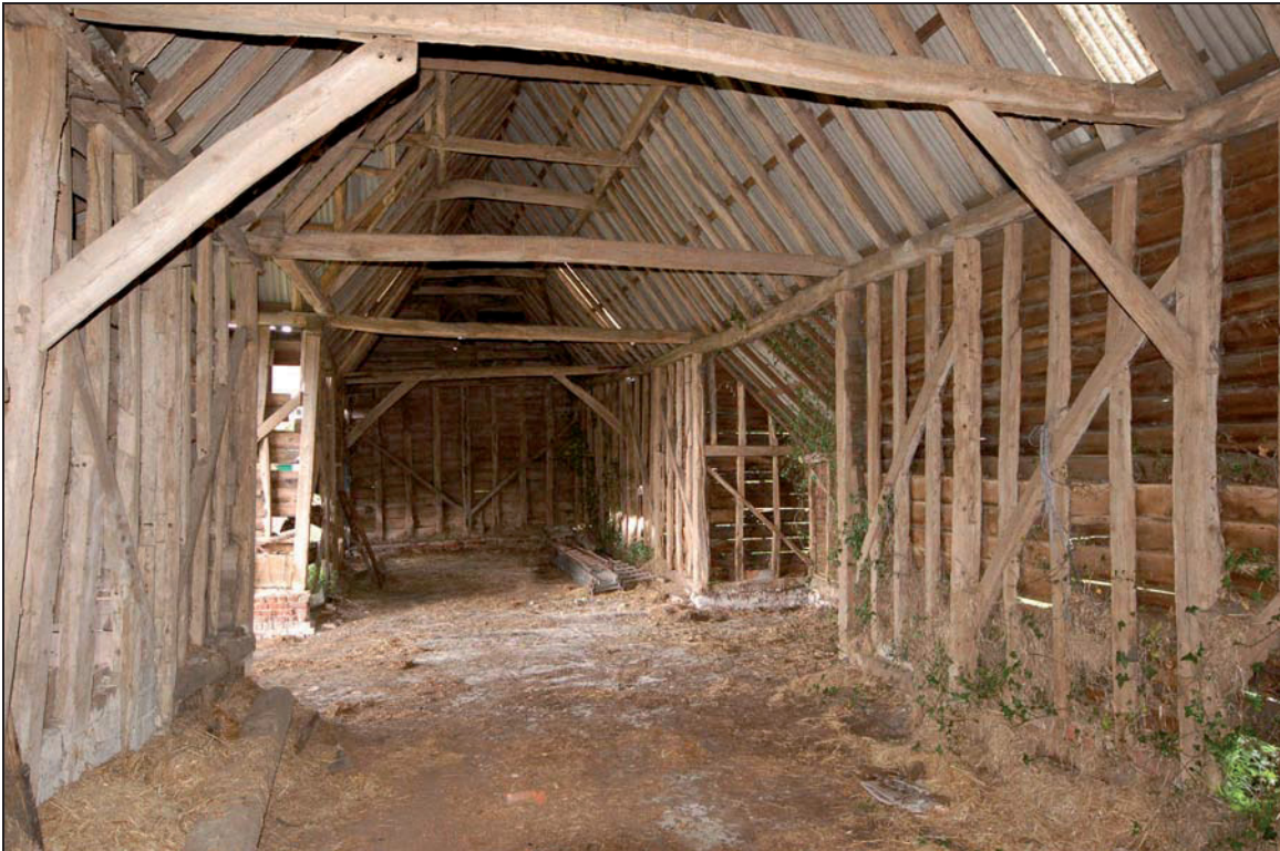
Plate 8 Interior of barn 2 viewed to north
