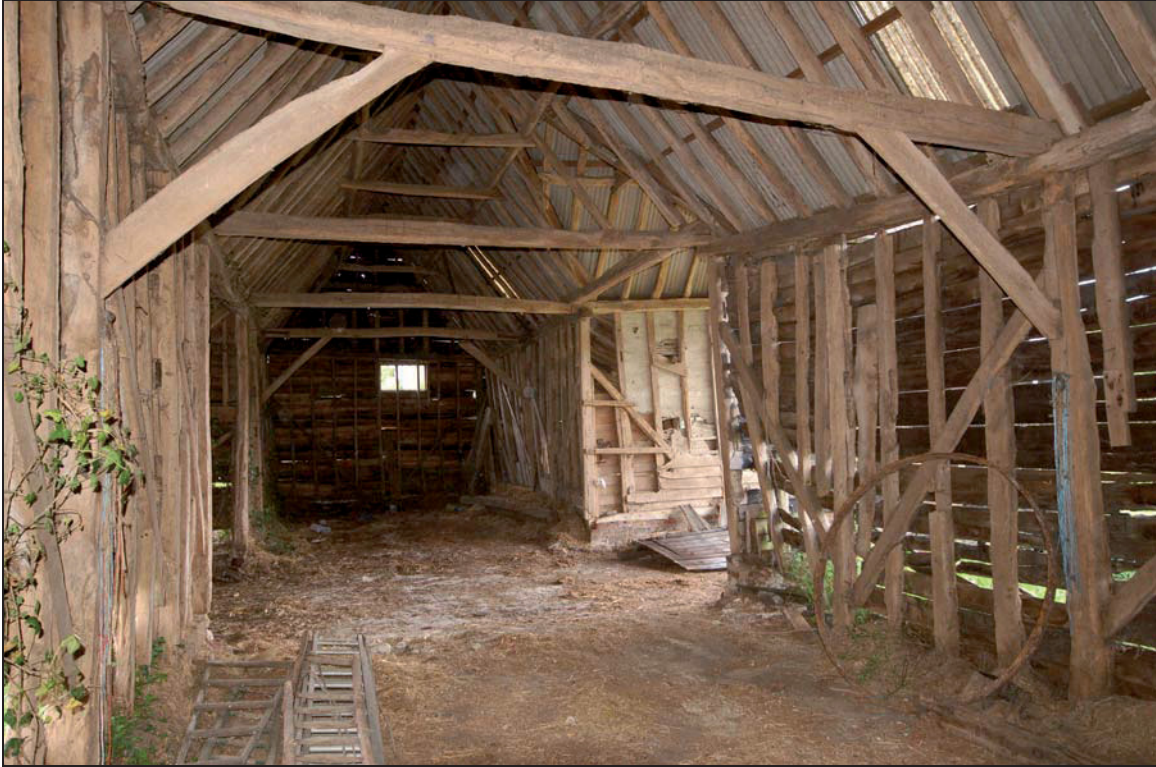
Plate 9 Interior of barn 2 viewed to rebuilt gable to south
