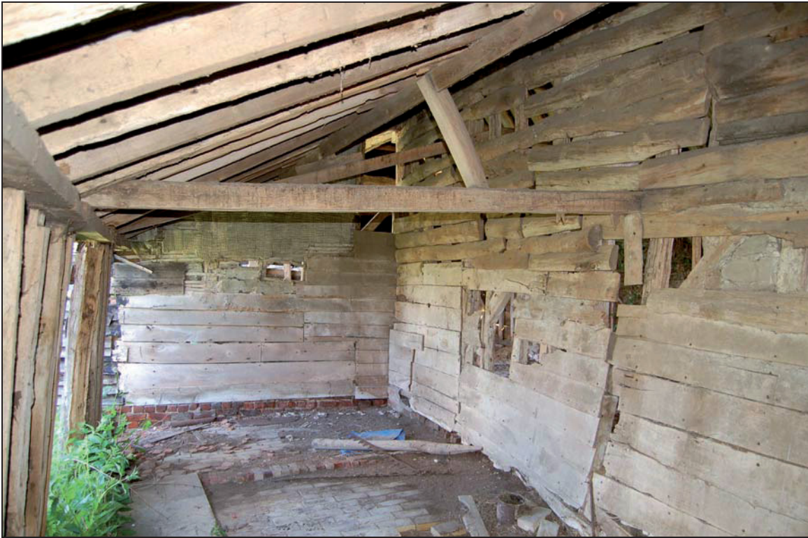
Plate 7 Enclosed walls of barn 2 from inside stalls 2a
