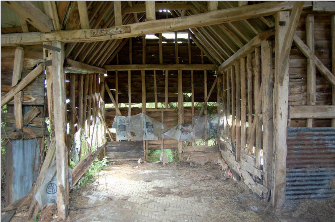
Plate 20 Porch and threshing floor in barn 3
