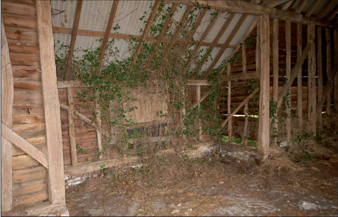
Plate 11 Short porch to rear of barn 2
