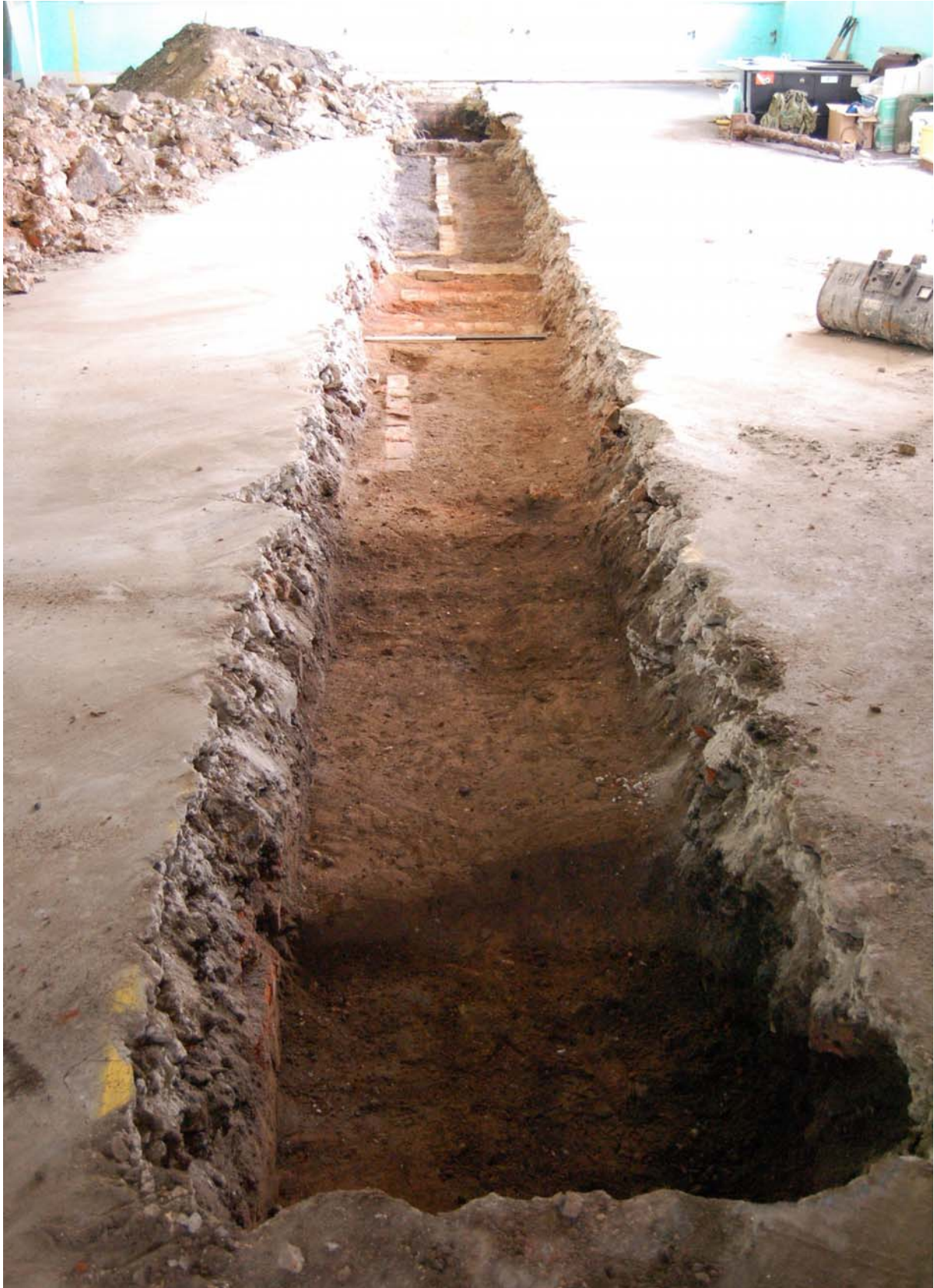
Plate 1 : Trench 2 after cleaning, looking northwest (Scale 1m)
