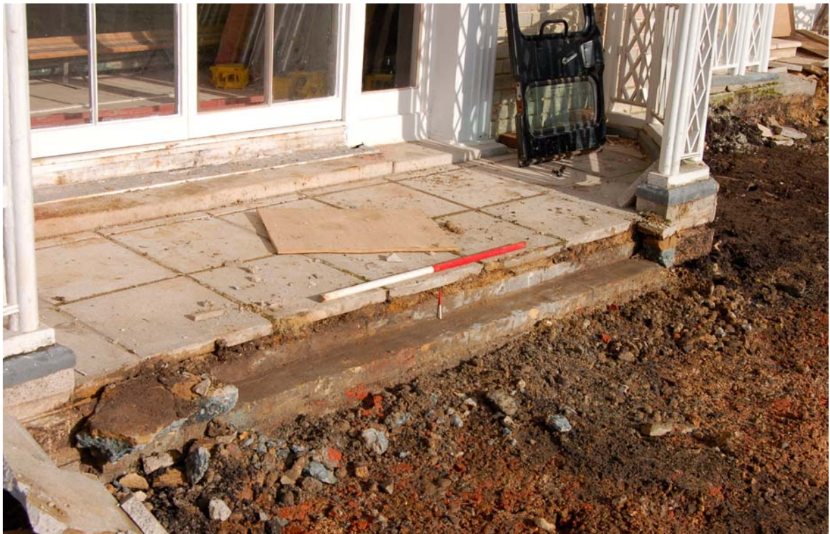
Plate 6. Brick step in front of west window looking north (0.10m & 1m scales)
