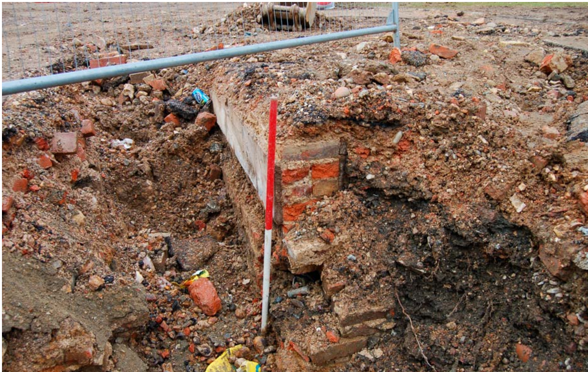
Plate 4. Wall 36 looking west (1m scale)
