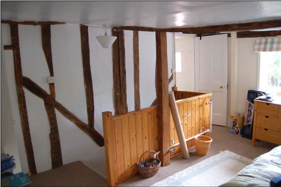
Plate 13 Primary-braced framing inside playroom on first floor
