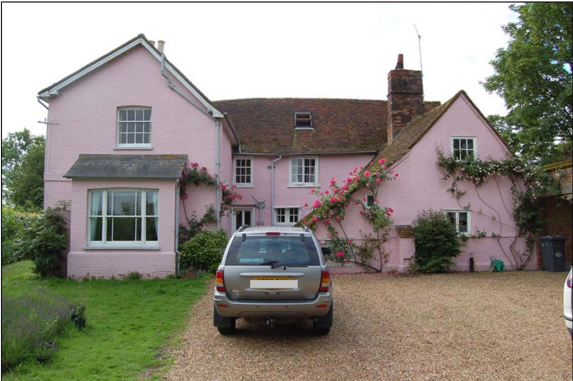
Plate 2 Driveway elevation (north-west)
