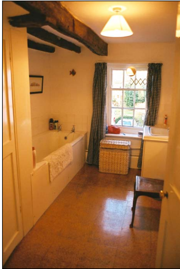
Plate 9 Remains of partition on first floor bathroom (reused timber)
