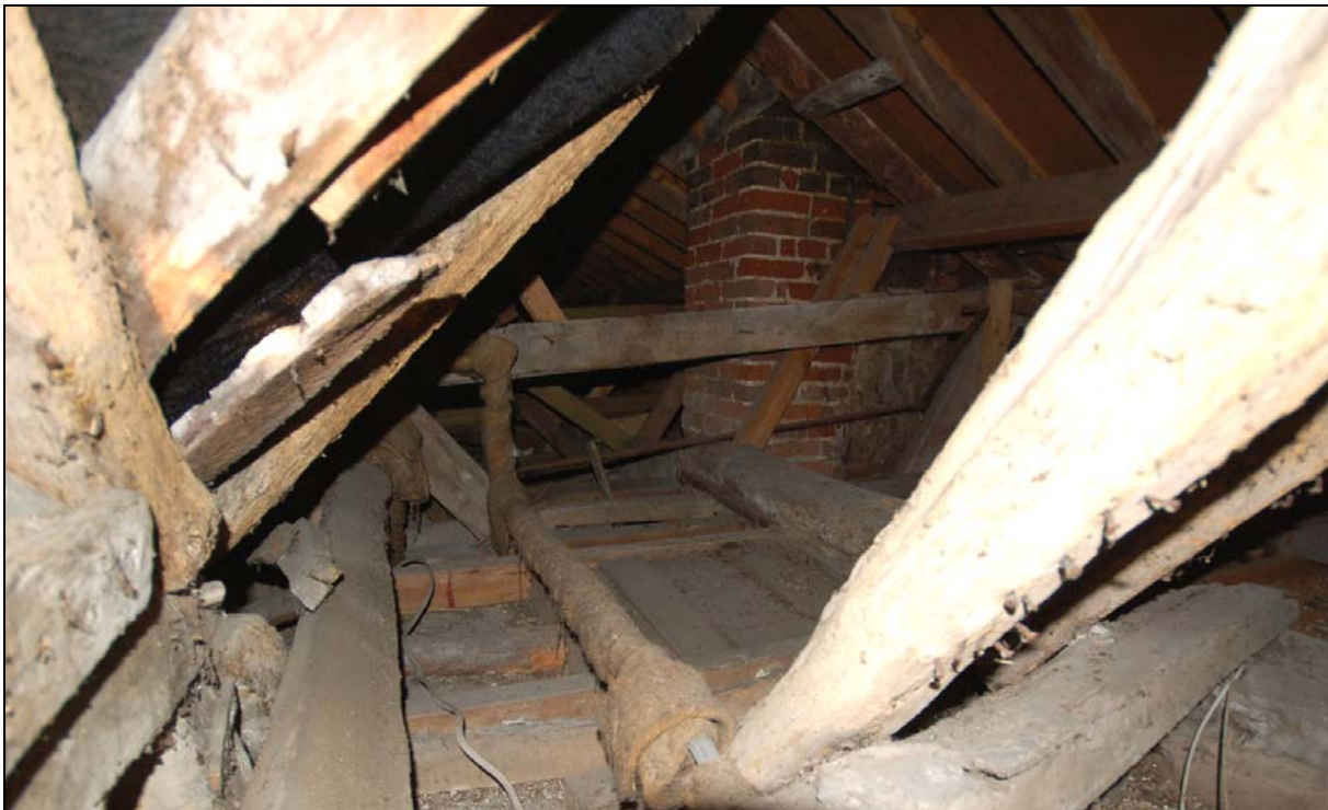
Plate 24 Rebuilt roof over cross wing
