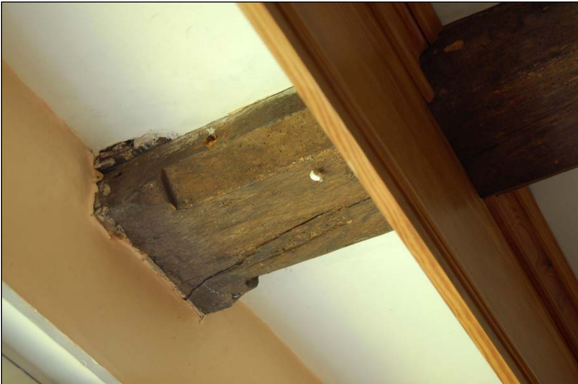
Plate 16 Lamb's tongue stop to stair hall bridging joist
