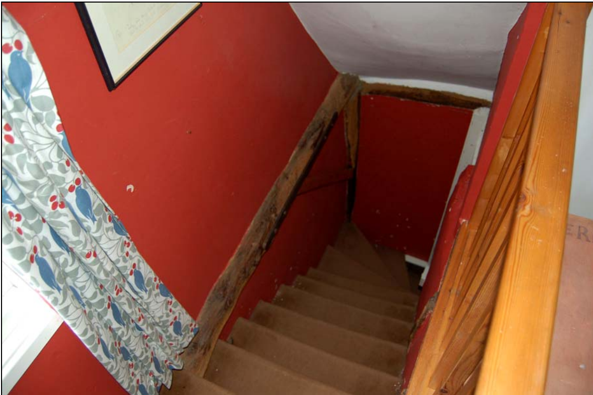
Plate 14 Back stair to attic
