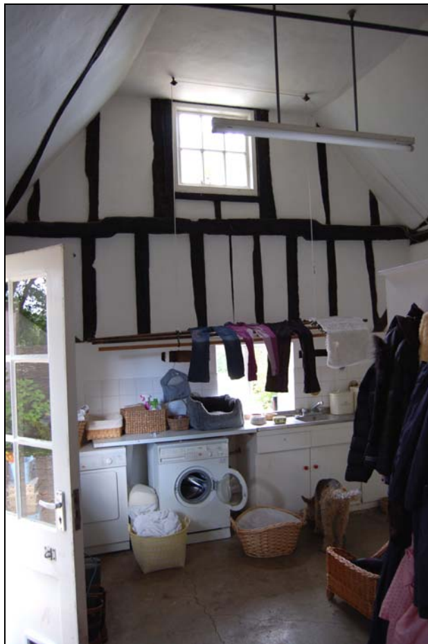
Plate 20 Framing to kitchen range gable
