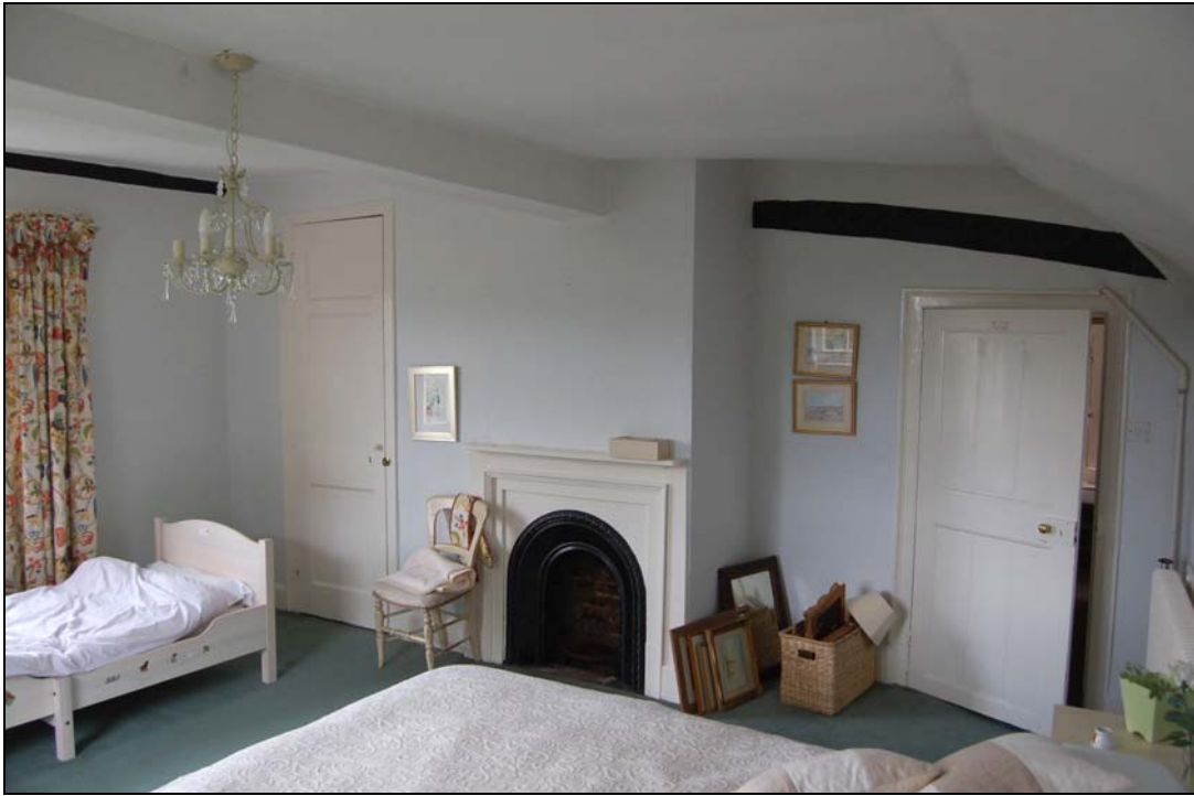
Plate 17 18th century timbers in cross wing bedroom
