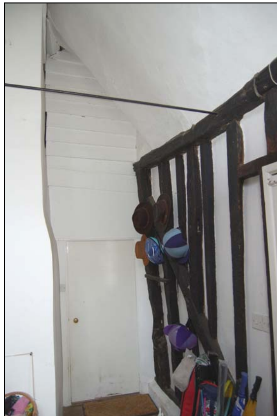
Plate 18 Trapped external boarding inside 17th century kitchen range
