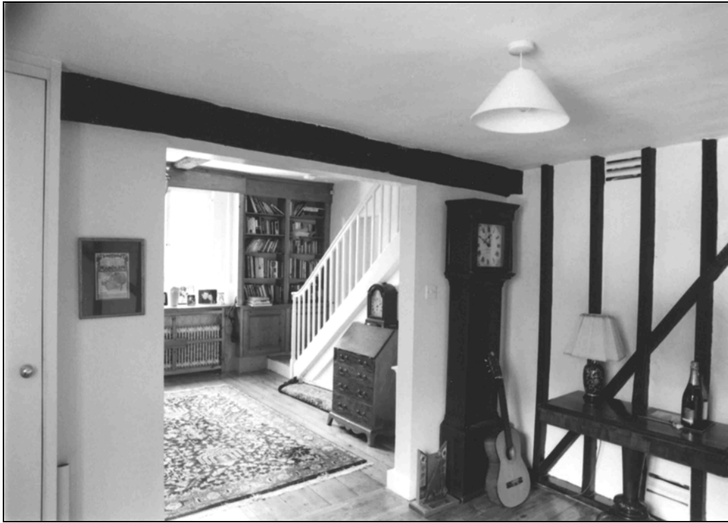
Plate 5 Midrail to front end of 16th century range, between entrance and stair hall
