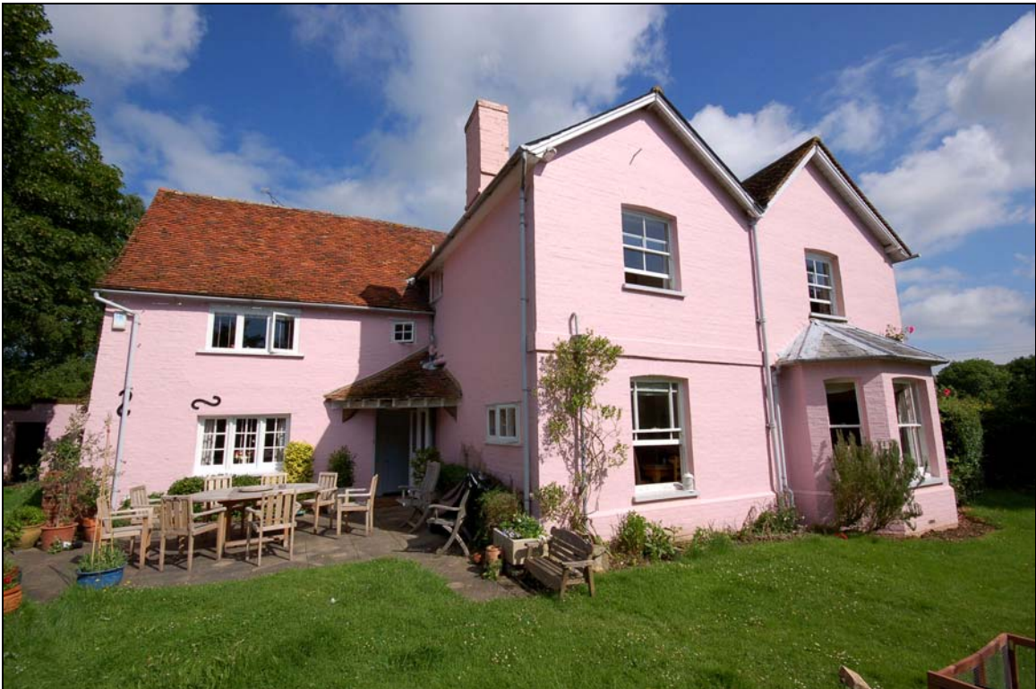
Plate 4 Garden elevation (south-east)
