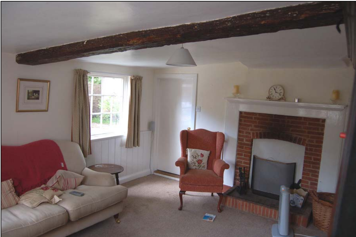
Plate 12 Bridging joist in snug
