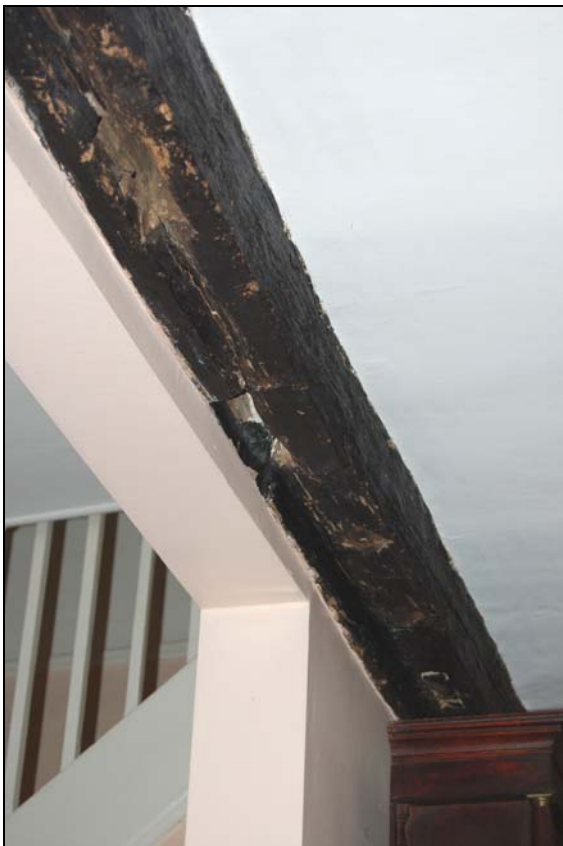
Plate 6 Mullion sockets in midrail soffit
