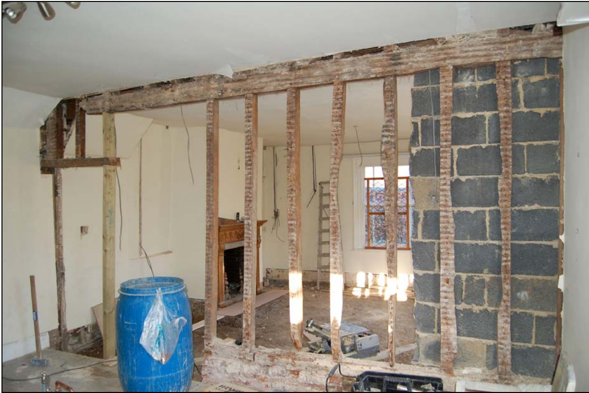
Plate 23 Typical 18th century stud walling between existing kitchen and dining room
