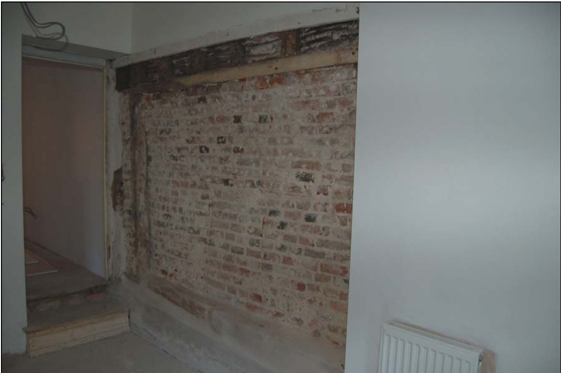
Plate 22 Stack wall in cellar exposed in building works
