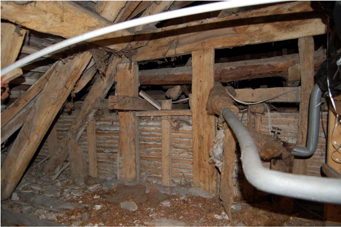
Plate 7 Gable timbers to early front, viewed in attic
