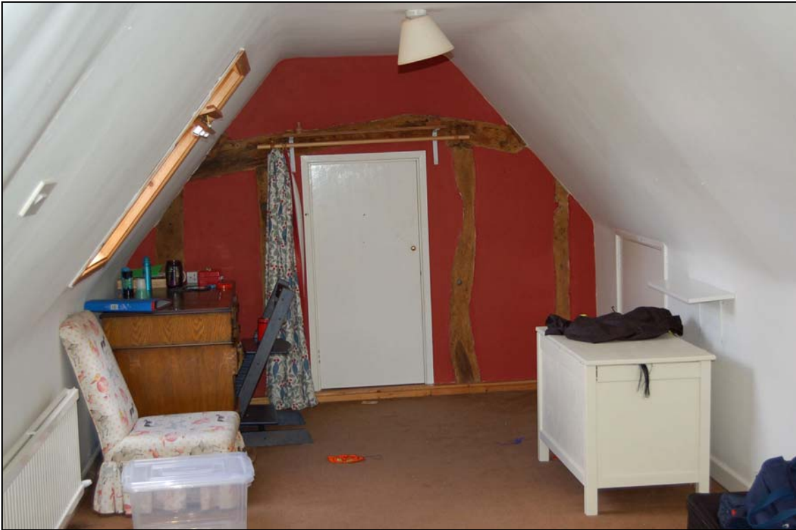
Plate 11 Continuation of partition walling into attic
