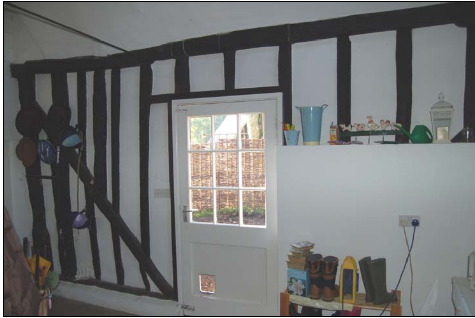
Plate 19 Exposed framing in kitchen range (utility room)
