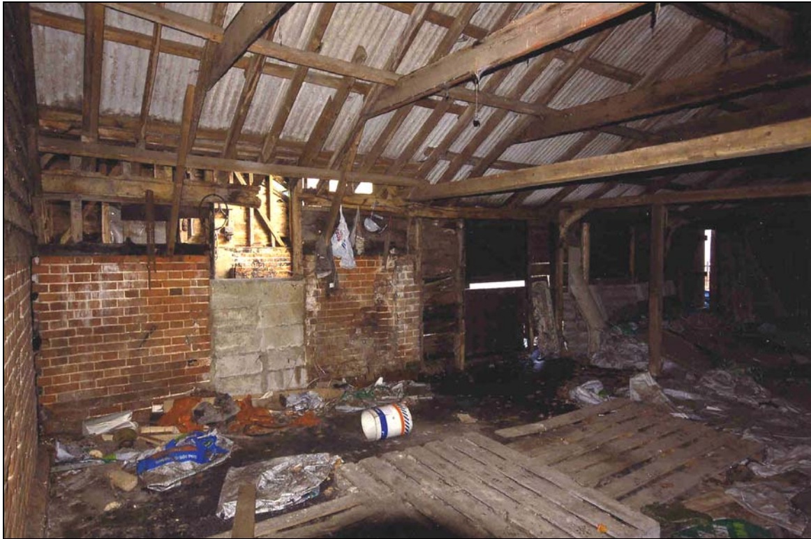
Plate 11 Interior of stables showing construction around porch and later infilling at front
