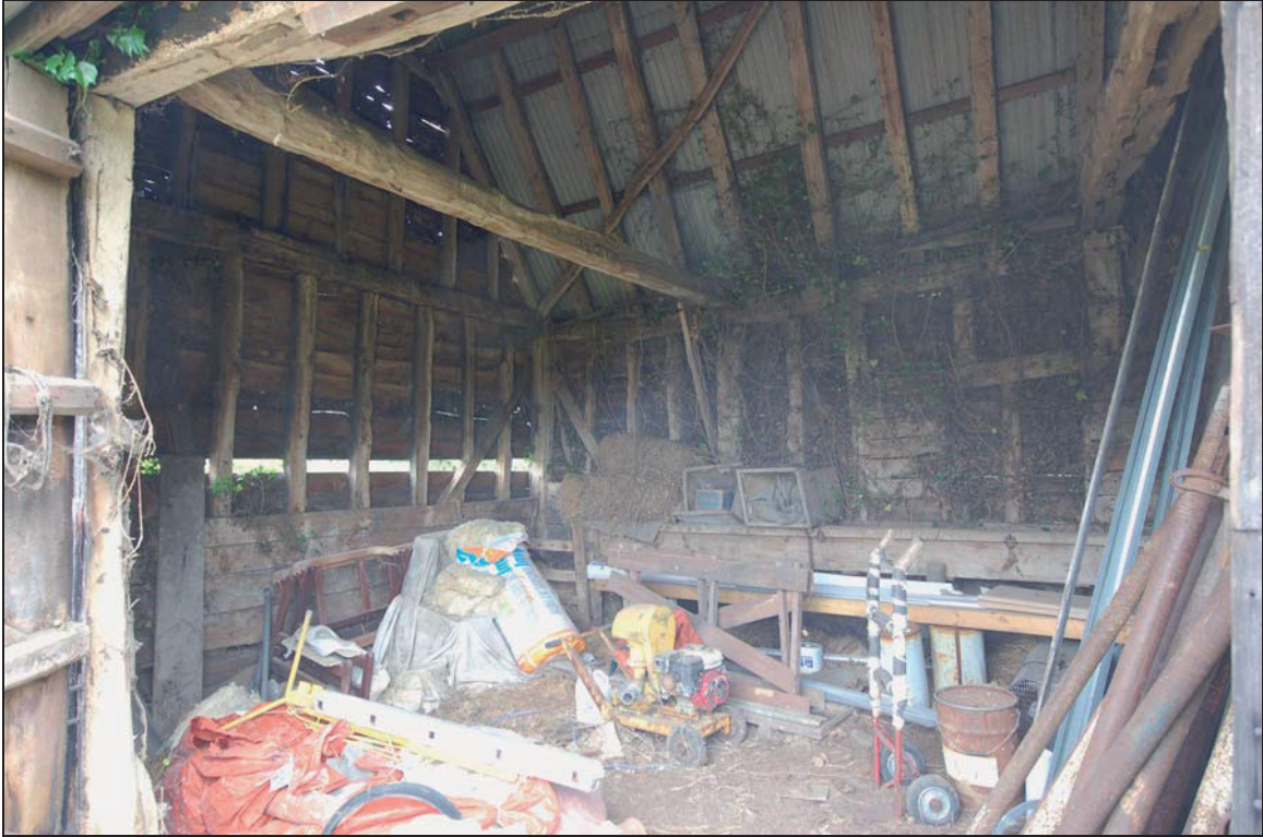
Plate 3 Interior of byre from doorway (west)
