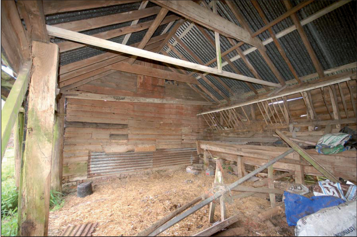
Plate 25 Interior of feeding shed viewed to hayloft door
