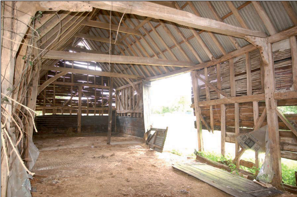
Plate 16 Interior of barn 3 viewed to west end
