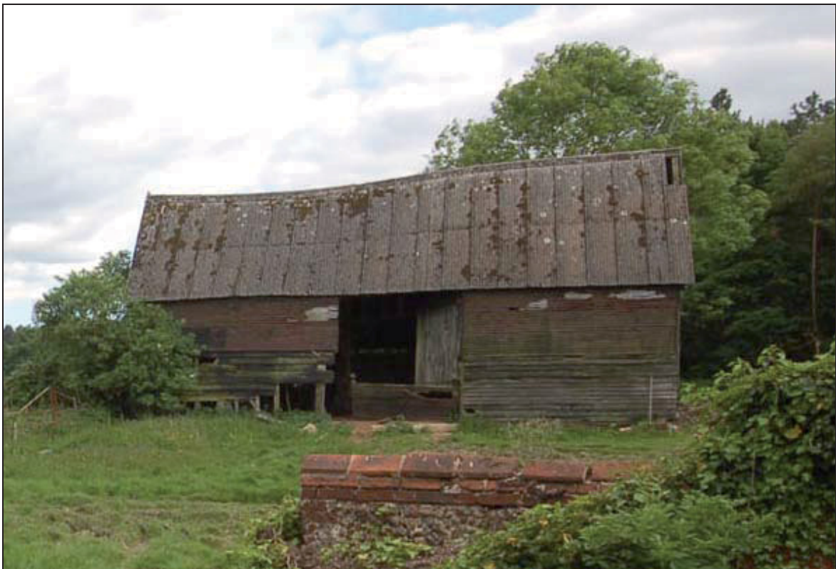
Plate 12 North elevation of barn 3
