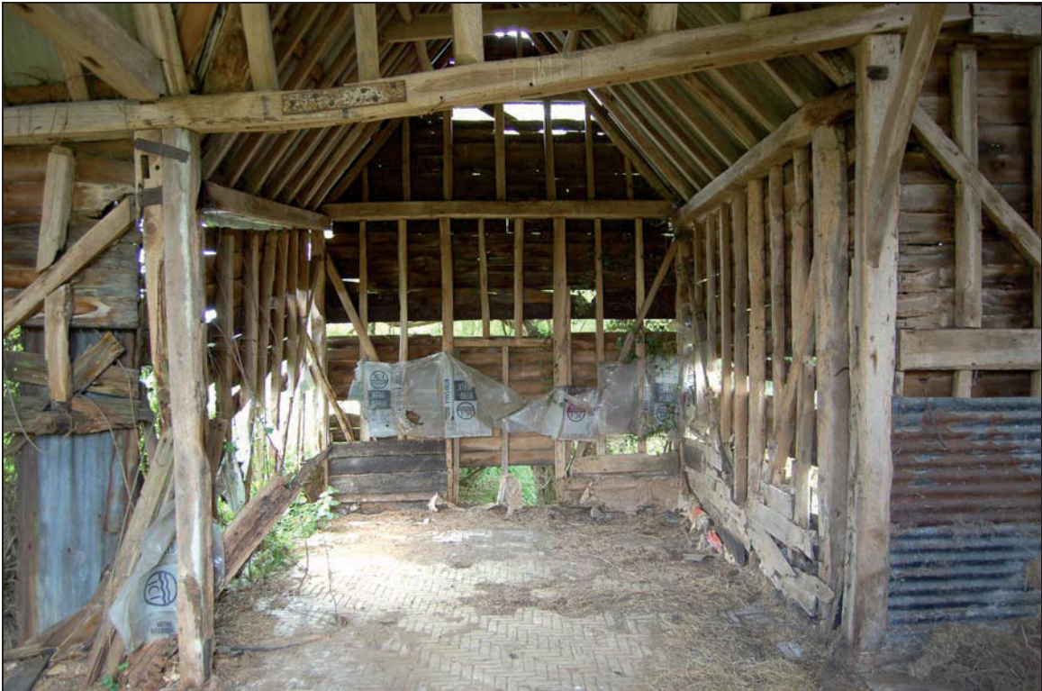
Plate 20 Porch and threshing floor in barn 3
