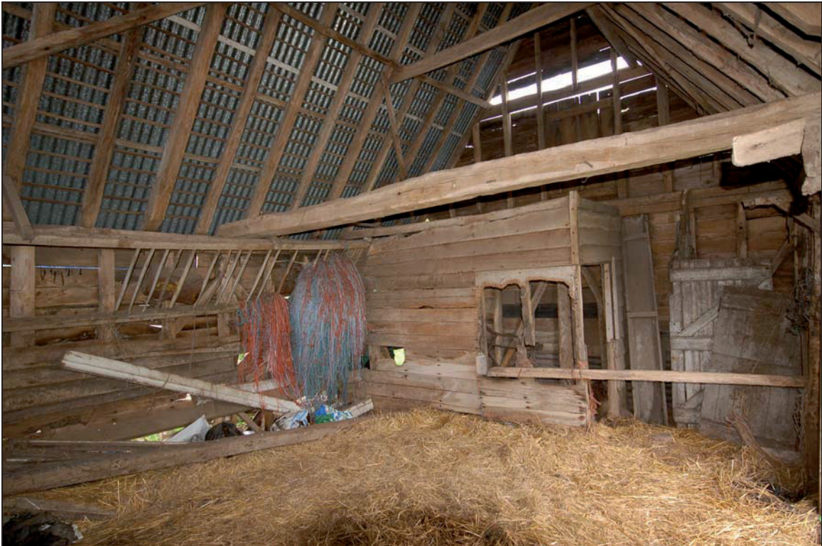
Plate 24 Feeding fixtures, store and hayloft door inside stables
