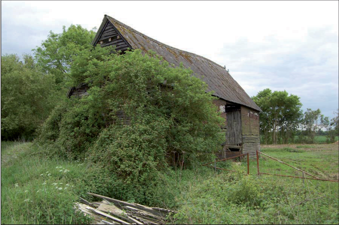
Plate 13 Barn 3 viewed from north-east
