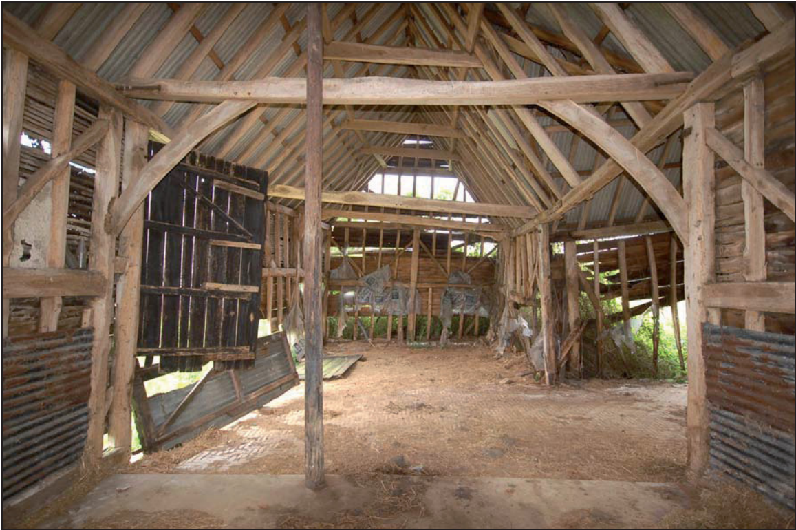
Plate 17 Interior of barn 3 viewed to east end
