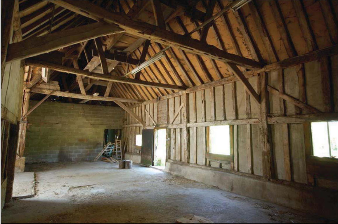
Plate 13 East side of Barn 3 viewed to west
