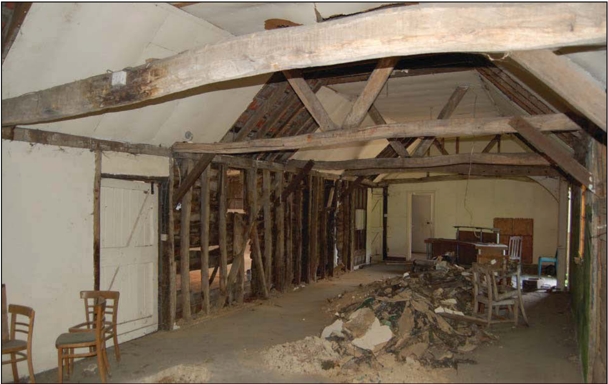
Plate 32 Interior of Shed 7 viewed to south-east
