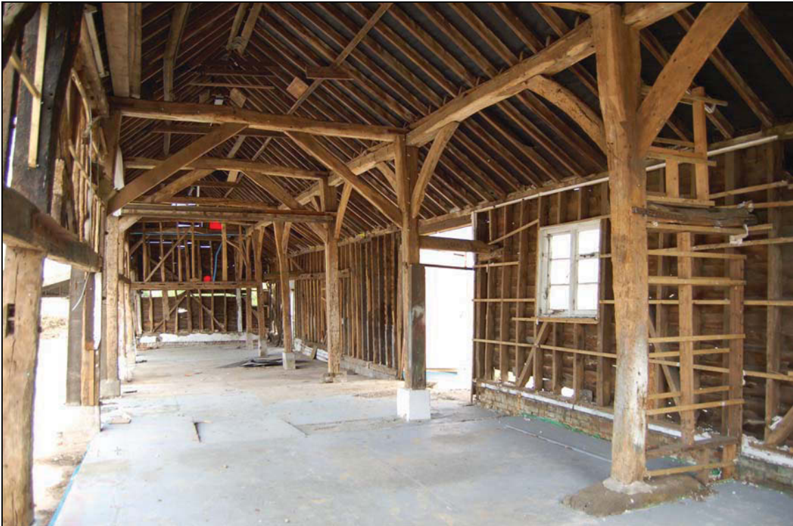
Plate 20 Interior of Barn 4 viewed to north end
