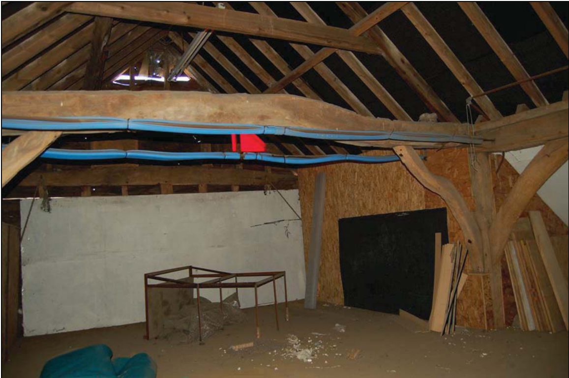
Plate 24 Crude bracing in northern bays
