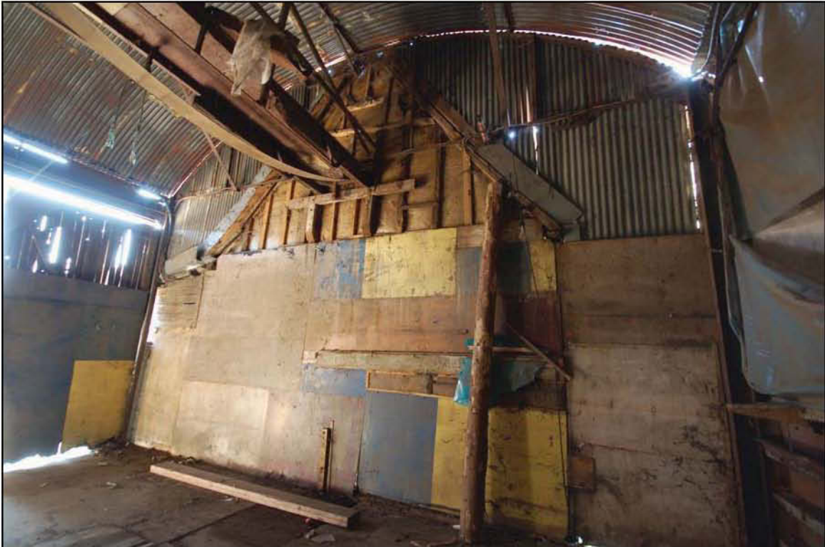
Plate 10 East wall of Barn 3 enclosed within Grain Store 13
