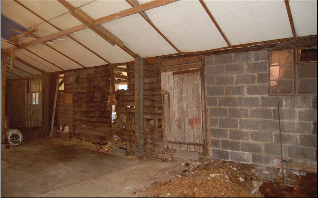
Plate 31 East wall of Shed 7 viewed inside Workshop 10
