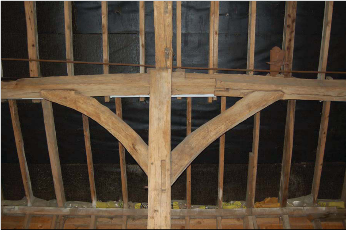
Plate 25 Bridge-scarf joint beside truss 4 viewed towards rebuilt aisle
