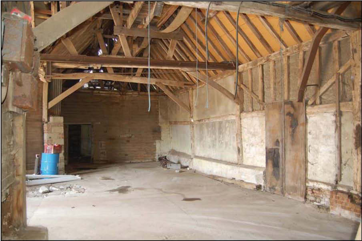
Plate 11 West side of Barn 3 viewed to west end
