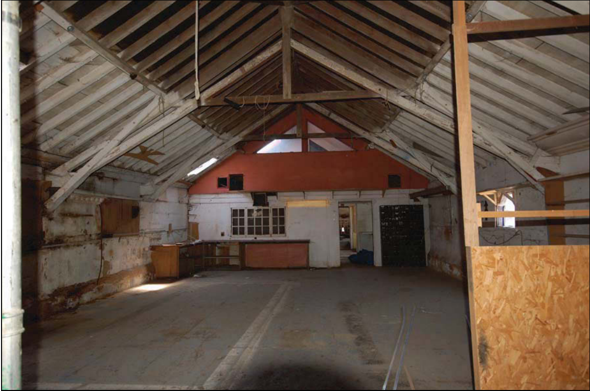
Plate 29 Interior of Building 6 viewed to north
