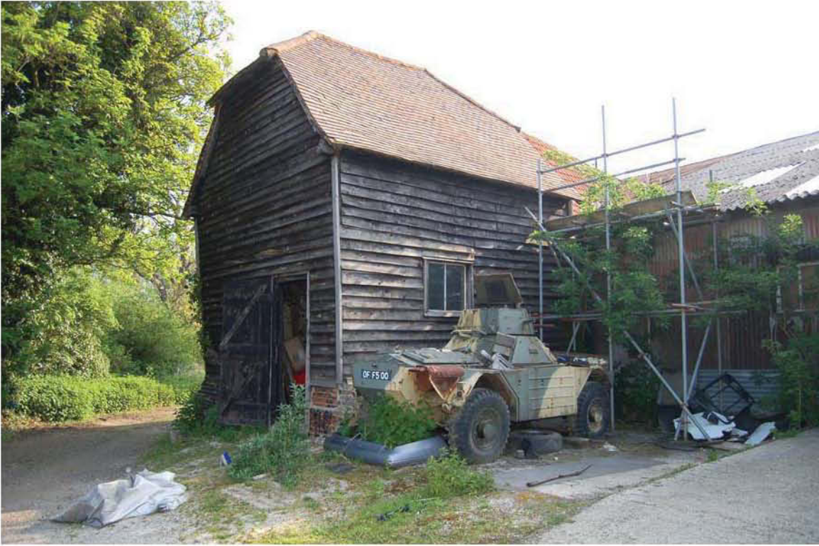
Plate 1 Dovecote 1 viewed to north-east
