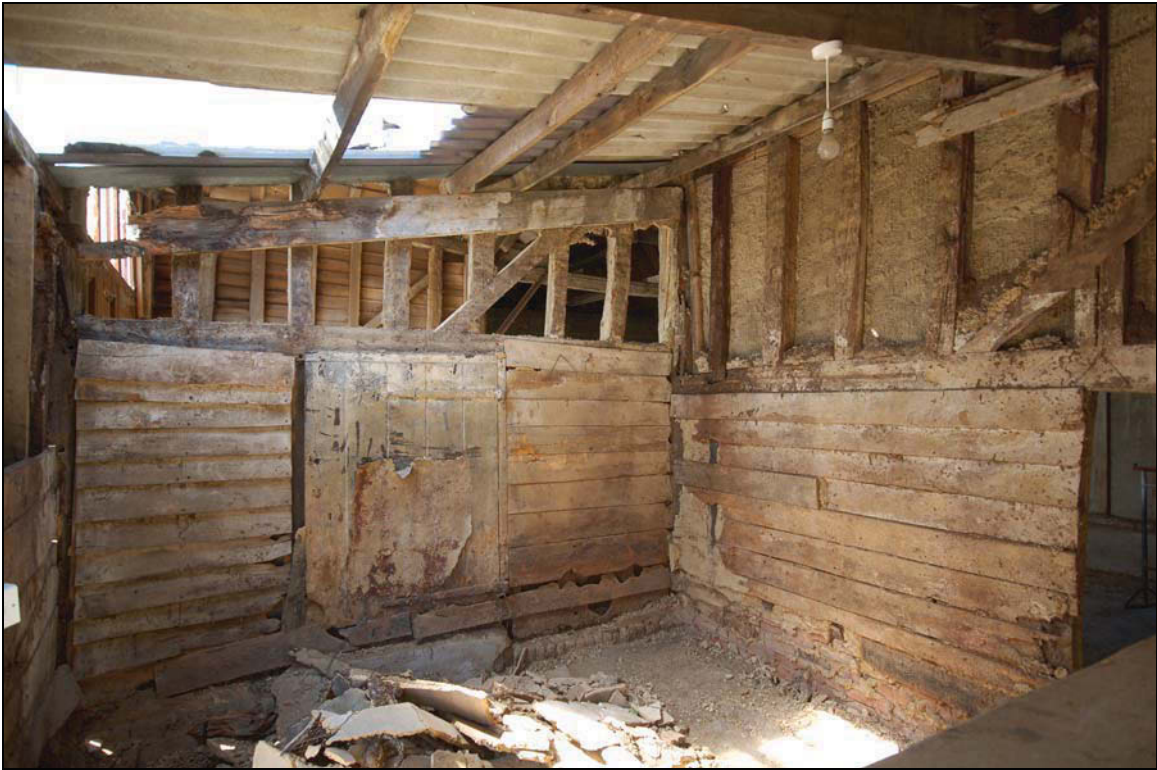
Plate 15 Side entrance to east porch viewed from inside Shed 3b
