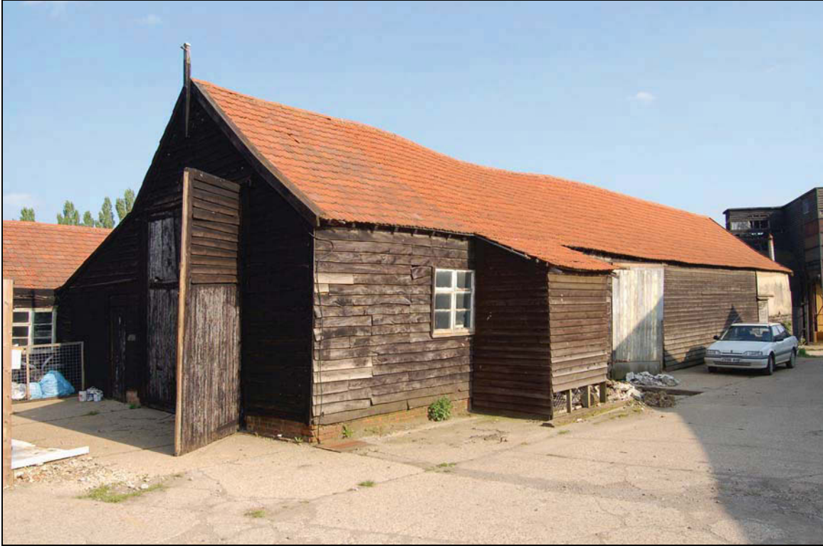
Plate 17 Barn 4 viewed to north-west
