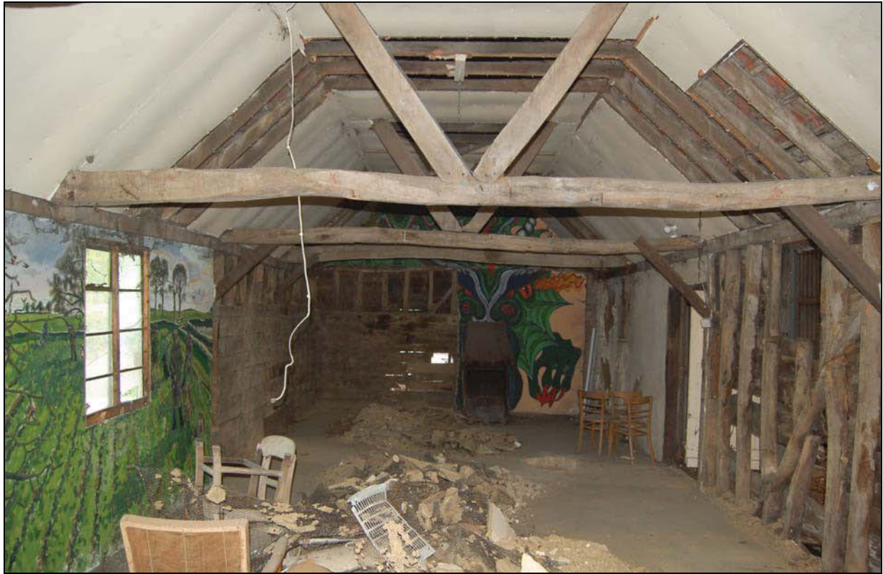
Plate 33 Interior of Shed 7 viewed to north end
