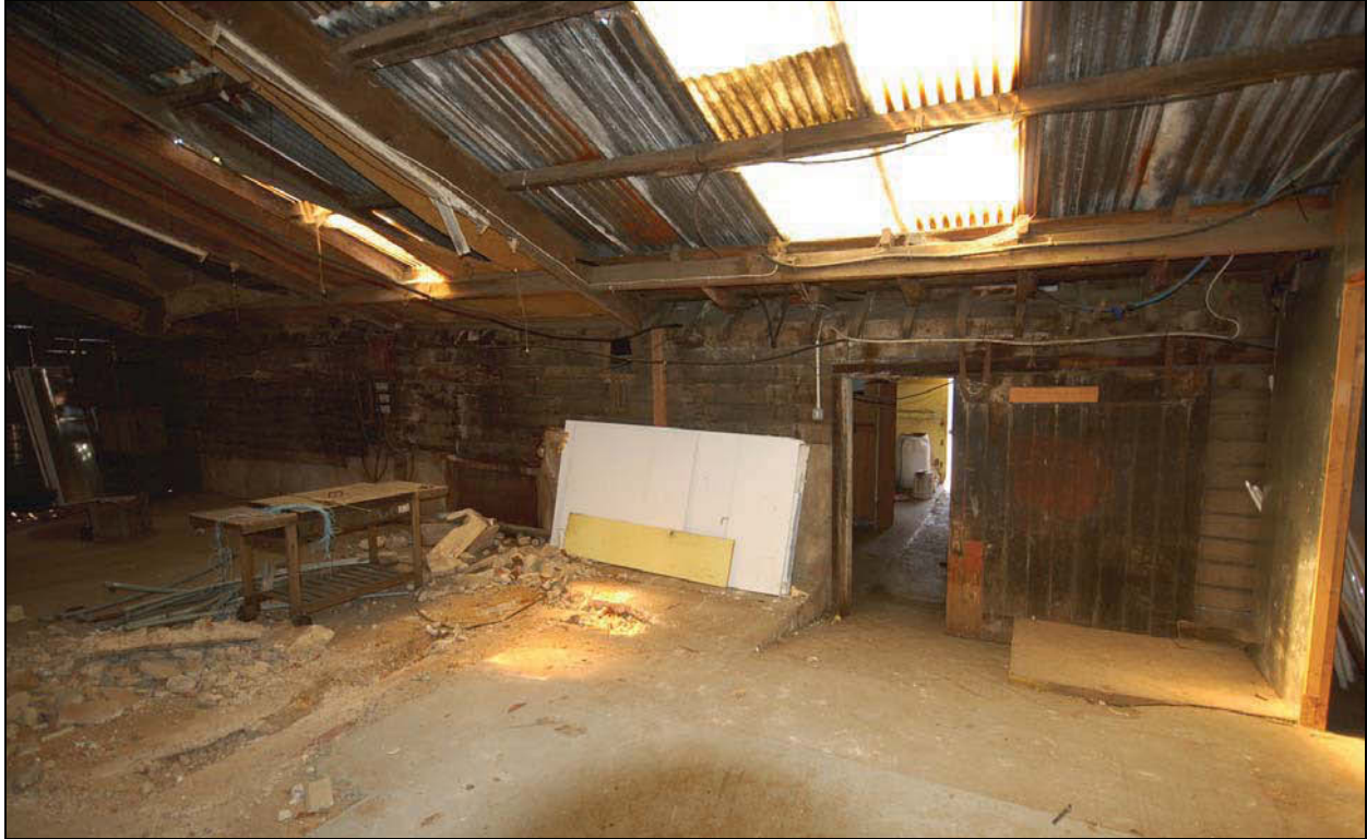
Plate 27 Plinth to Barn 4 porch viewed inside Building 5
