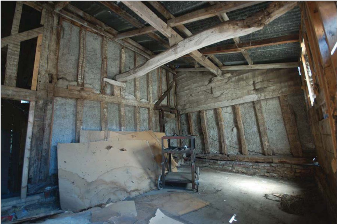
Plate 16 Interior of Shed 3a viewed toward west porch
