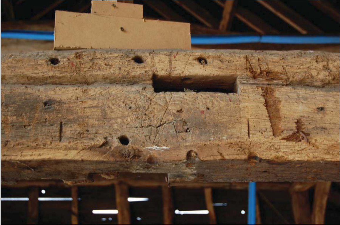
Plate 23 'Fair face' mark on midrail of north partition
