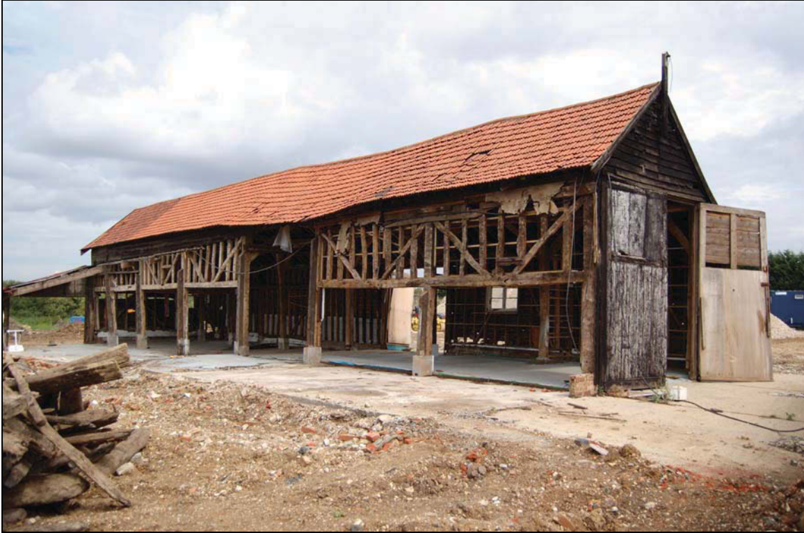
Plate 19 West side of Barn 4 after removal of Building 5
