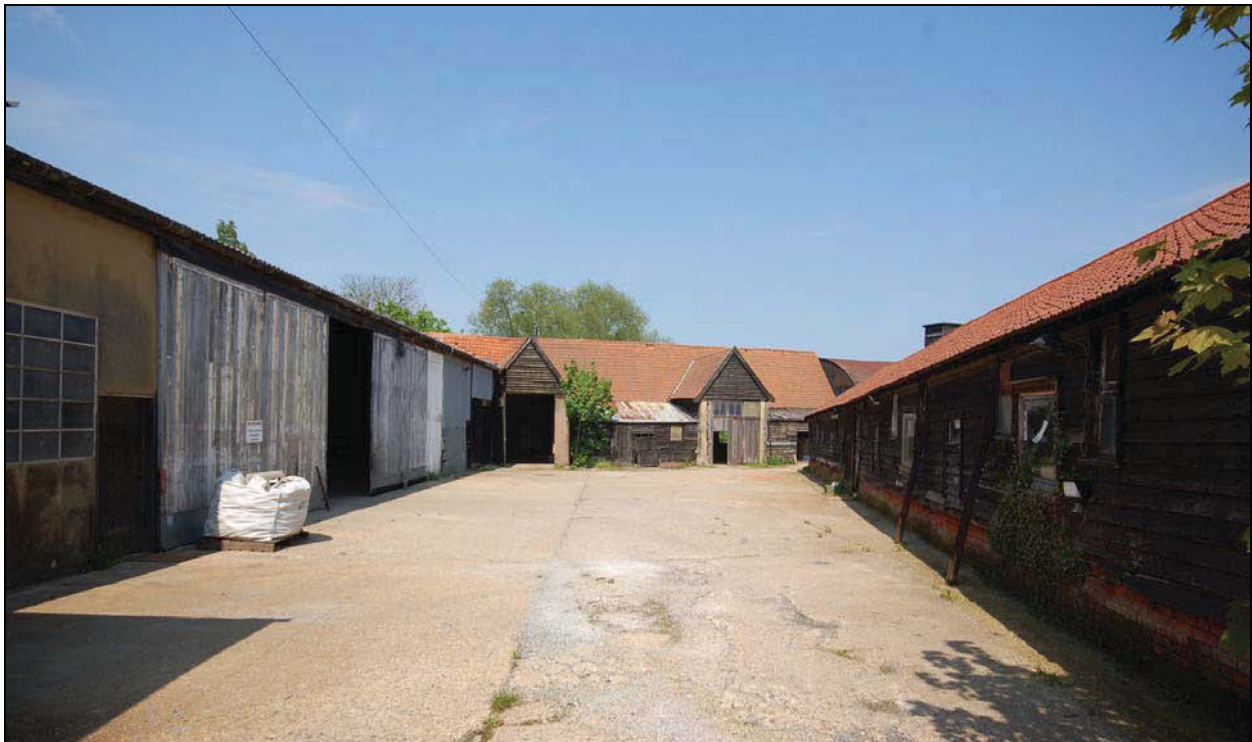
Plate 28 West elevation of Building 6 (to right) opposite Workshops 9 & 10
