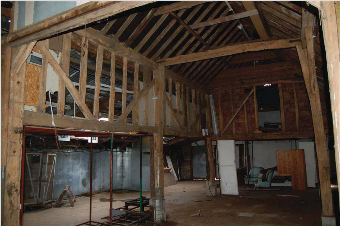
Plate 22 Removed lower register on west side of Barn 4
