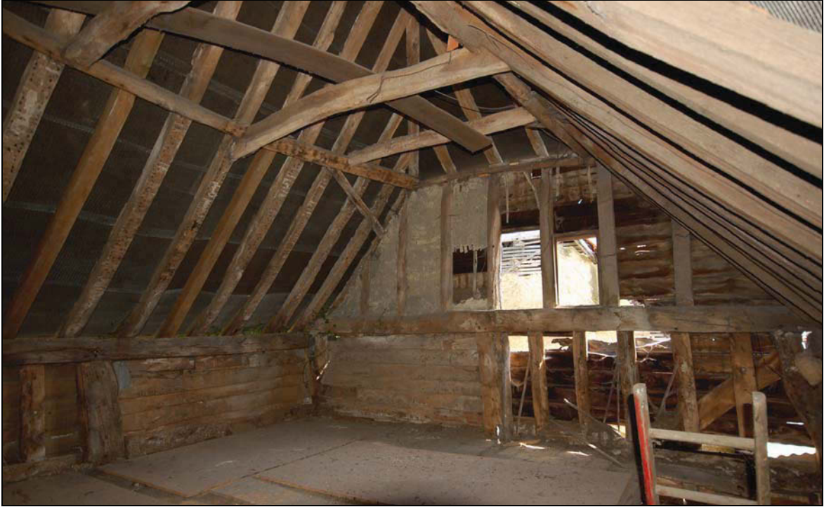
Plate 3 Inserted first floor of Dovecote 1 viewed to north-east
