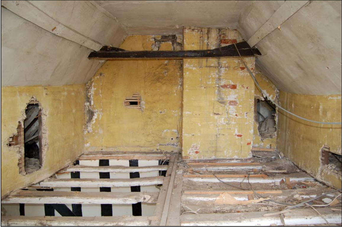
Plate 15 Attic of building 2
