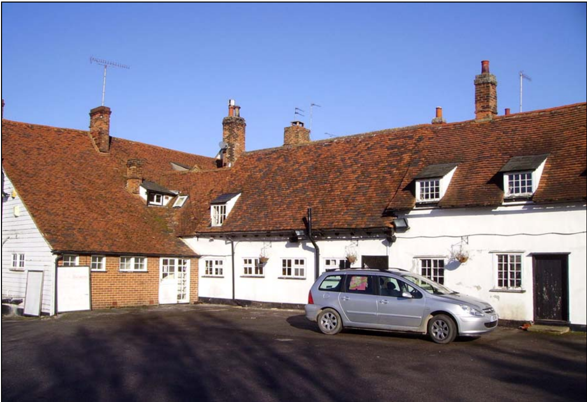
Plate 16 Rear of public house before conversion
