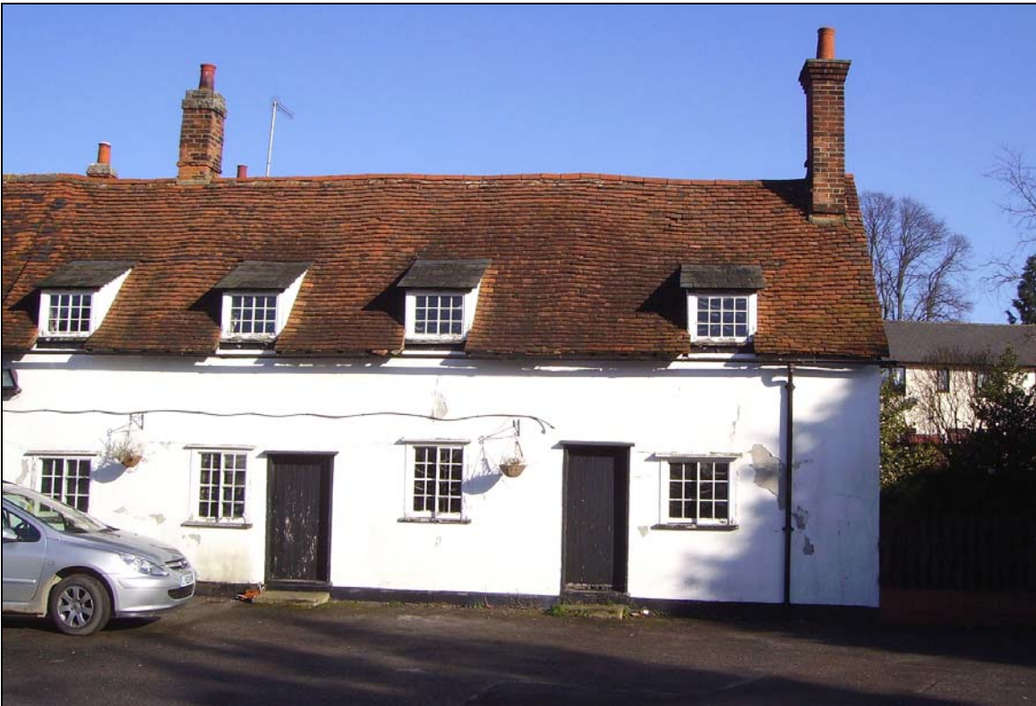
Plate 20 Cottages before refurbishment
