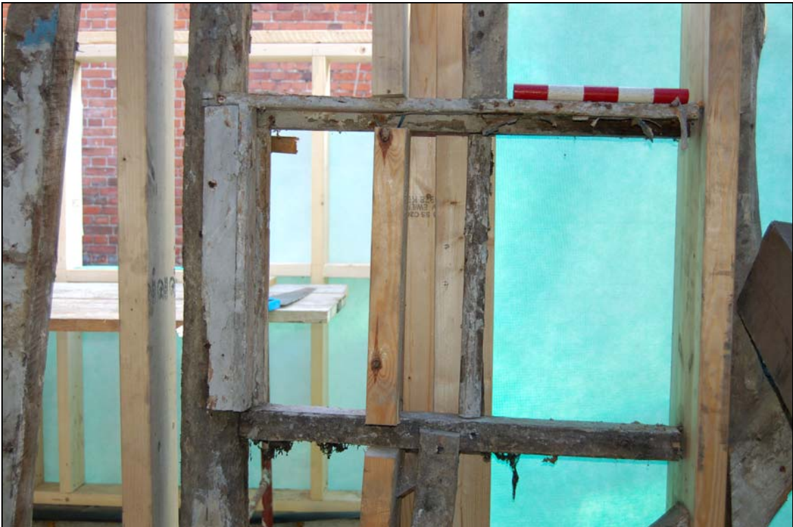
Plate 24 Remains of 18th-century window on north-east wall
