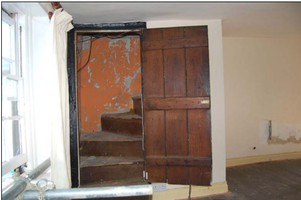
Plate 12 Attic stair (north-east end)
