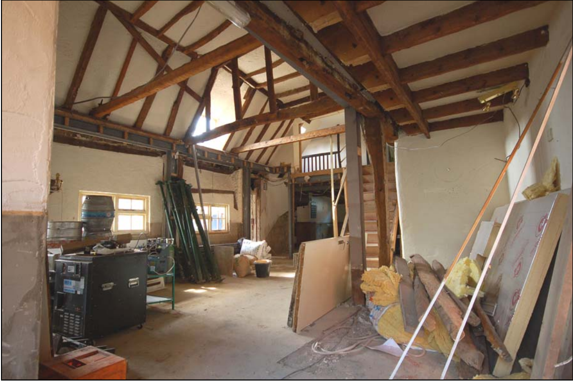
Plate 19 Removed north-east wall of rear wing
