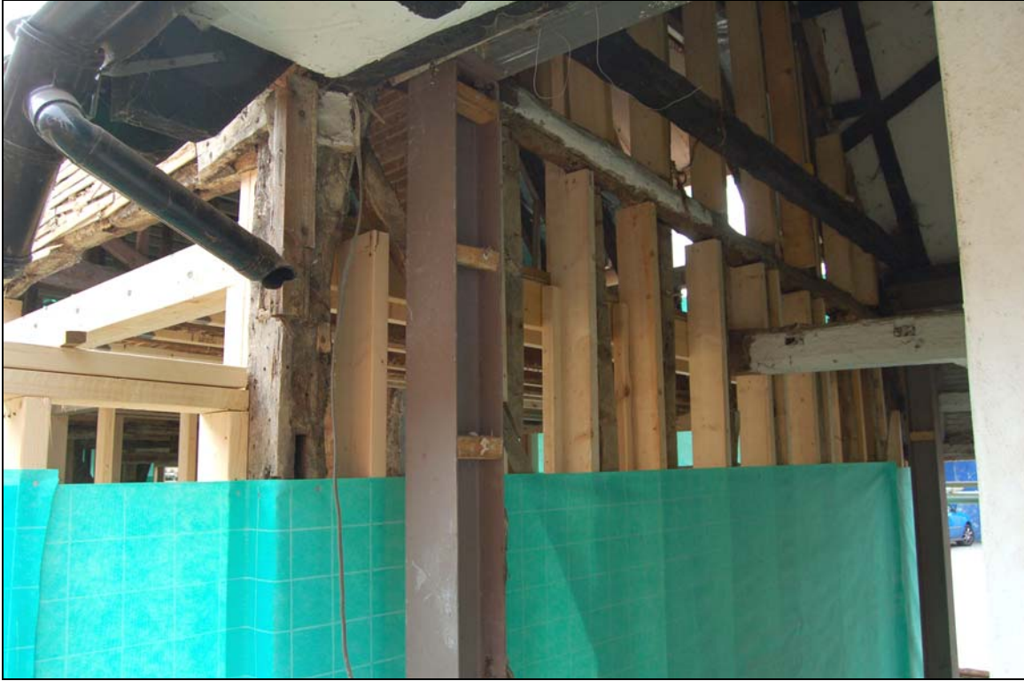
Plate 17 Jowled corner post and rebuilt end wall of former rear wing
