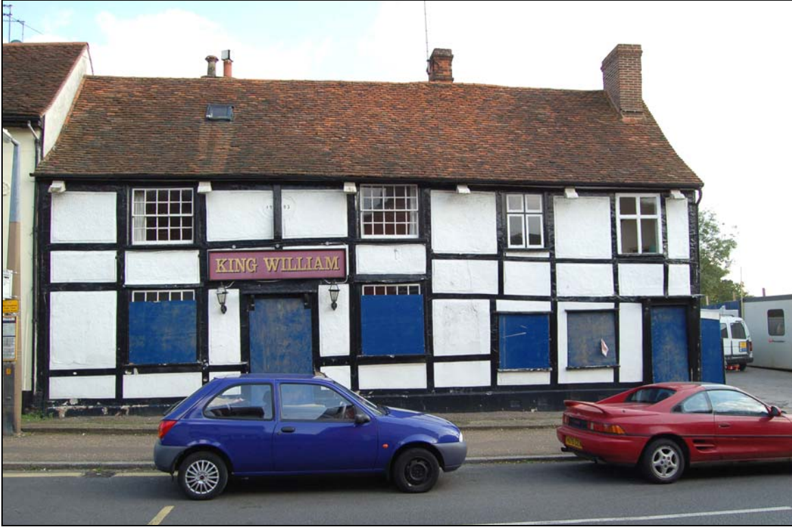
Plate 1 The King William from Church Street (main façade)
