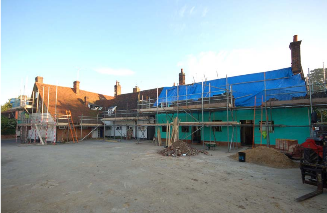
Plate 5 King William and cottages during refurbishment
