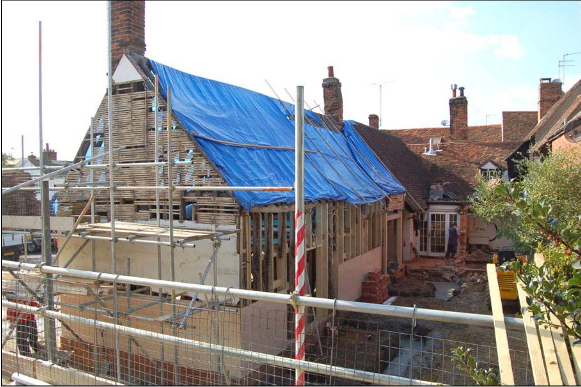
Plate 21 Cottages during refurbishment and rear of public house
