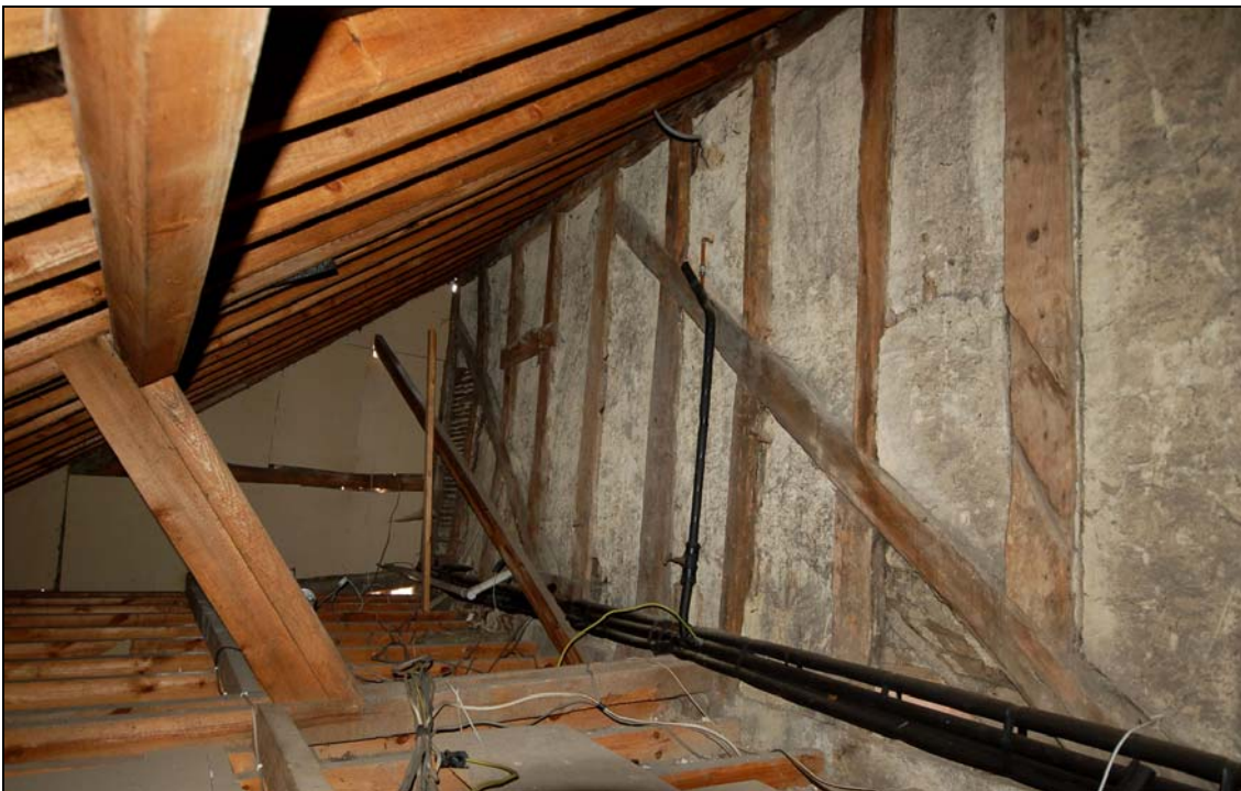
Plate 6 Primary-braced timbers behind the catslide roof
