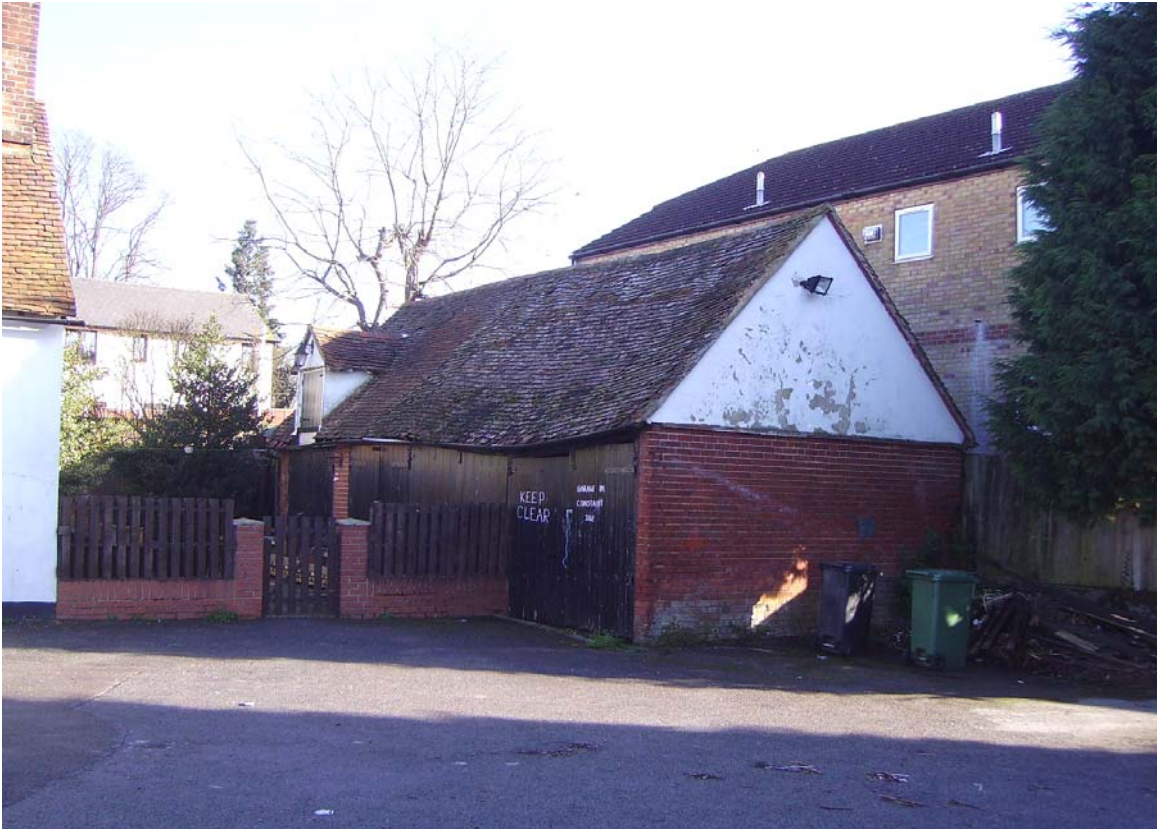
Plate 25 Coach house before conversion
