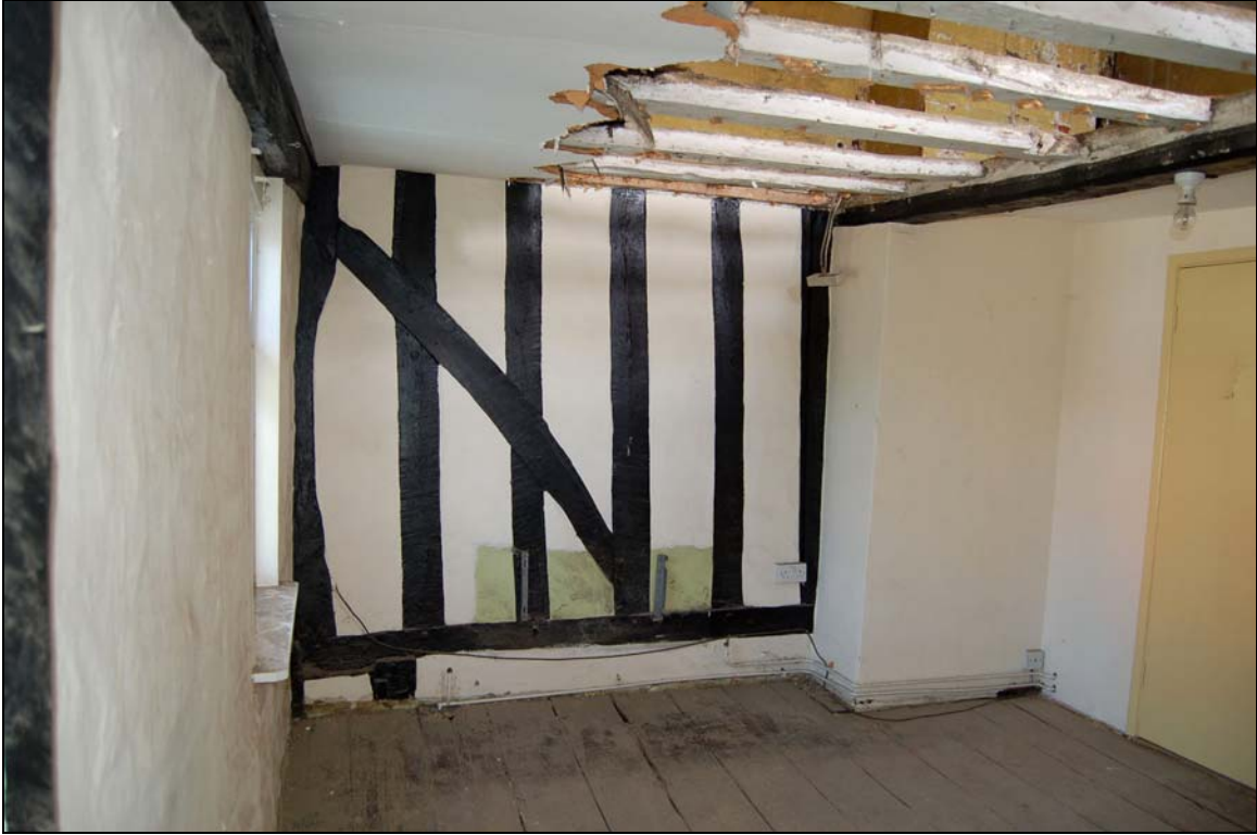
Plate 3 Original south-eastern end wall
