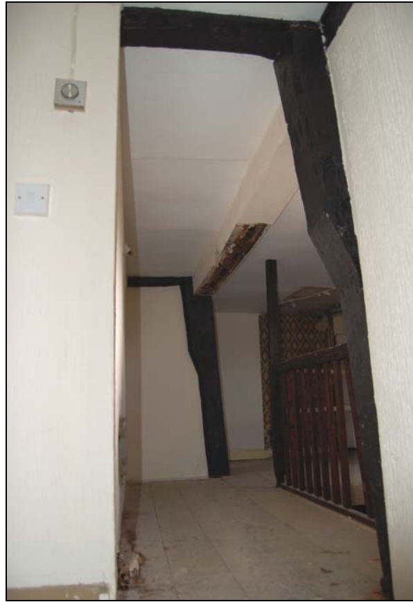
Plate 11 Jowled bay posts on line of former rear wall
