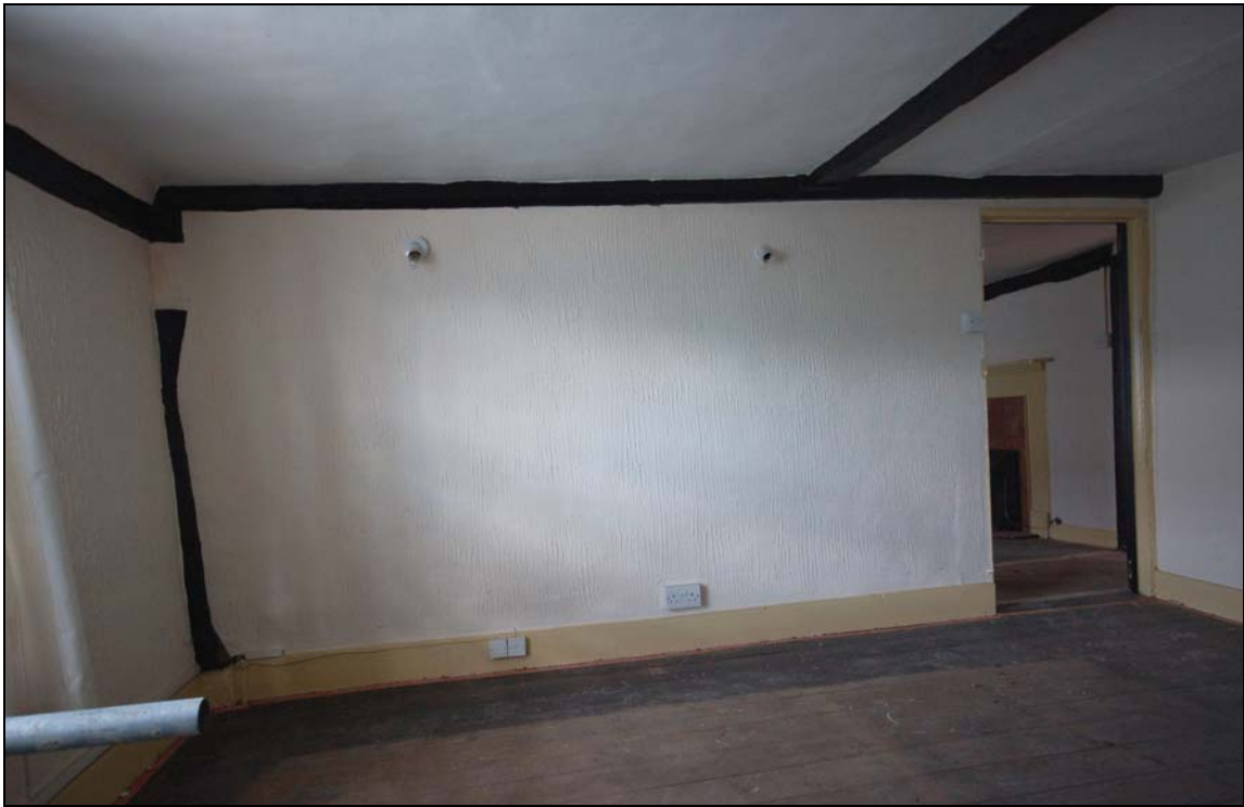
Plate 10 Inserted first floor partition wall
