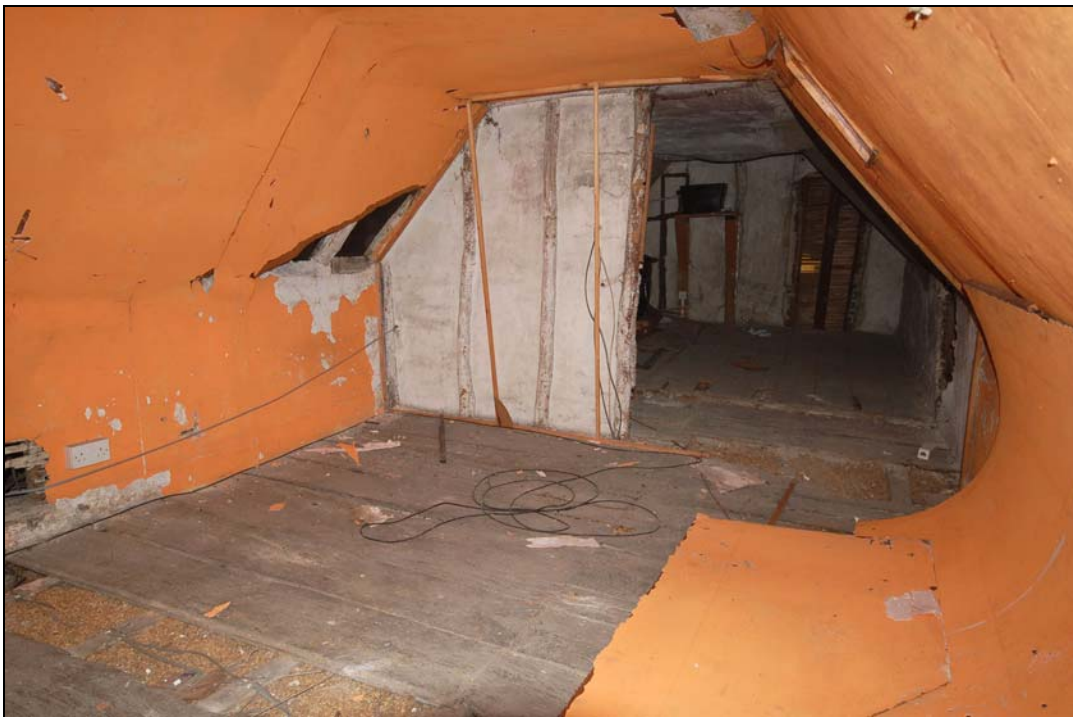
Plate 14 Main attic and original end wall (beyond partition)
