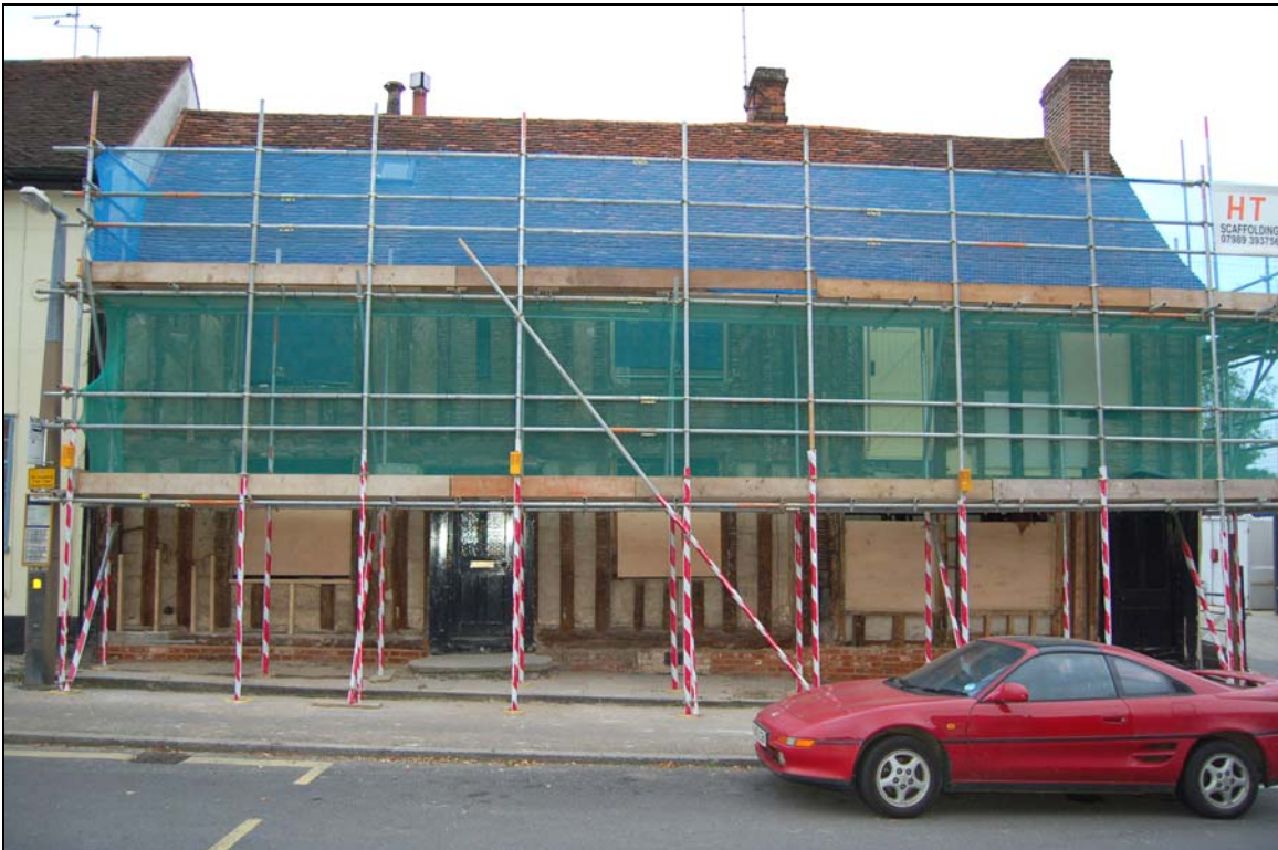
Plate 2 Framing exposed on the main façade
