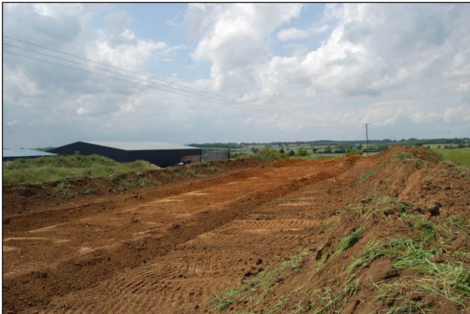
Plate 2. Industrial unit site. Central section stripped by bulldozer. Looking south-west
