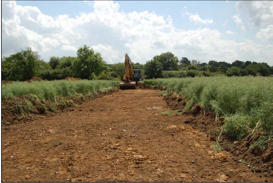
Plate 1. Haul road. Looking south
