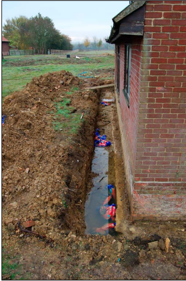
Plate 3. Underpinning trench, north side of house. 1m scale bar
