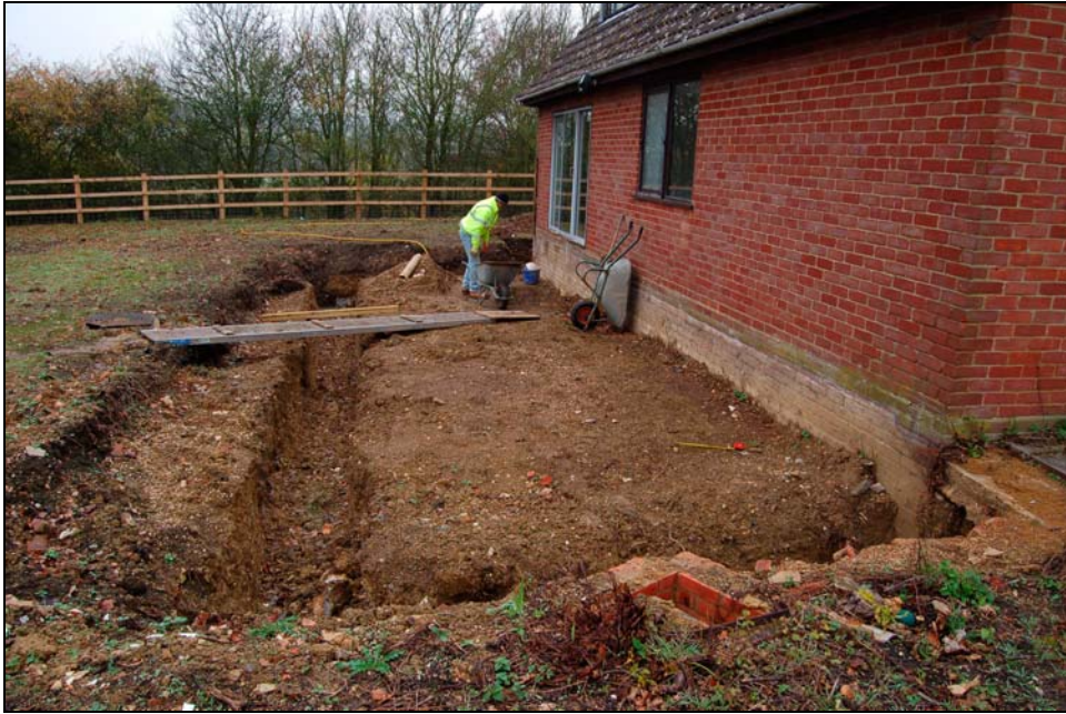
Plate 1. Ground clearance and extension foundation trench, south side of house
