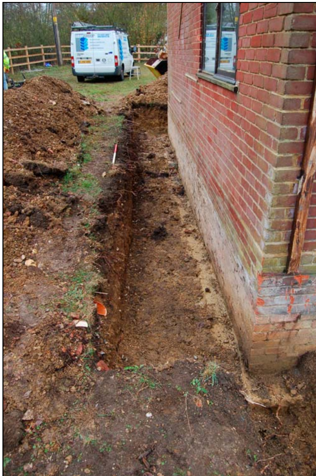
Plate 2. Underpinning trench, west side of house. 1m scale bar
