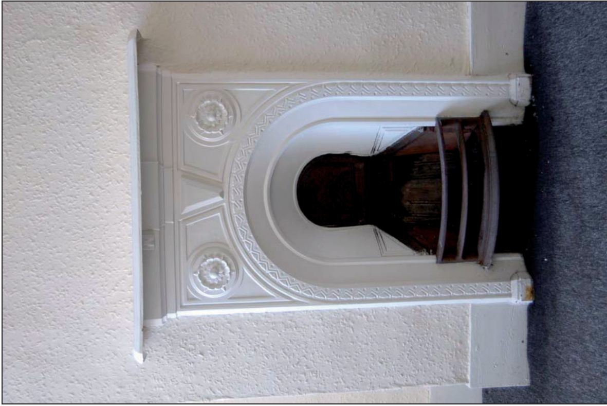
Plate 23 Typical bedroom fireplace (cottage 9)
