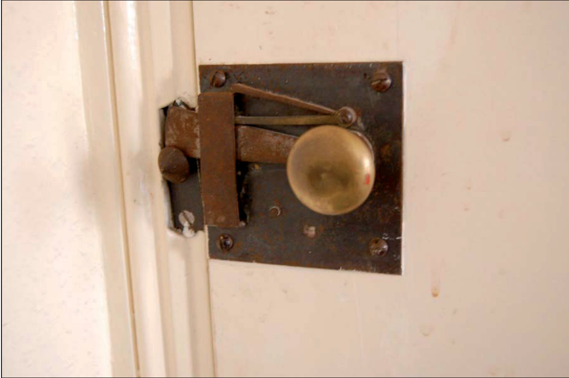
Plate 25 Sprung latch mechanism (cottage 3)
