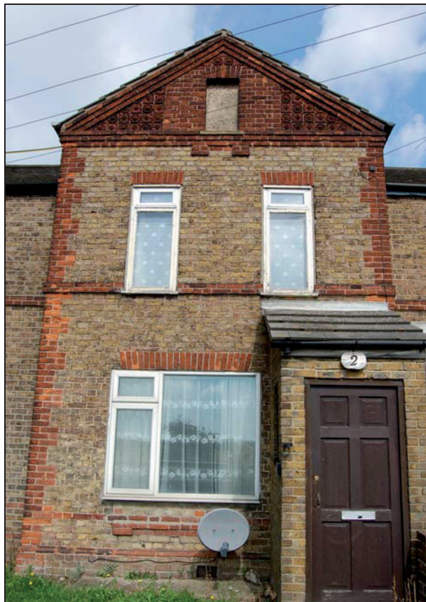
Plate 4 Gable of cottage 2
