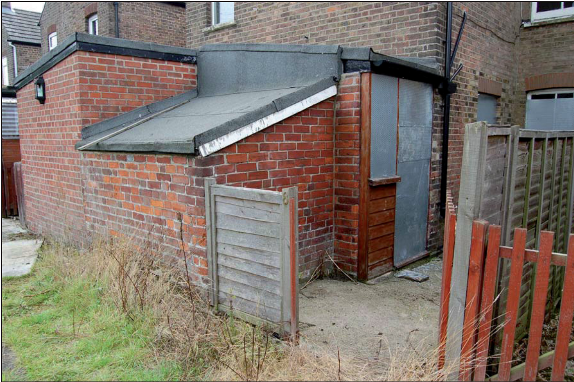
Plate 13 Surviving outbuildings enclosed under modern roof (cottage 8)
