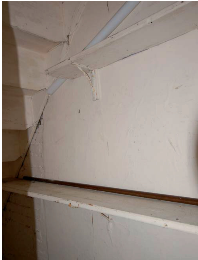
Plate 18 Shelves inside stair cupboard
