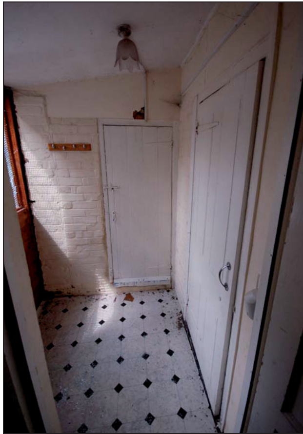
Plate 20 Enclosed toilet/coal house range
