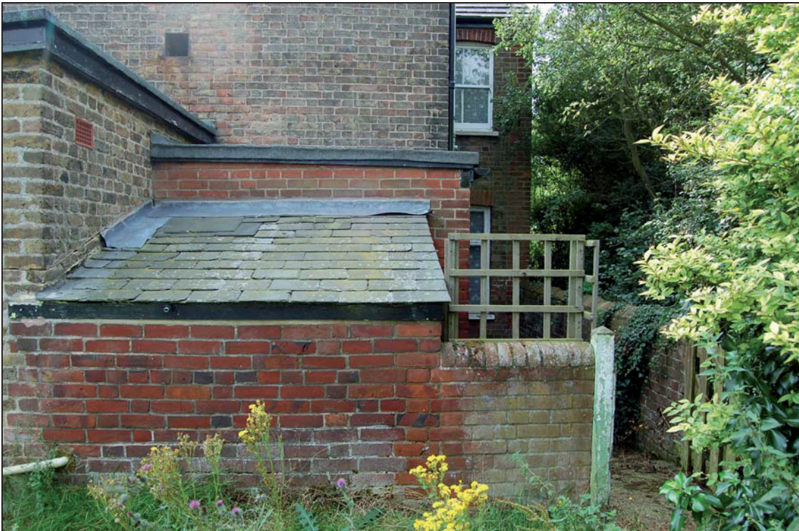
Plate 14 Rear wall and enclosed outbuildings (cottage 10)
