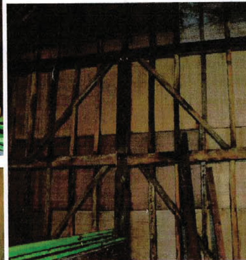
Detail of replacement central storey post at southern gable end.
