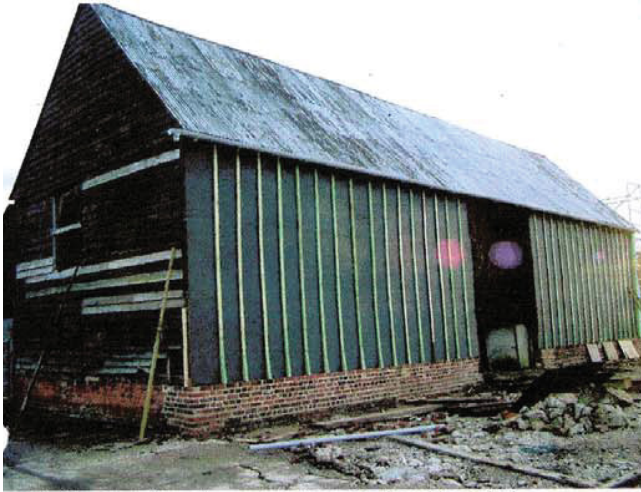
Outside view of north-west wall, repaired and boarded.
