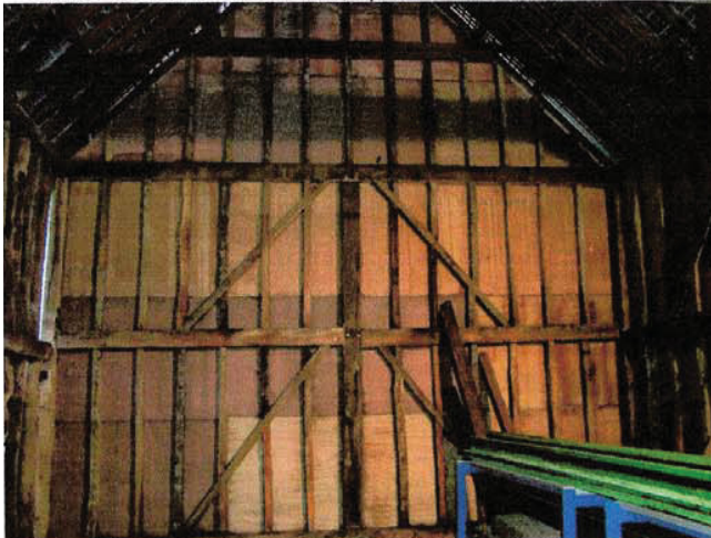
Internal view of repaired southern gable wall.
