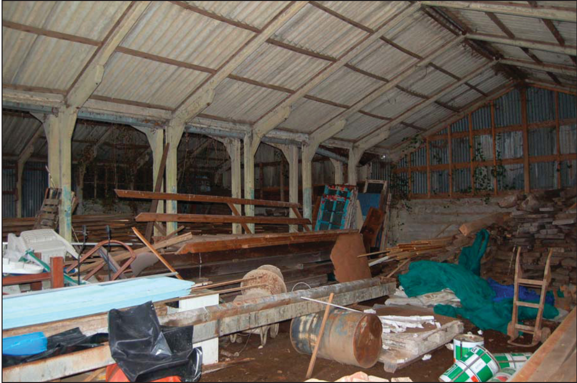
Plate 17 Interior of building 10
