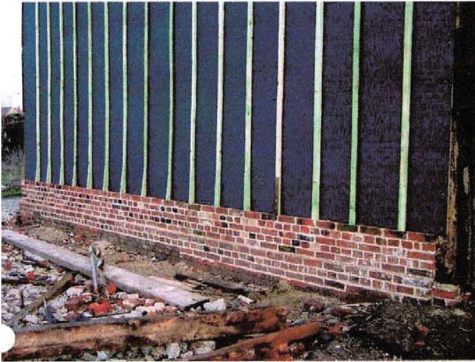
North-west corner plinth rebuilt from where slurry tank removed.
