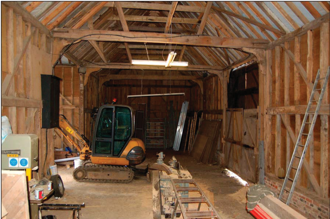
Plate 4 Refurbished barn interior viewed to south-west
