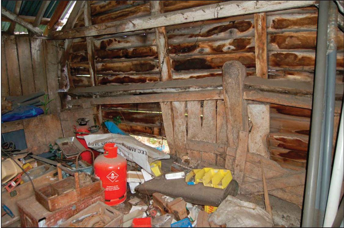
Plate 11 Nag stable wall built onto existing stock fence
