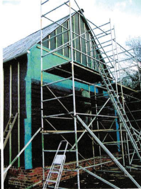
Southern gable having weather board applied.
