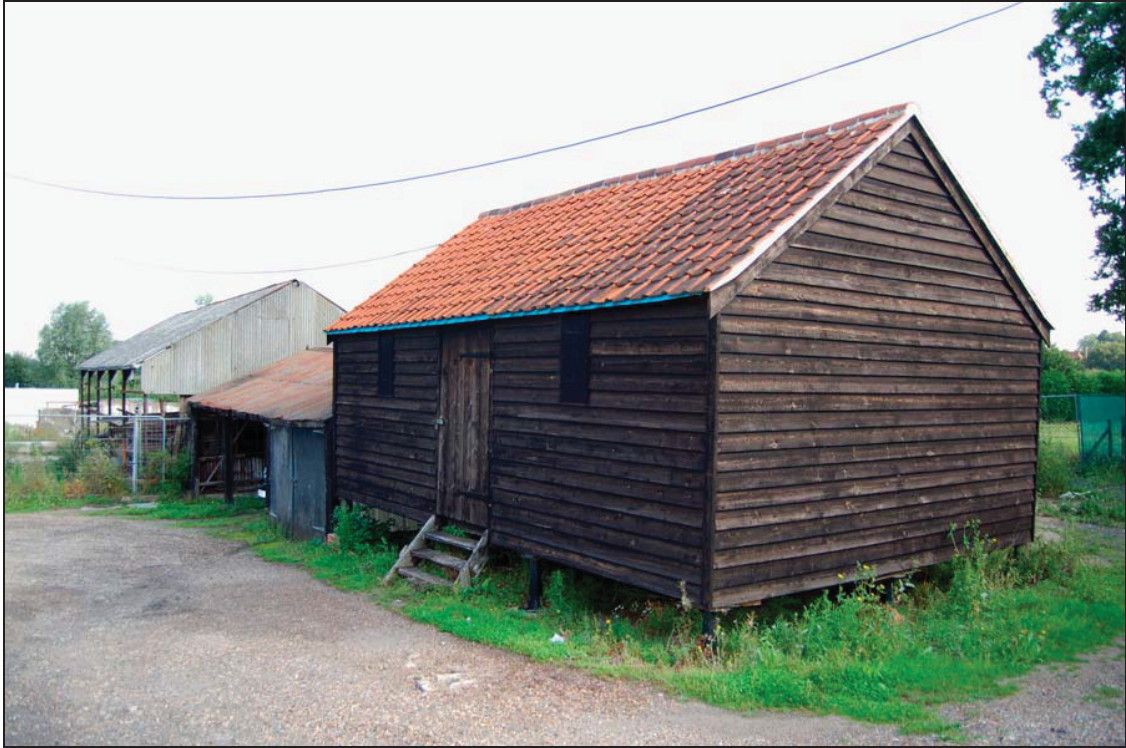
Plate 5 Granary viewed to north
