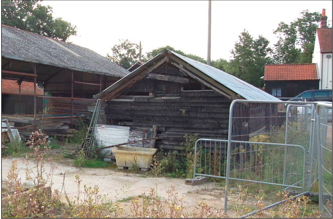
Plate 7 Nag stable viewed to south-east
