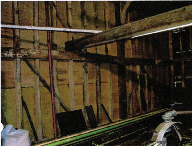
Inside view of north-west wall after repair.
