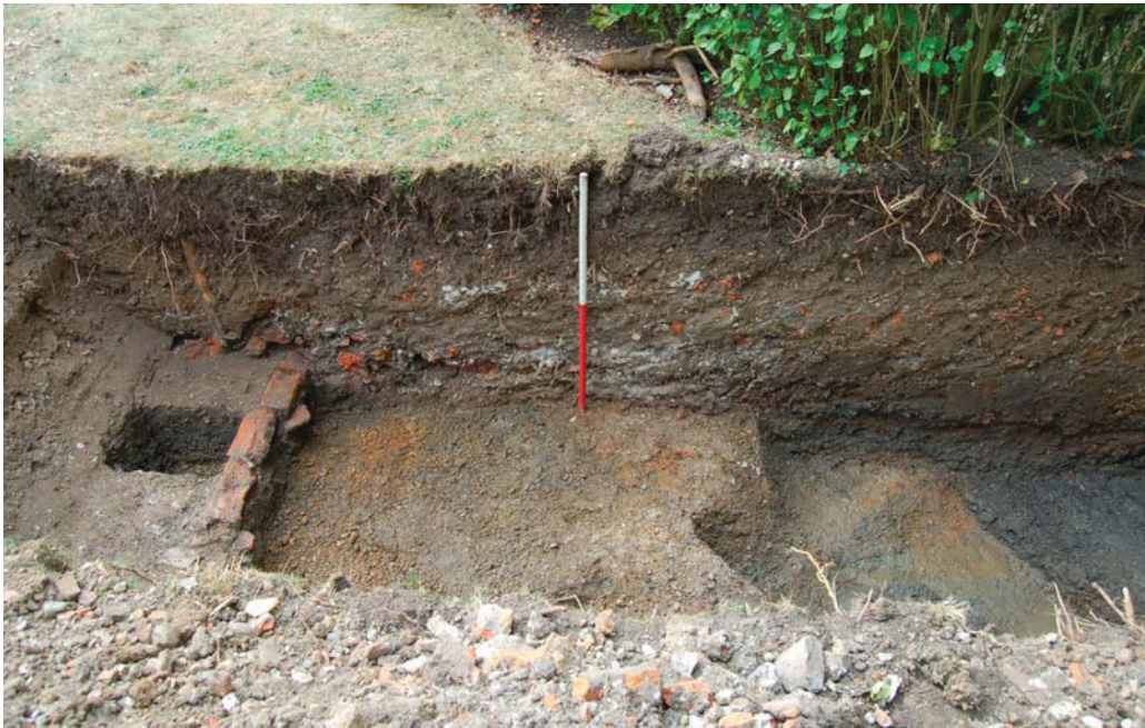
Plate 3: Wall 10, looking south, 1m scale
