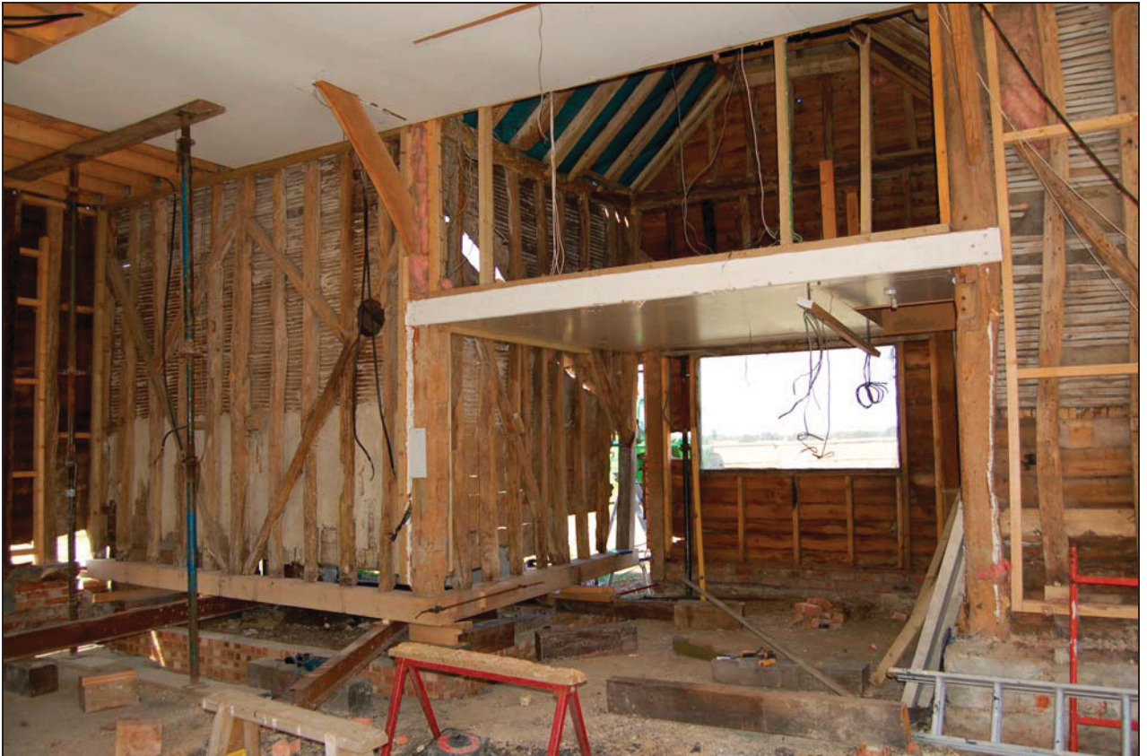
Plate 6 Porch and diamond-shaped bracing on north side of barn 1
