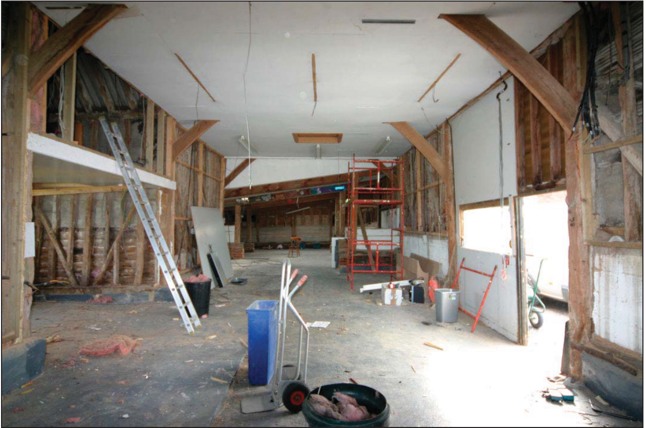
Plate 5 Interior of barn 1 viewed towards barn 2
