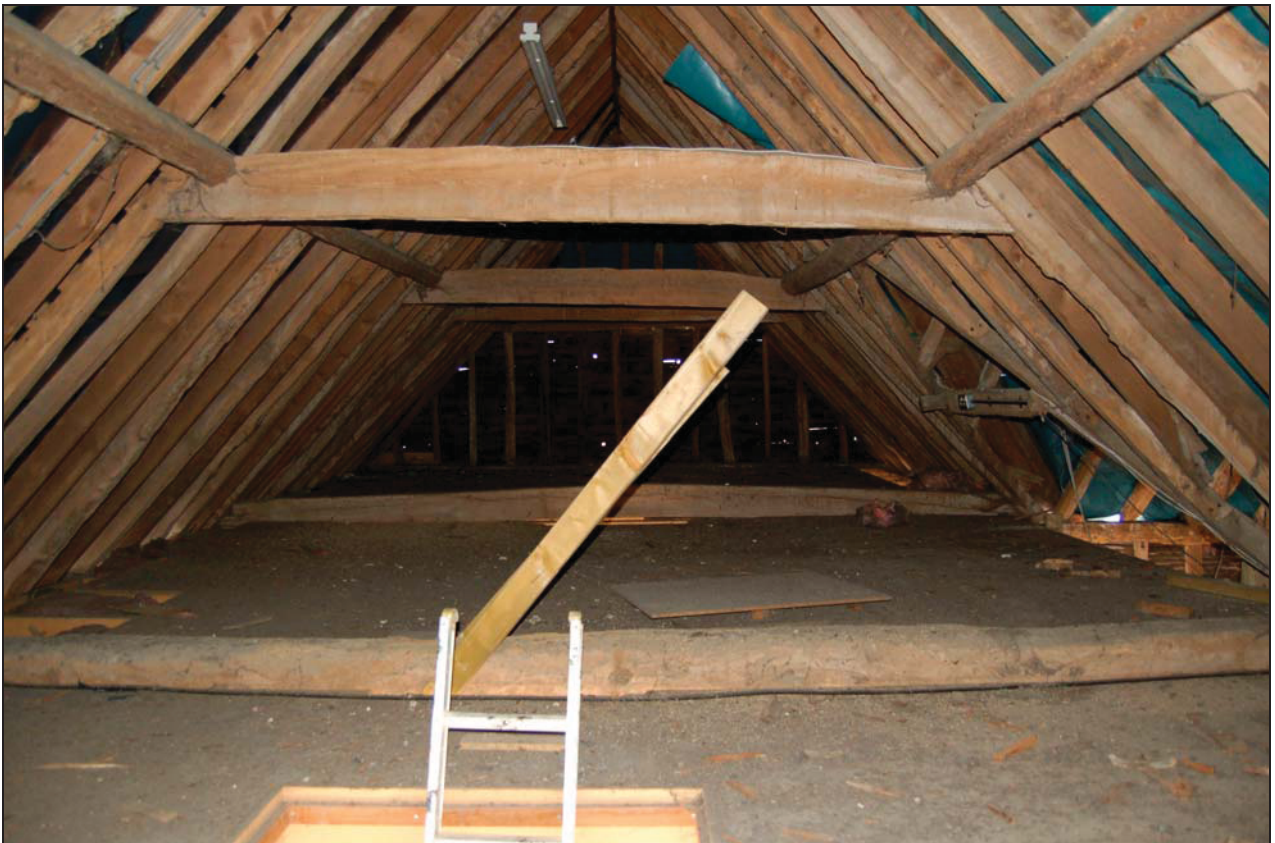
Plate 10 Roof frame in barn 1, viewed to west
