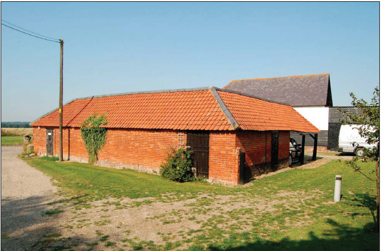
Plate 14 Brick range 3 viewed to north
