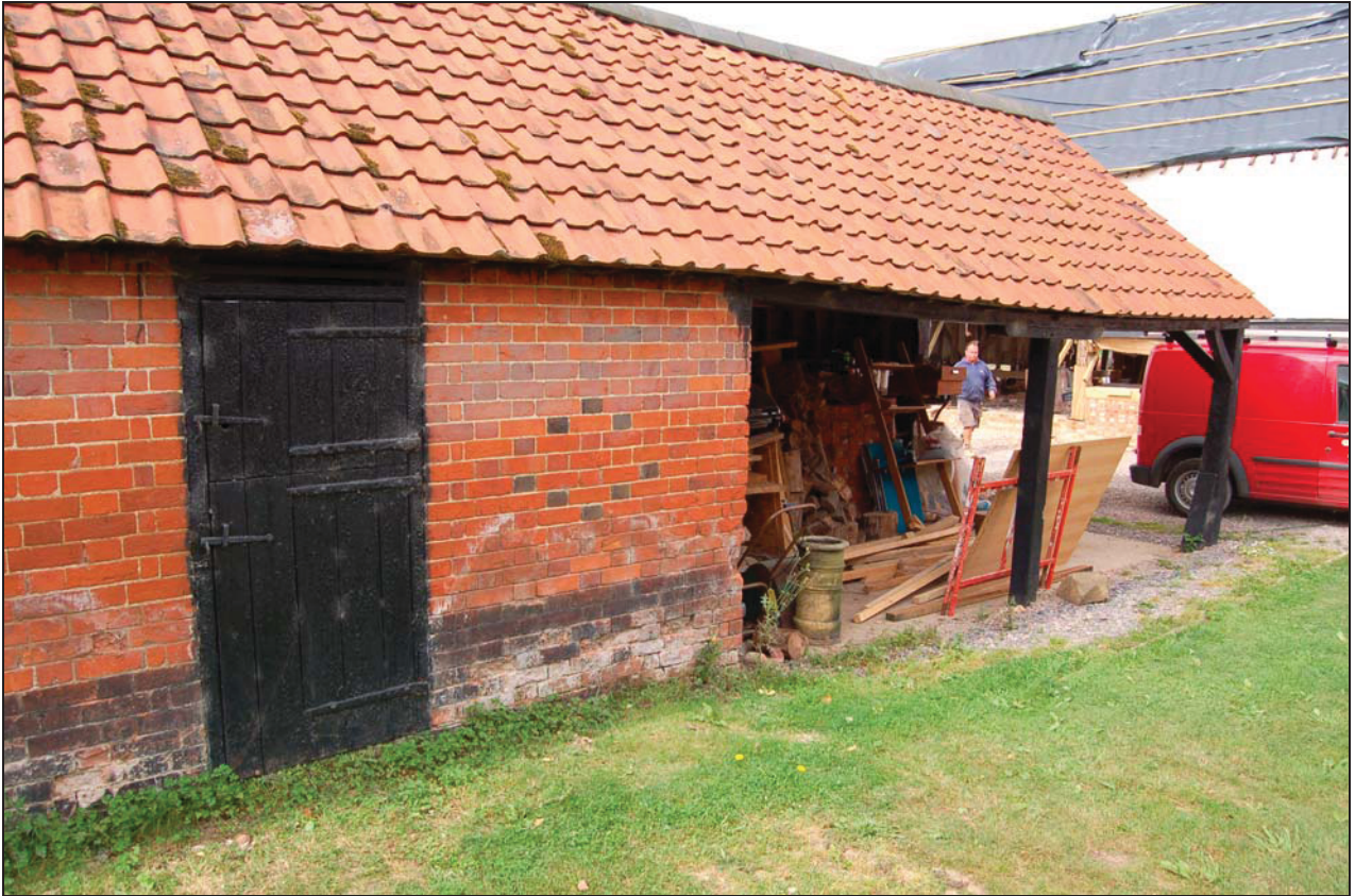
Plate 17 Typical doorway on eastern side of range and diamond patterned brickwork
