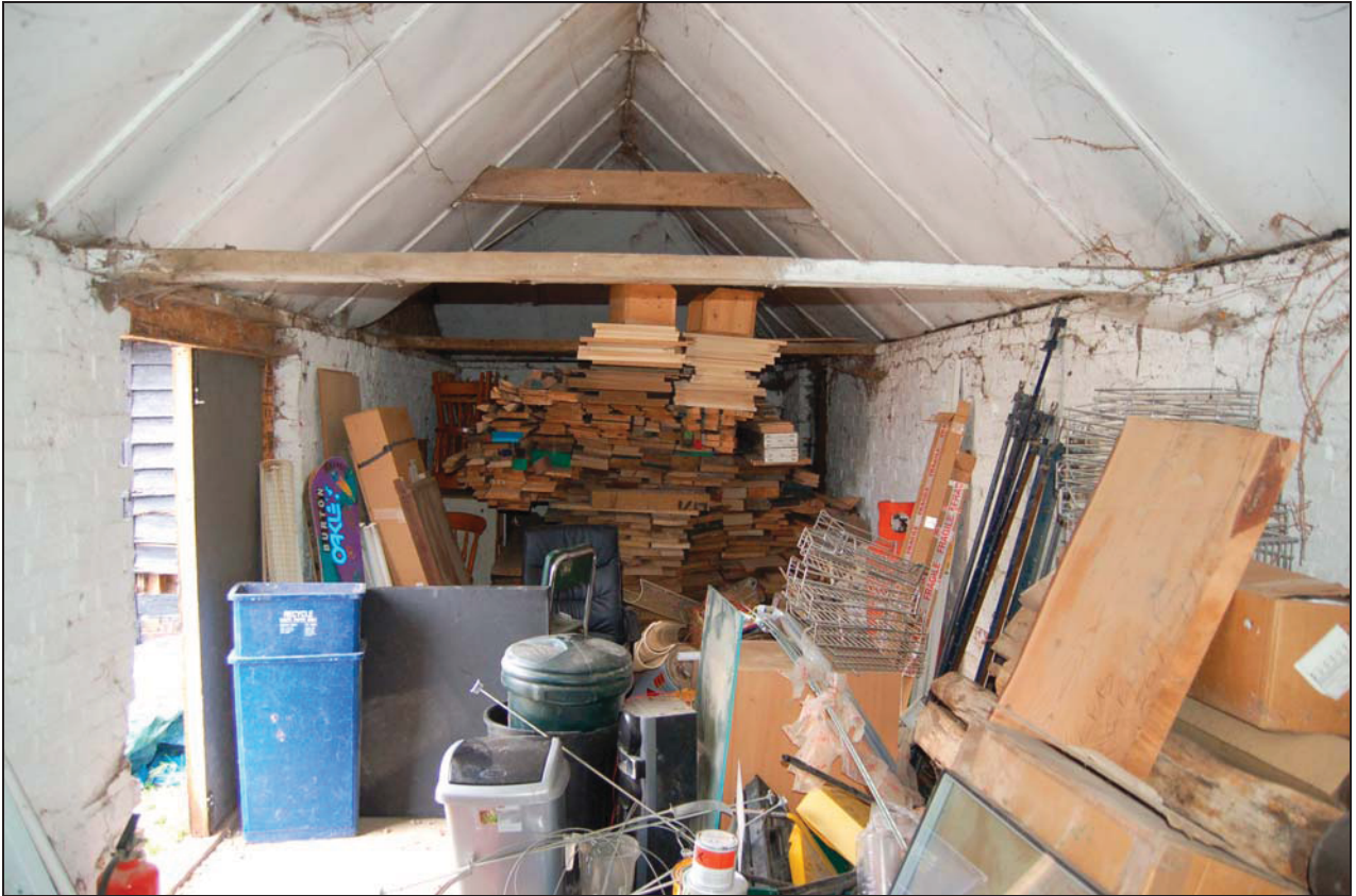
Plate 19 Interior of cowhouse viewed to east
