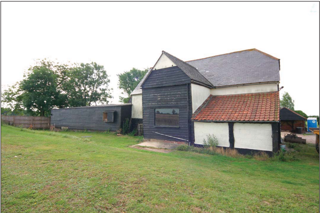
Plate 2 Barns 1 & 2 viewed to south-east
