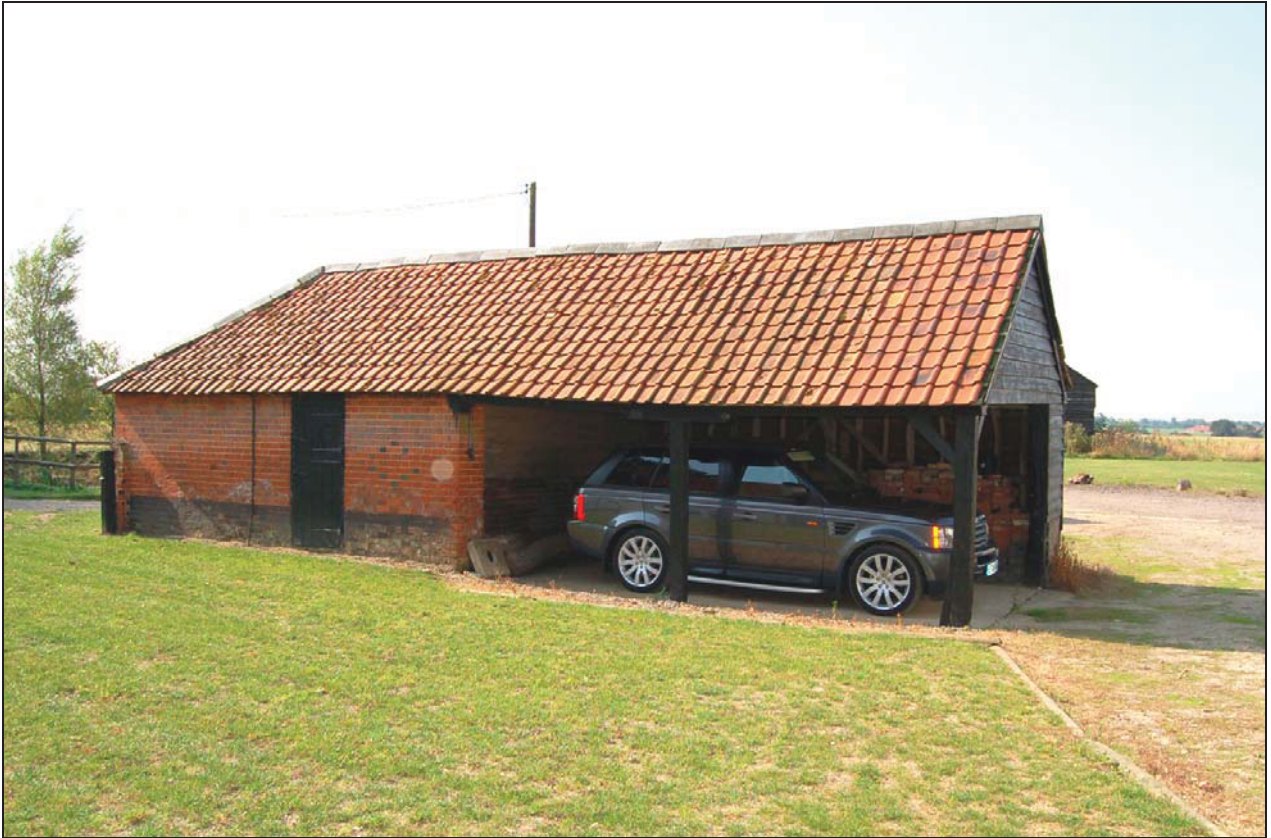
Plate 15 Loose box and shed viewed to west
