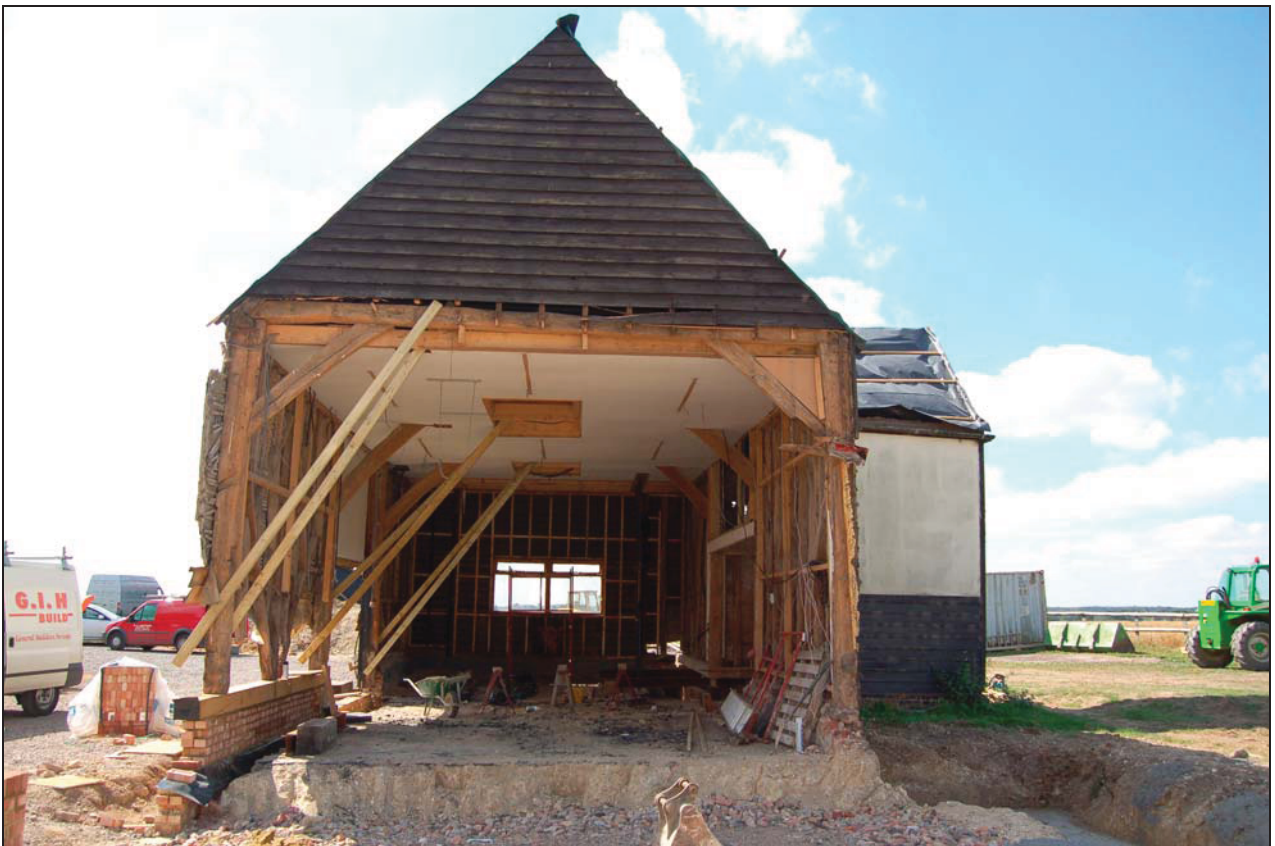
Plate 8 East end of barn 1, after barn 2 demolition
