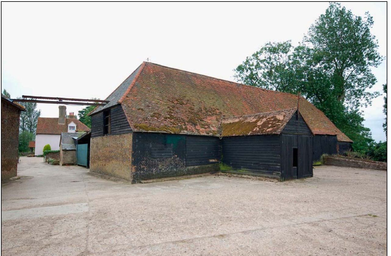
Plate 2 Barn viewed to south
