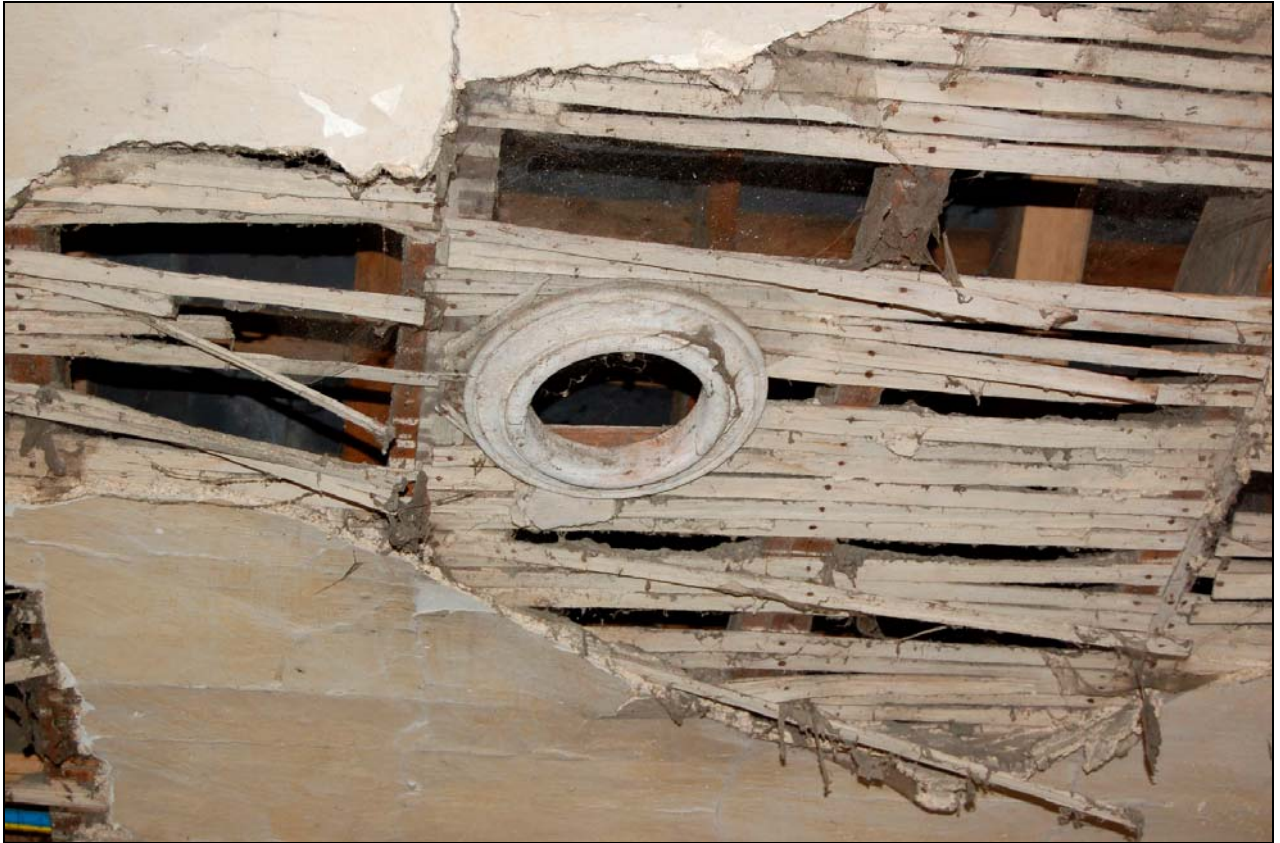
Plate 21 Ceiling vent inside tackroom
