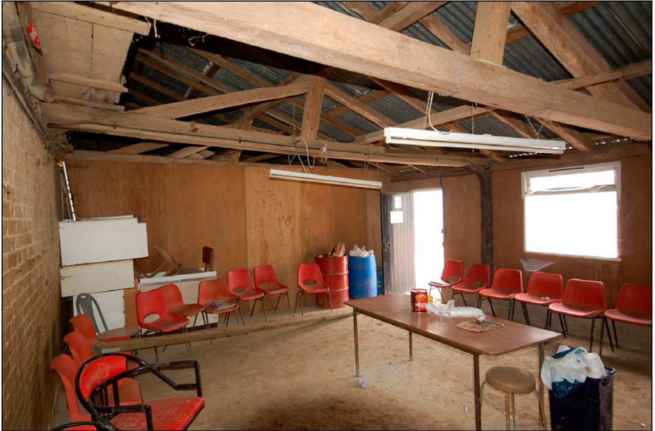
Plate 23 Mess room inside former cart shed
