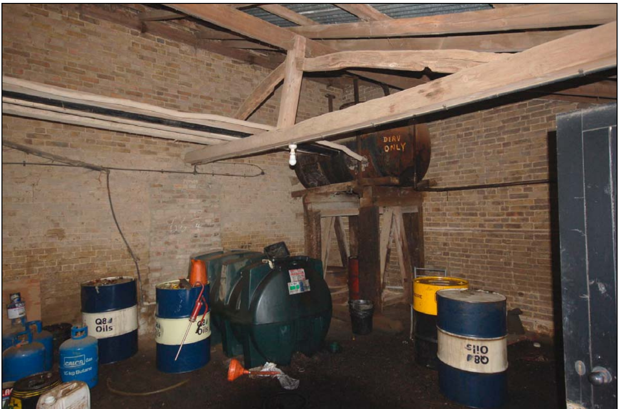
Plate 24 Diesel shed inside former cart shed
