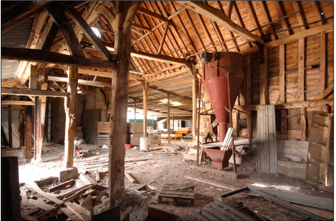
Plate 9 Aisle framing and extant southern wall of barn
