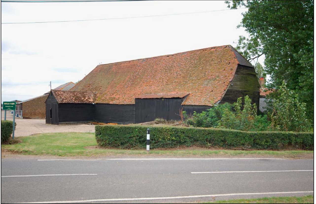
Plate 1 Barn viewed to south-east
