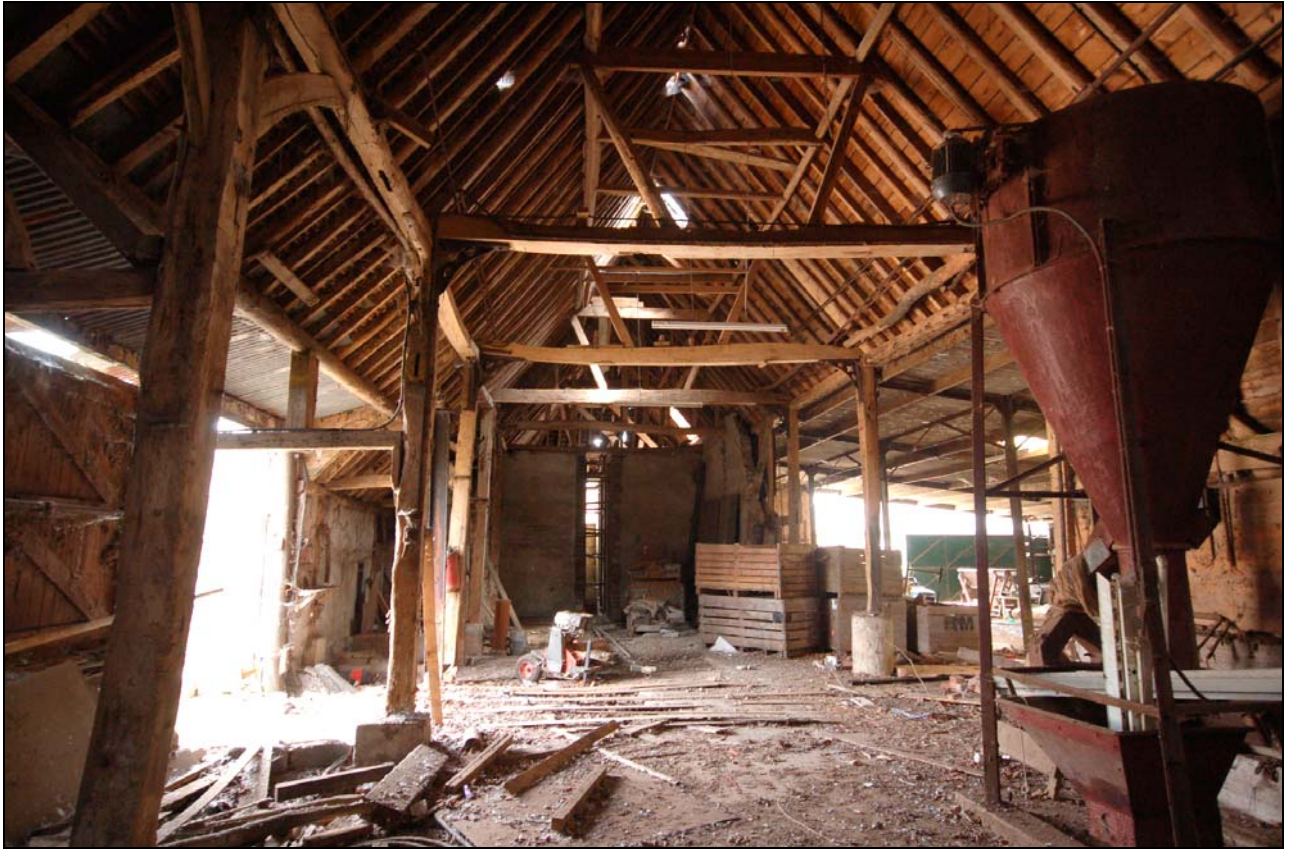
Plate 7 Interior of barn viewed to east
