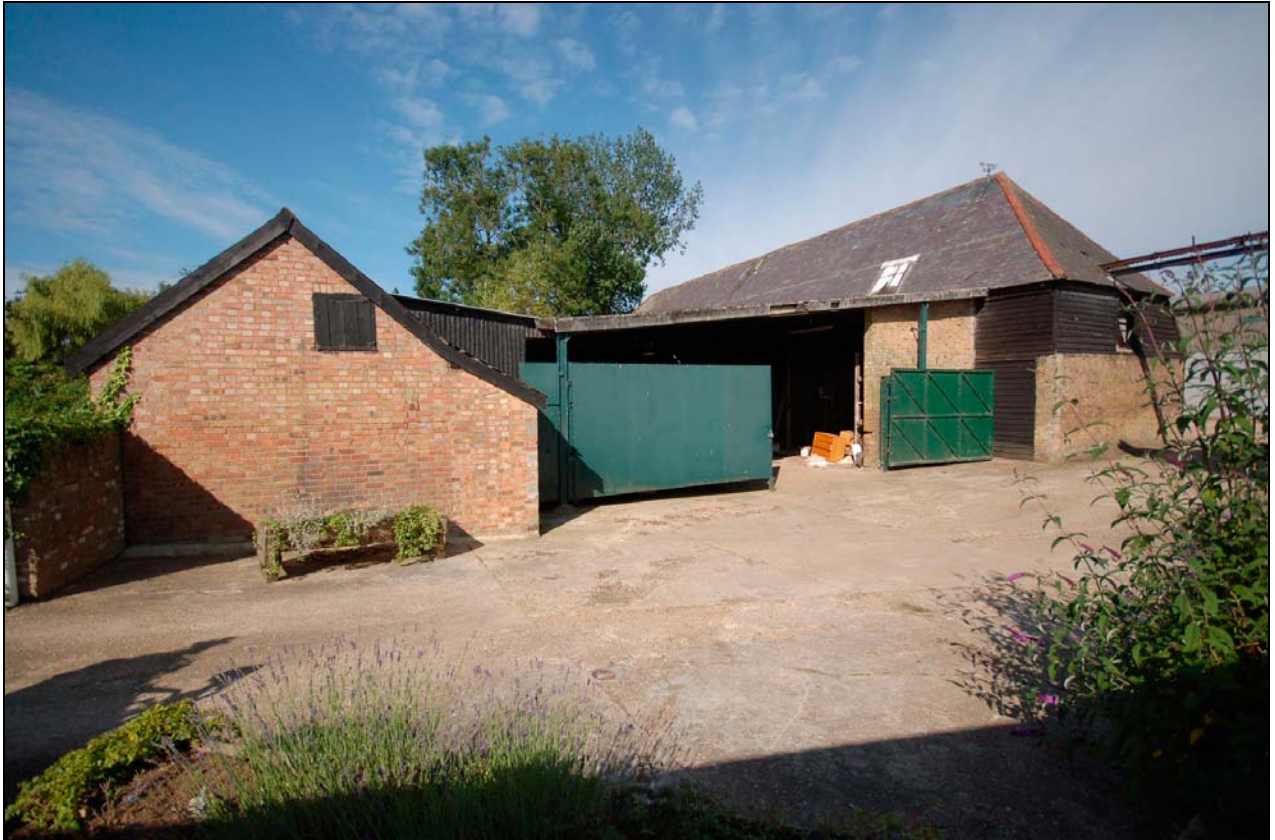
Plate 3 Rear of barn and covered yard viewed to north
