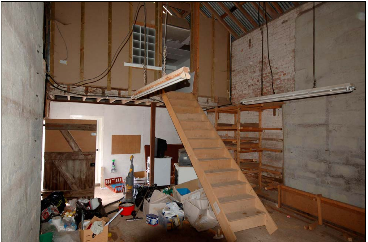
Plate 16 Interior of granary viewed to west
