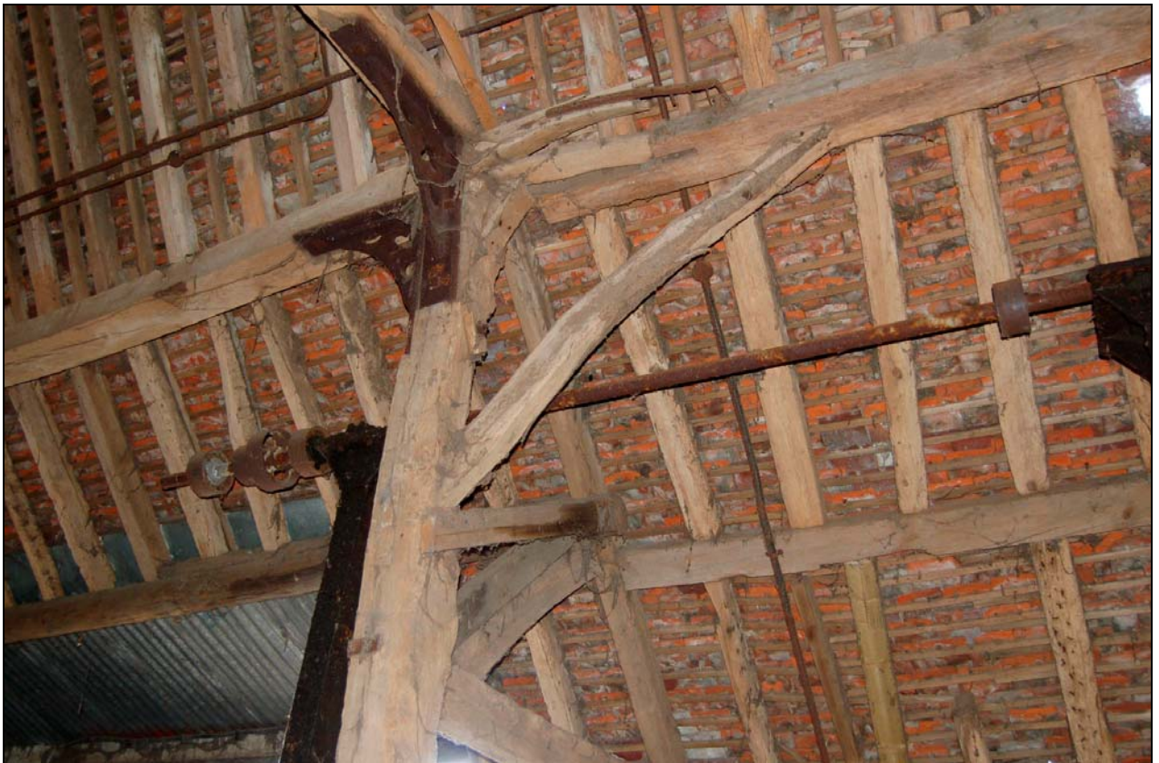
Plate 8 Detail of bladed scarf joint and aisle roof
