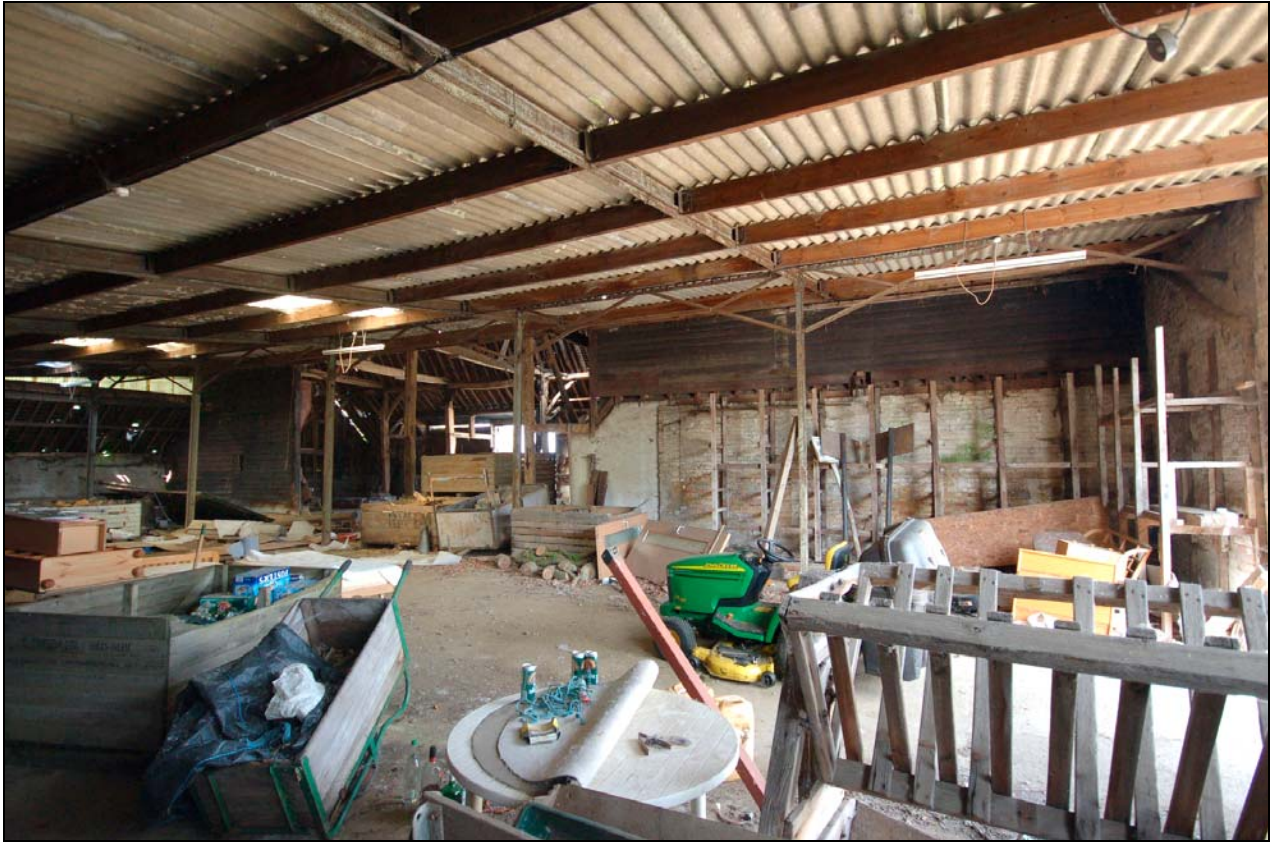
Plate 5 South wall of barn viewed to north-west
