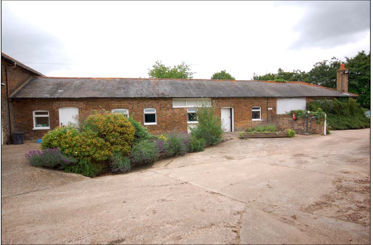
Plate 17 Stable viewed across former yard to east
