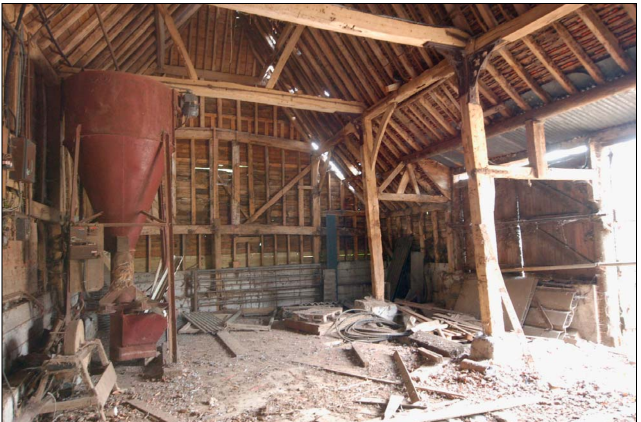
Plate 10 Partially-rebuilt western wall
