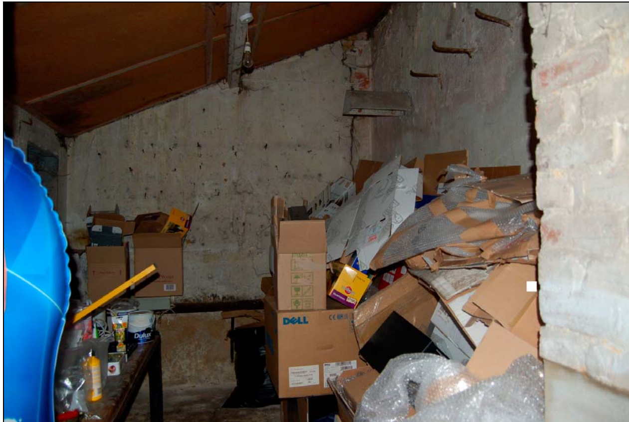
Plate 8 Interior of harness room 2 viewed to west
