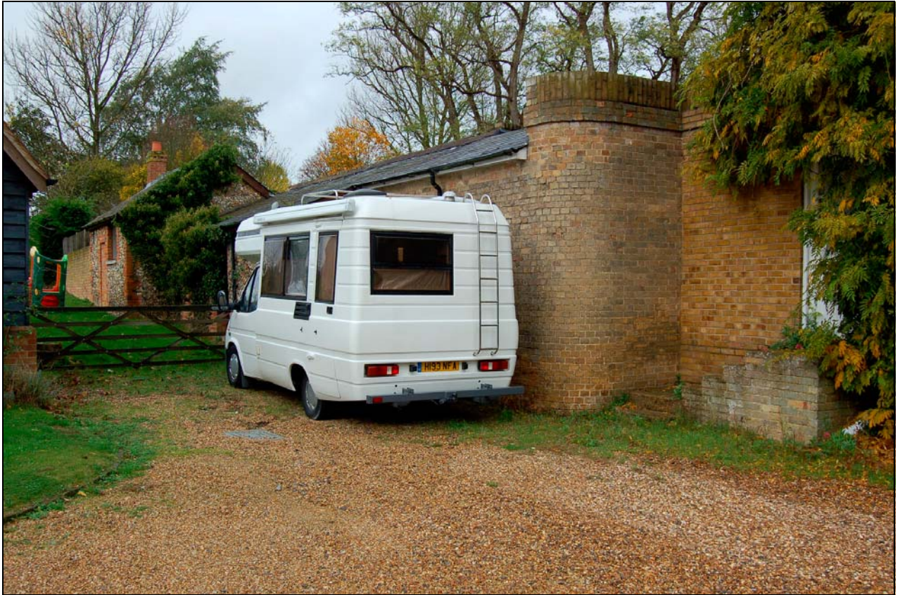
Plate 3 Utility room and outbuilding range viewed to west, along former farm track
