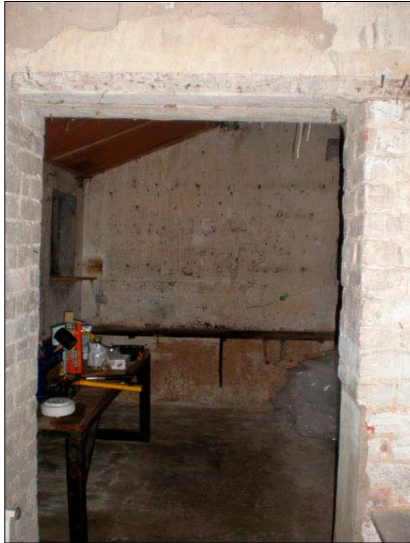
Plate 6 Interior of harness room 2, viewed to west
