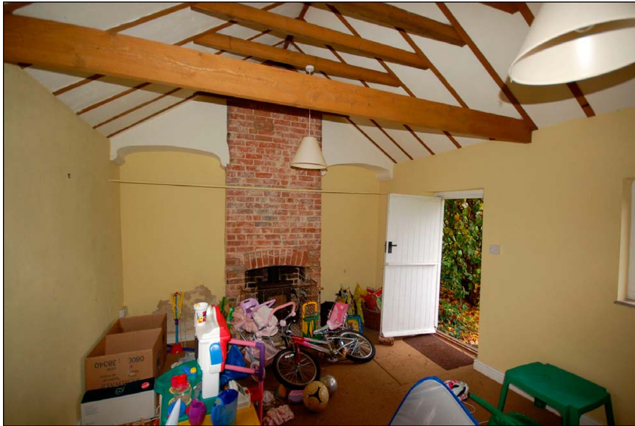
Plate 10 Schoolroom interior viewed to west
