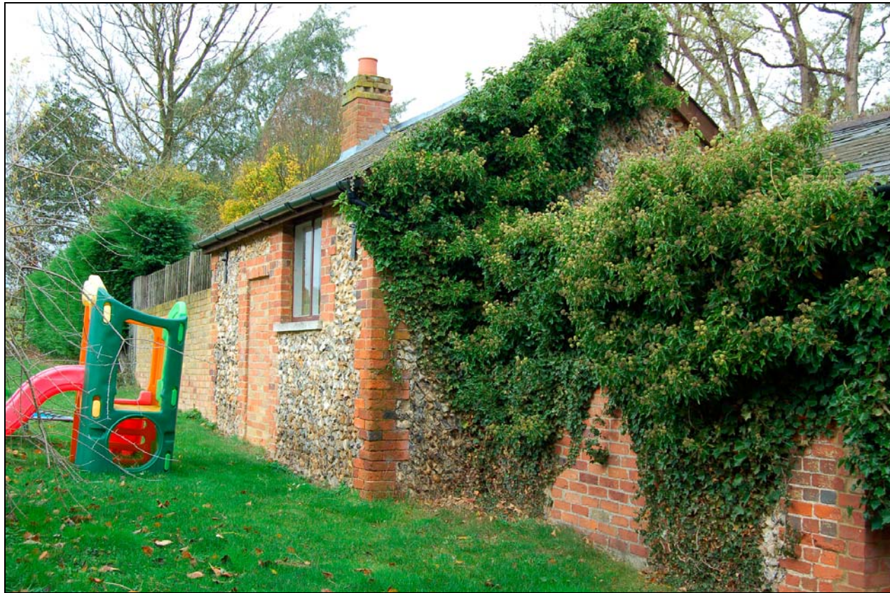
Plate 9 South elevation of schoolroom, viewed to west
