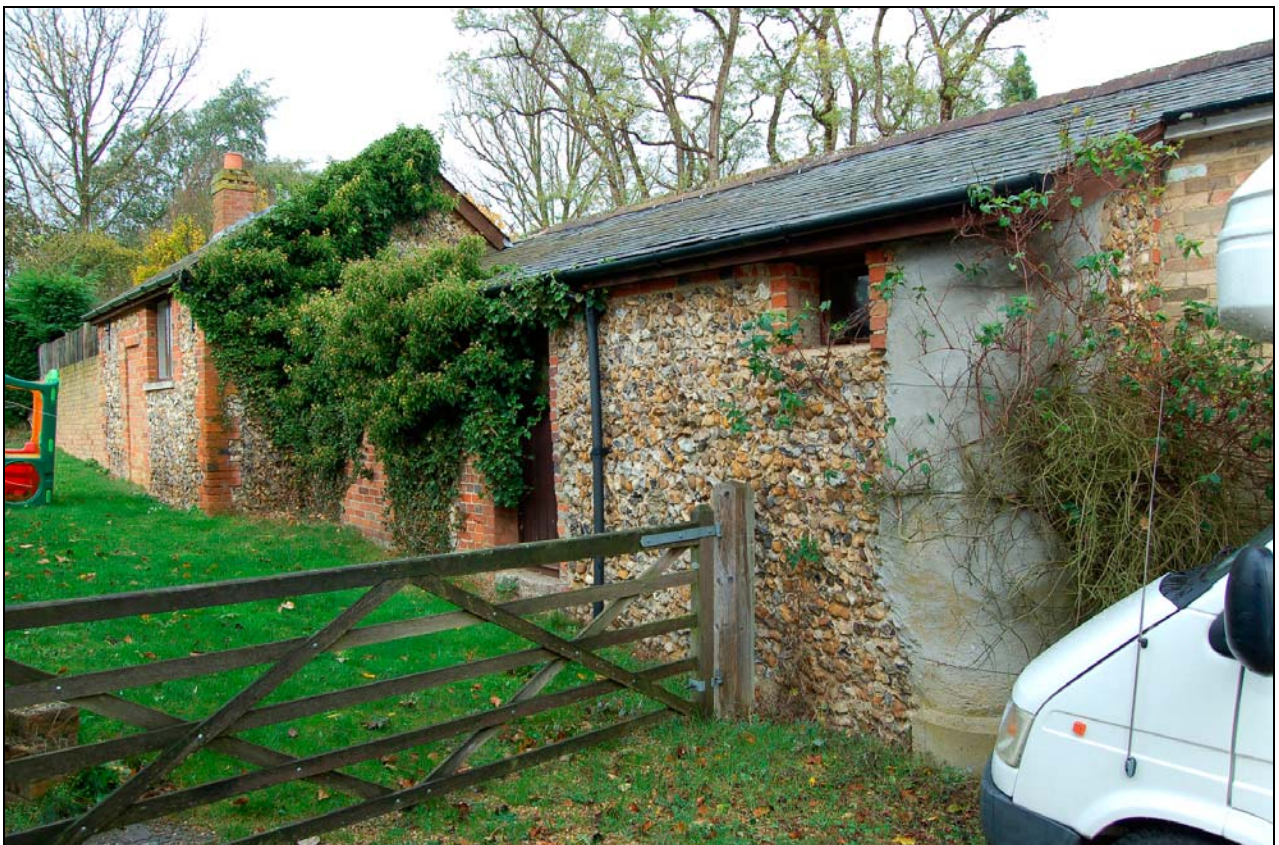
Plate 4 Former dairy, harness room and schoolroom viewed to west
