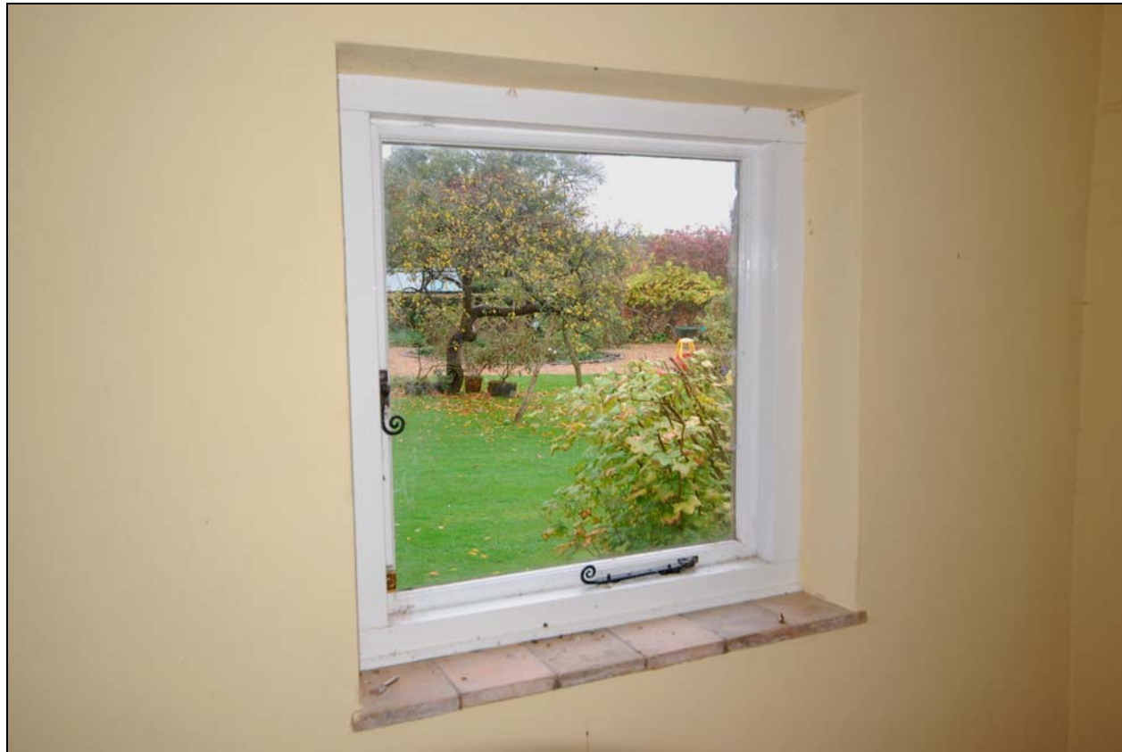
Plate 11 Typical replacement window (in schoolroom)
