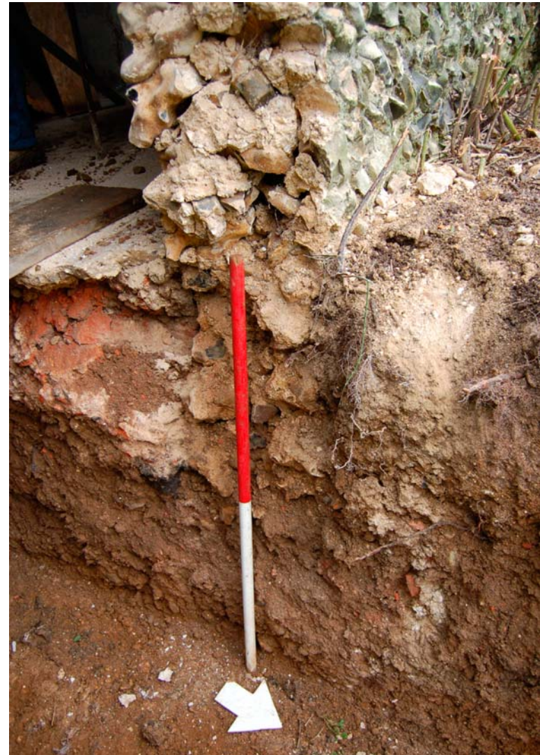
Plate 14 Northern wall of former dairy building (1m scale)
