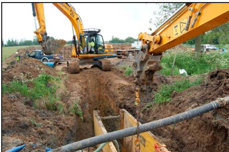
Plate 3. Excavation of the pipe trench across the Boreham Brook, looking west
