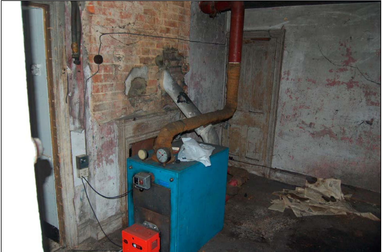
Plate 7 Interior of boiler room
