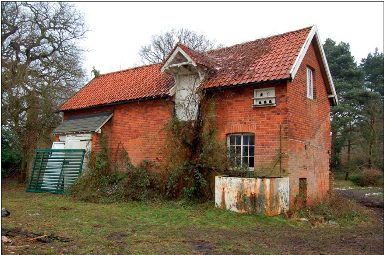
Plate 28 Stable viewed from south-west
