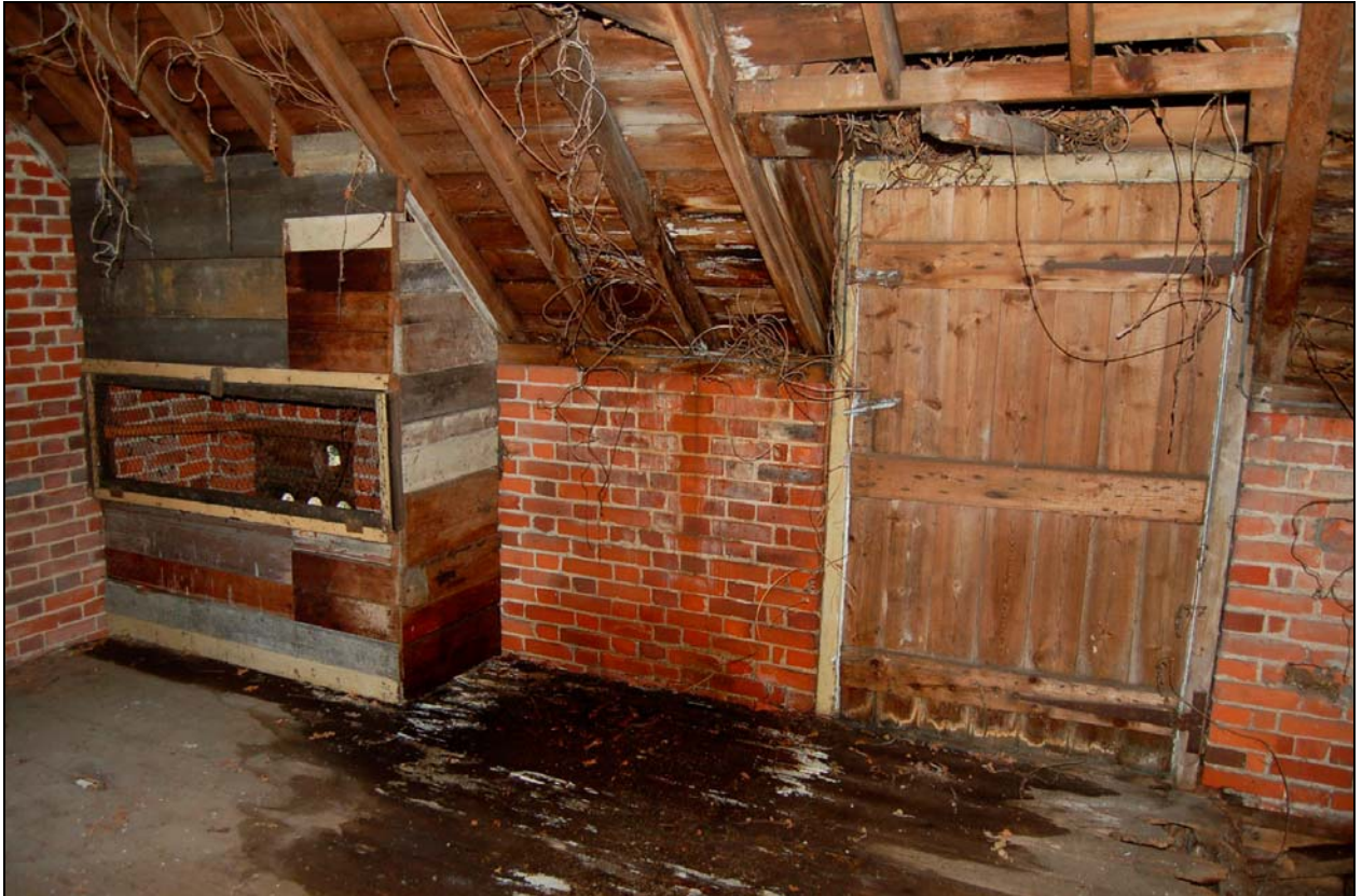
Plate 35 Dovecote and taking-in door at south end of hay loft
