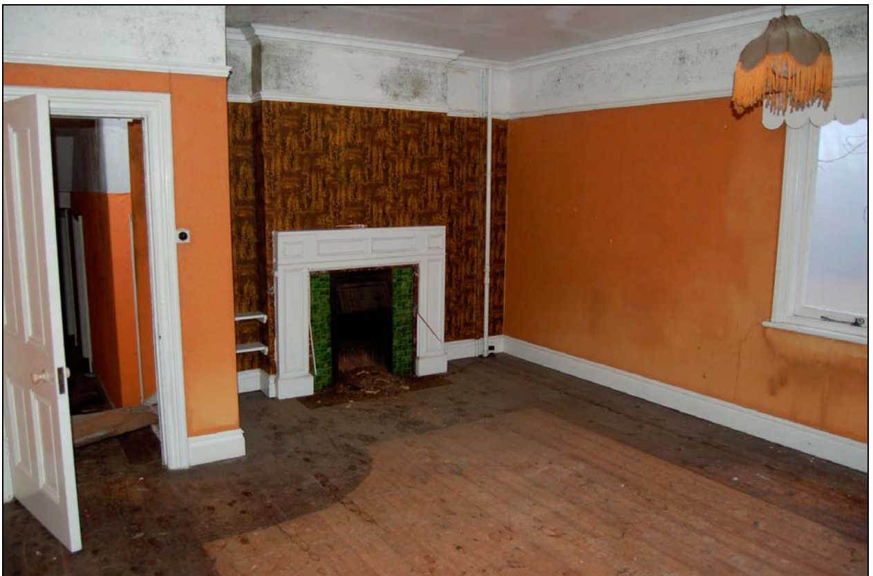
Plate 24 Surviving fireplace in bedroom 2
