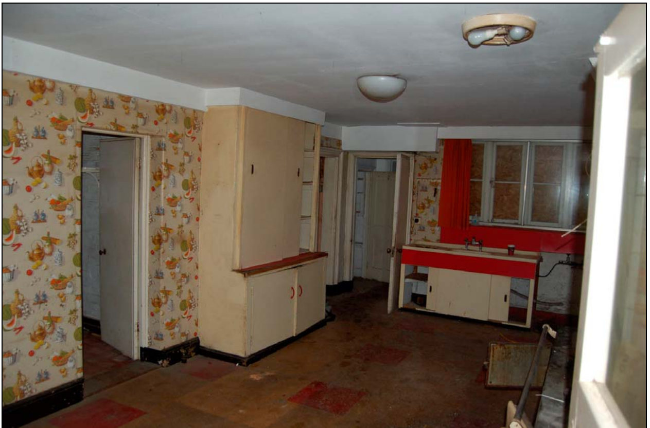
Plate 8 Kitchen viewed to east
