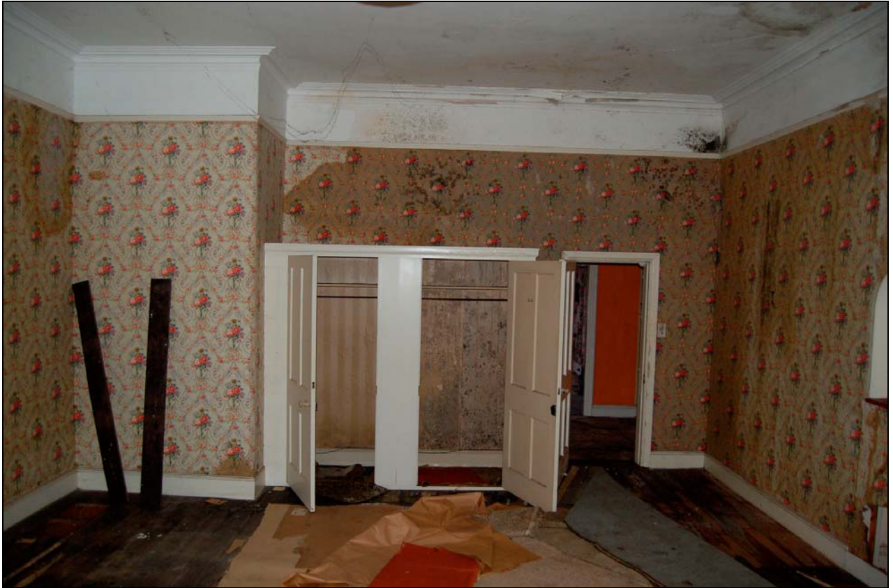
Plate 23 Fixtures in bedroom 1
