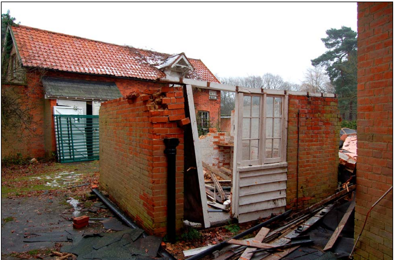
Plate 36 Remains of store room 3 viewed to east
