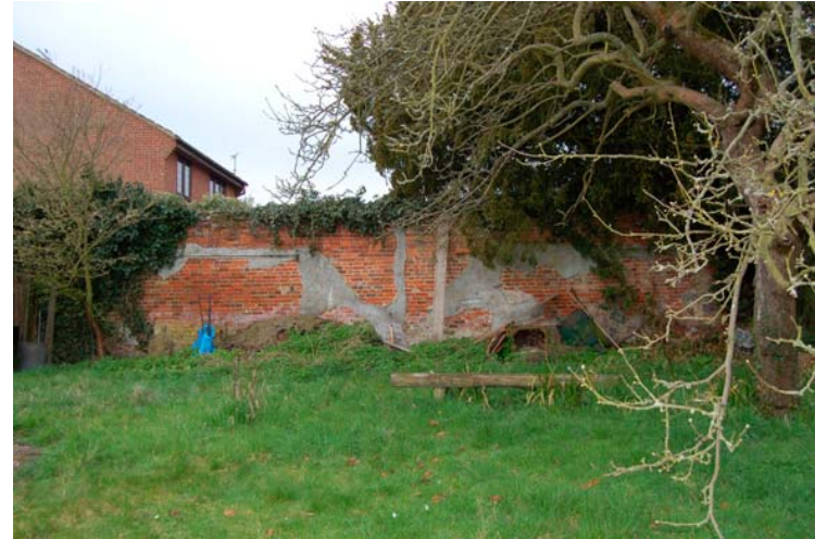
Plate 6. Rear boundary wall, looking south.
