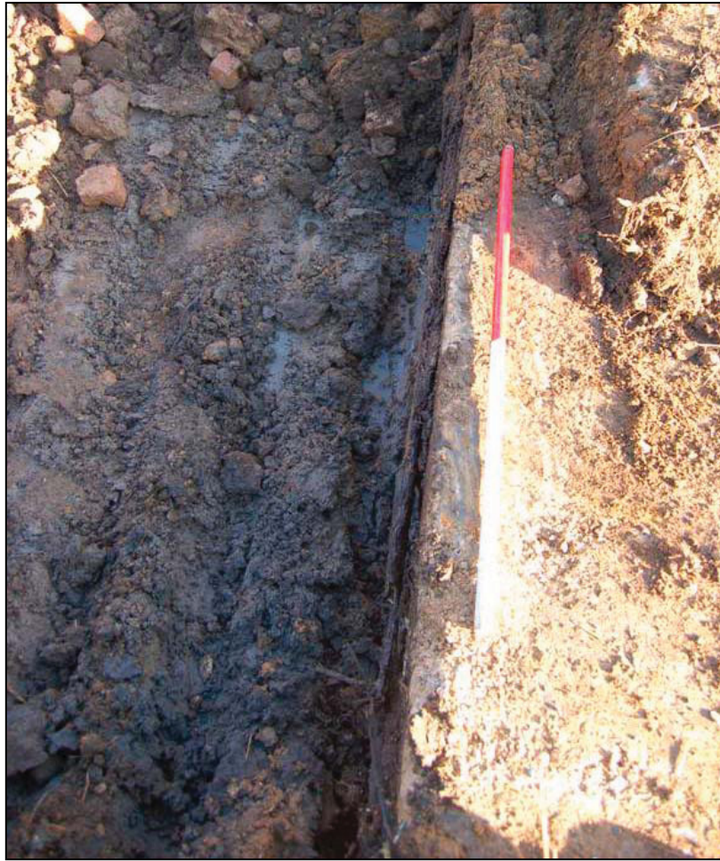
Plate 1. Wooden shuttering in test-pit 1 (1m scale)
