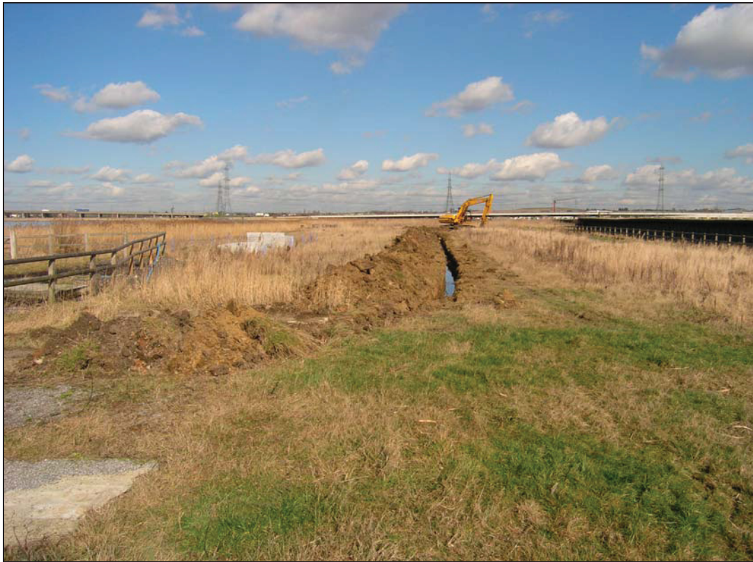
Plate 3. Southern end of electricity cable trench, looking north
