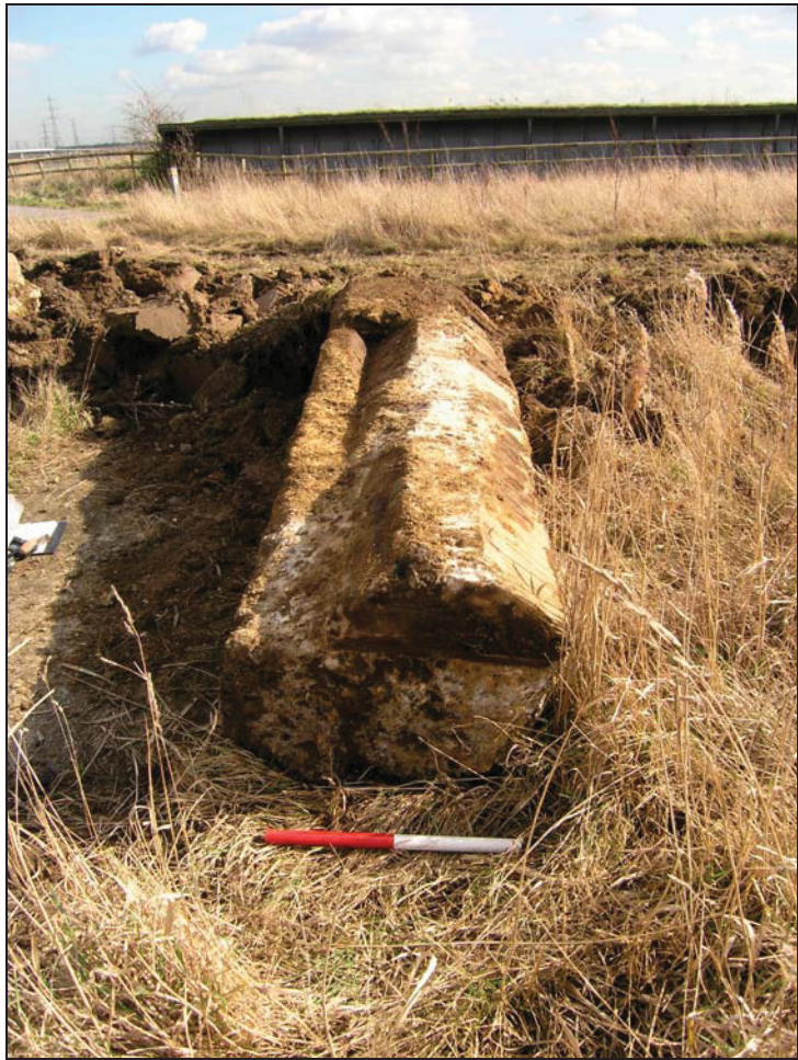
Plate 5. Removed section of concrete sill (0.5m scale)
