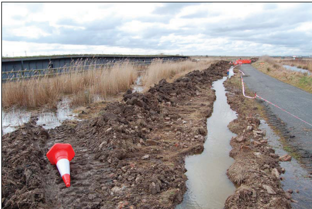
Plate 6. Northern end of electricity cable trench, looking south
