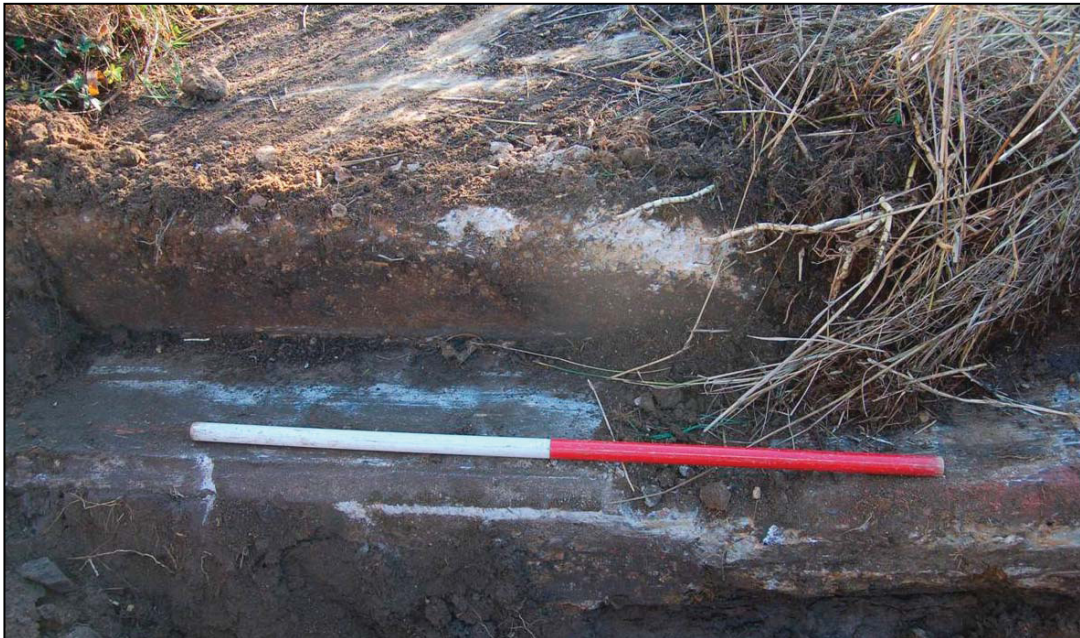
Plate 2. Chamfered edge of concrete raft in test-pit 2 (1m scale)
