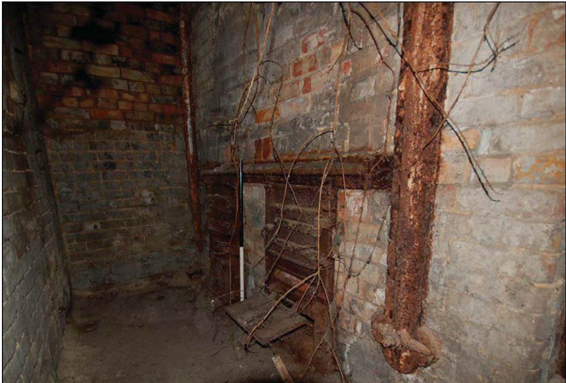
Plate 16 Fire boxes at back of oven (1m scale)
