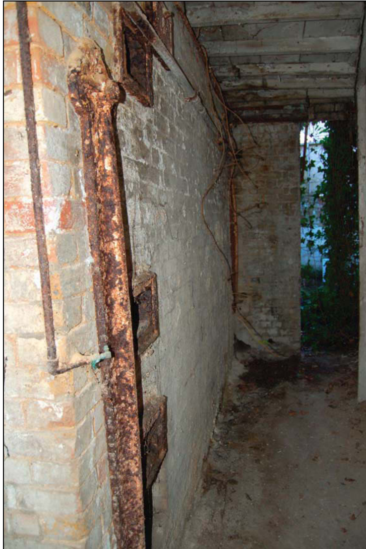
Plate 13 Passage viewed to north-west
