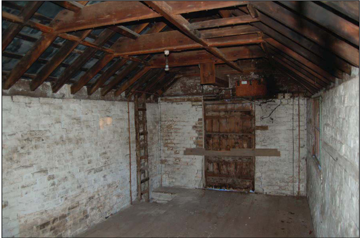
Plate 21 First floor viewed to north-west (loading door)
