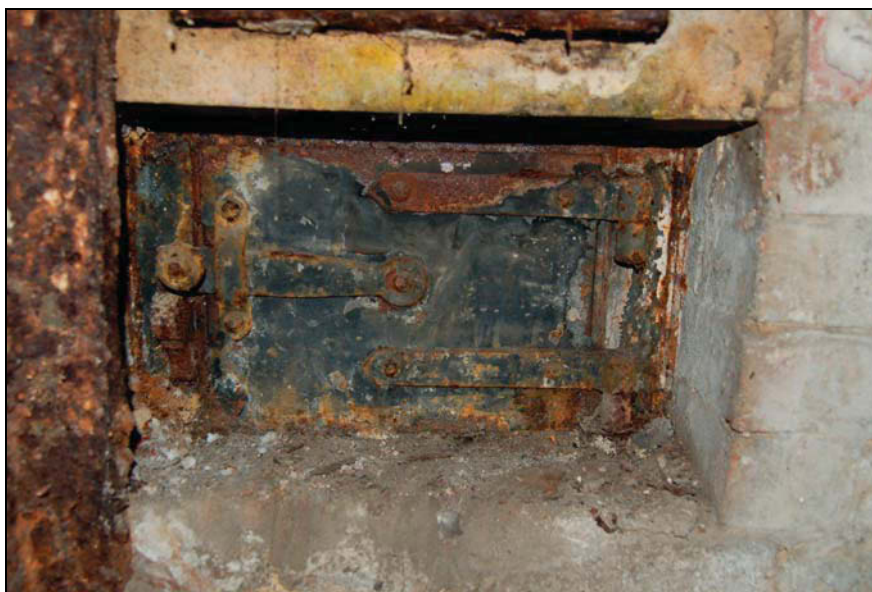
Plate 14 Inspection door at base of flue wall
