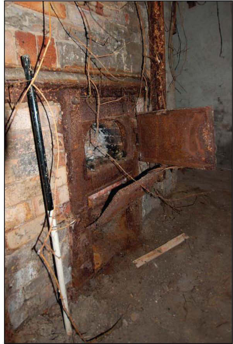
Plate 18 View inside fire box (1m scale)
