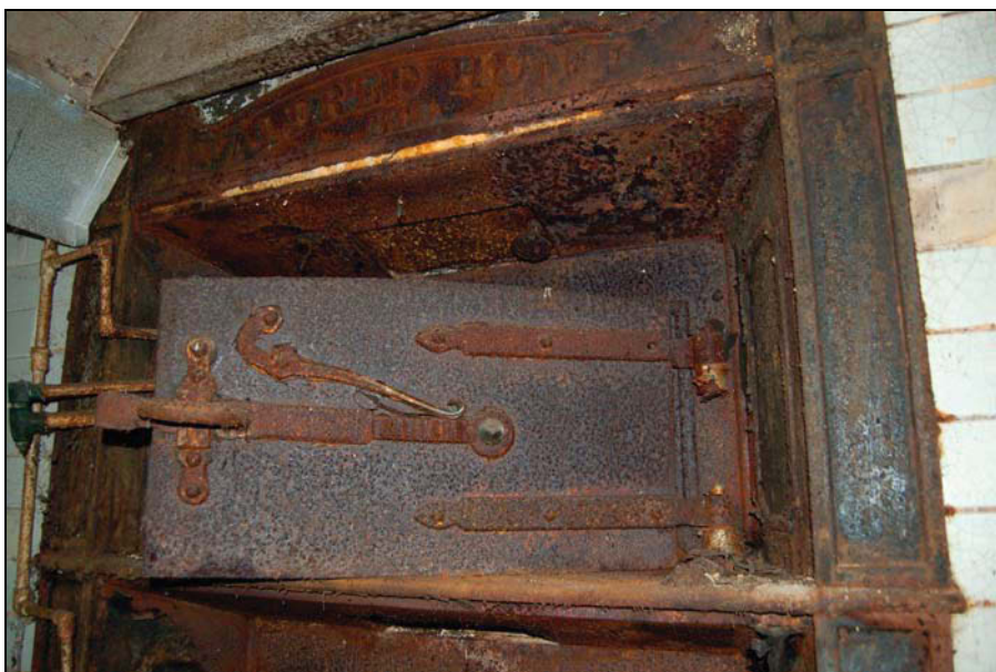
Plate 10 Door detail on oven
