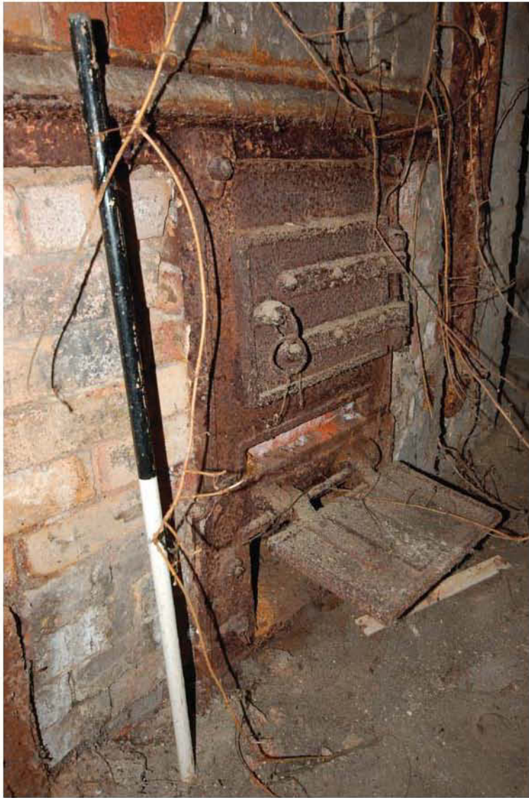
Plate 17 Detail of fire box (1m scale)
