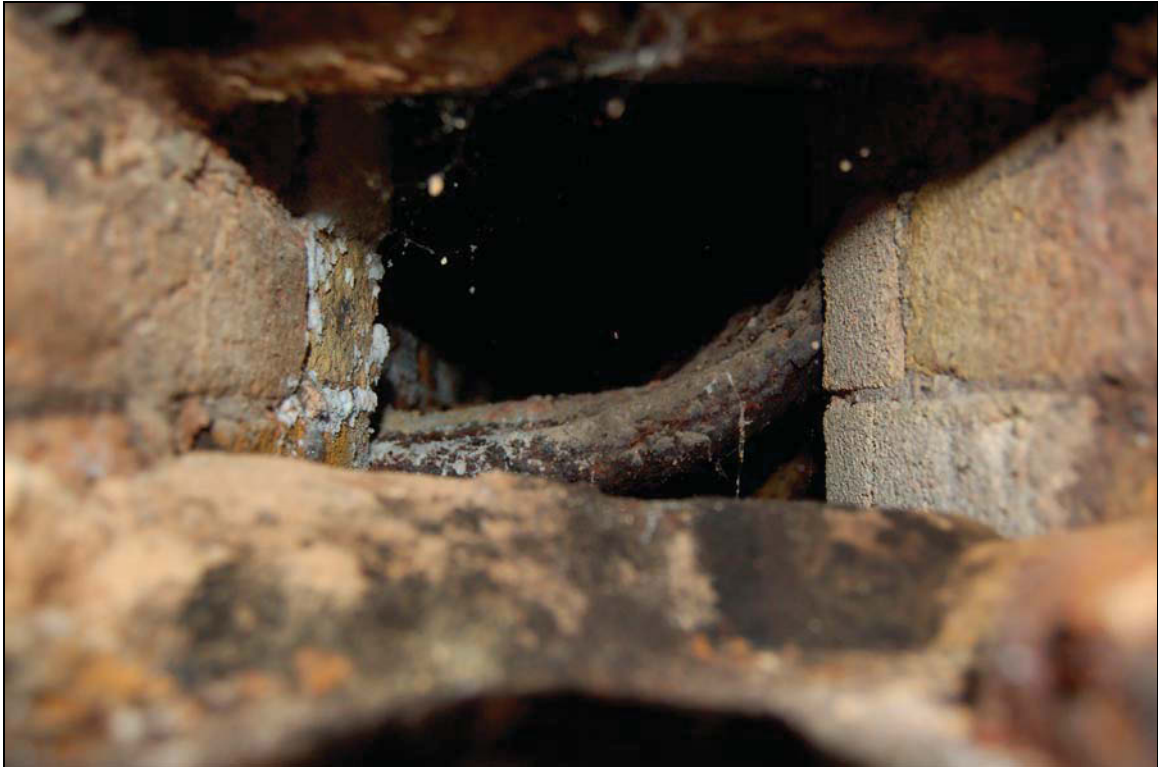
Plate 15 Heating bars in flue viewed through inspection hole
