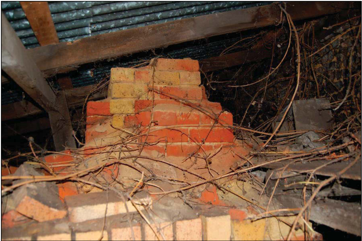
Plate 20 Remains of chimney
