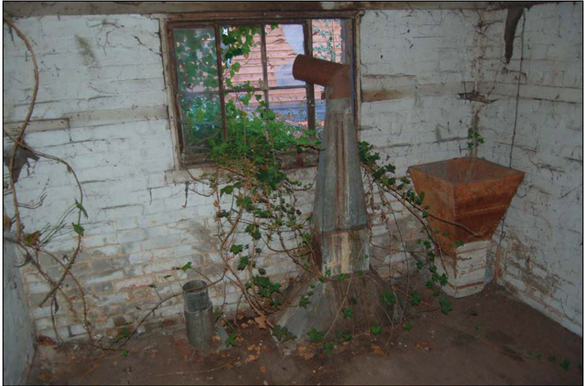
Plate 23 Flour hopper at south-east end
