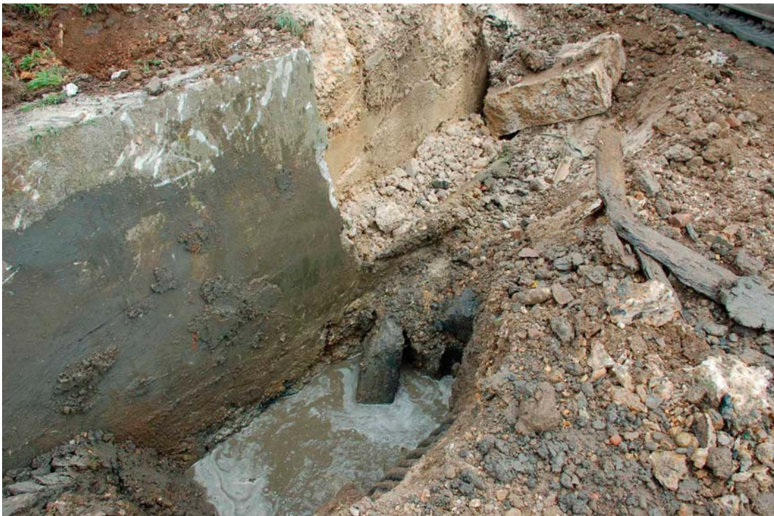
Plate 4. Wooden stake in front of northern bank abutment.
