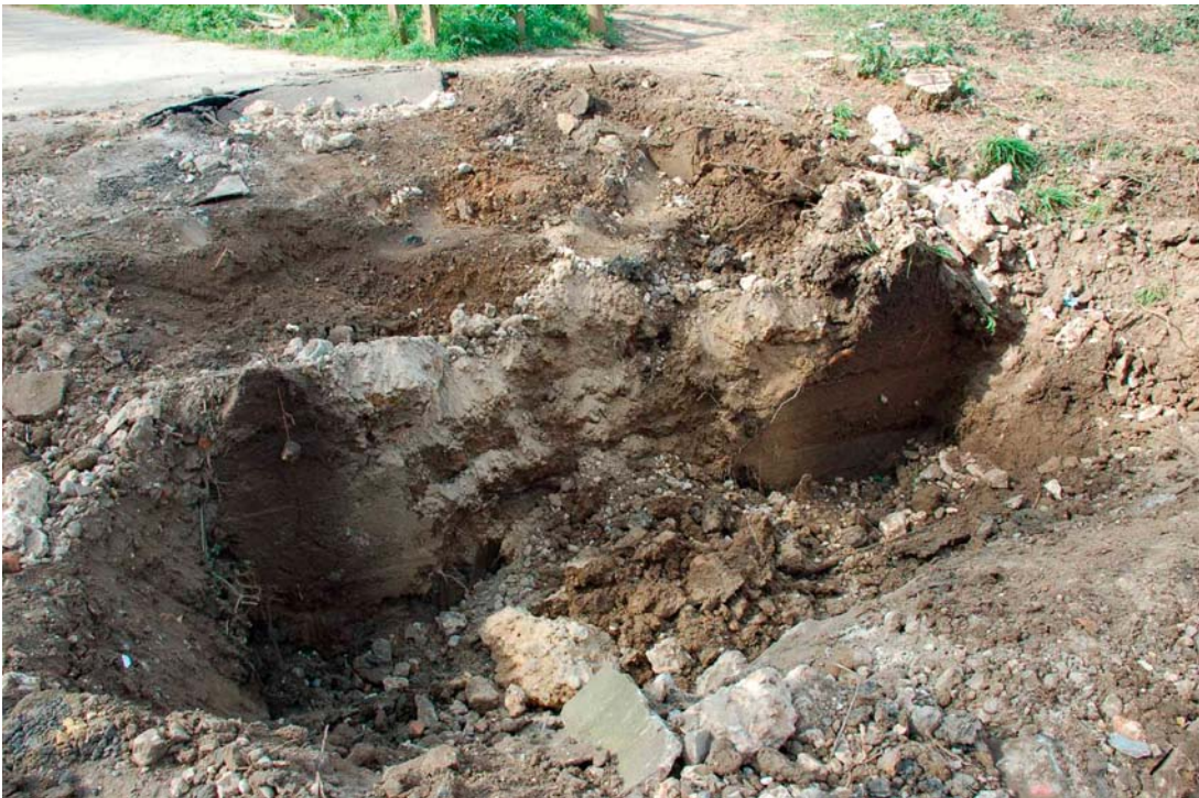
Plate 2. Southern bank after abutment removal, looking south-west.
