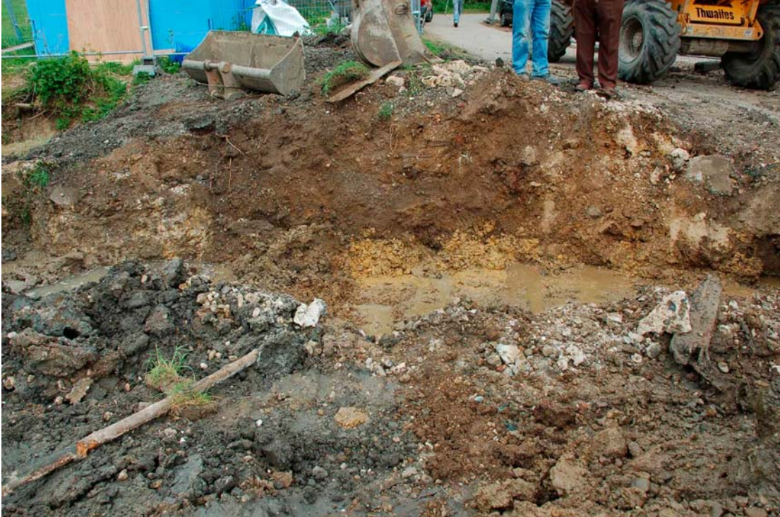
Plate 3. Northern river bank after abutment removal (infilled river channel), looking north.
