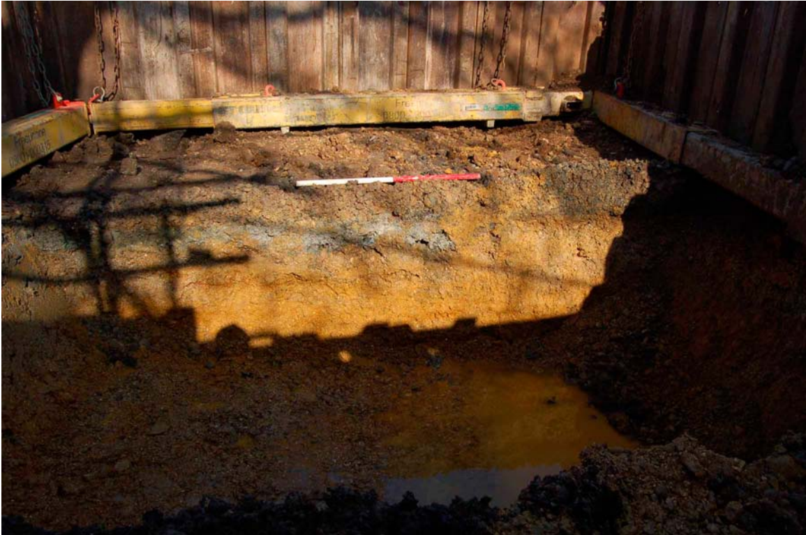
Plate 12. Northern groundworks. 1m scale.
