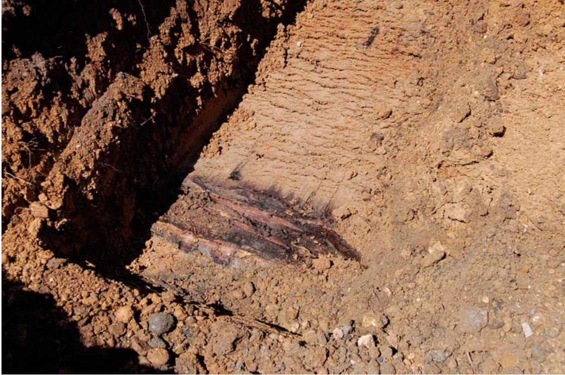
Plate 7. Exposed timber in stage 2 trench, southern groundworks.
