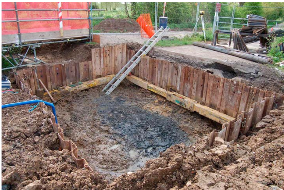
Plate 10. Southern groundworks, metal shuttering.
